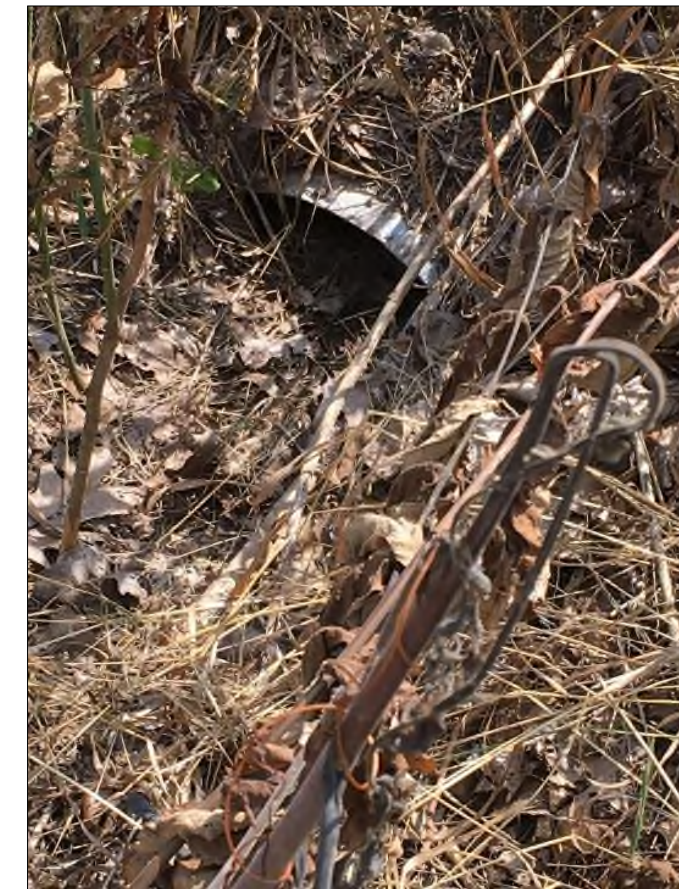
PLUGGED CULVERT
