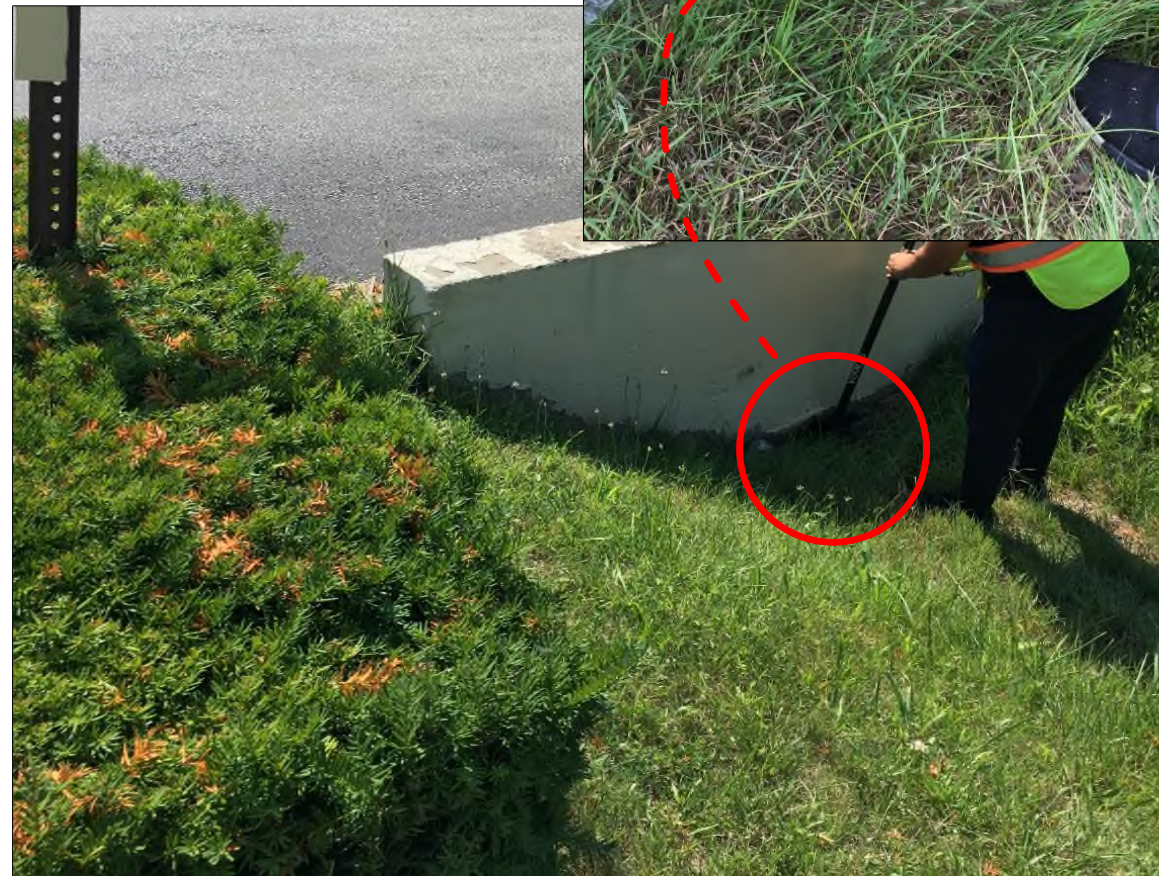
PLUGGED CULVERT
