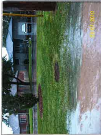
ROAD FLOODING IN LOW LYING AREAS CAUSING INFLOW INTO SANITARY SEWER MANHOLE
