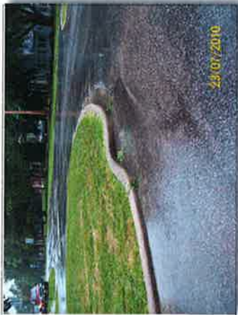
STORMWATER PONDING AT SANITARY MANHOLES
