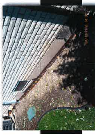
EXPOSED FOUNDATION/POOR GRADING
