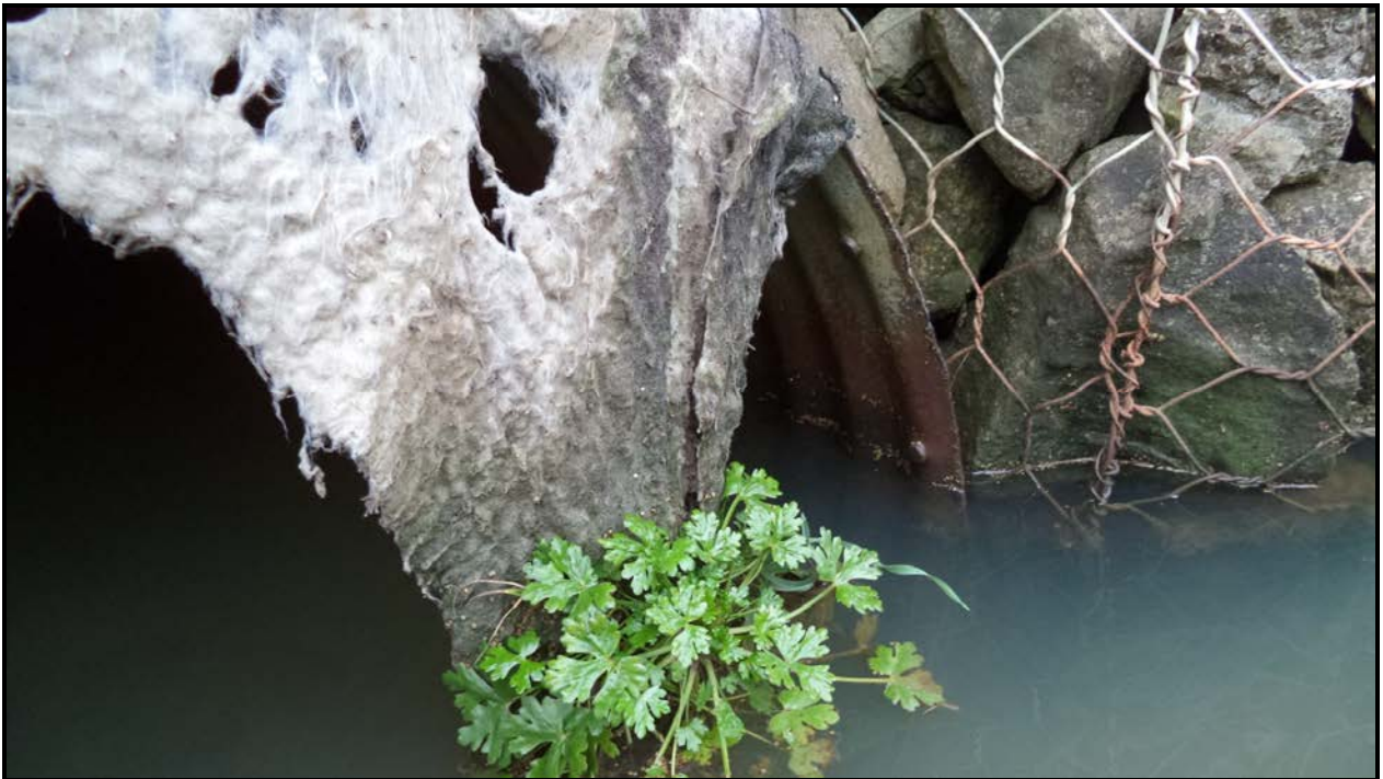
Photograph 2 – Culvert Barrel (East Elevation)
