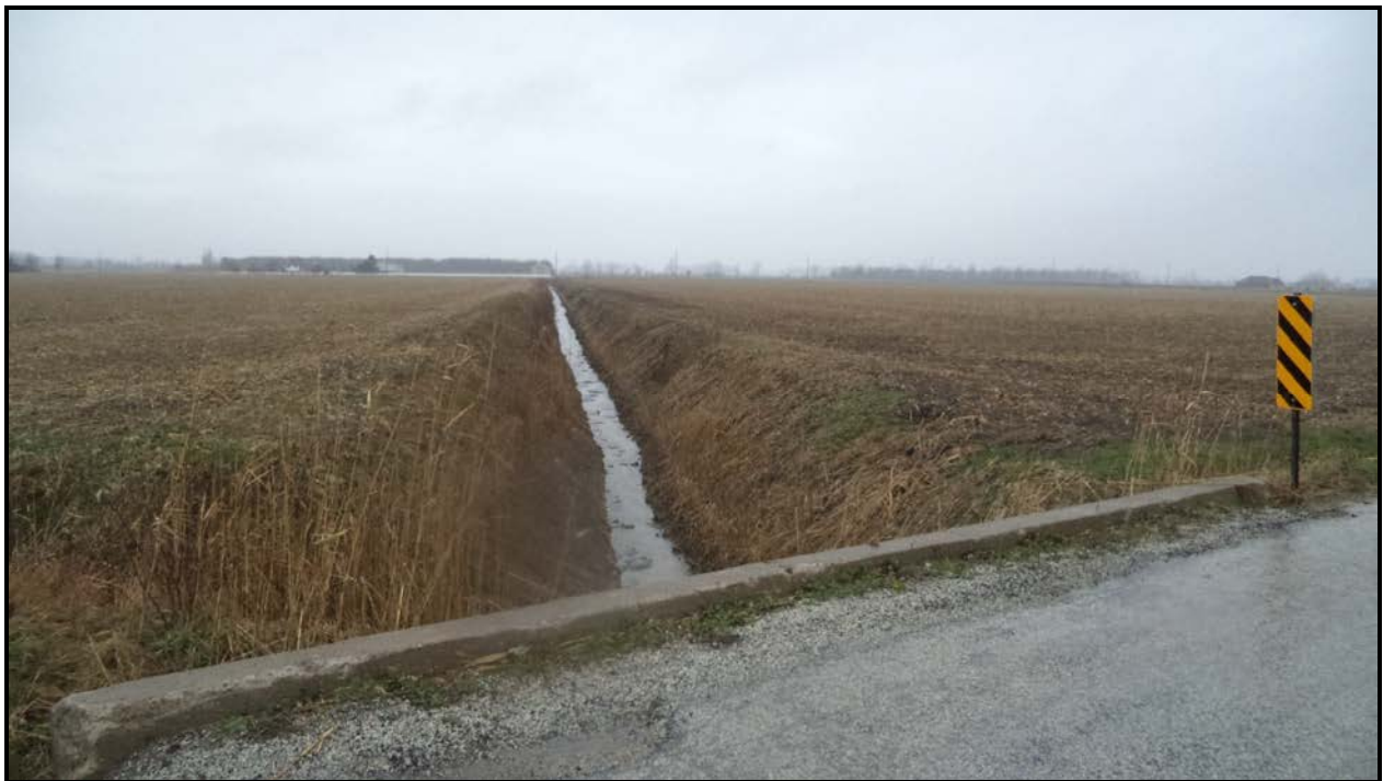
Photograph 8 –Water Stream (Snake Lane Road West Side – Looking West)
