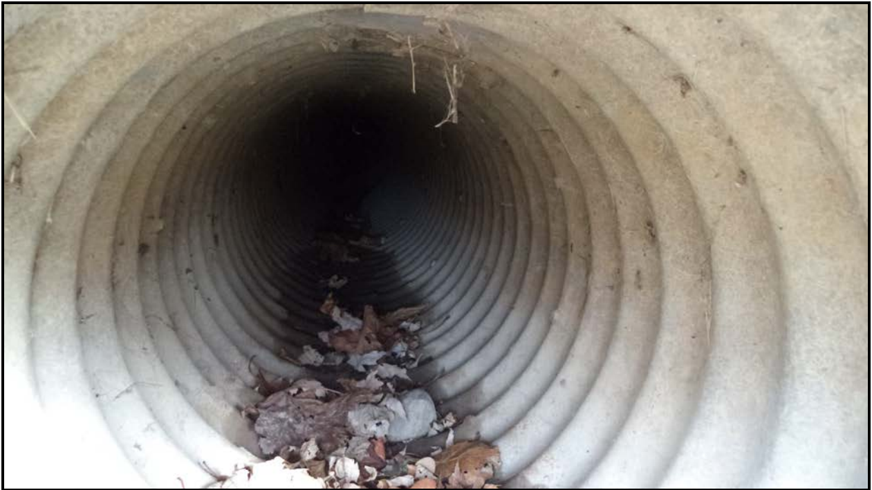
Photograph 2 – Culvert Barrel
