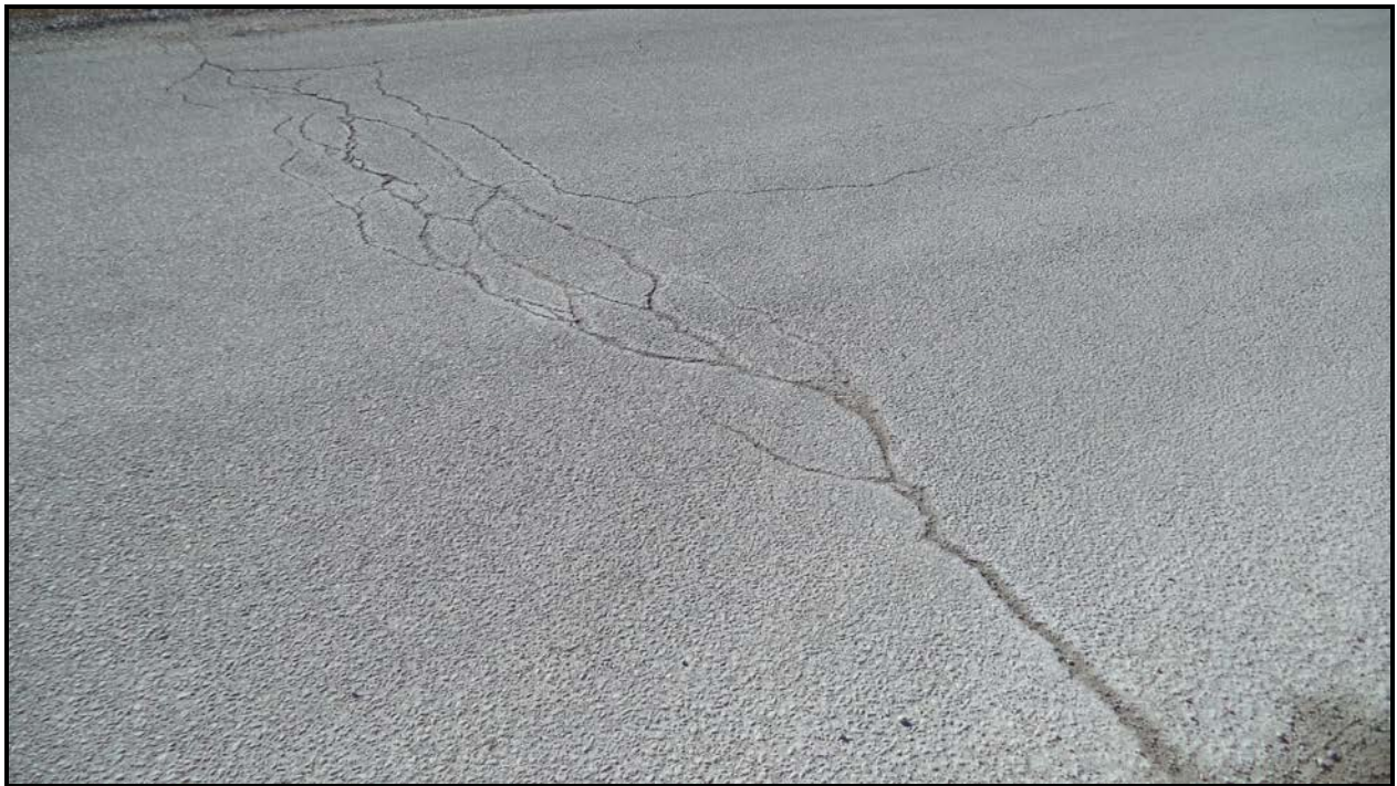
Photograph 6 – Wearing Surface at East Approach
