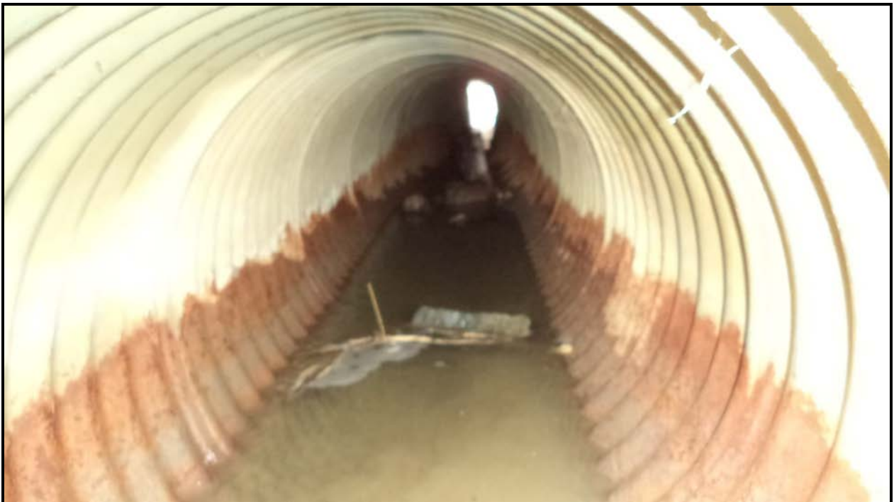
Photograph 2 – Culvert Barrel (Looking West)
