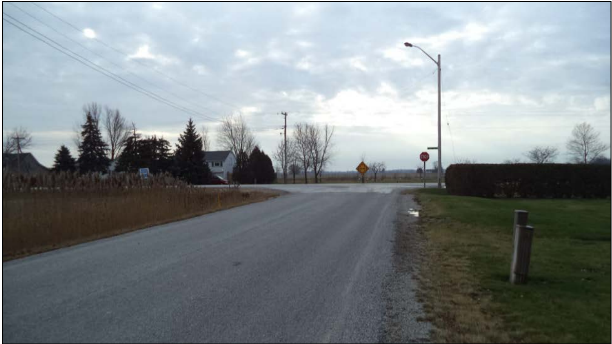
Photograph 1 – Road over Culvert (Looking South)
