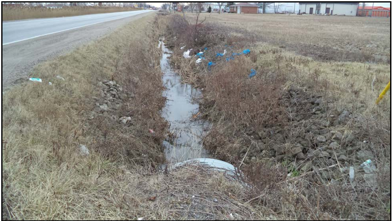
Photograph 8 – Water Stream (Manning Road West Side - Looking South)
