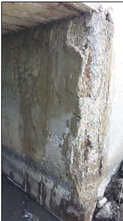
Photograph 2 – Culvert inside Boxes
