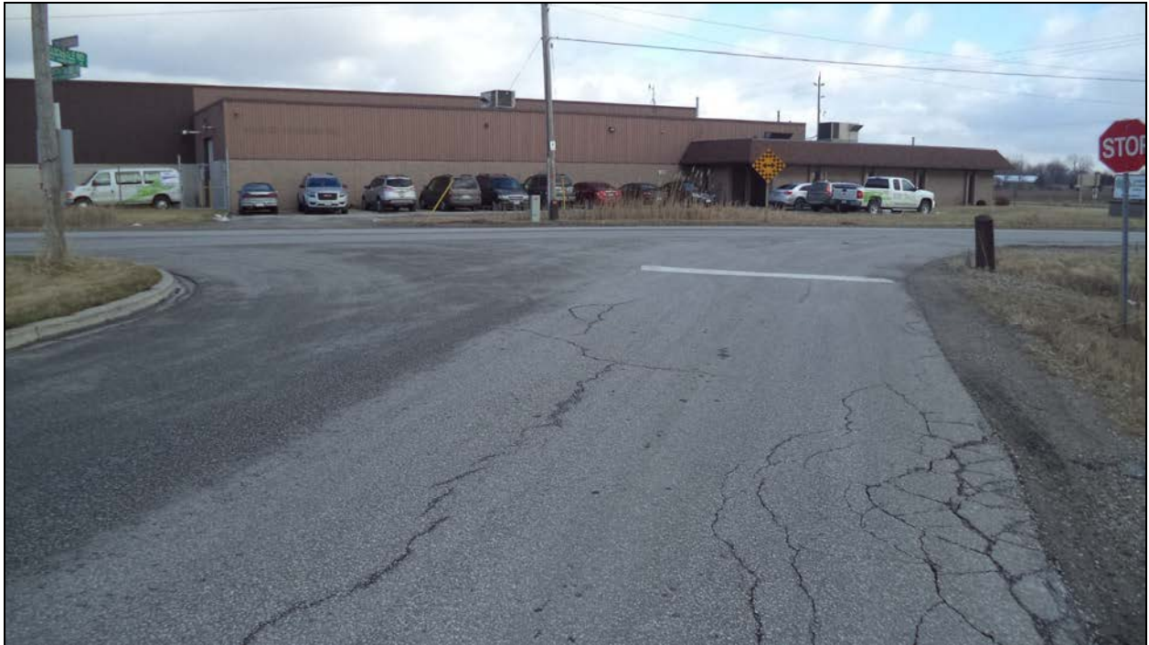
Photograph 1 – Road view (Oldcastle) over Culvert (Looking North)
