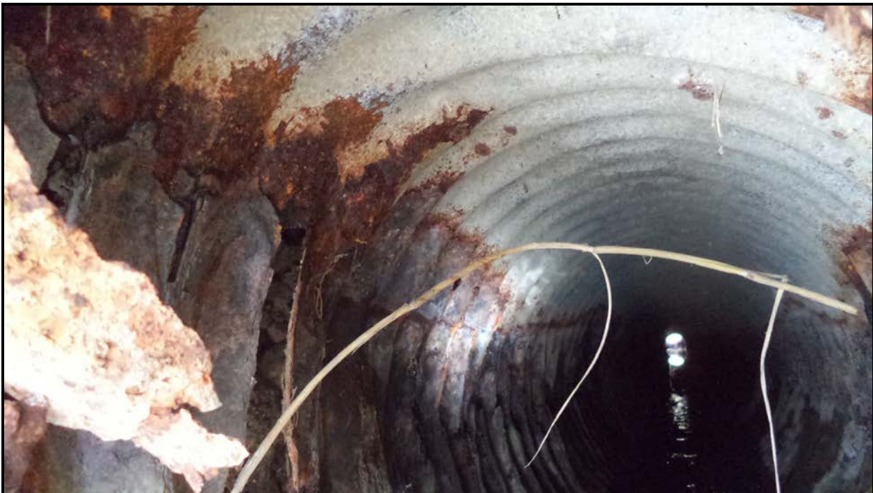
Photograph 2 – Culvert Barrel top at South Inlet
