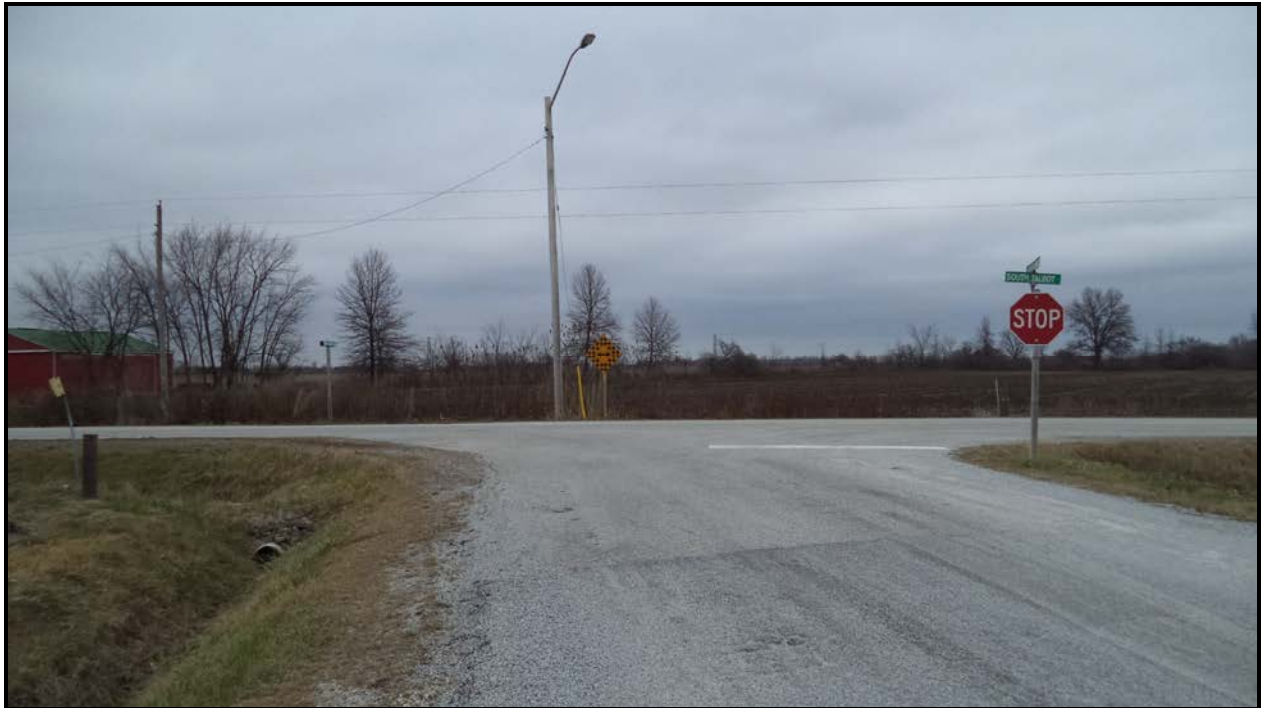
Photograph 1 – Road over Culvert (Looking North)
