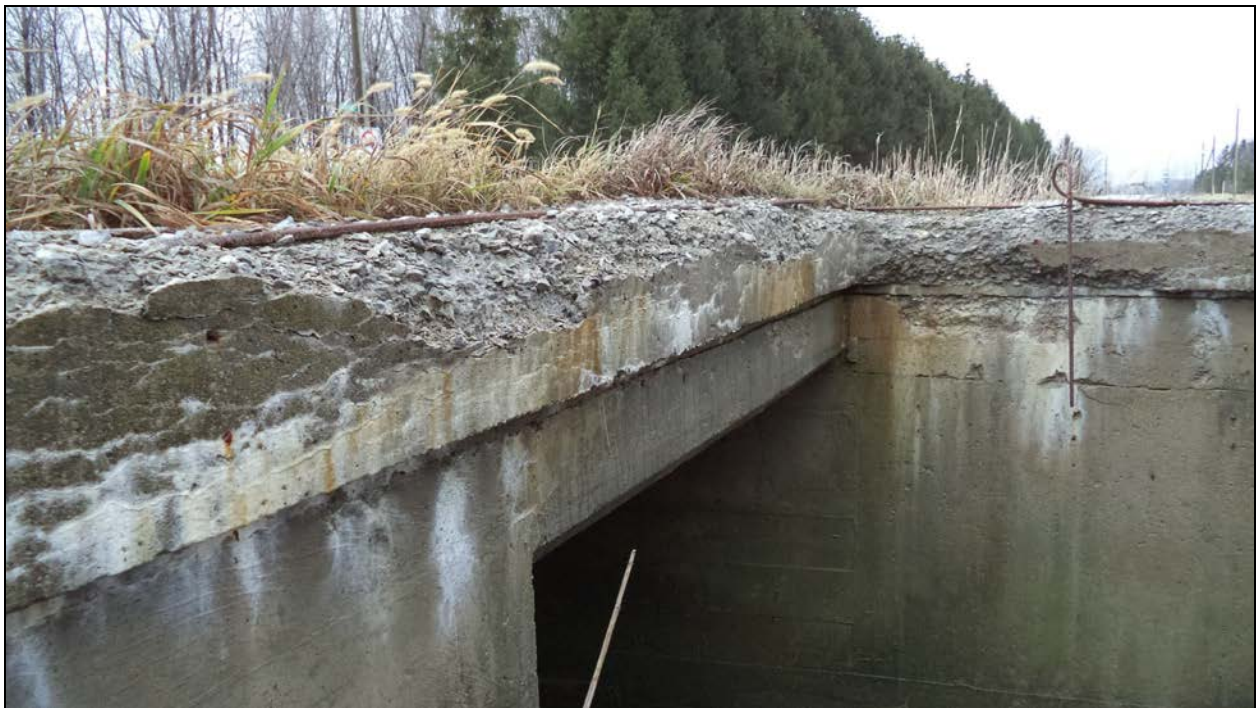
Photograph 4 – Headwall at the North Elevation
