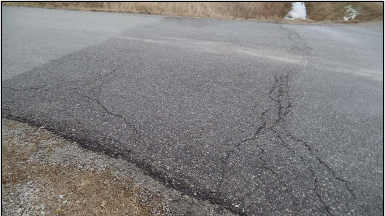
Photograph 7 – Wearing Surface over Culvert (Looking East)
