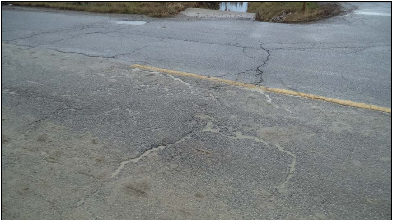
Photograph 7 – Wearing Surface over Culvert (Looking South)
