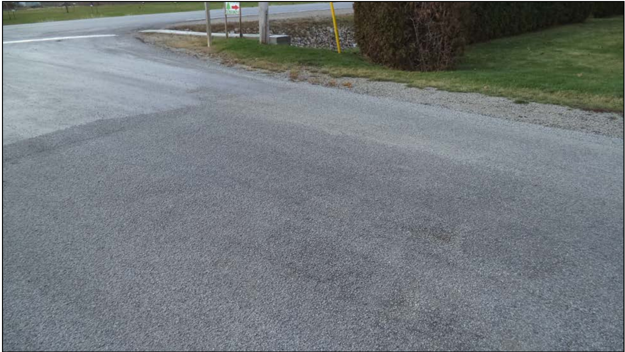
Photograph 7 – Wearing Surface at South Approach
