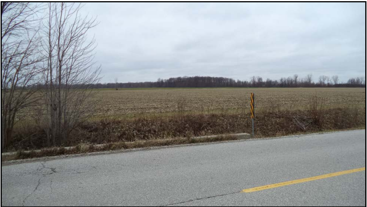
Photograph 6 – Wearing Surface over Culvert (Looking South)
