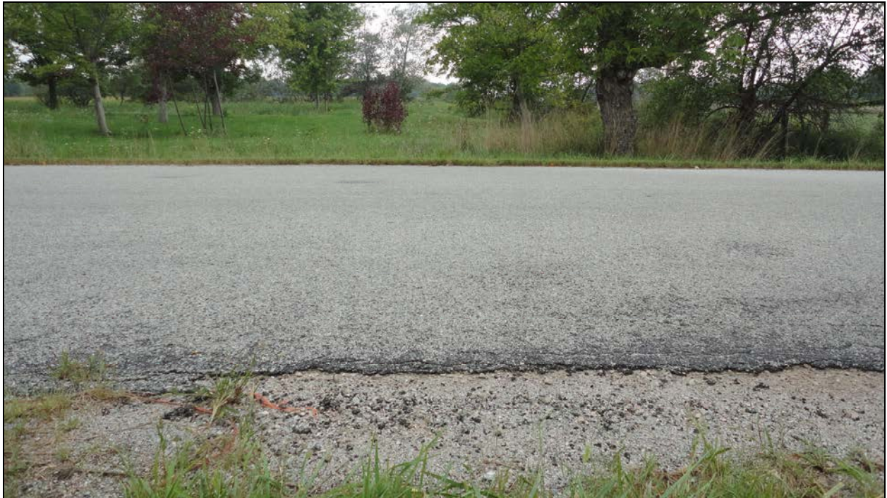
Photograph 3 – Wearing Surface over Culvert (Looking West)
