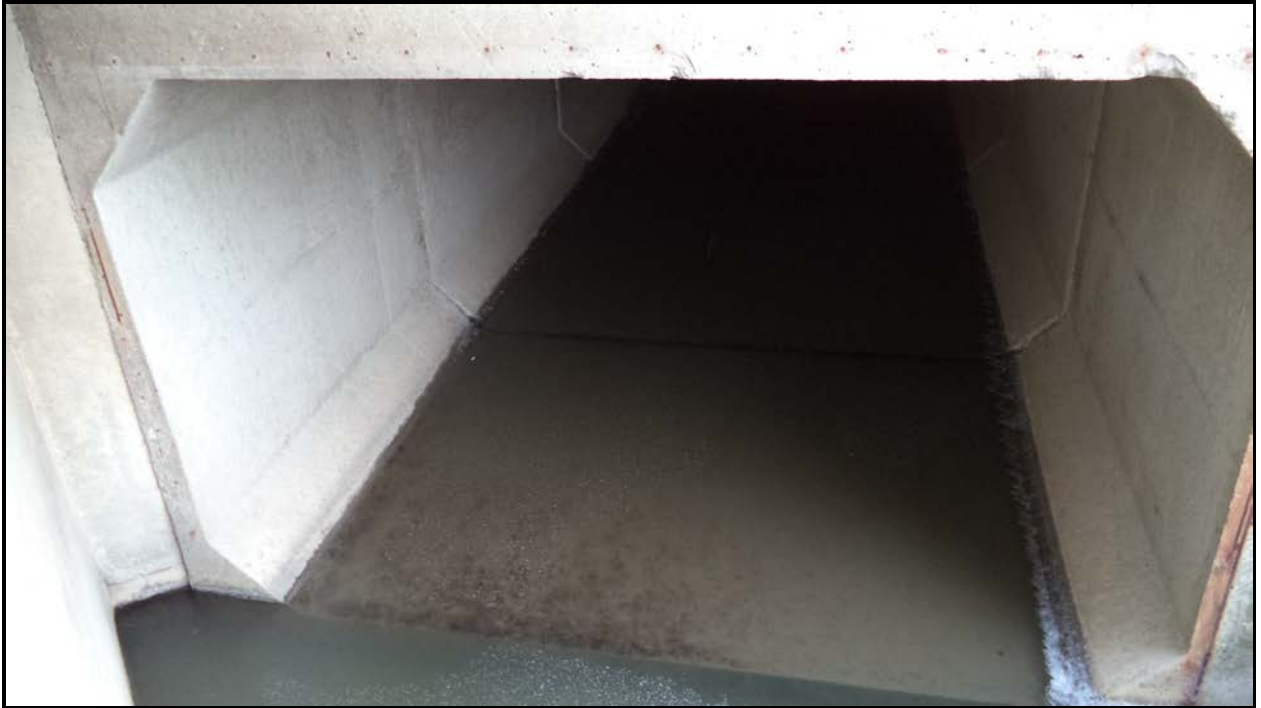
Photograph 3 – Western Culvert Inlet (Inside Box – Limited Inspection)
