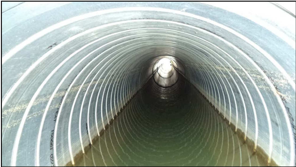
Photograph 2 – Culvert Barrel (Looking East)
