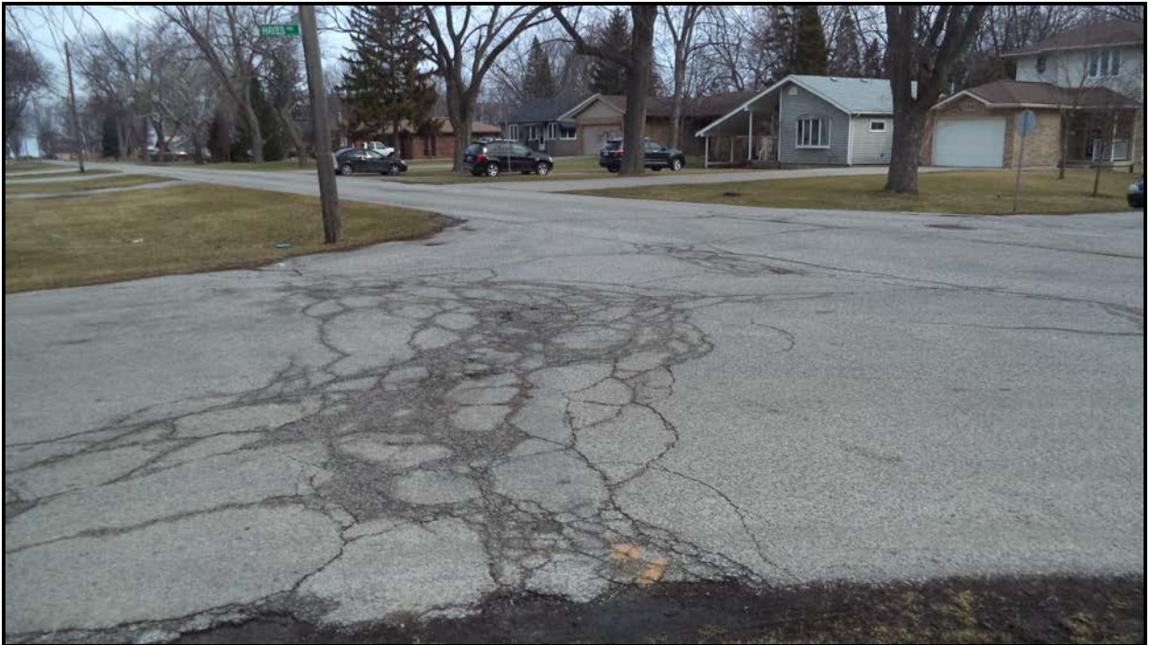
Photograph 1 – Road over Culvert (Looking North)
