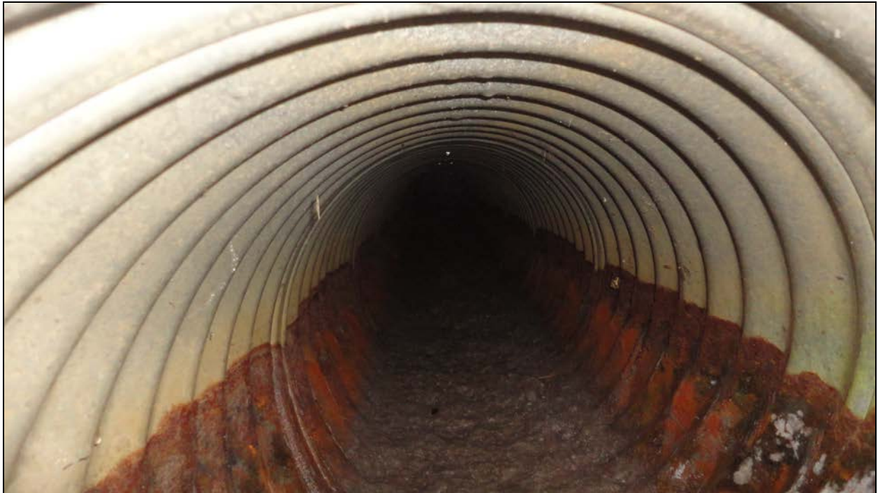
Photograph 7 – Culvert Parallel to Road at West Edge (Intersecting with Crossing Culvert)
