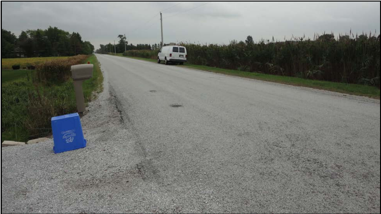
Photograph 1 – Road over Culvert (Looking South)
