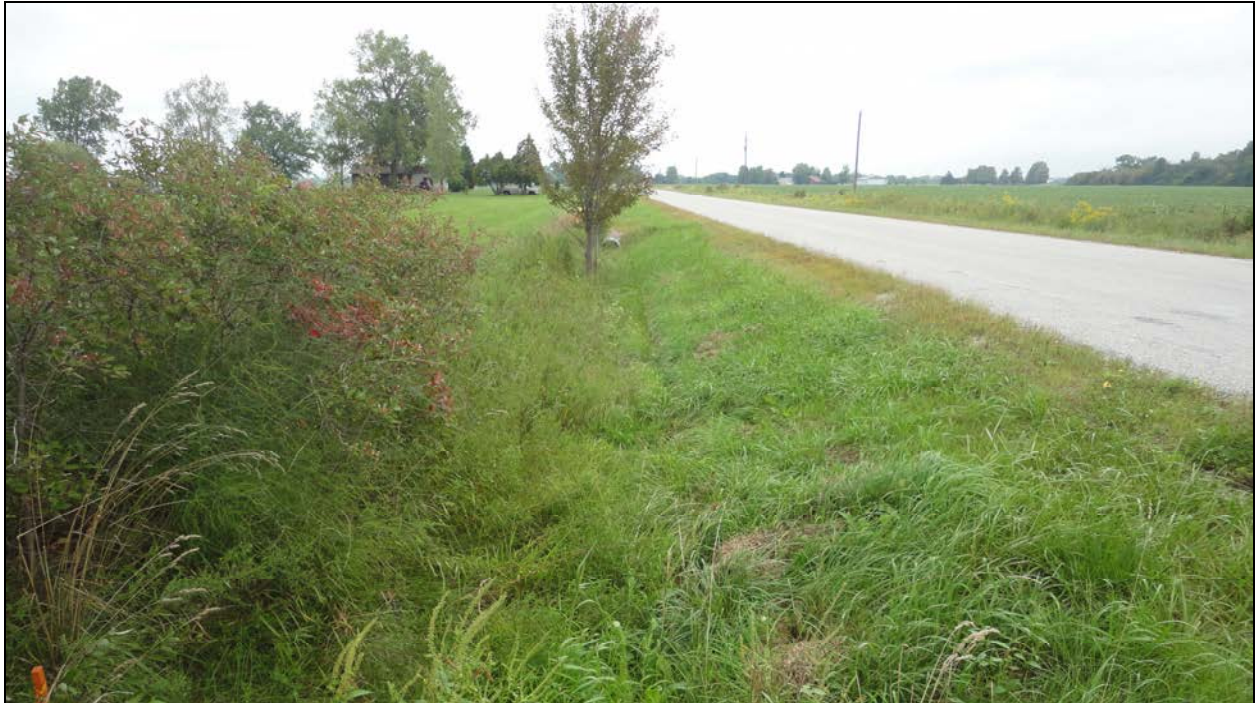
Photograph 4 – West Embankments & Waterways (Looking West)
