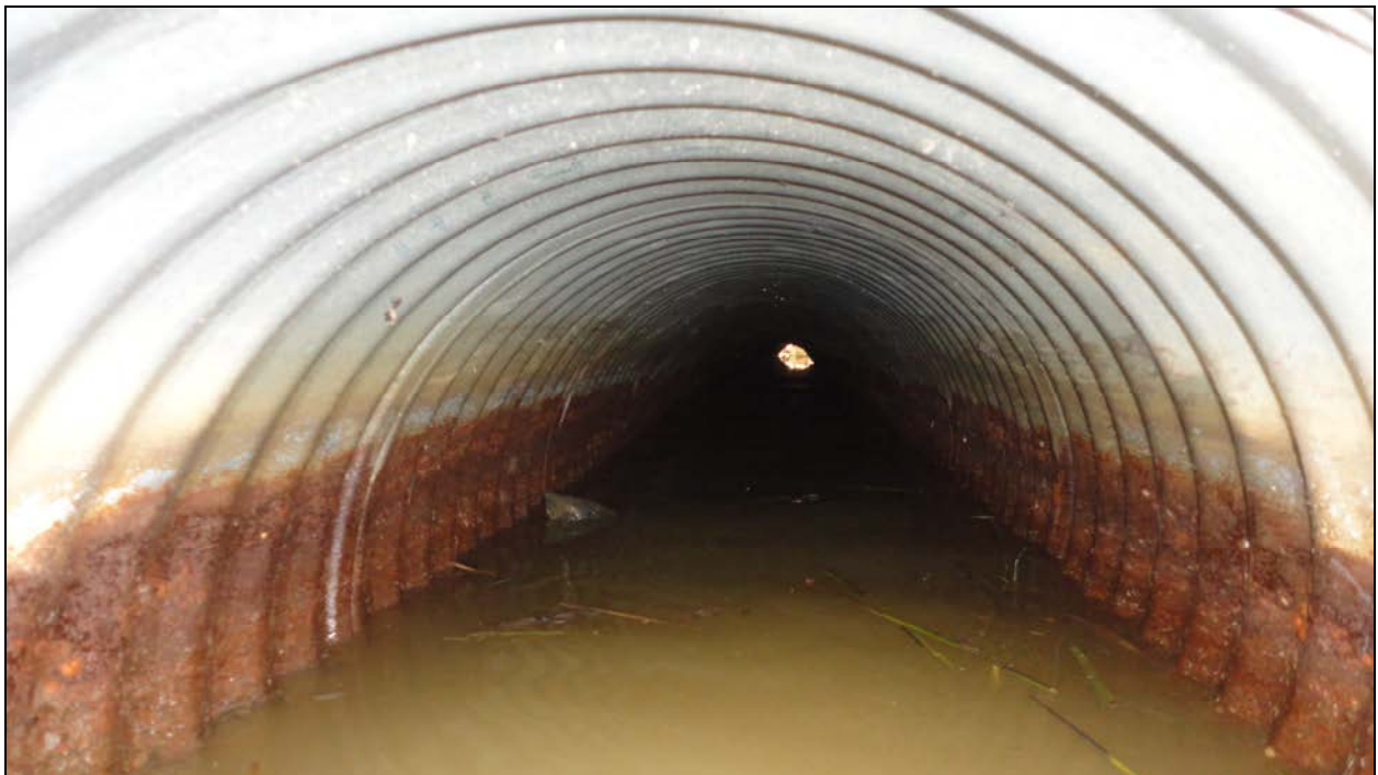
Photograph 6 – Culvert Barrel (Looking West)
