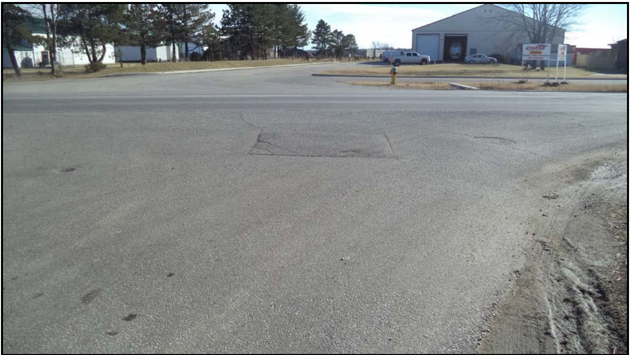
Photograph 6 – Wearing Surface at South Approach
