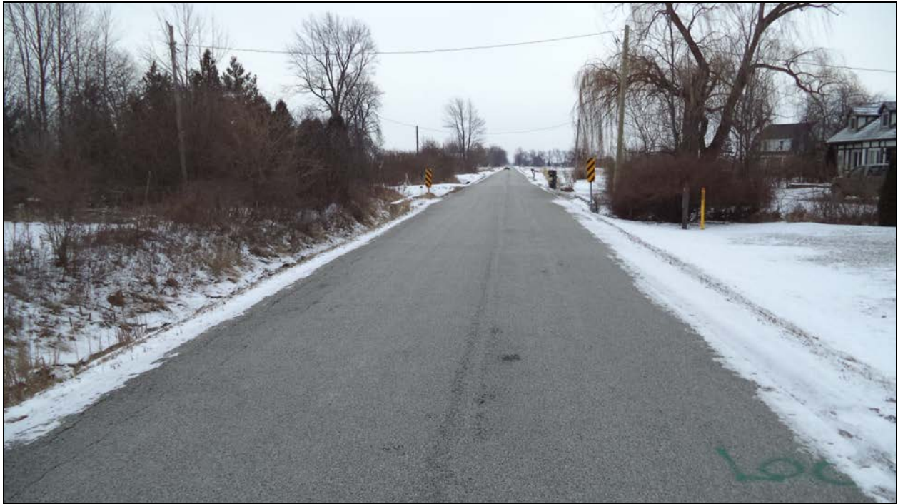
Photograph 1 – Road over Culvert (Looking South)
