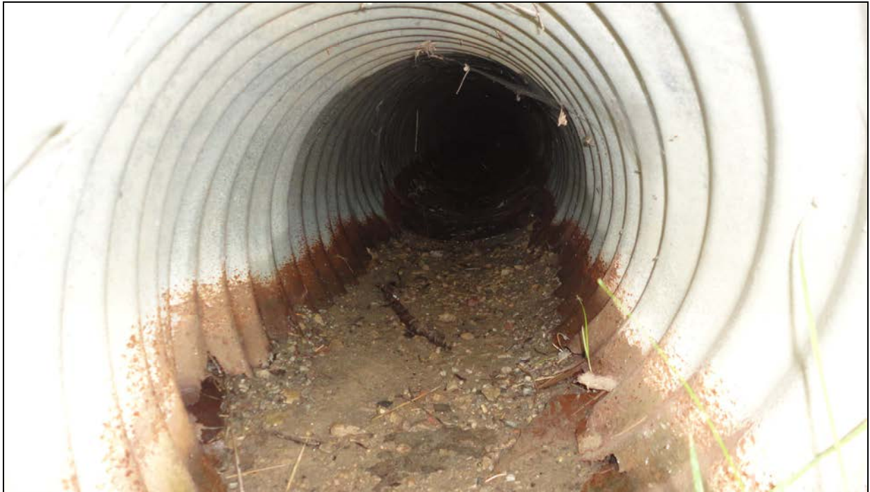
Photograph 3 – Culvert Barrel (Looking West)
