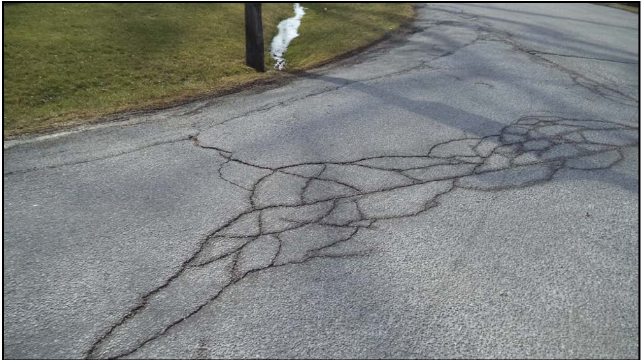
Photograph 5 – Wearing Surface over Culvert (Looking South)
