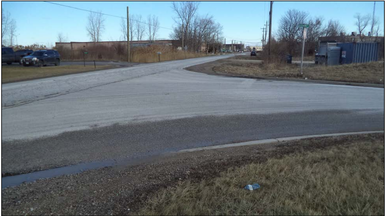
Photograph 1 – Road over Culvert (Looking North)
