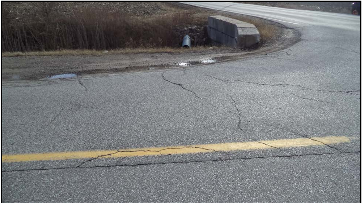
Photograph 5 – Wearing Surface at East Approach (Looking South)
