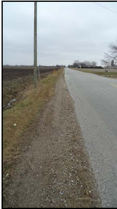
Photograph 7 – Wearing Surface at Northern Road Side
