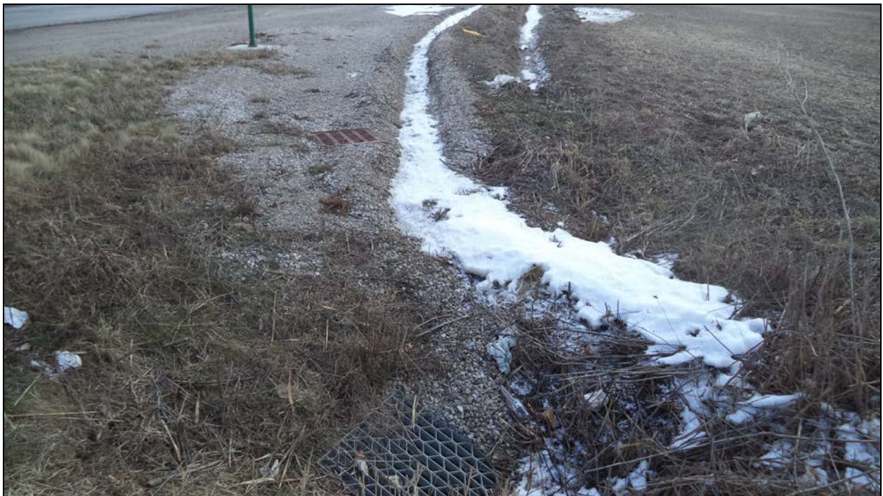
Photograph 2 – Manhole, East Side of Oldcastle Road at the Intersection
