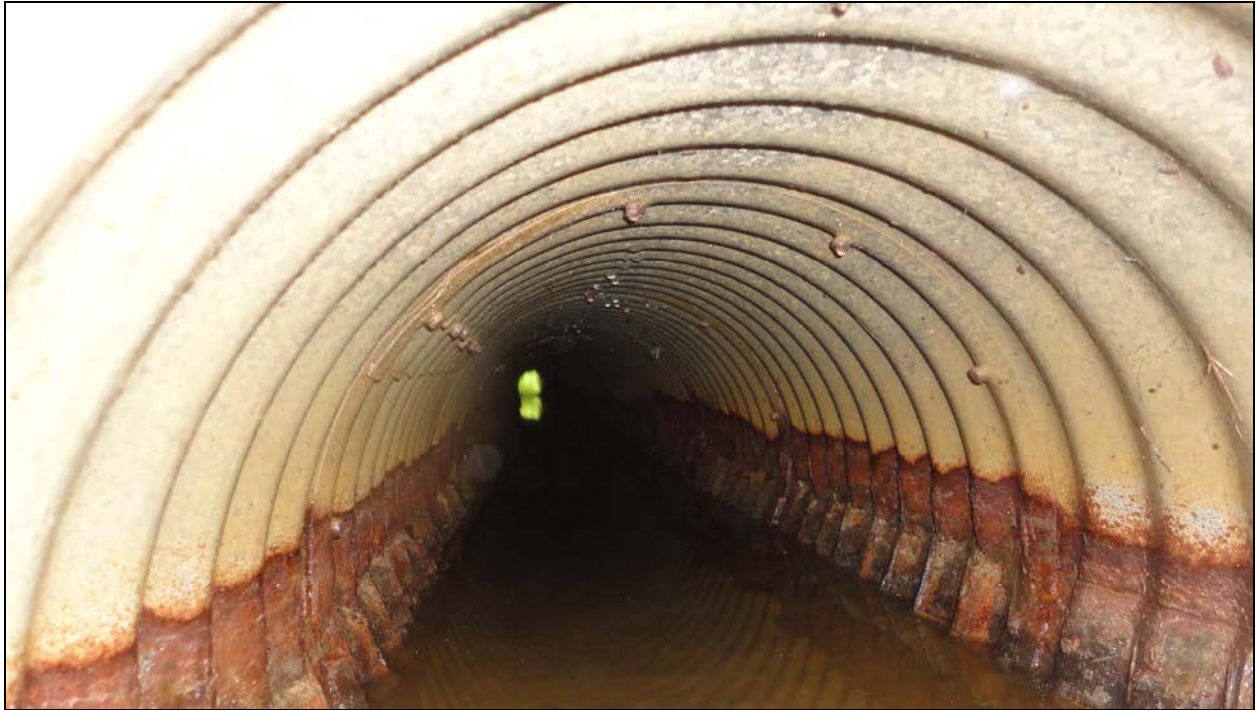
Photograph 4 – Culvert Barrel (Looking East)
