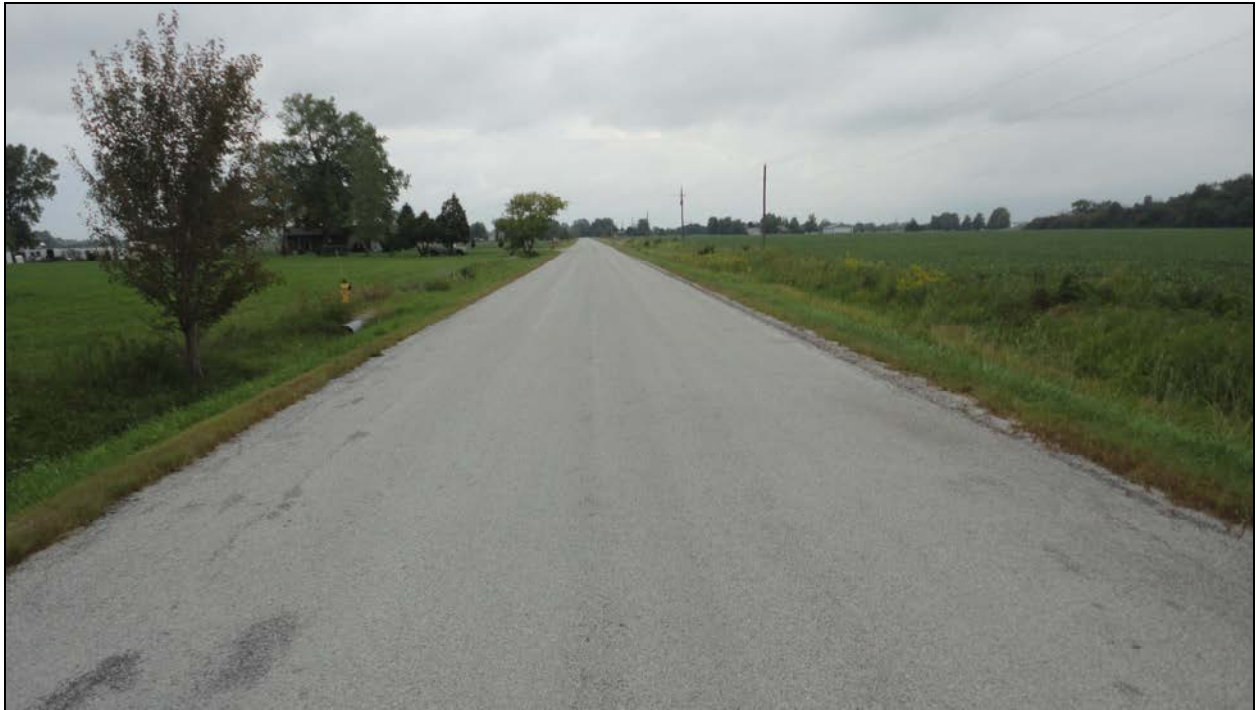
Photograph 1 – Wearing Surface over Culvert (Looking West)
