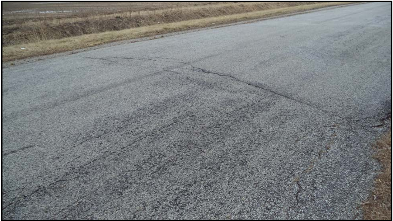
Photograph 5 – Wearing Surface over Culvert (Looking South)
