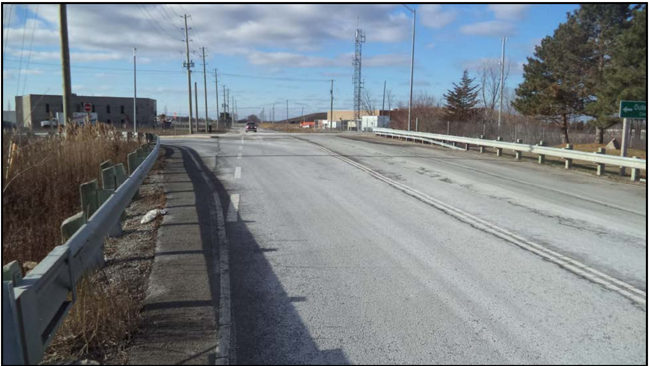
Photograph 6 – Wearing Surface over Culvert (Looking North)
