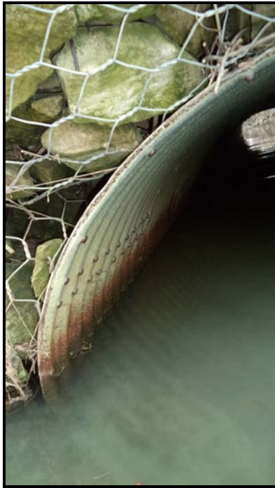
Photograph 3 – Culvert Barrel (East Elevation)
