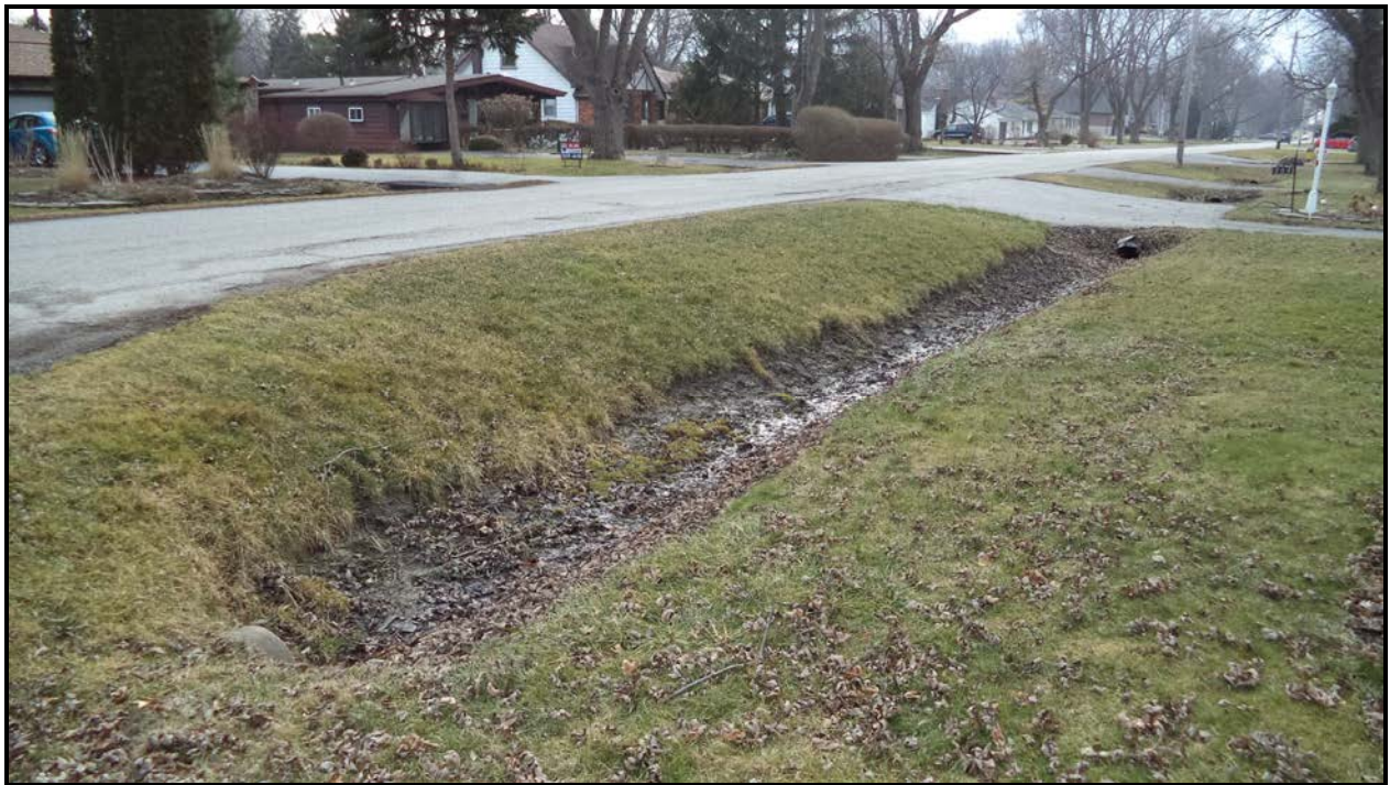
Photograph 6 – Water Stream (Edgewater Road West Side – Looking South)
