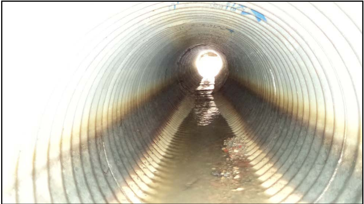
Photograph 3 – Culvert Barrel (Looking East)
