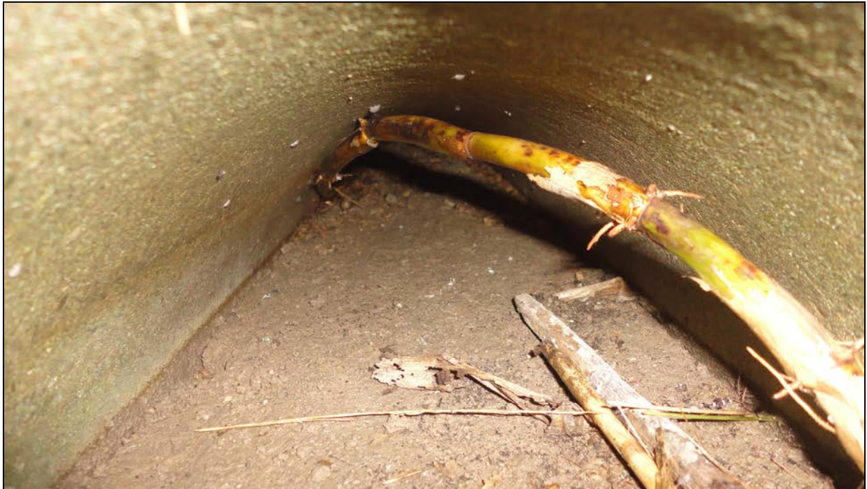
Photograph 5 –Culvert Barrel (Looking West)
