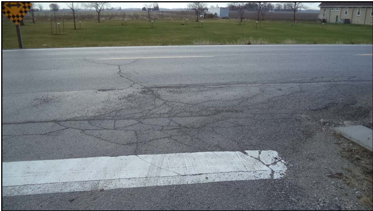
Photograph 6 – Wearing Surface at South Approach
