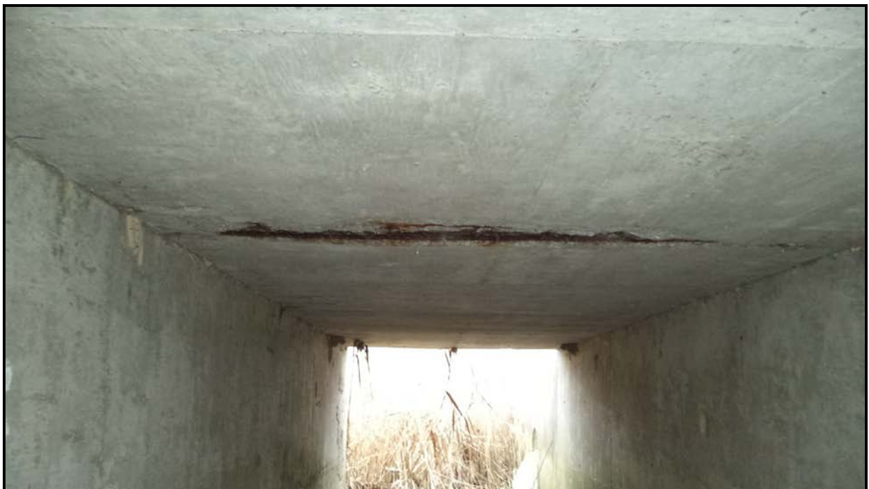
Photograph 4 – Culvert Barrel - Soffit
