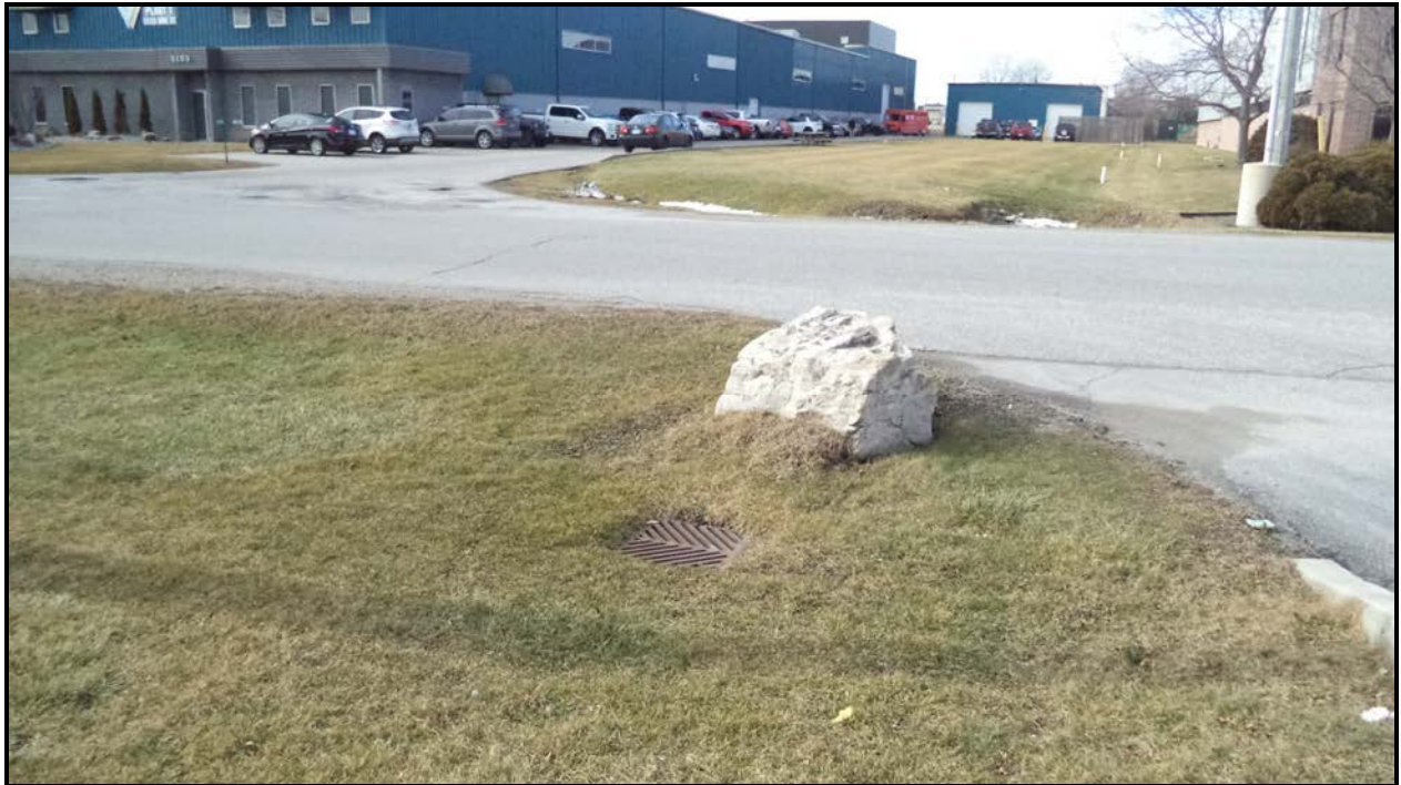
Photograph 1 – Road over Culvert (Looking North)
