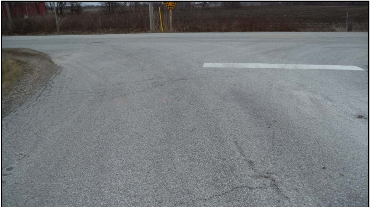
Photograph 5 – Wearing Surface over Culvert (Looking North)
