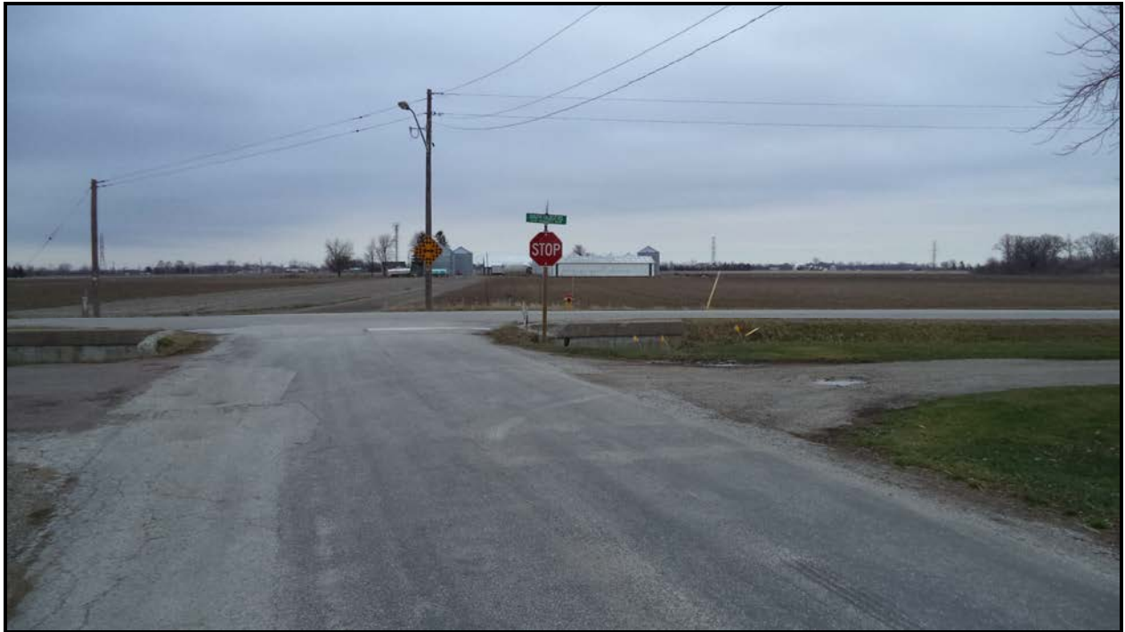
Photograph 1 – Road over Culvert (Looking North)
