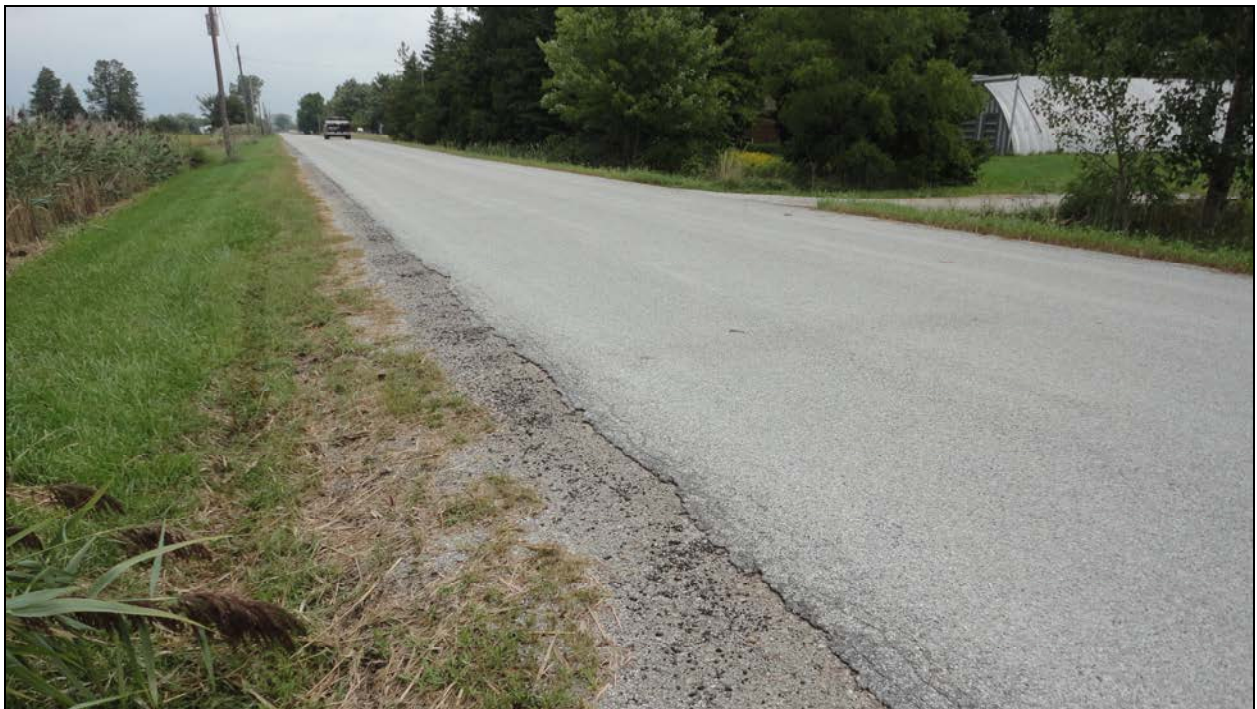
Photograph 2 – Wearing Surface over Culvert (Looking South)
