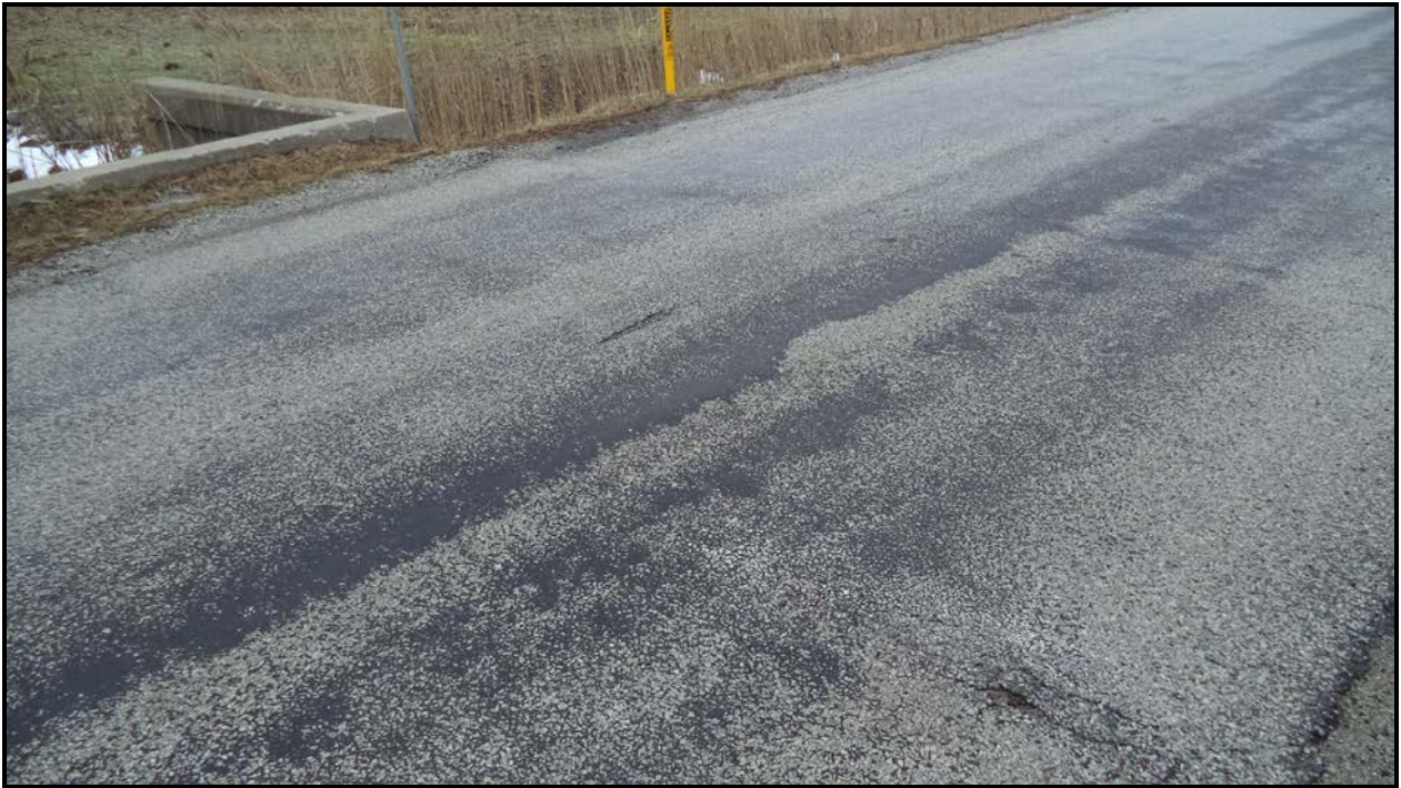
Photograph 9 – Wearing Surface over Culvert (Looking South)
