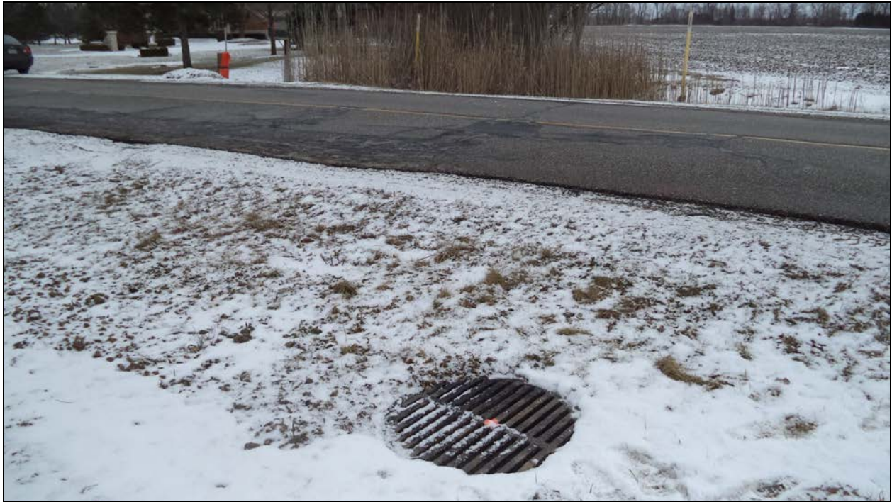
Photograph 1 – Road over Culvert (Looking East)
