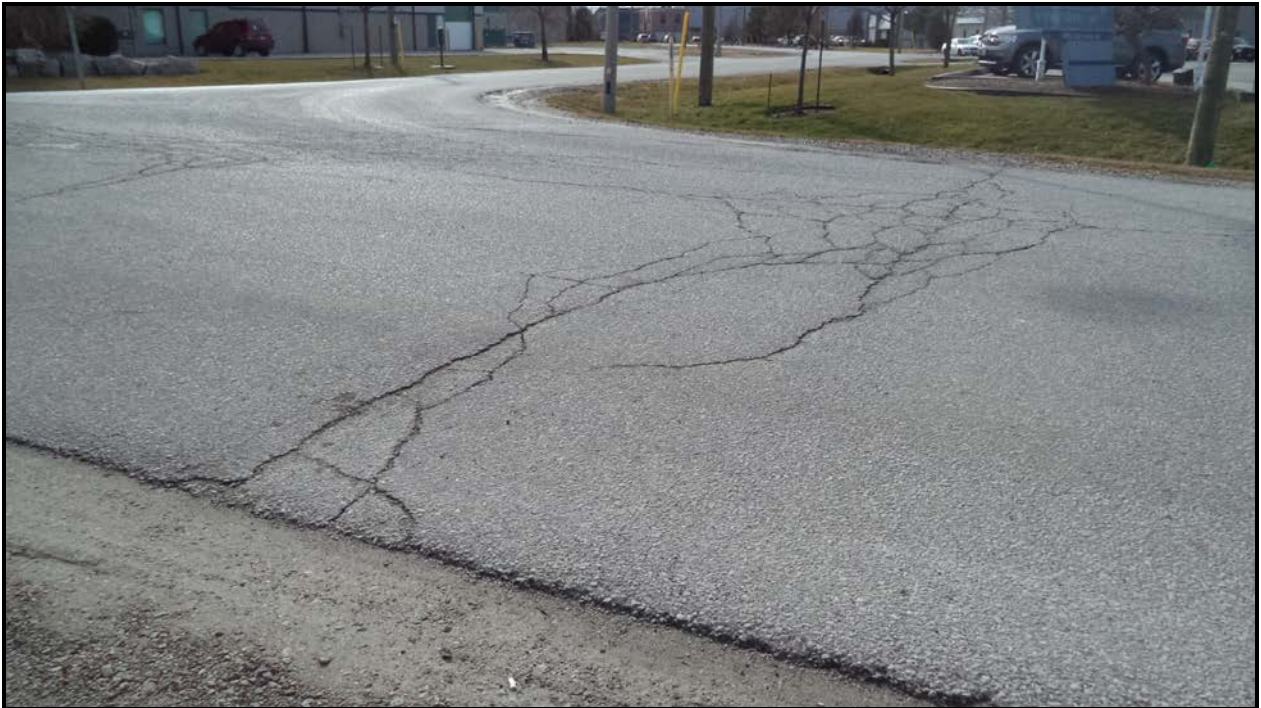
Photograph 5 – Wearing Surface over Culvert (Looking South)
