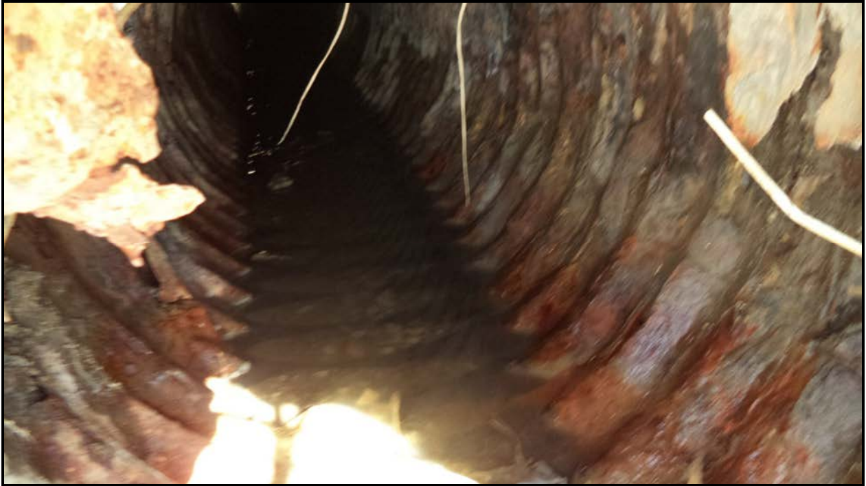
Photograph 3 – Culvert Barrel Bottom at South Inlet
