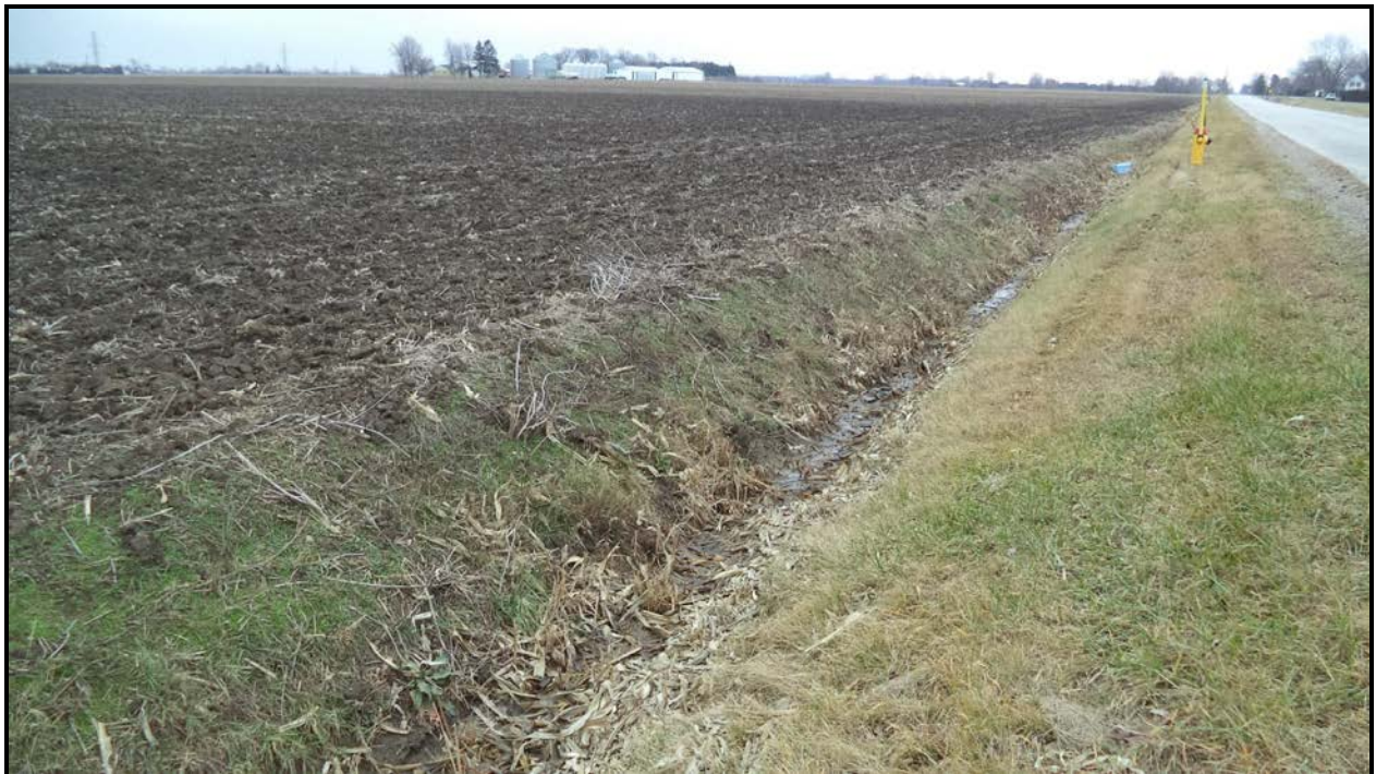
Photograph 8 – Water Stream (South Talbot Road East Side – Looking East)
