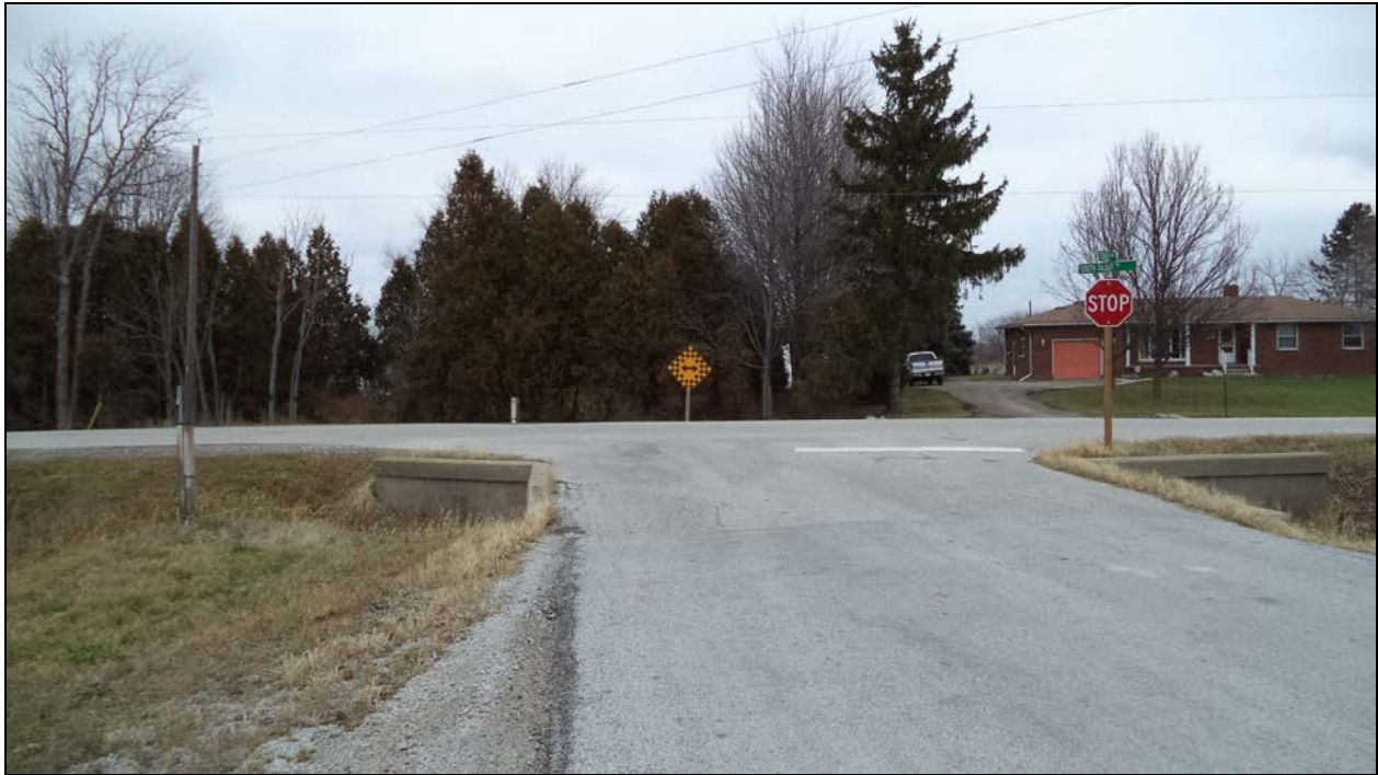
Photograph 1 – Road over Culvert (Looking North)
