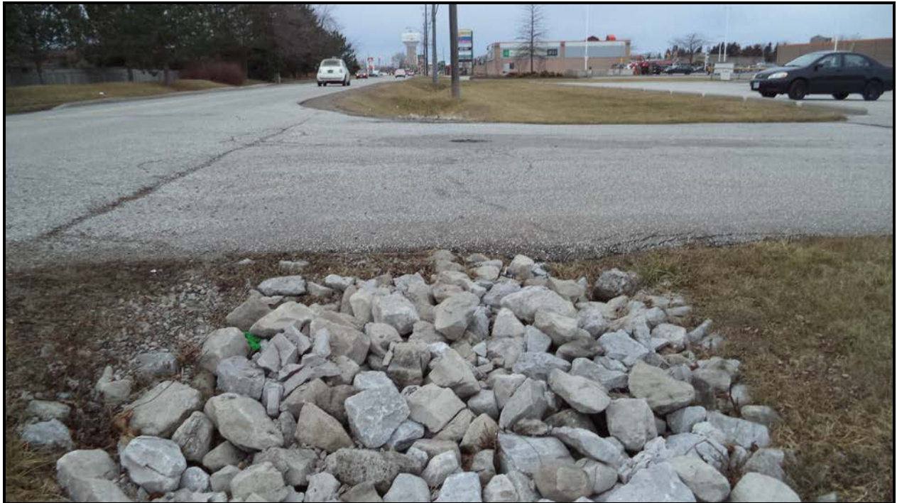
Photograph 5 – Wearing Surface over Culvert (Looking West)
