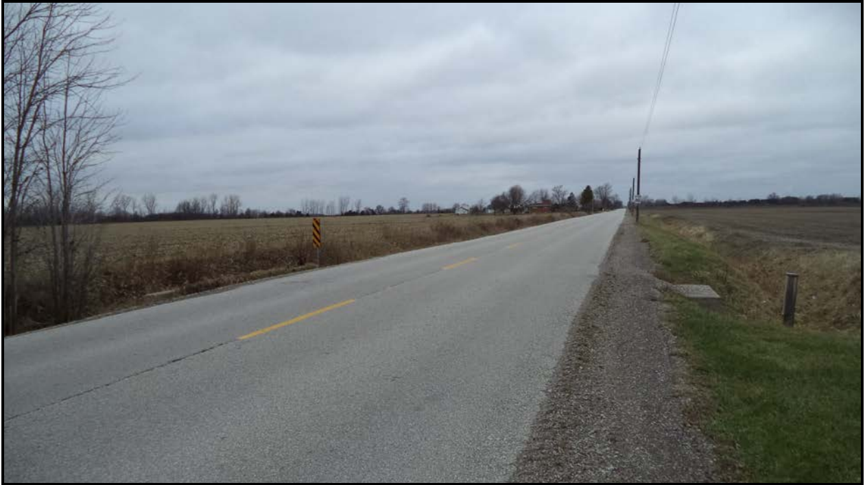
Photograph 1 – Road over Culvert (Looking West)
