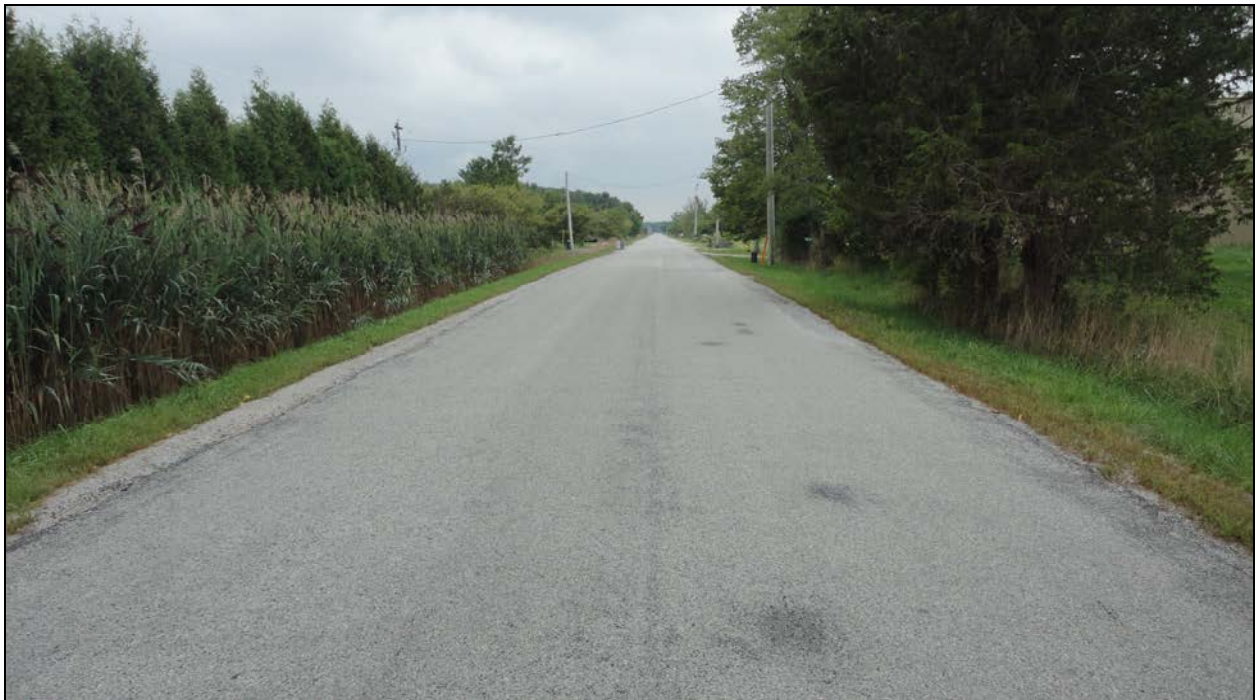
Photograph 2 – Wearing Surface over Culvert (Looking South)
