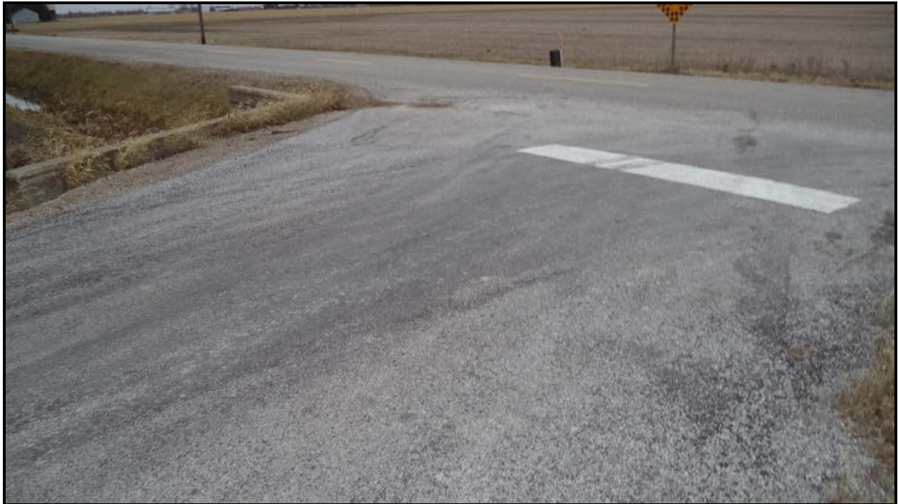
Photograph 5 – Wearing Surface over Culvert (Looking North)
