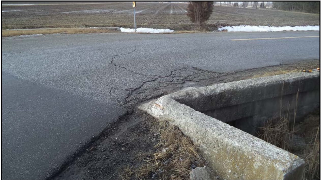
Photograph 5 – Wearing Surface over Culvert (Looking South)
