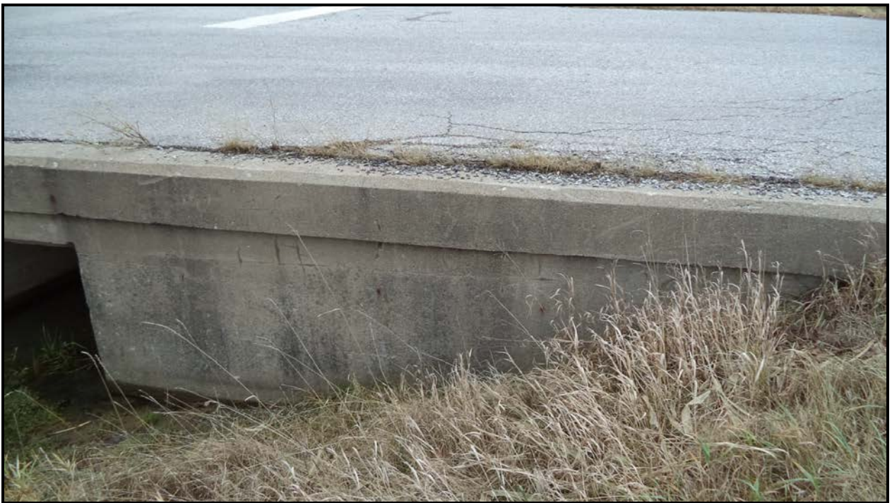
Photograph 6 – Wearing Surface at South Approach
