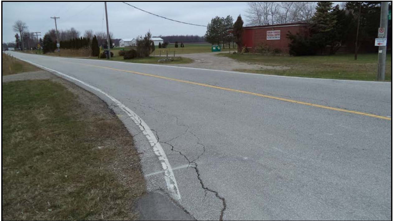
Photograph 7 – Wearing Surface at South Approach (Looking South)
