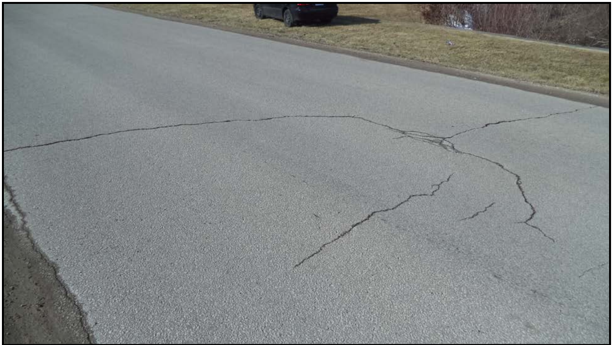
Photograph 6 – Wearing Surface at South Approach
