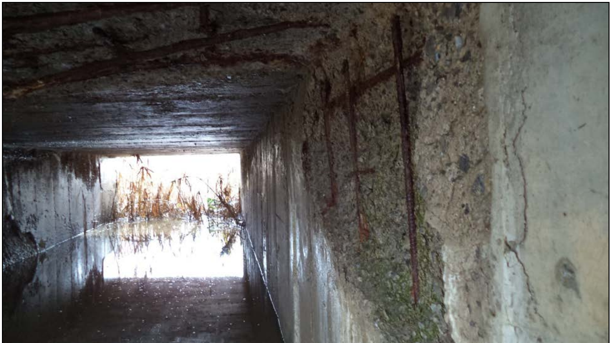
Photograph 4 – Culvert Barrel (Looking South)
