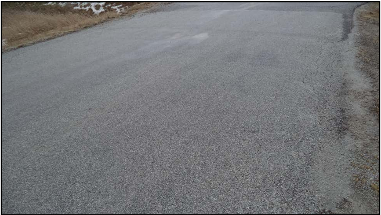
Photograph 8 – Wearing Surface at North Approach
