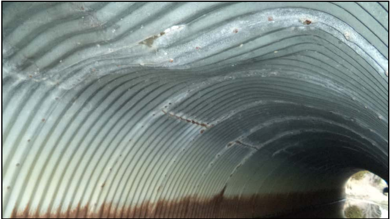
Photograph 3 – Culvert Barrel (Looking North)
