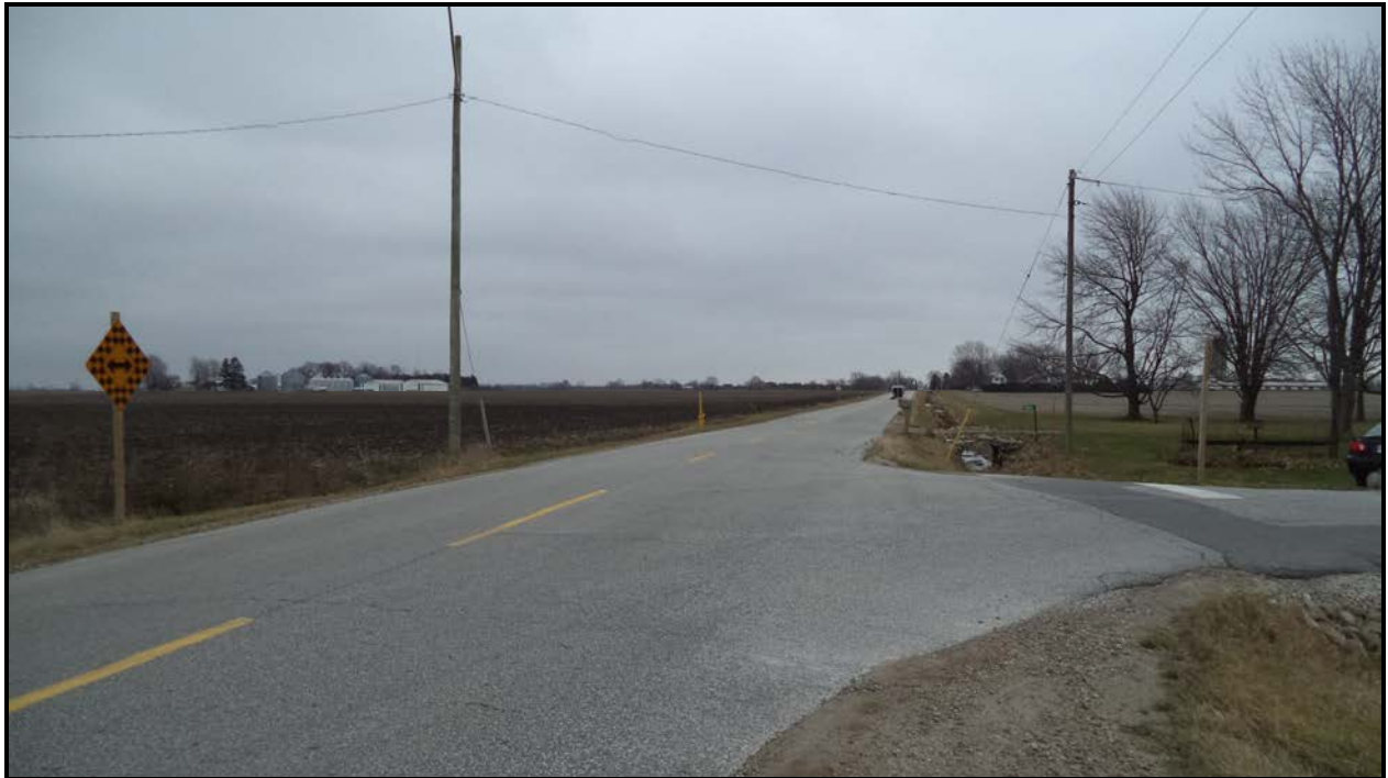
Photograph 1 – Road over Culvert (Looking East)
