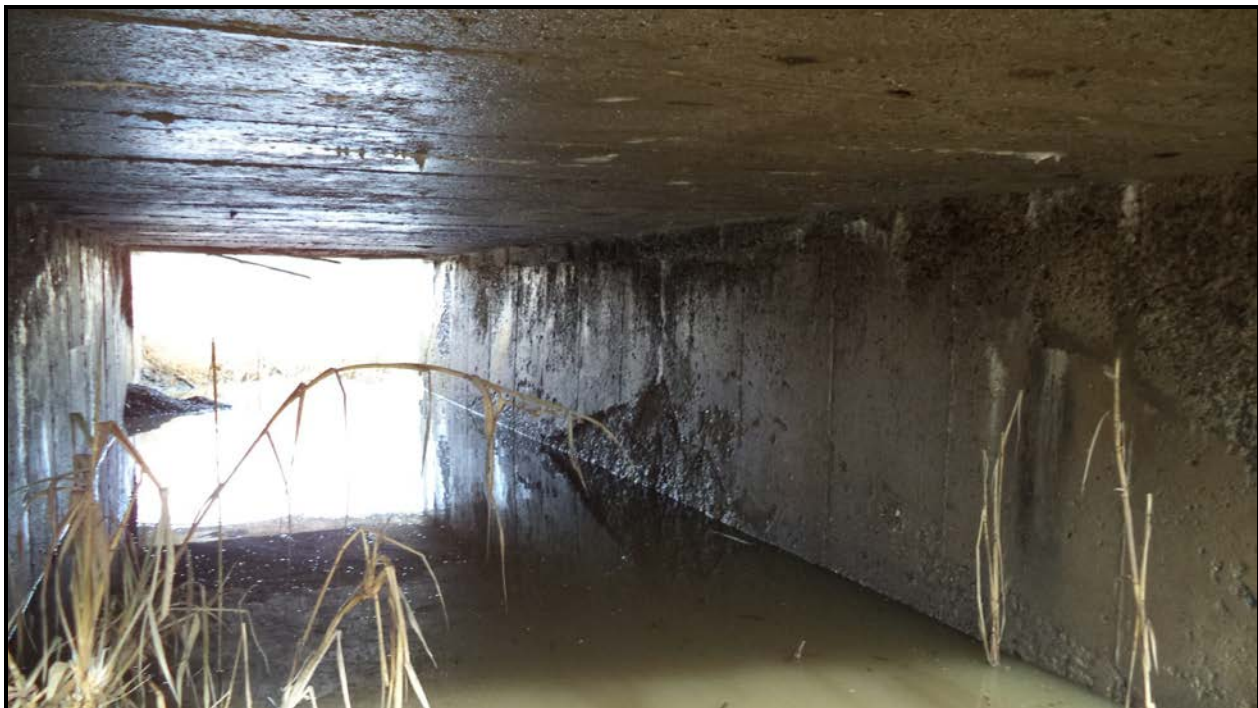
Photograph 2 – Culvert Barrel (Looking North)
