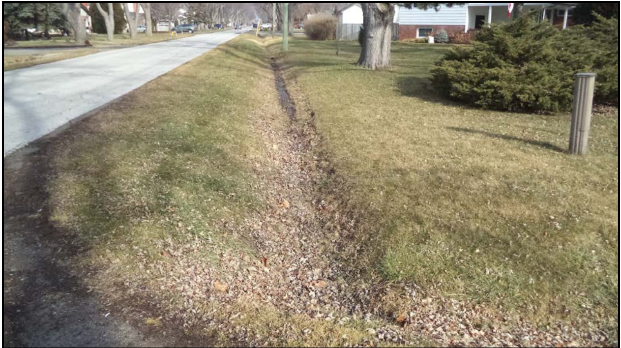
Photograph 7 – Water Stream (Arlington Blvd. Road East Side - Looking North)
