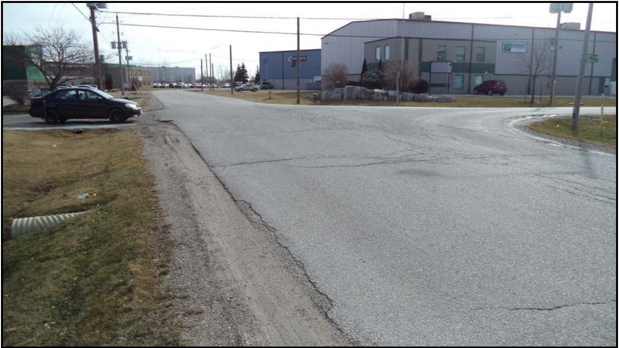
Photograph 1 – Road over Culvert (Looking North)
