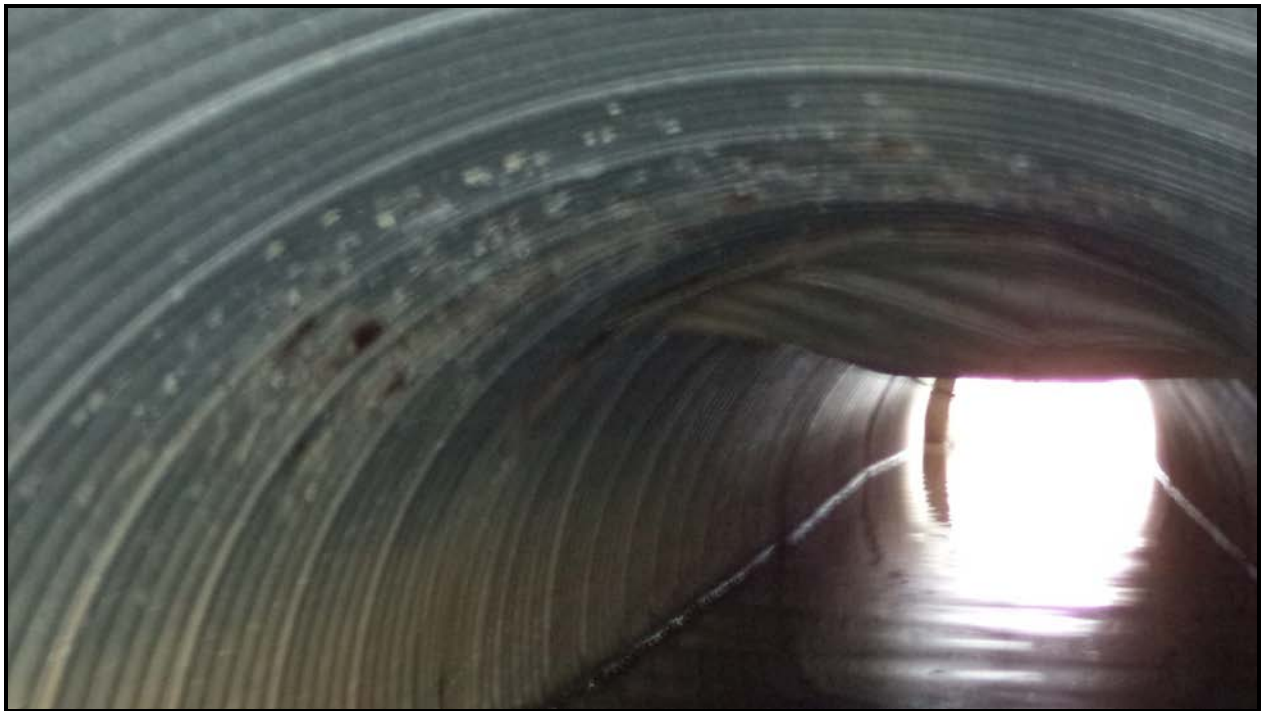
Photograph 2 – Culvert Barrel Looking North
