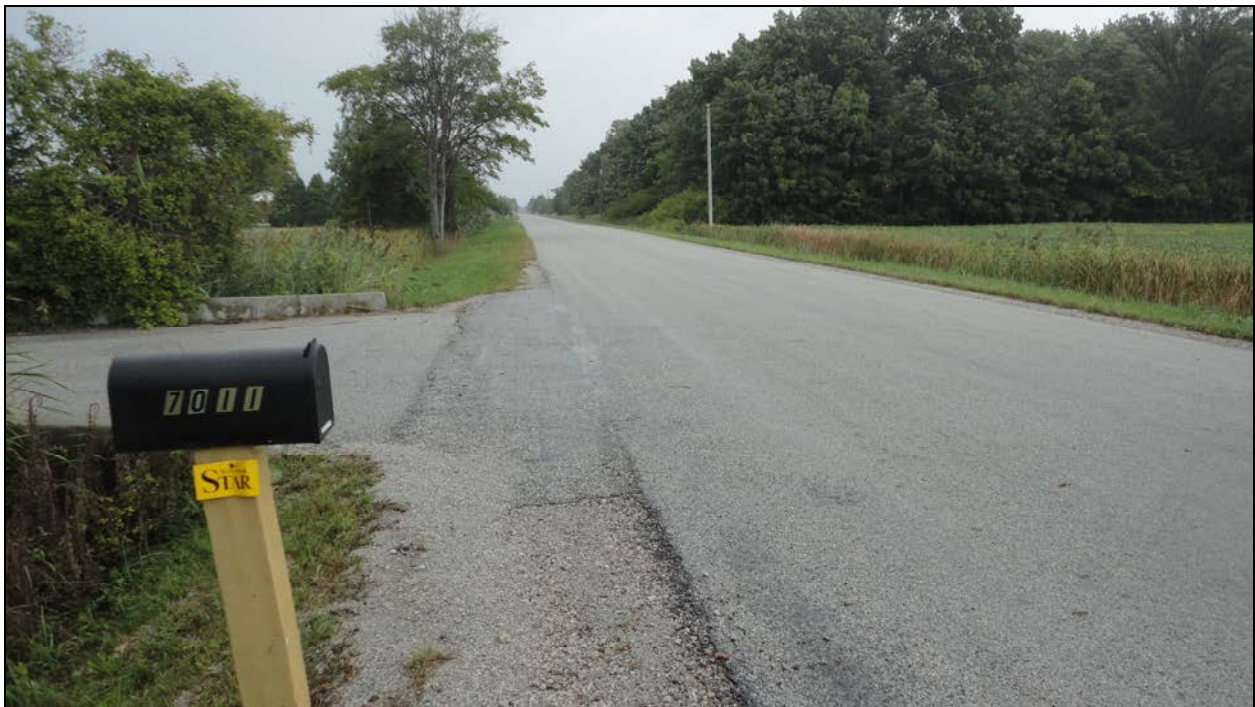
Photograph 2 – Wearing Surface over Culvert (Looking North)
