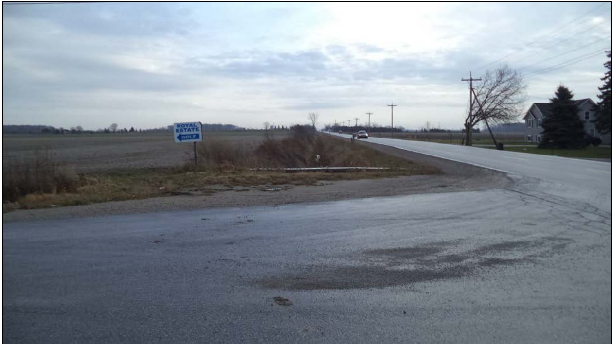
Photograph 5 – Wearing Surface over Culvert (Looking East)
