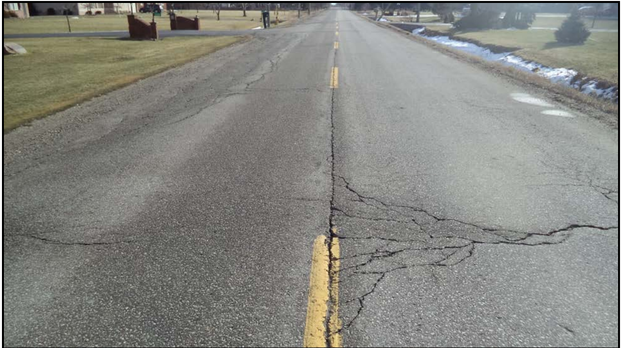
Photograph 5 – Wearing Surface over Culvert (Looking East)
