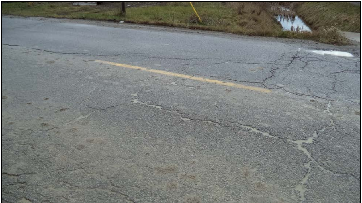
Photograph 8 – Wearing Surface at East Approach (Looking South)
