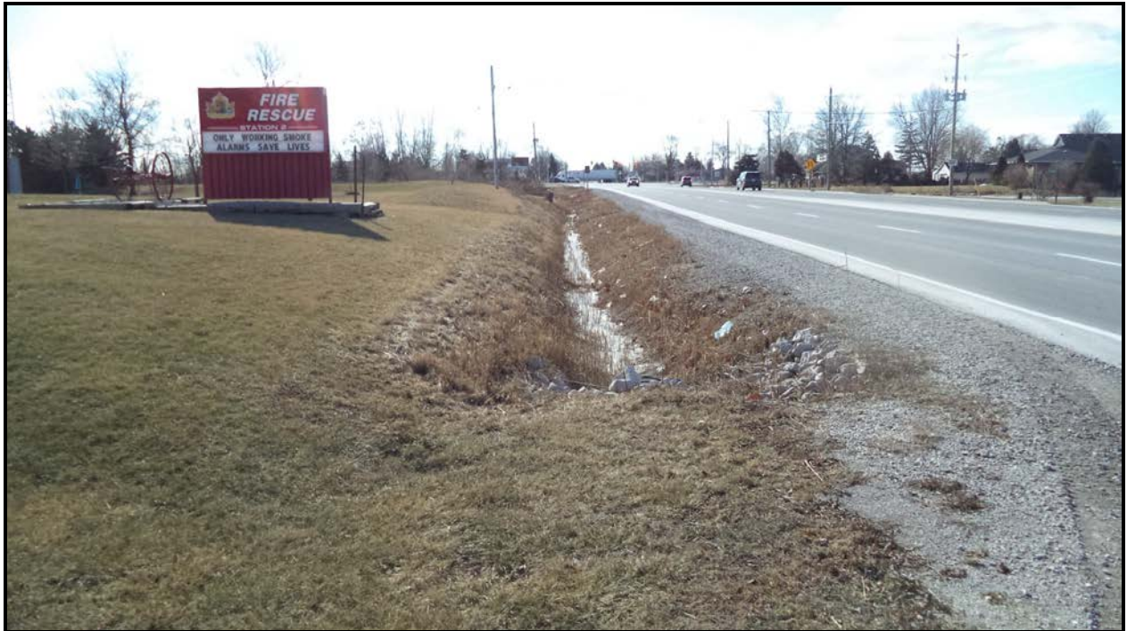
Photograph 5 – Water Stream (McCord Lane South Side - Looking South)
