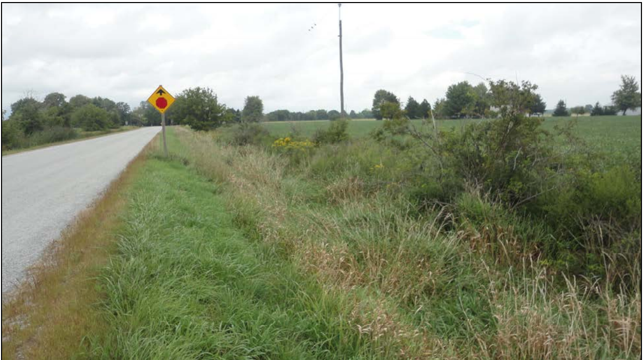
Photograph 4 – East Embankments & Waterway (Looking North)
