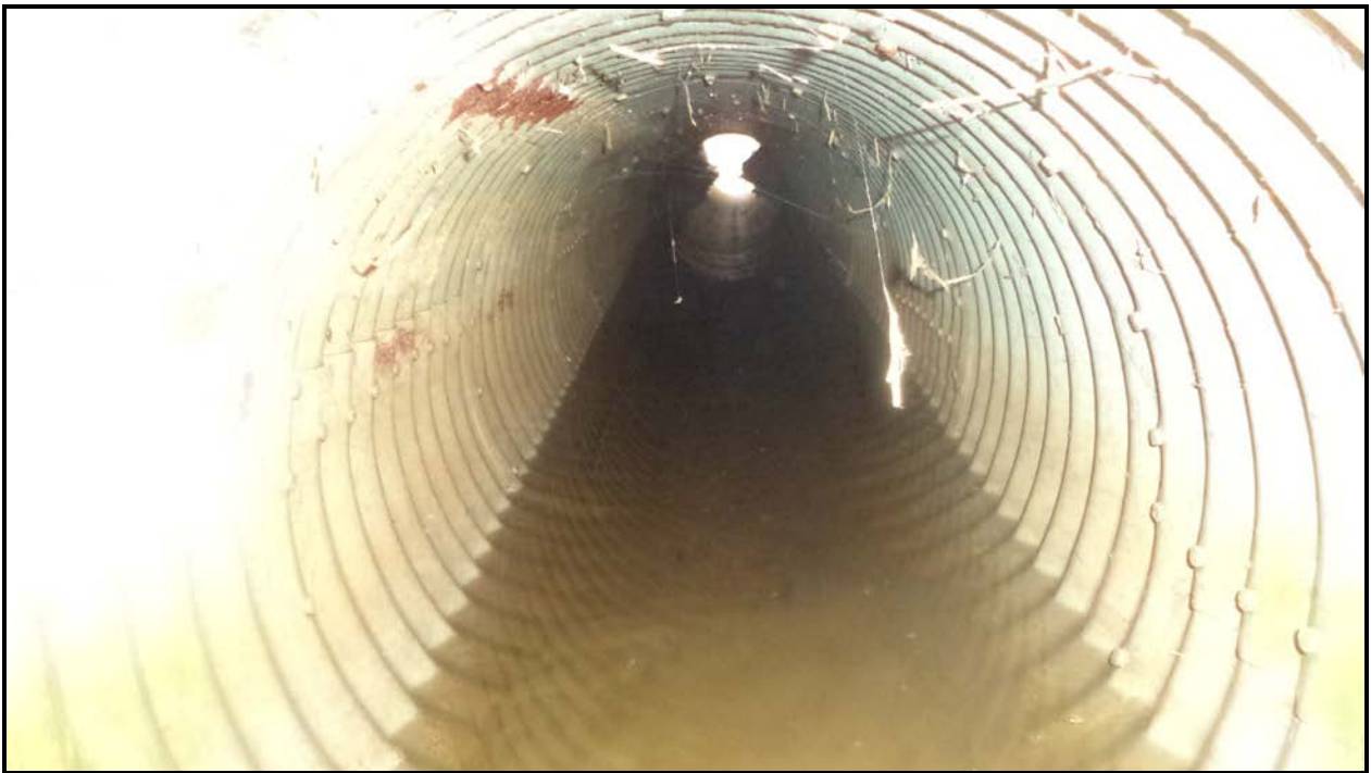
Photograph 2 – Culvert Barrel (Looking East)
