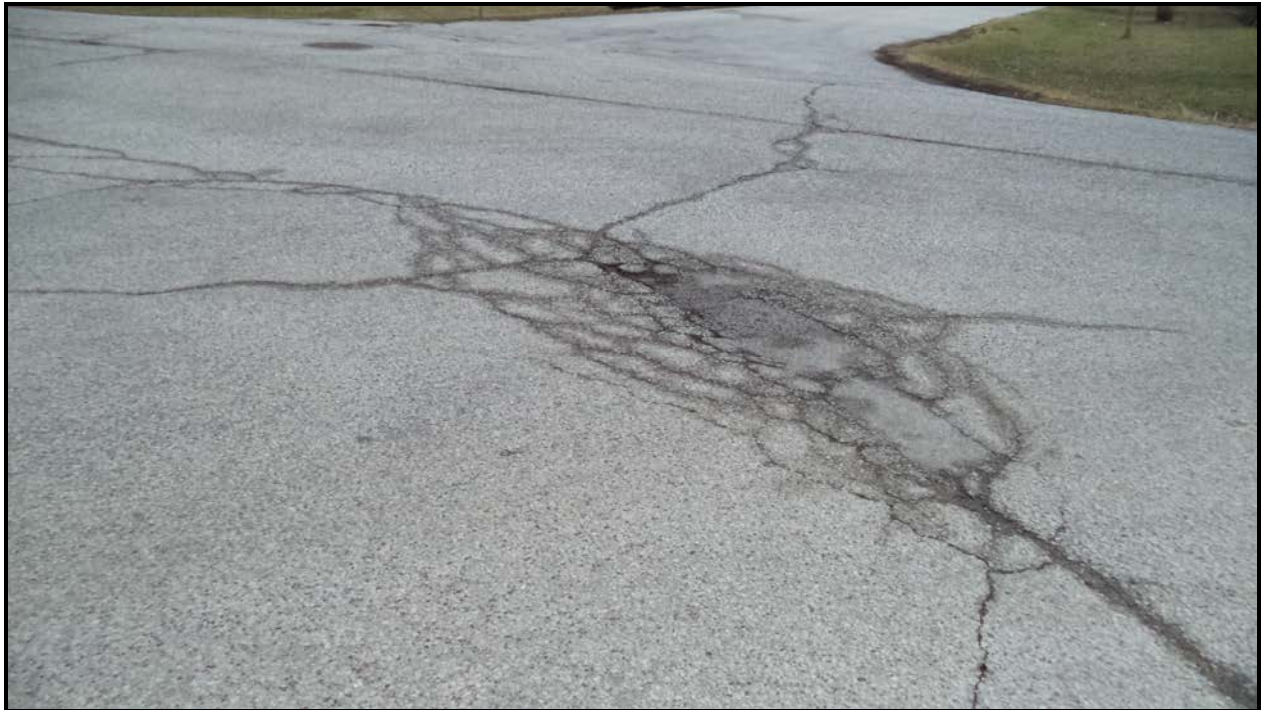
Photograph 7 – Wearing Surface at East Approach
