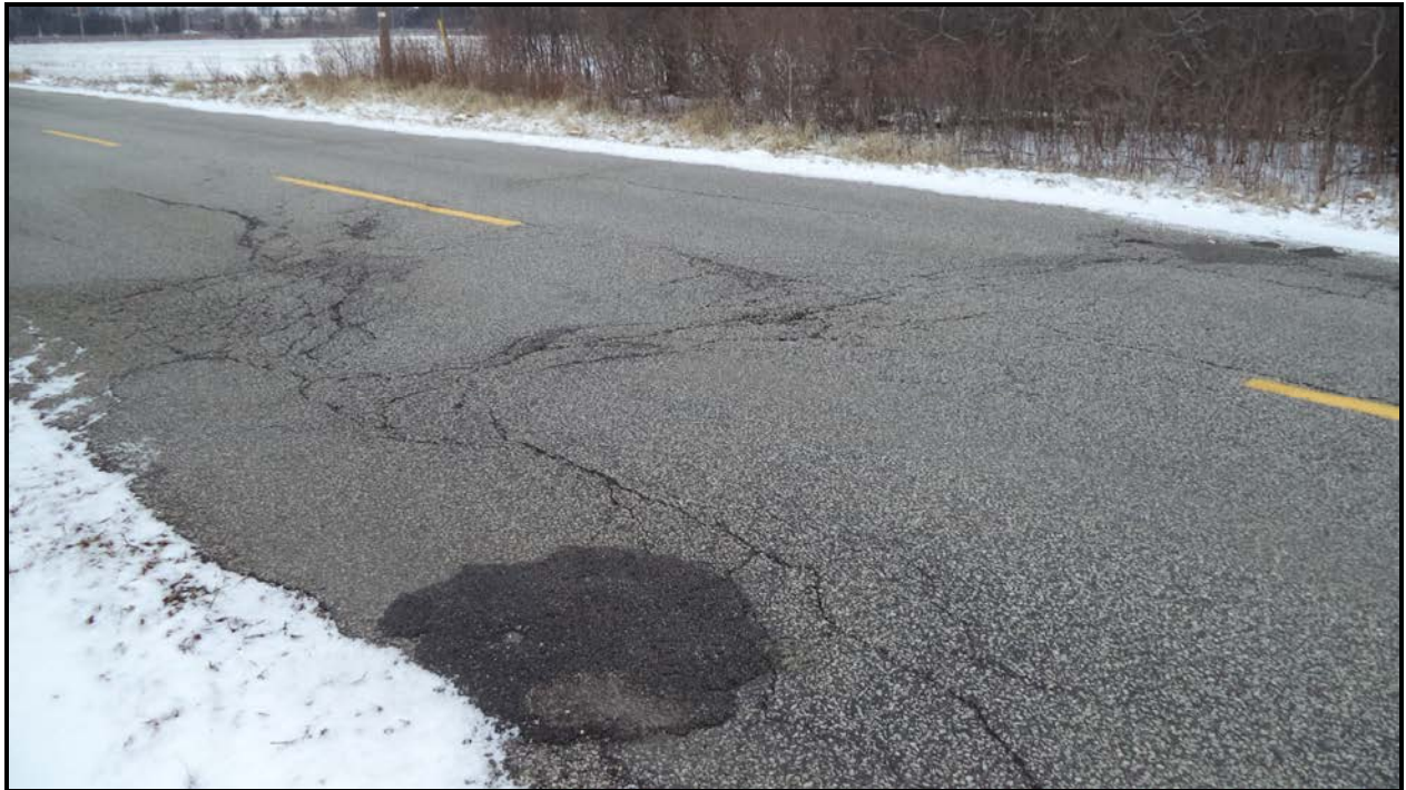
Photograph 7 – Wearing Surface over Culvert
