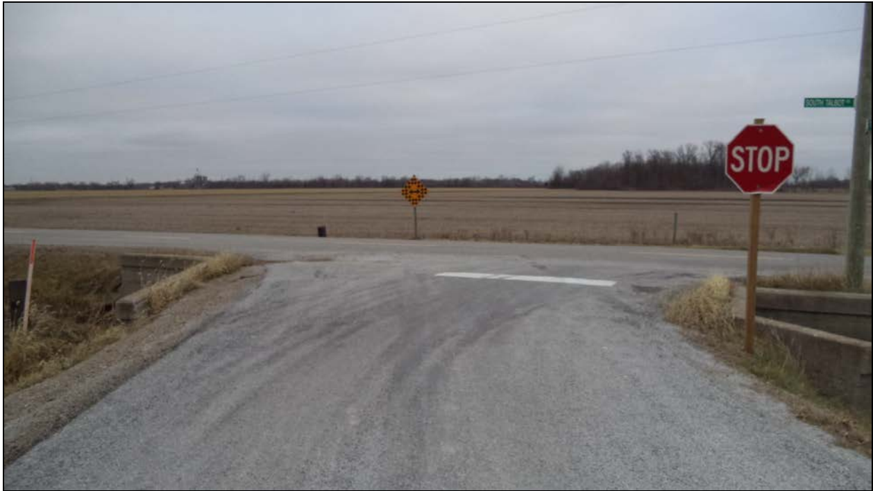
Photograph 1 – Road over Culvert (Looking North)
