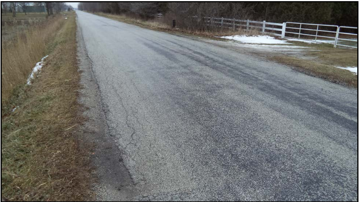
Photograph 10 – Wearing Surface at South Approach
