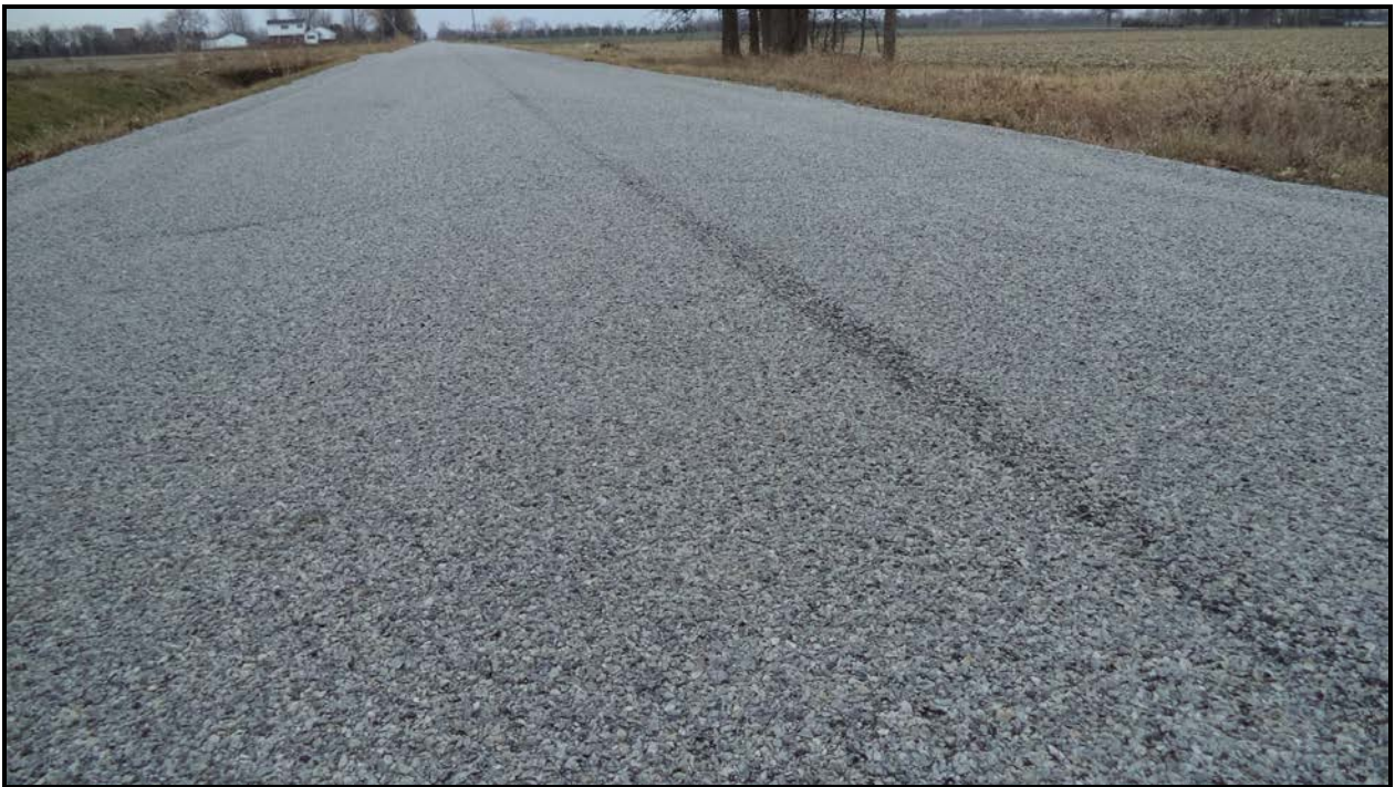
Photograph 6 – Wearing Surface at North Approach (Looking South)
