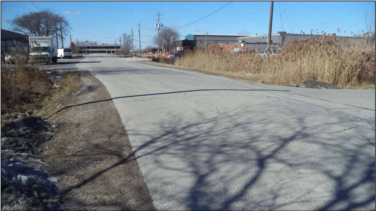
Photograph 1 – Road over Culvert (Looking East)
