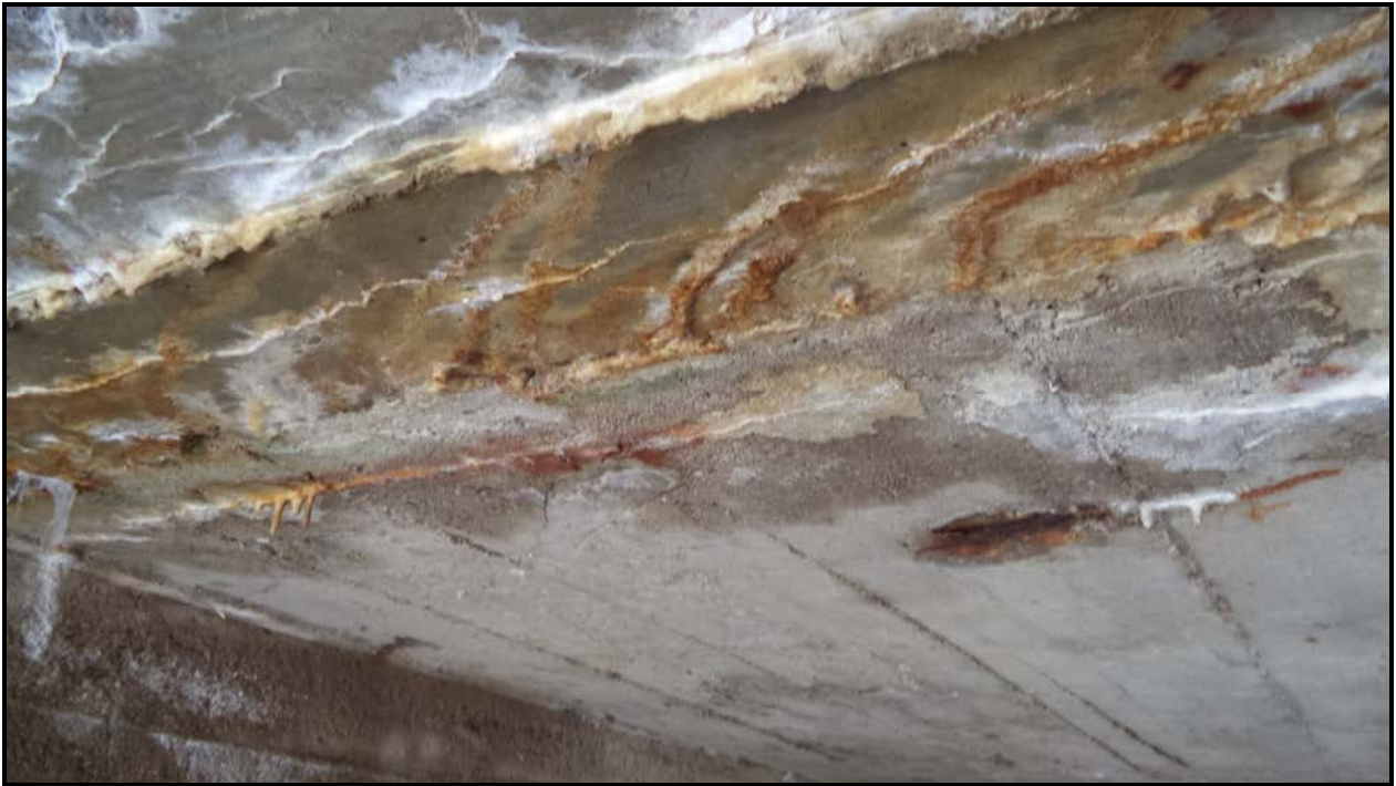
Photograph 3 – Culvert Barrel - Soffit
