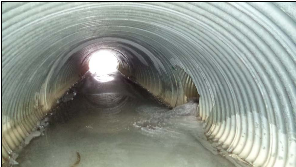
Photograph 2 – Culvert Barrel (Looking West)
