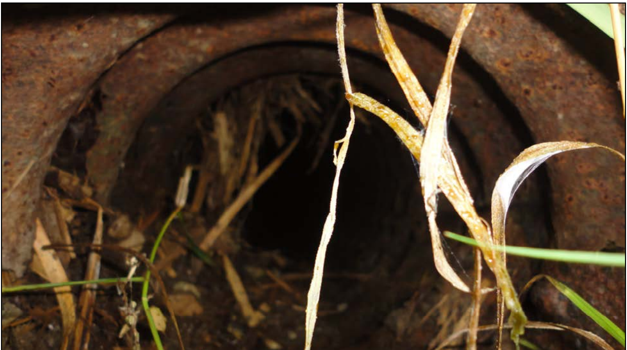
Photograph 6 – Culvert Barrel (Looking West)
