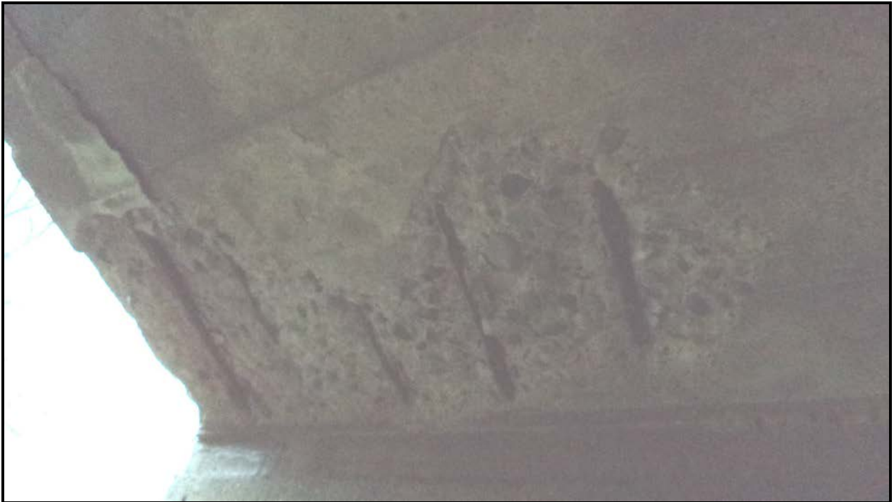
Photograph 3 – Culvert Barrel Soffit
