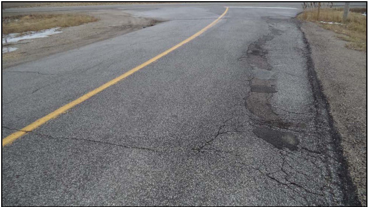
Photograph 6 – Wearing Surface at North Approach
