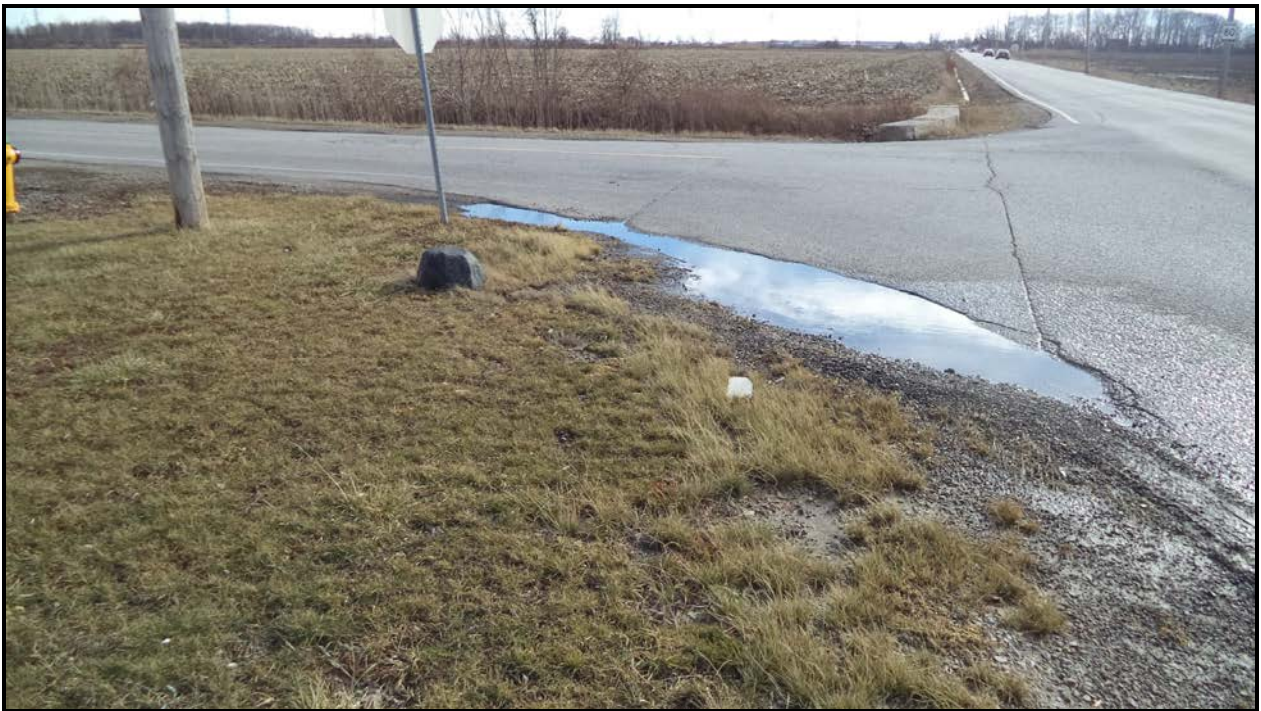
Photograph 4 – Wearing Surface over Culvert (Looking South)
