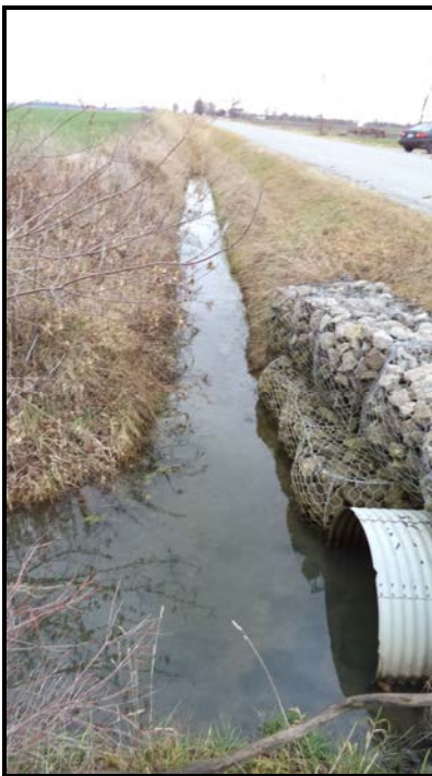
Photograph 8 –Water Stream (Concession Road 9 West Side - Looking North)
