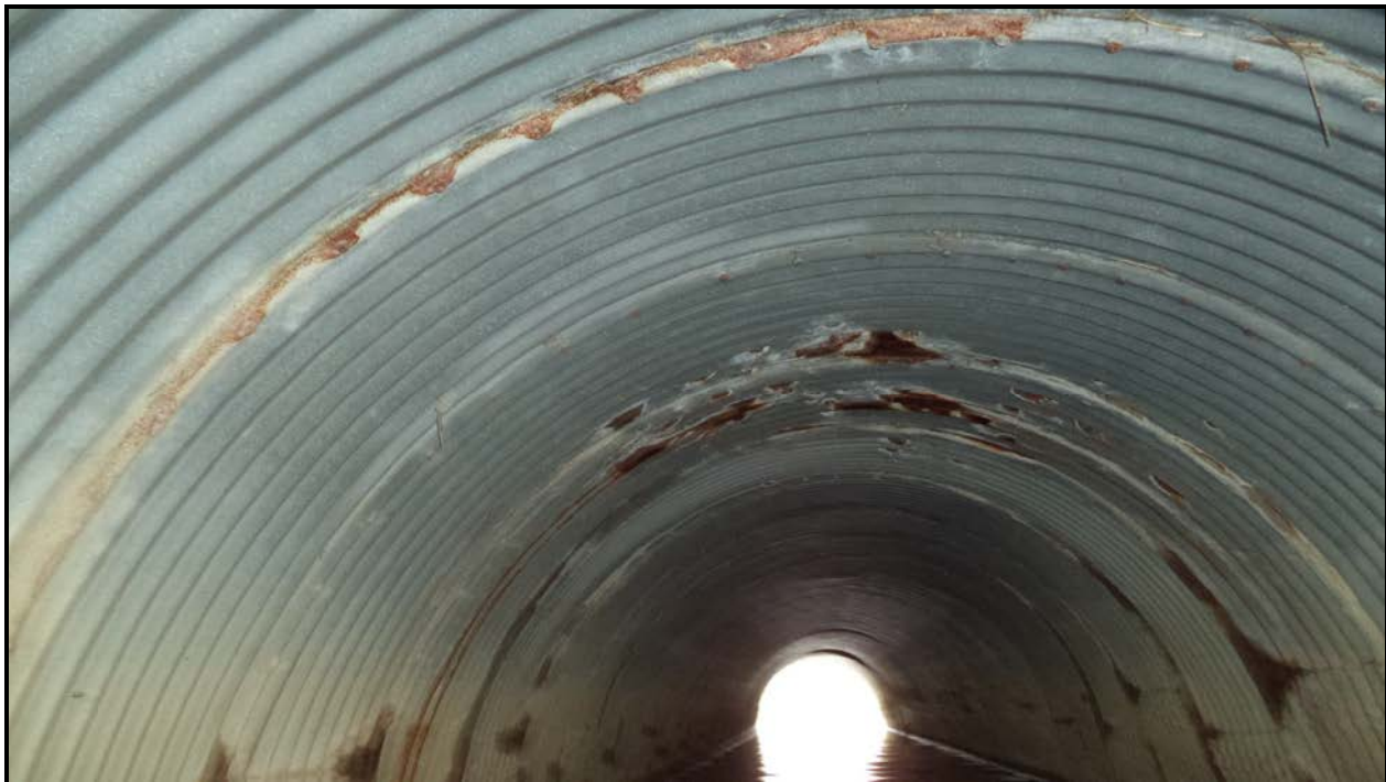
Photograph 2 – Culvert Barrel Top (Looking South)
