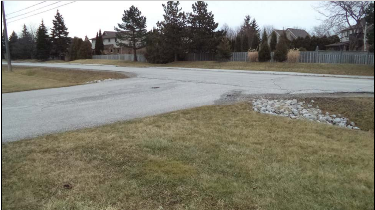
Photograph 1 – Road over Culvert (Looking South)
