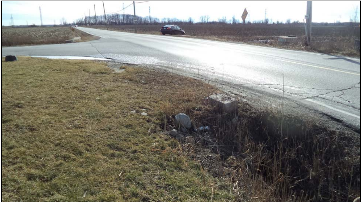
Photograph 1 – Road over Culvert (Looking North)
