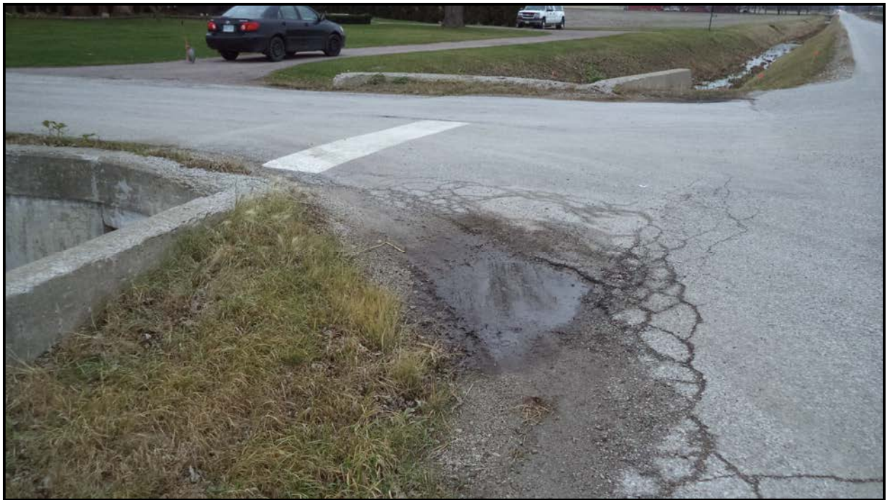
Photograph 9 – Wearing Surface over Culvert (Looking West)
