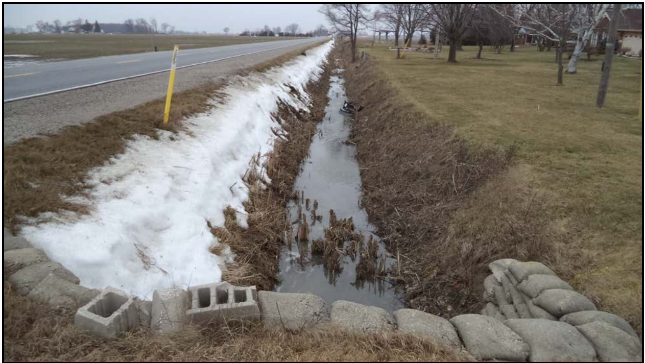
Photograph 10 – Water Stream (Concession Road 11 West Side - Looking West)
