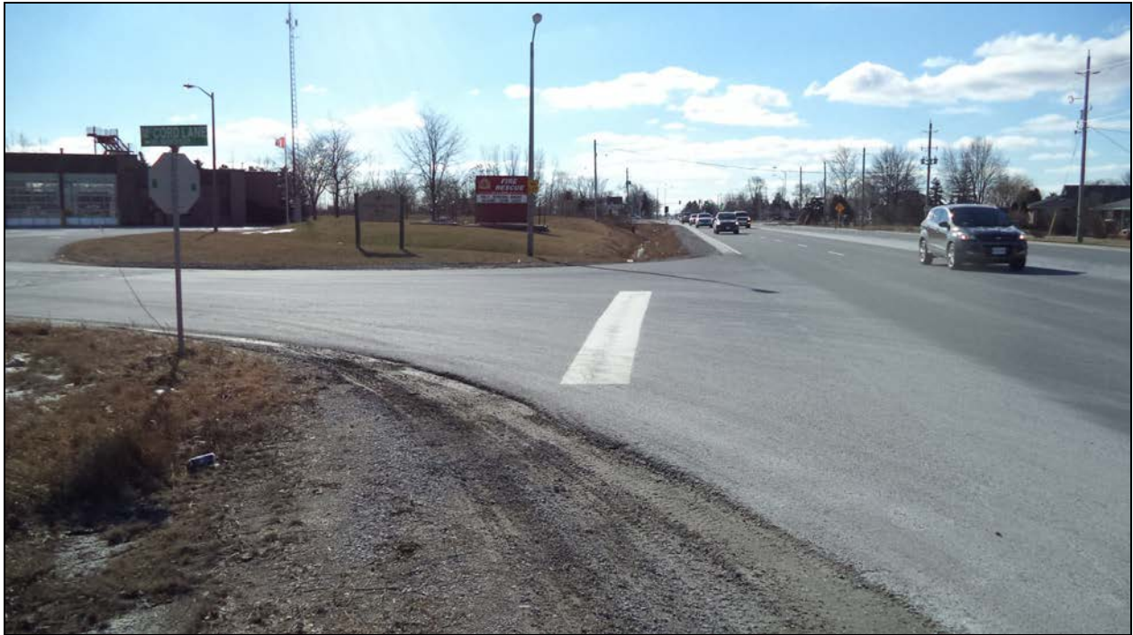
Photograph 1 – Road over Culvert (Looking North)
