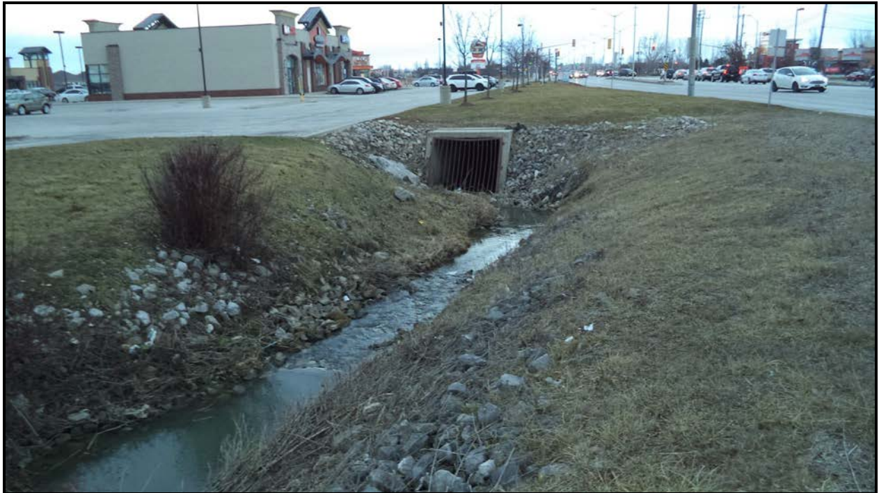
Photograph 1 – Road over Culvert (Looking North)
