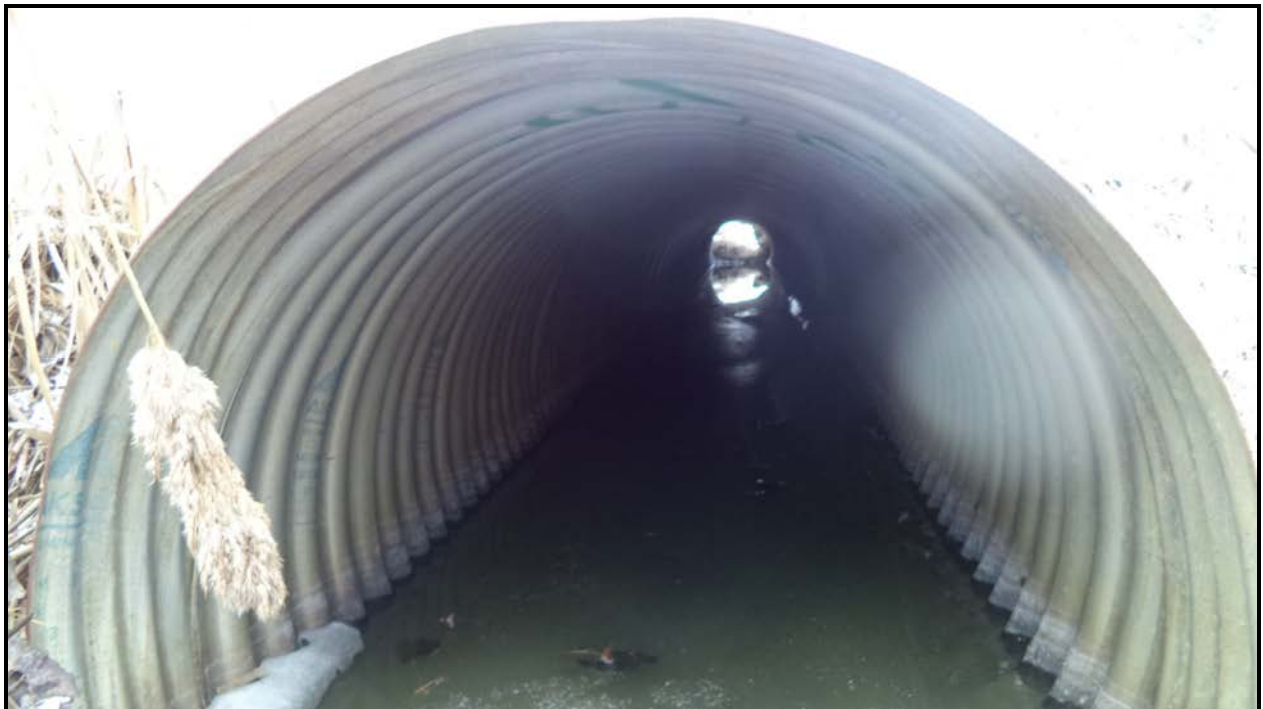
Photograph 2 – Culvert Barrel (Looking South)
