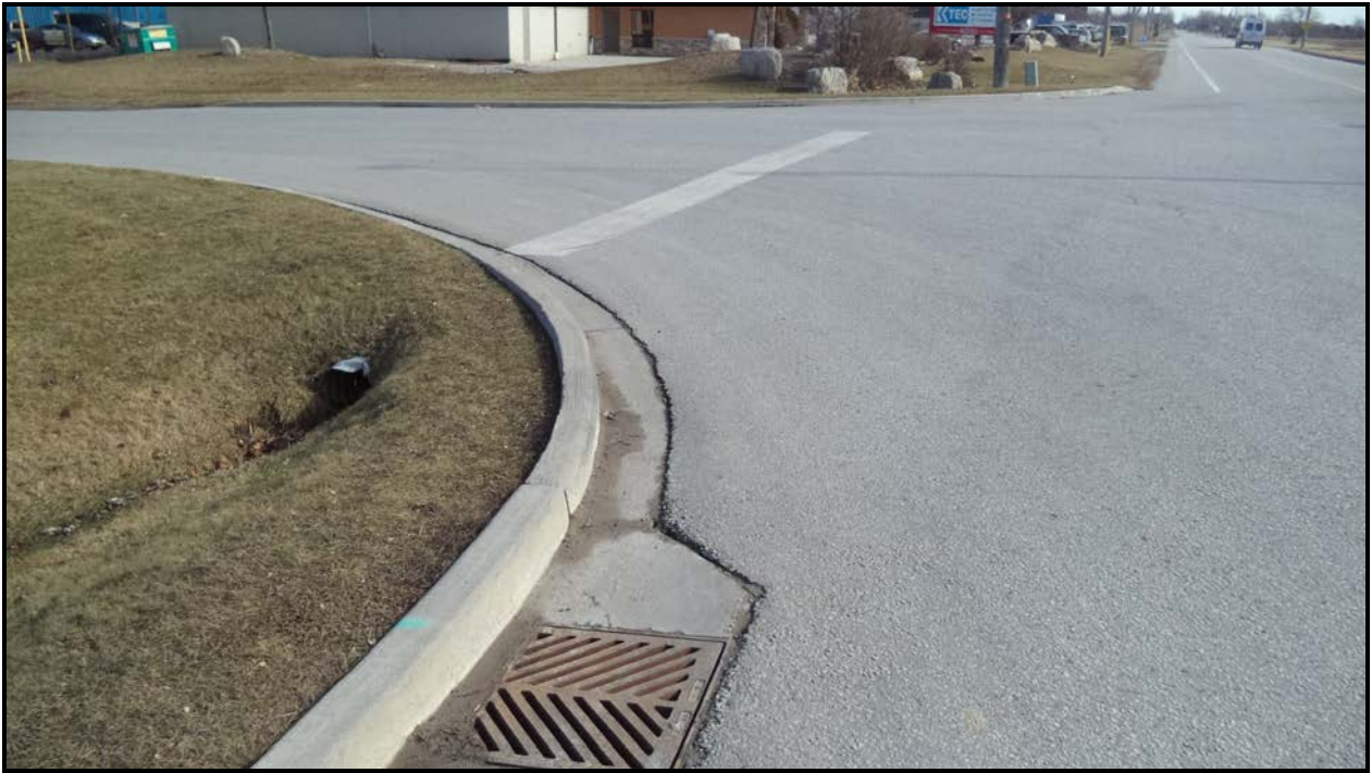
Photograph 6 – Wearing Surface over Culvert (Looking East)
