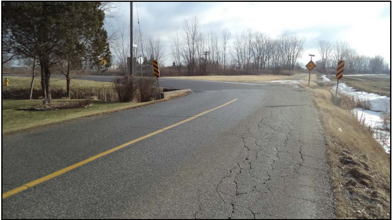
Photograph 1 – Road over Culvert (Looking South)
