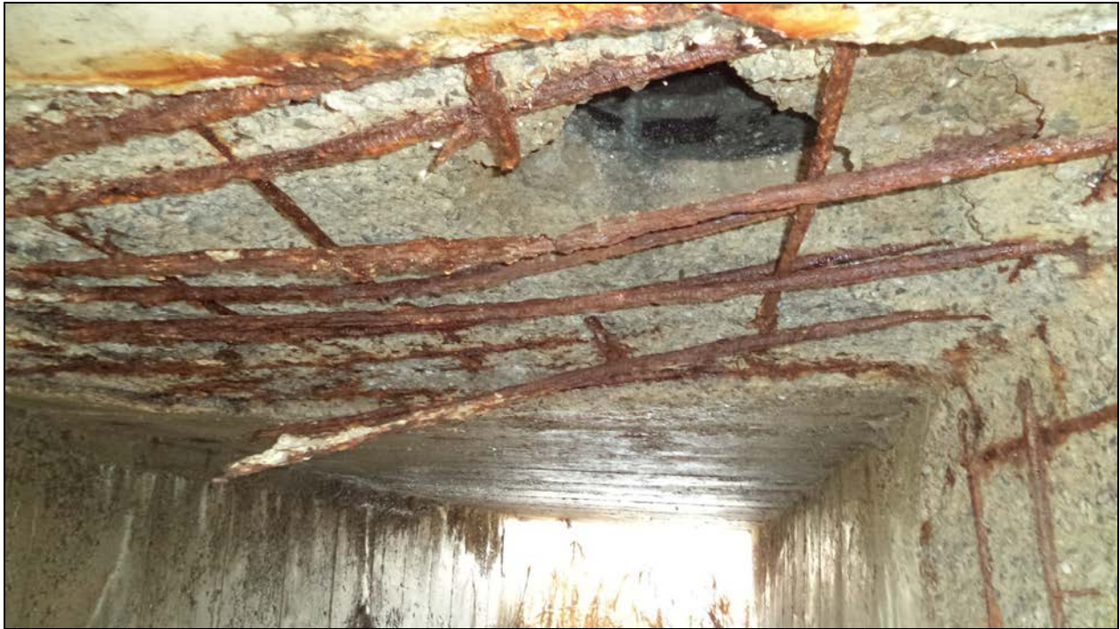
Photograph 3 – Culvert Barrel (Looking South)
