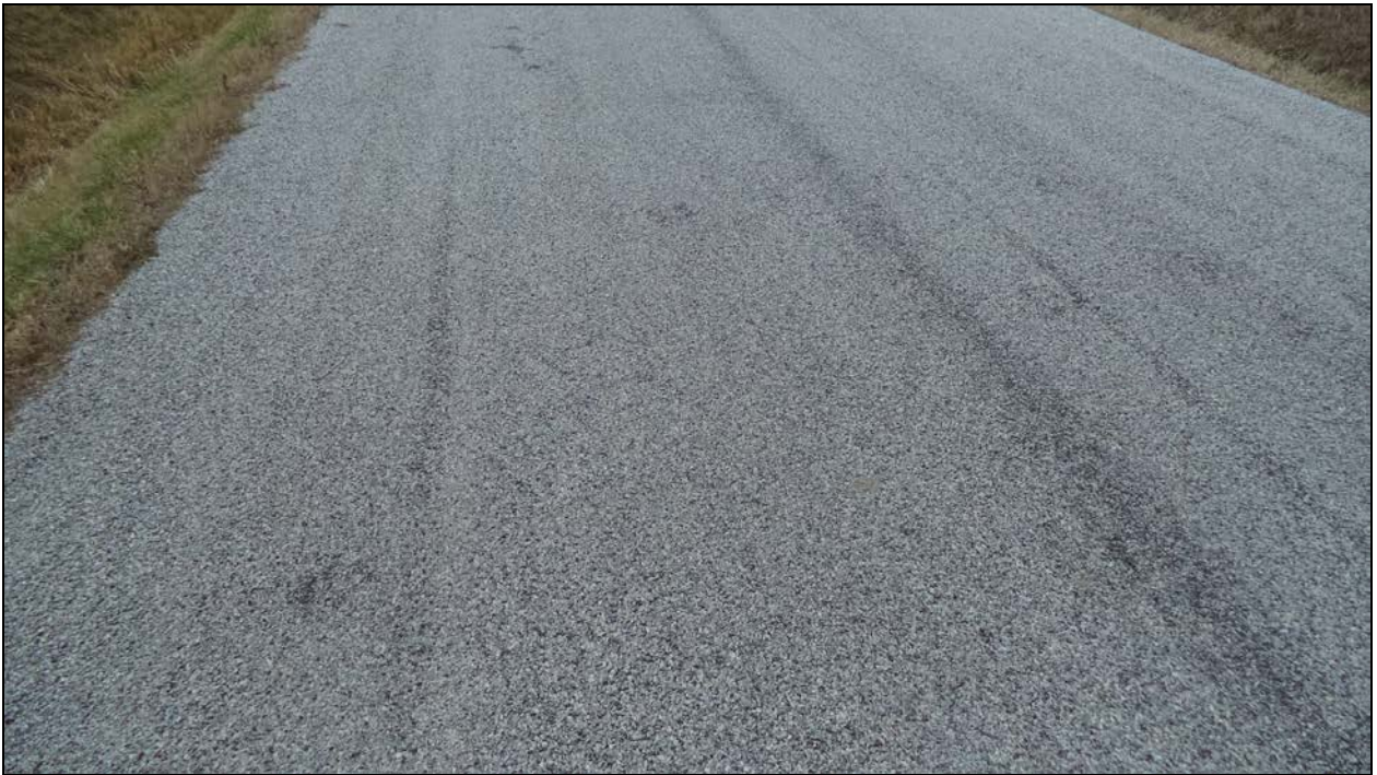
Photograph 6 – Wearing Surface at North Approach (Looking South)
