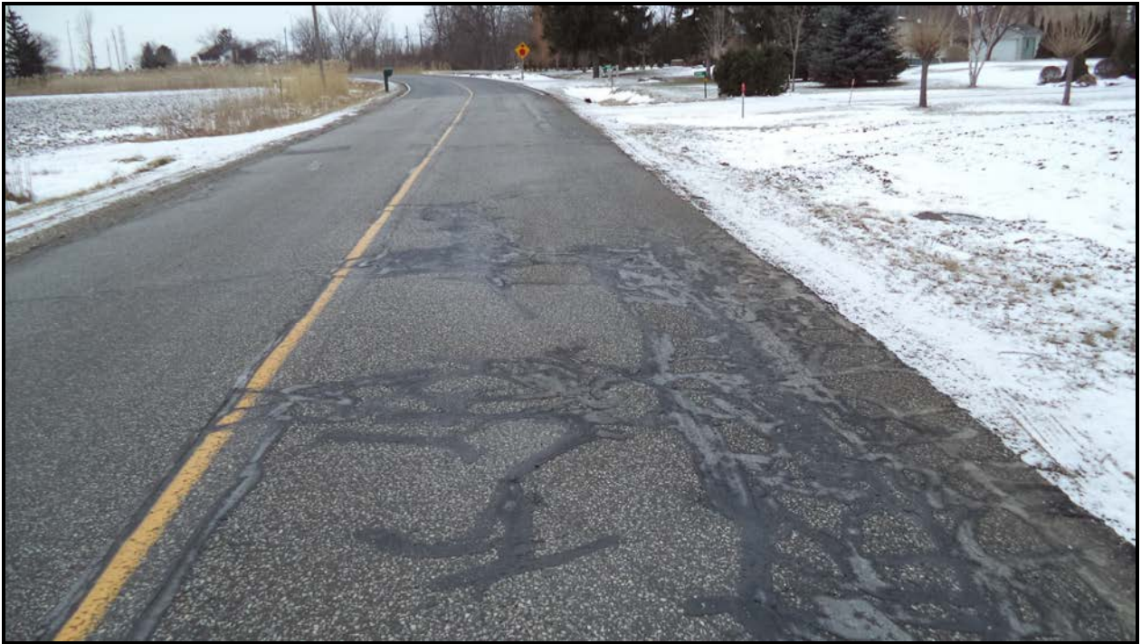
Photograph 5 – Wearing Surface over Culvert (Looking South)
