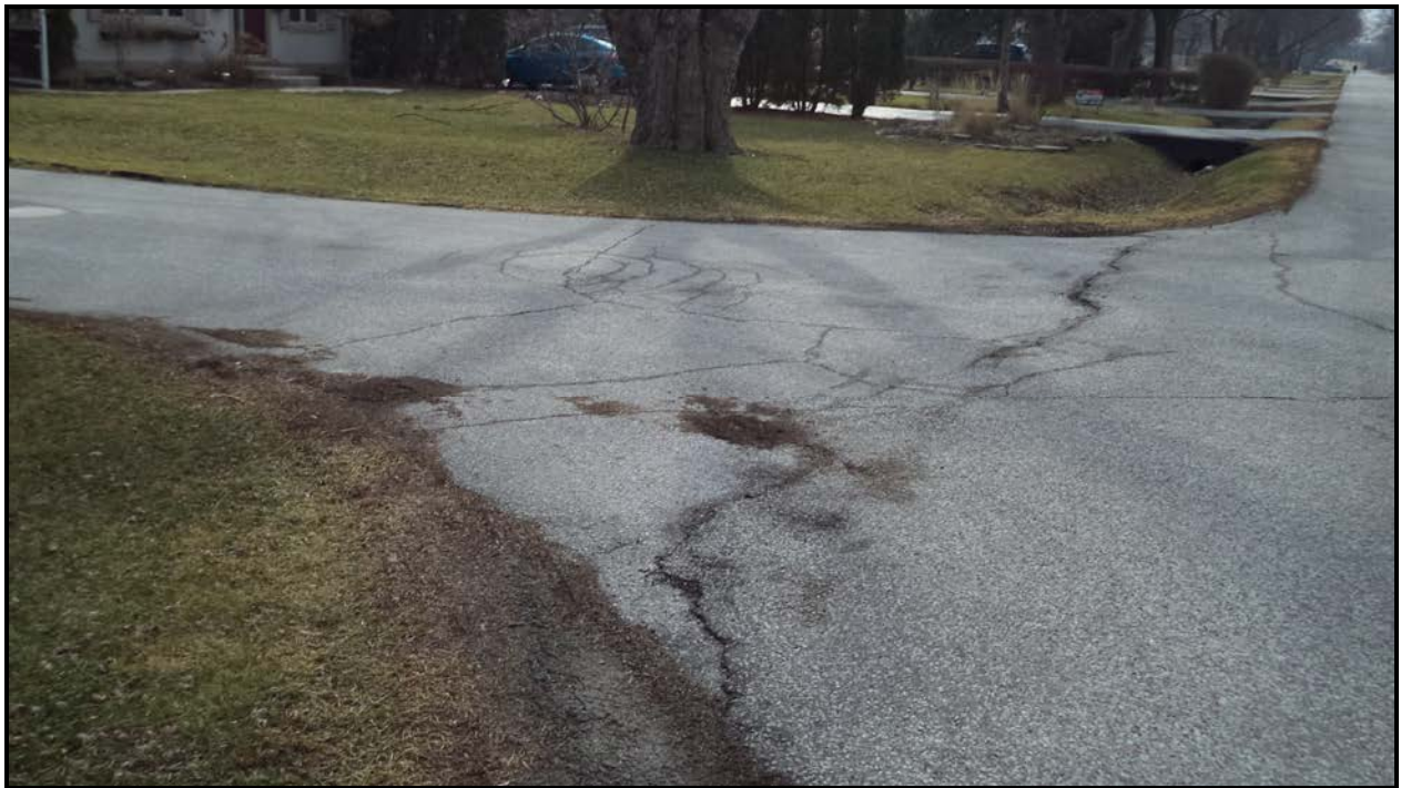
Photograph 6 – Wearing Surface over Culvert (Looking South)
