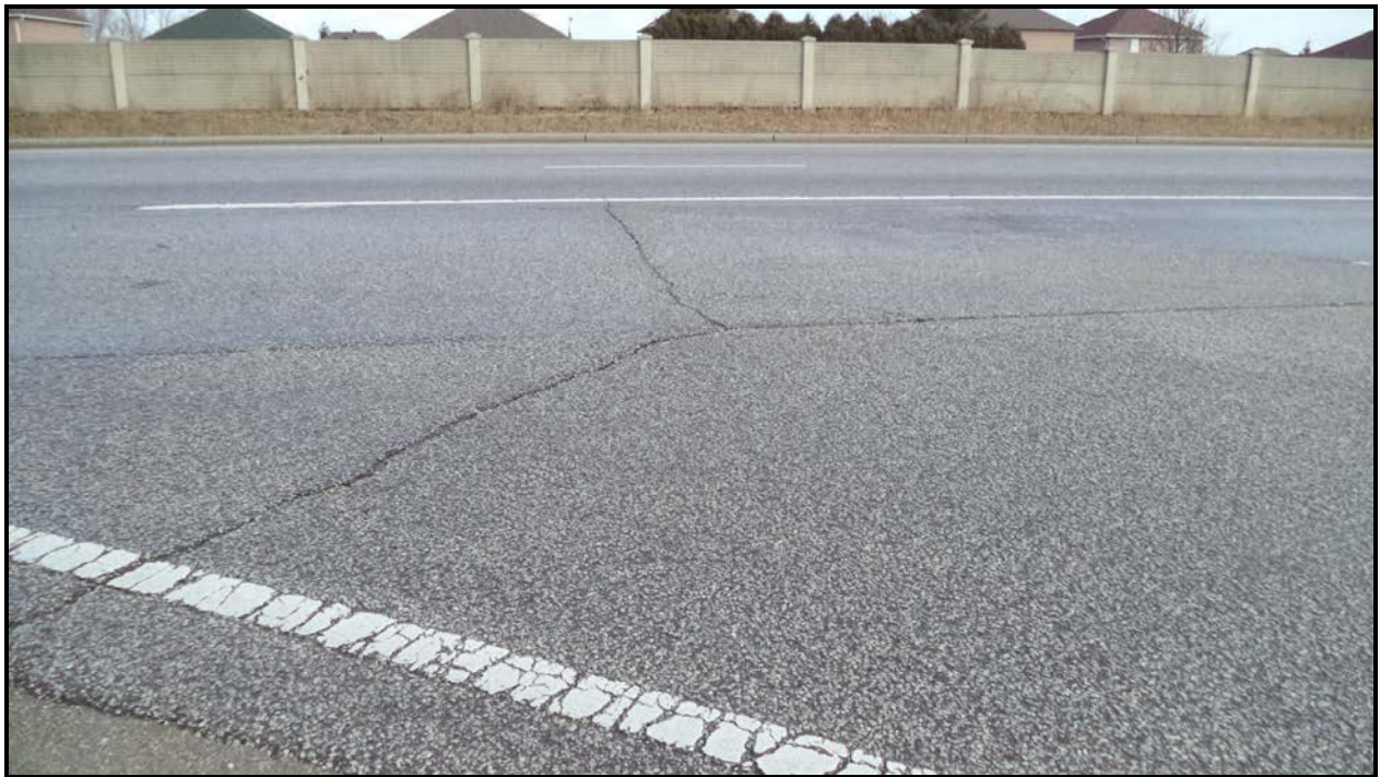
Photograph 6 – Wearing Surface at North Approach
