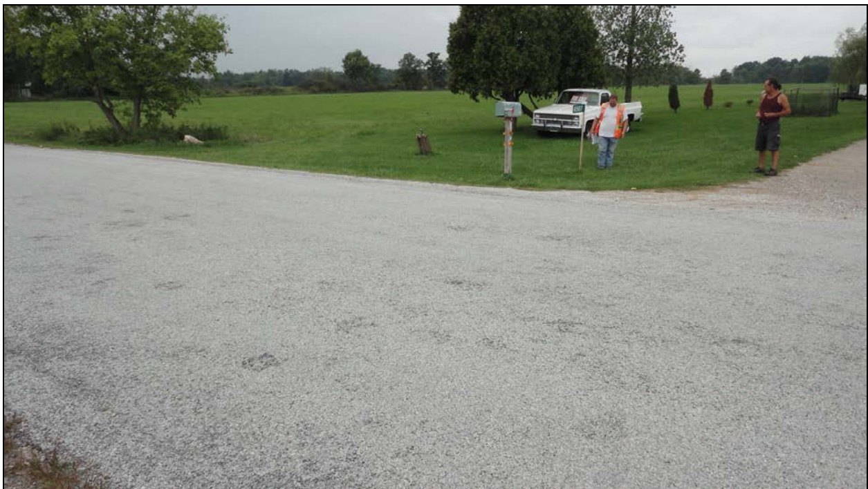
Photograph 2 – Wearing Surface over Culvert (Looking West)
