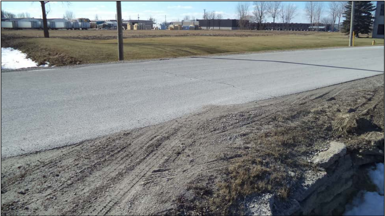
Photograph 1 – Road over Culvert (Looking South)
