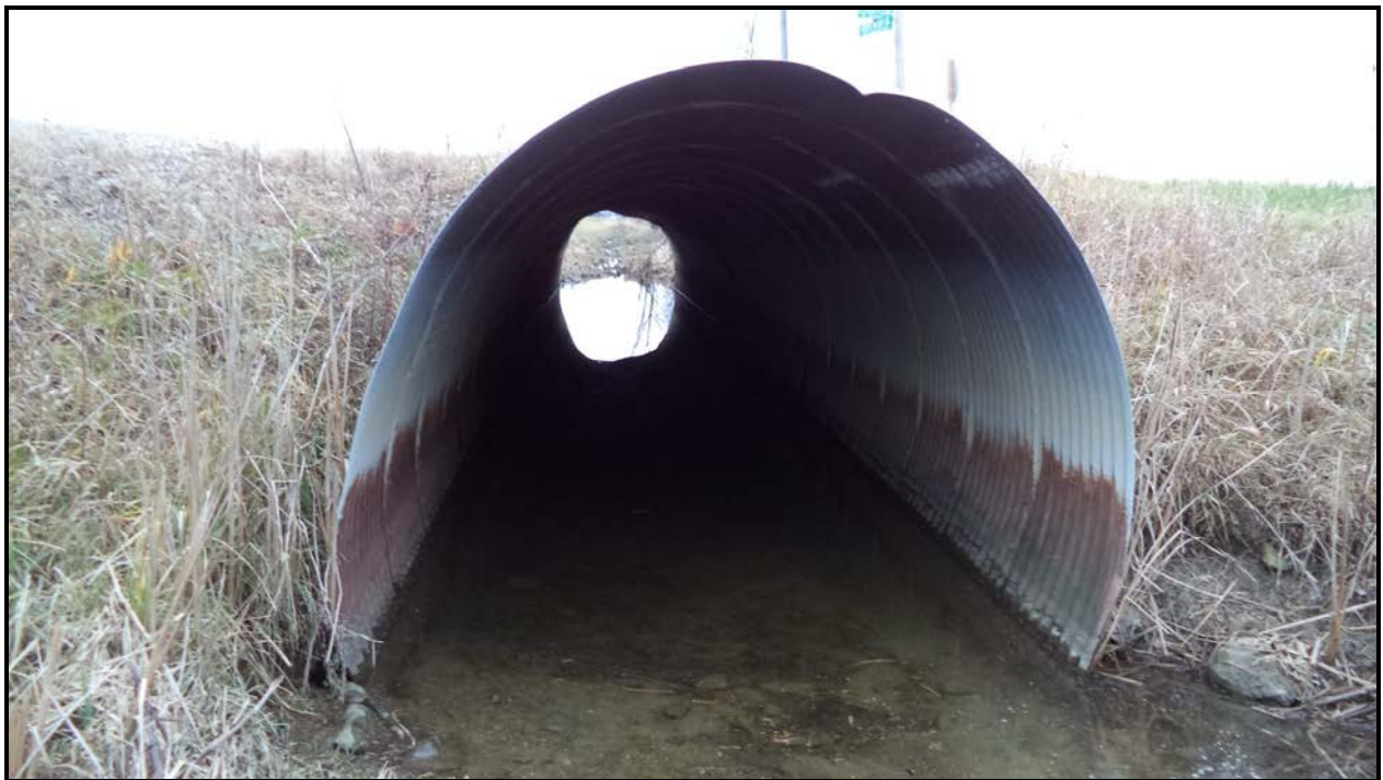
Photograph 4 – Culvert Barrel (Looking East)
