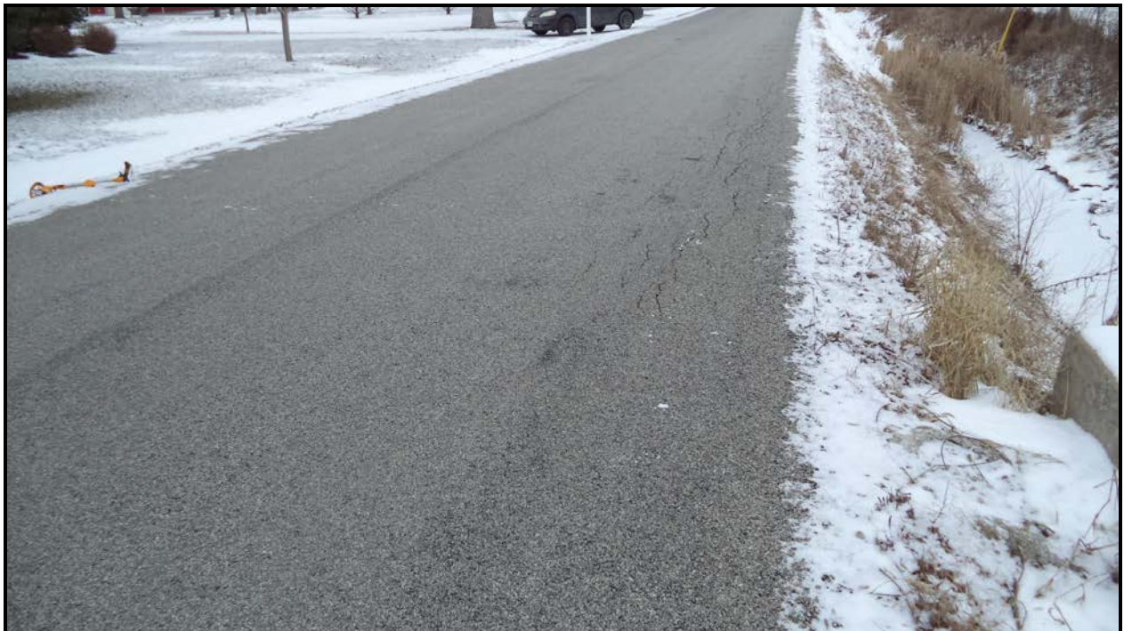
Photograph 8 – Wearing Surface over Culvert (Looking North)
