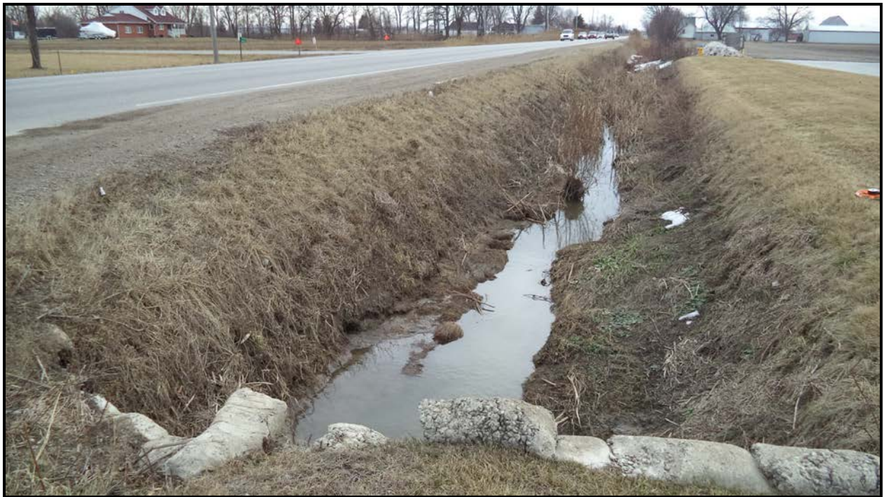
Photograph 10 – Water Stream (Manning Road West Side - Looking South)
