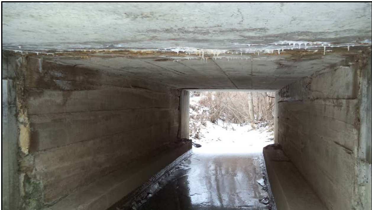
Photograph 2 – Culvert Barrel (Looking West)
