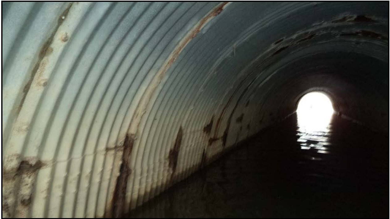
Photograph 3 – Culvert Barrel Side (Looking South)
