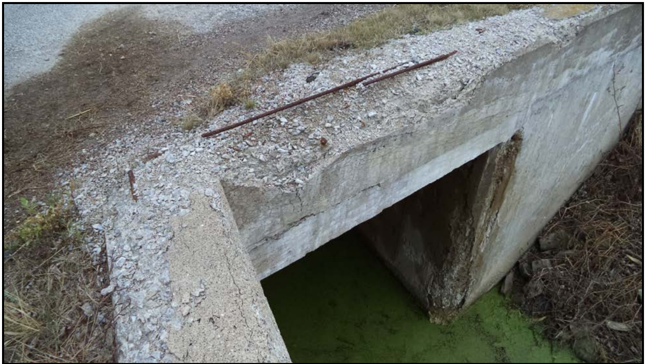
Photograph 8 – Headwall (West Elevation)
