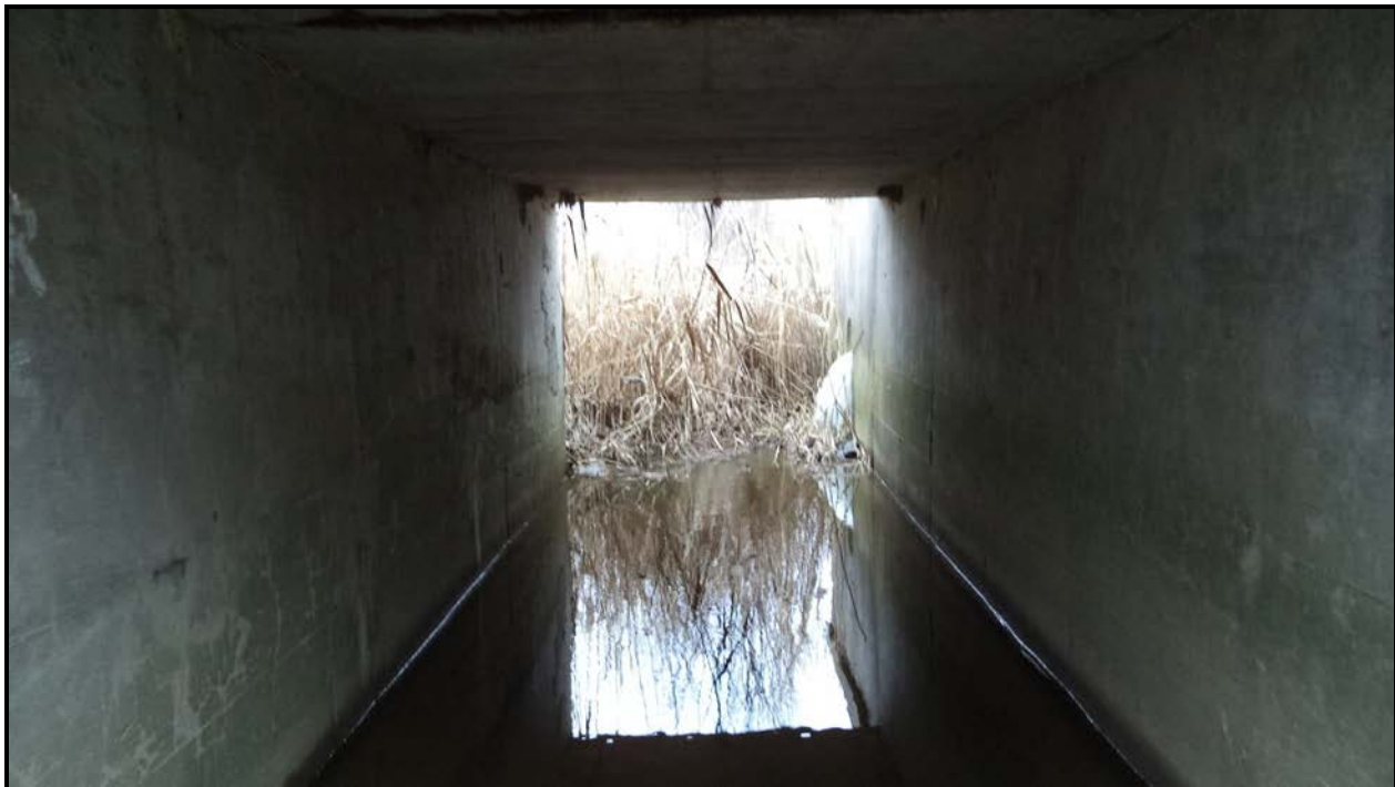
Photograph 2 – Culvert Barrel (Looking West)
