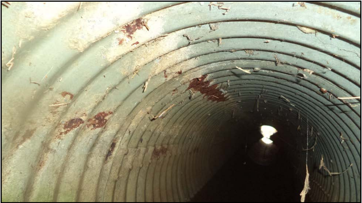
Photograph 3 – Culvert Barrel Top
