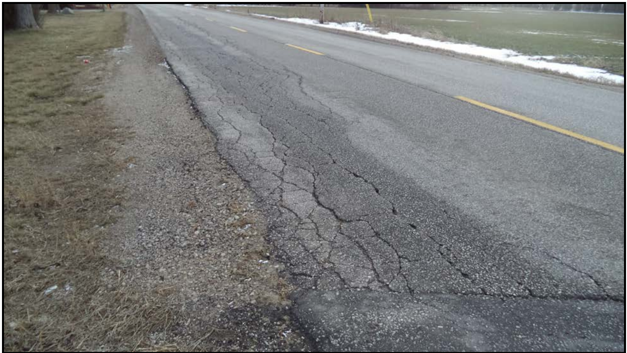
Photograph 6 – Wearing Surface at East Approach
