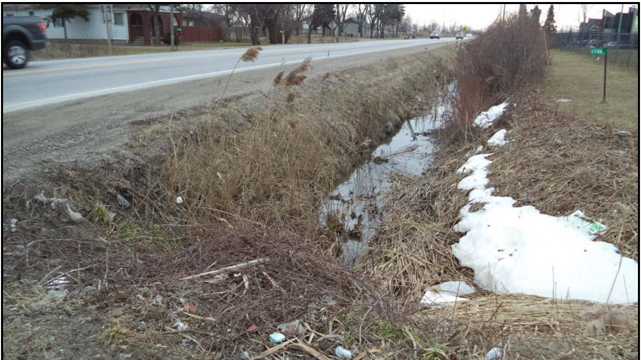
Photograph 10 – Water Stream (Manning Road West Side - Looking South)
