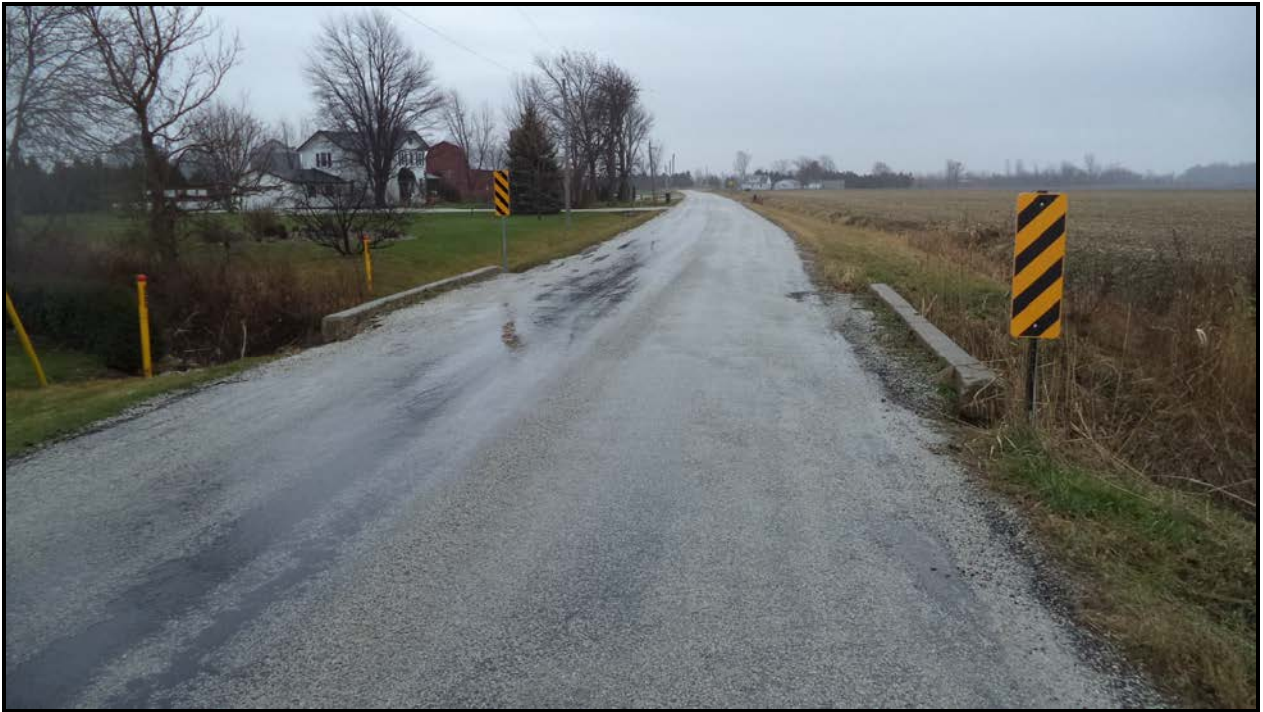
Photograph 1 – Road over Culvert (Looking South)
