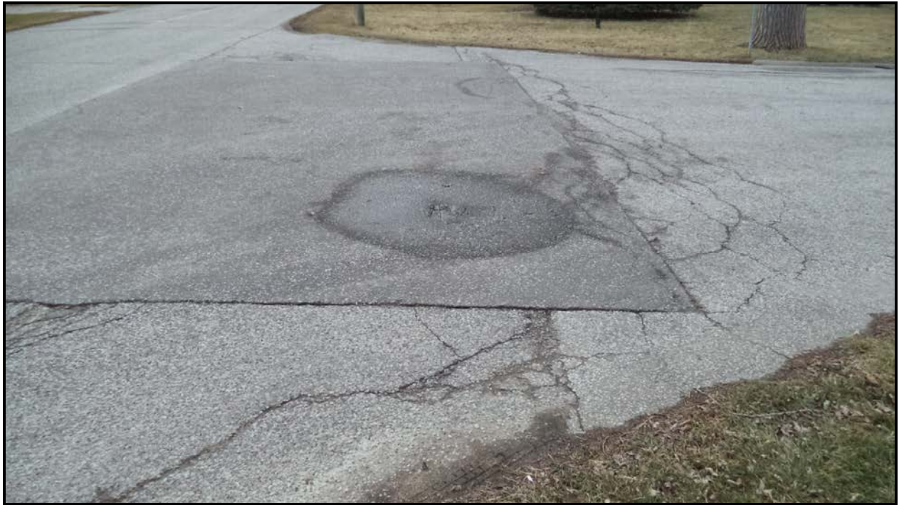
Photograph 5 – Wearing Surface over Culvert (Looking South)
