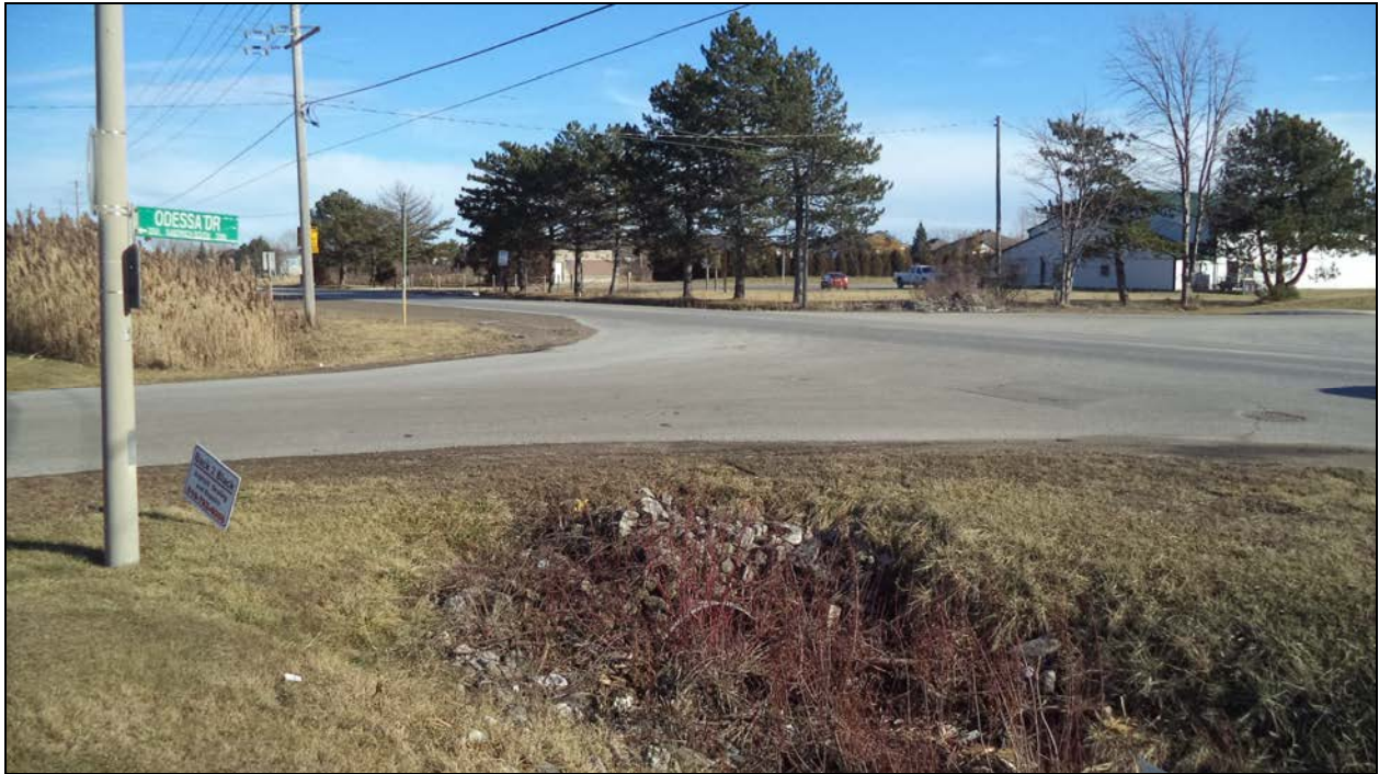
Photograph 1 – Road over Culvert (Looking West)
