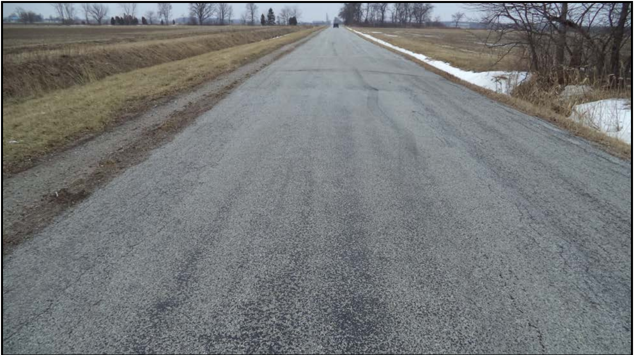
Photograph 1 – Road over Culvert (Looking South)
