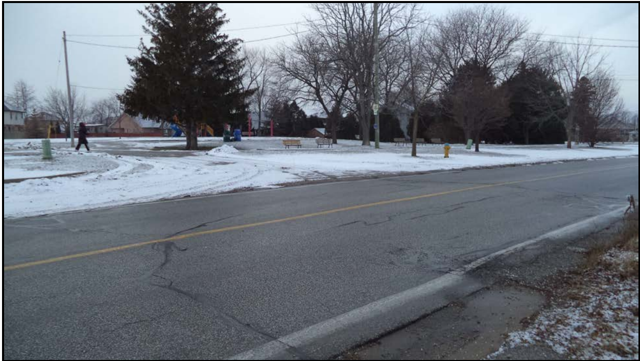
Photograph 1 – Road over Culvert (Looking South)
