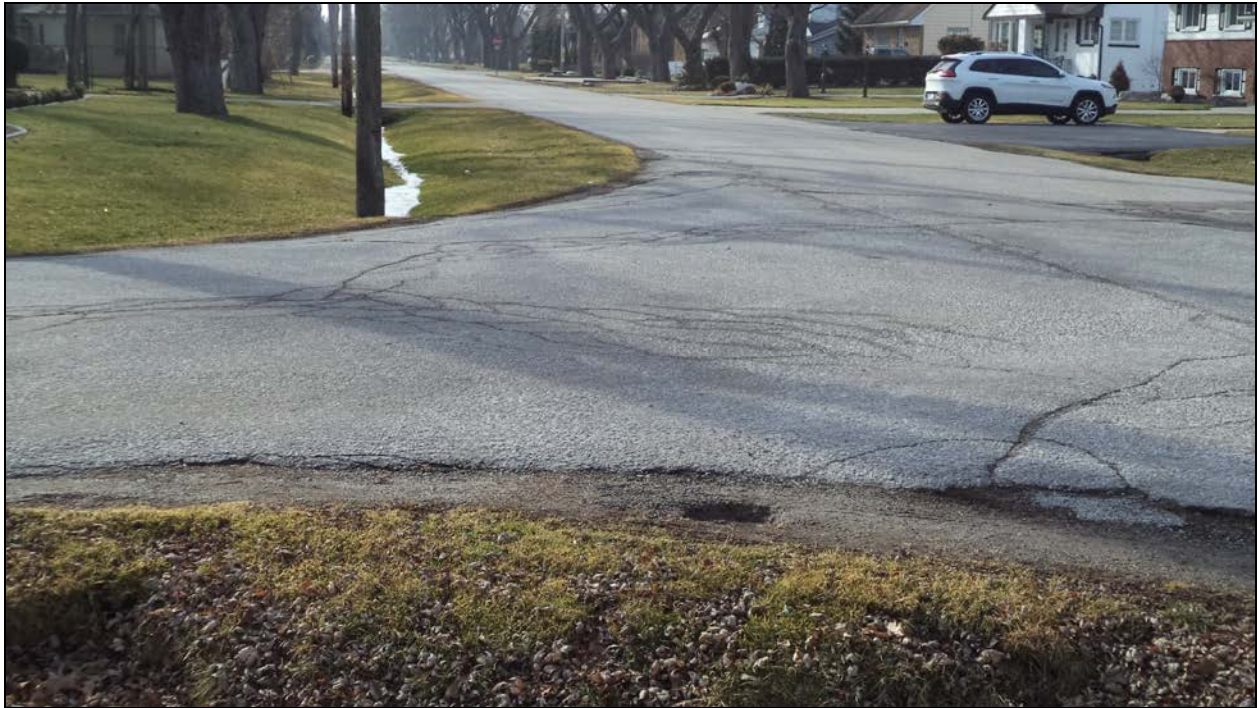
Photograph 1 – Road over Culvert (Looking West)
