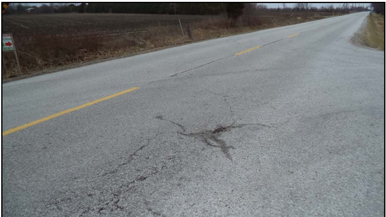
Photograph 6 – Wearing Surface at North Approach (Looking East)
