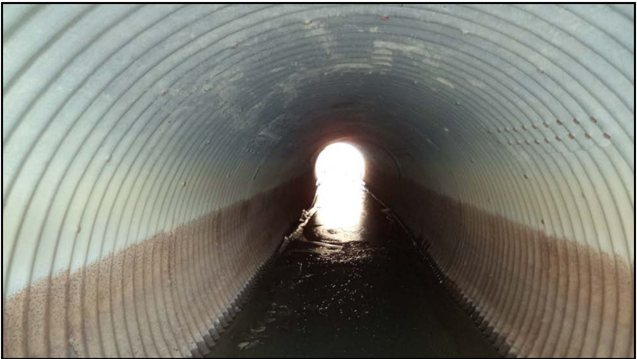
Photograph 2 – Culvert Barrel
