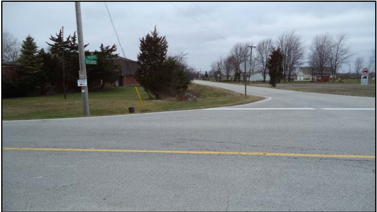
Photograph 5 – Wearing Surface over Culvert (Looking West)
