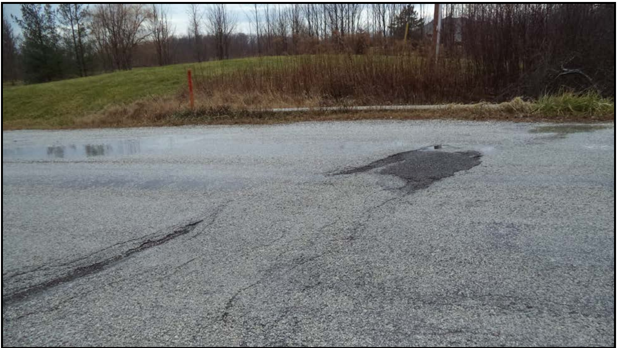
Photograph 2 – Wearing Surface over Culvert (Looking West)
