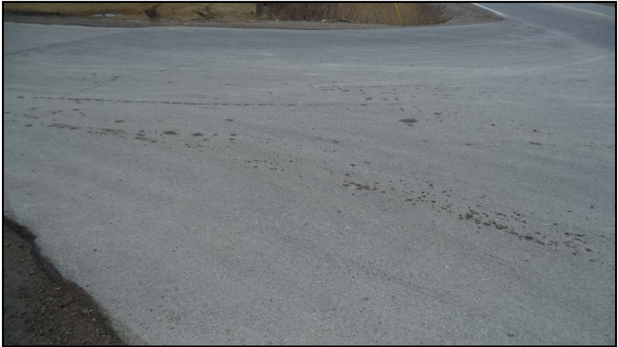
Photograph 7 – Wearing Surface over Culvert (Looking North)
