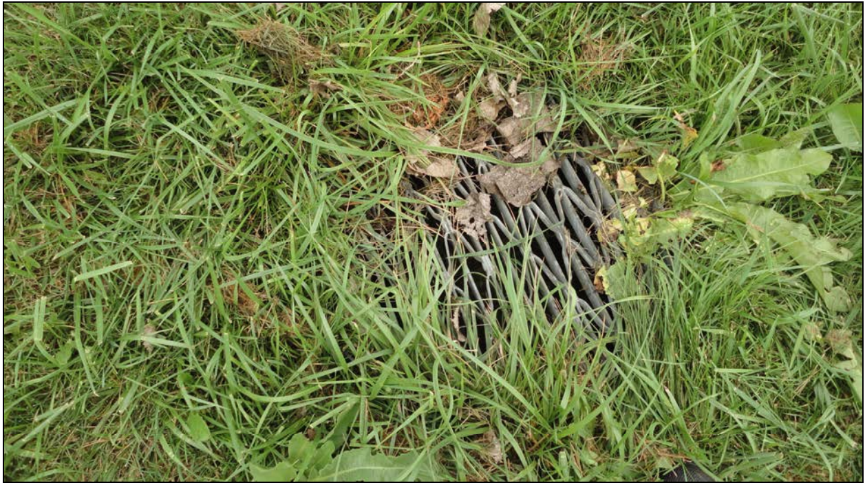
Photograph 3 – Inlet Manhole at West Elevation
