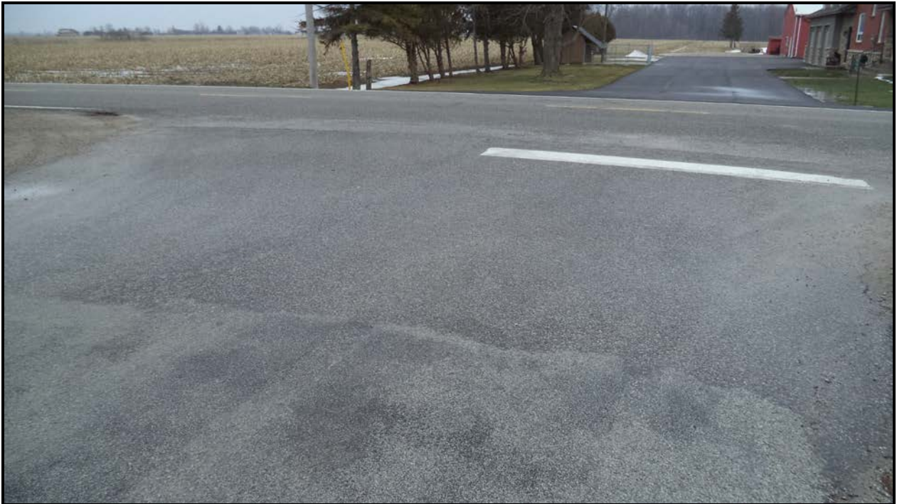
Photograph 5 – Wearing Surface over Culvert (Looking South)
