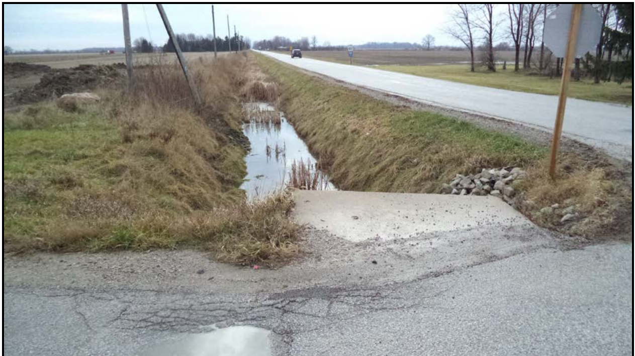
Photograph 10 – Water Stream (South Talbot Road South Side - Looking South)
