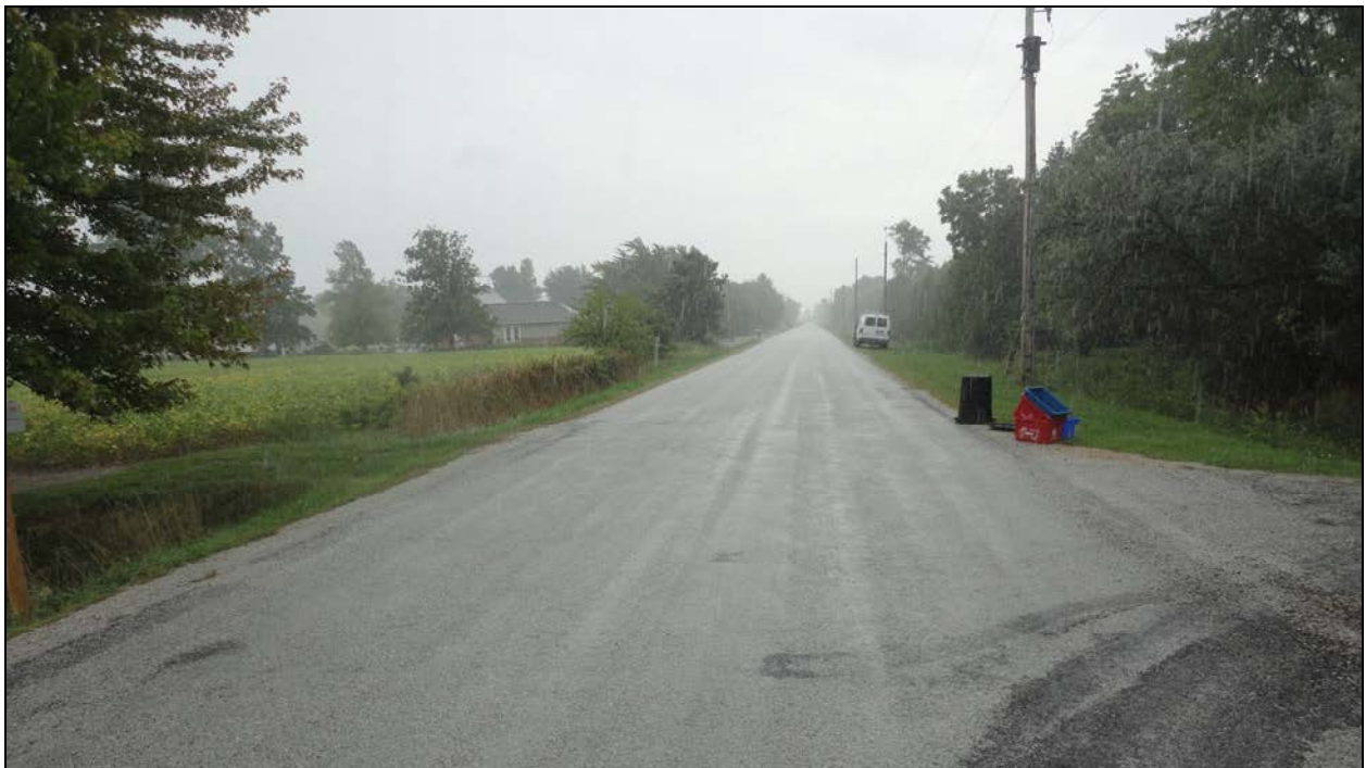
Photograph 2 – Wearing Surface over Culvert (Looking South)
