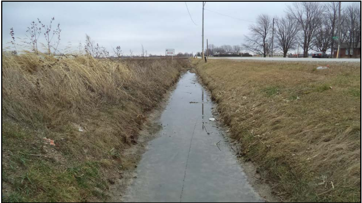
Photograph 7 – Water Stream (Sexton Side Road East Side – Looking East)
