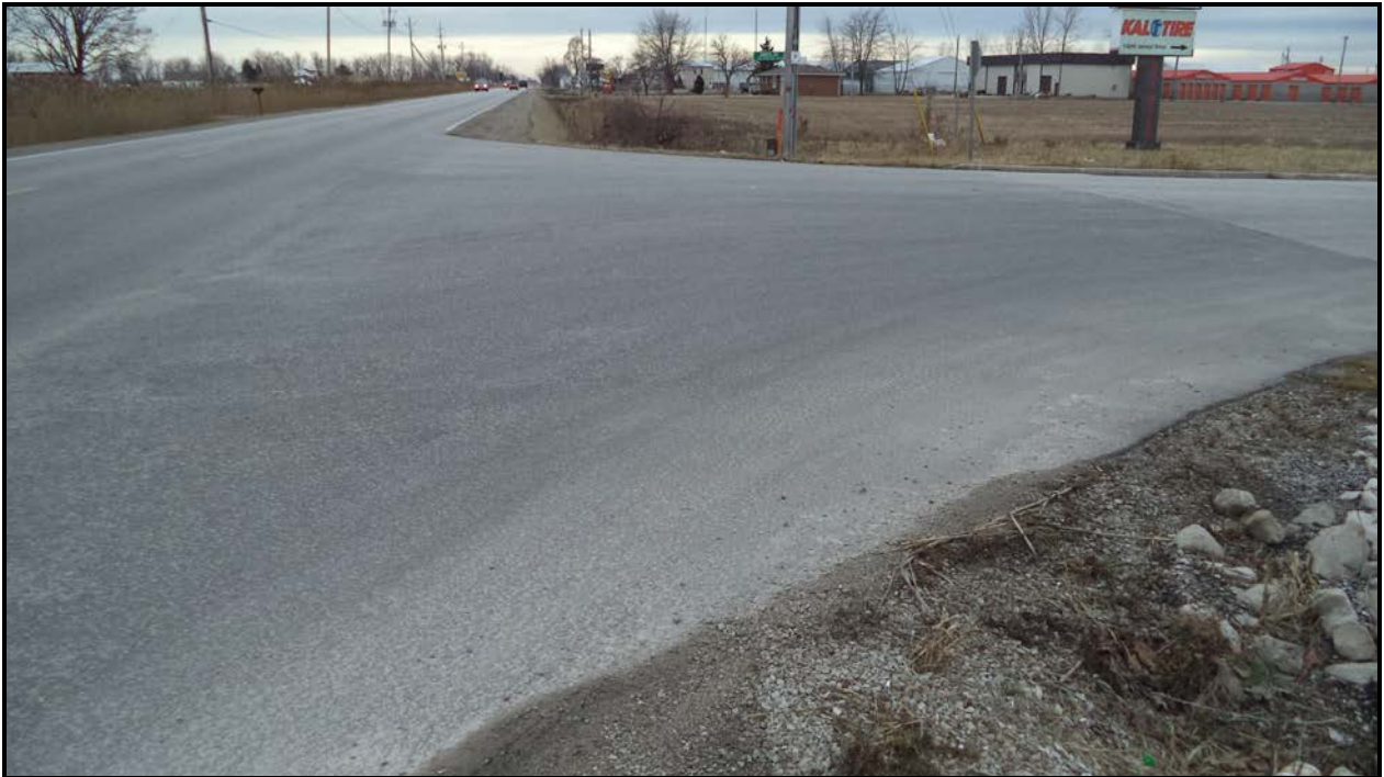
Photograph 5 – Wearing Surface over Culvert (Looking North)
