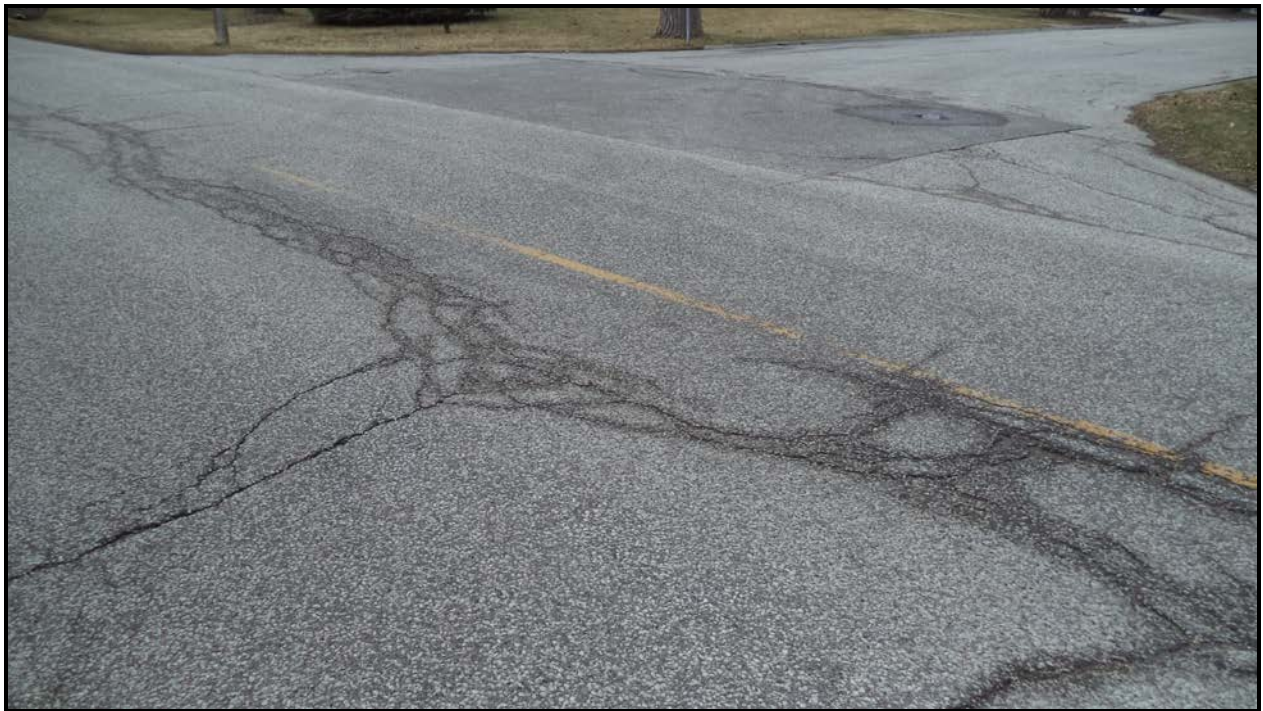
Photograph 6 – Wearing Surface at East Approach
