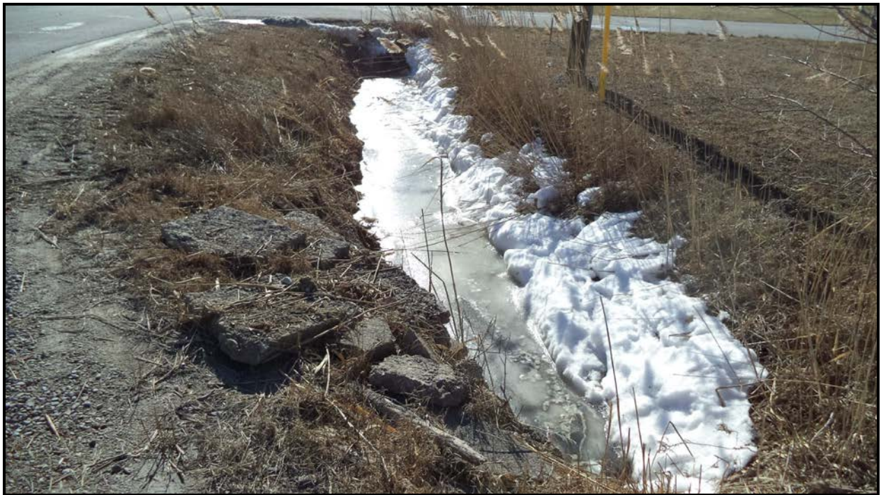
Photograph 8 – Water Stream (Moyanahan Street South Side - Looking South)
