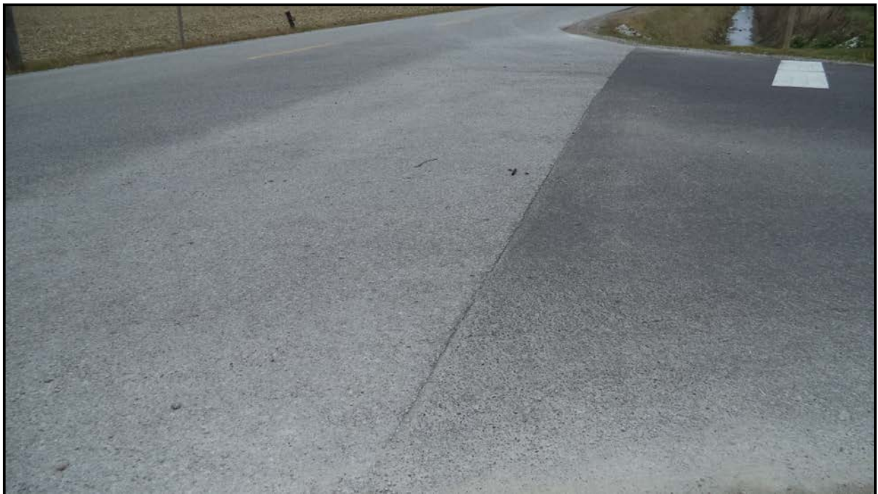
Photograph 6 – Wearing Surface at South Approach
