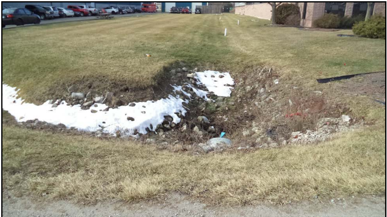
Photograph 6 – Water Stream (Ure Street West Side - Looking West)
