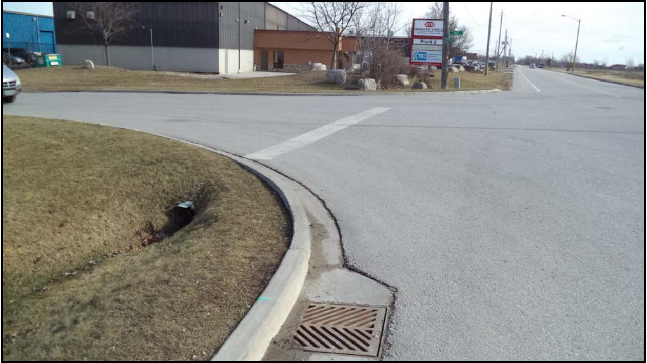
Photograph 1 – Road over Culvert (Looking North)
