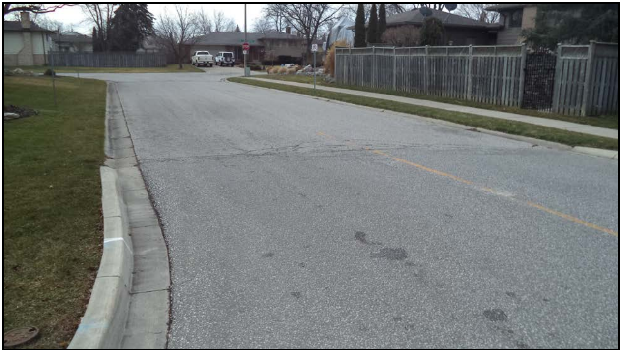
Photograph 8 – Wearing Surface at South Approach
