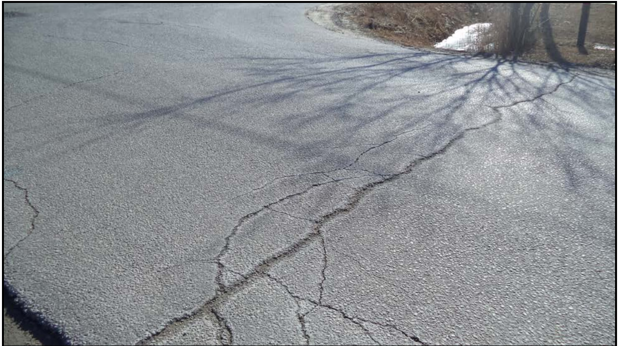
Photograph 7 – Wearing Surface over Culvert (Looking South)
