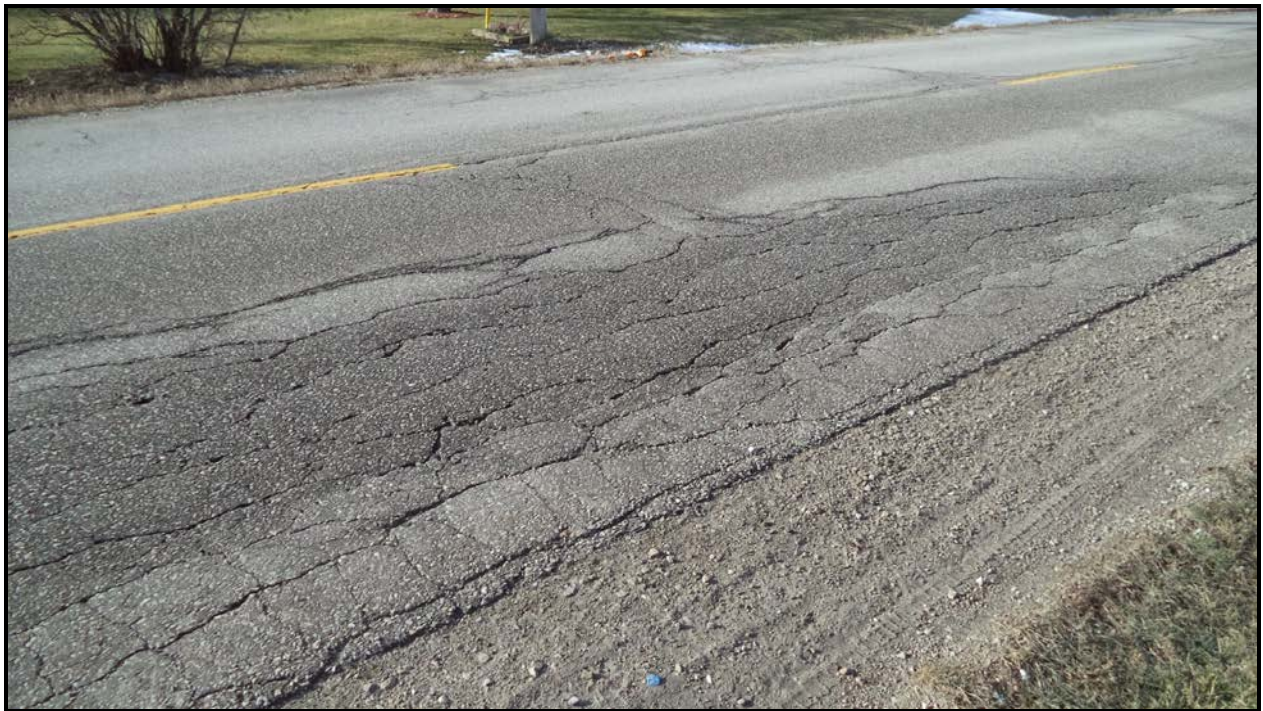
Photograph 6 – Wearing Surface at East Approach
