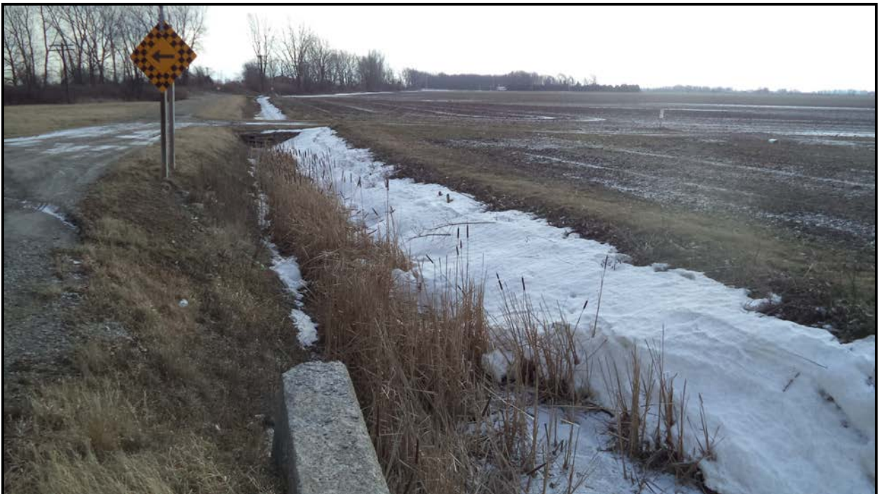
Photograph 8 – Water Stream (North Talbot Road South Side - Looking East)
