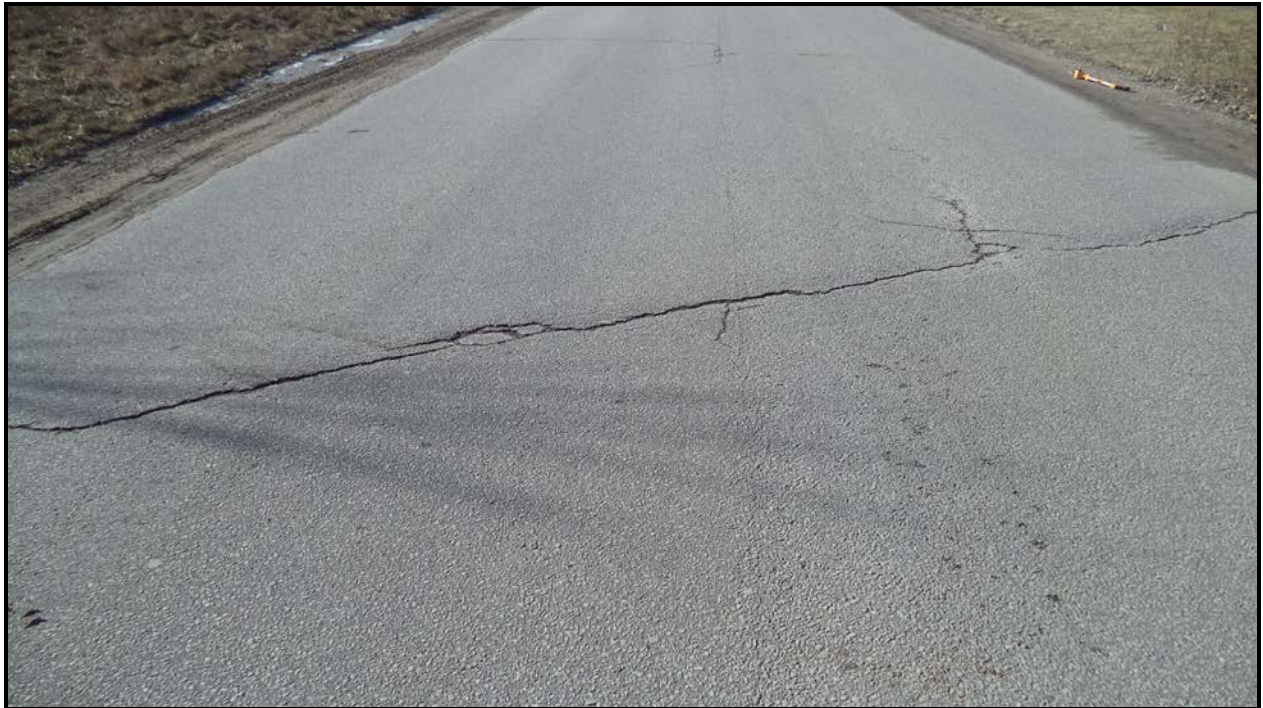
Photograph 5 – Wearing Surface over Culvert (Looking South)
