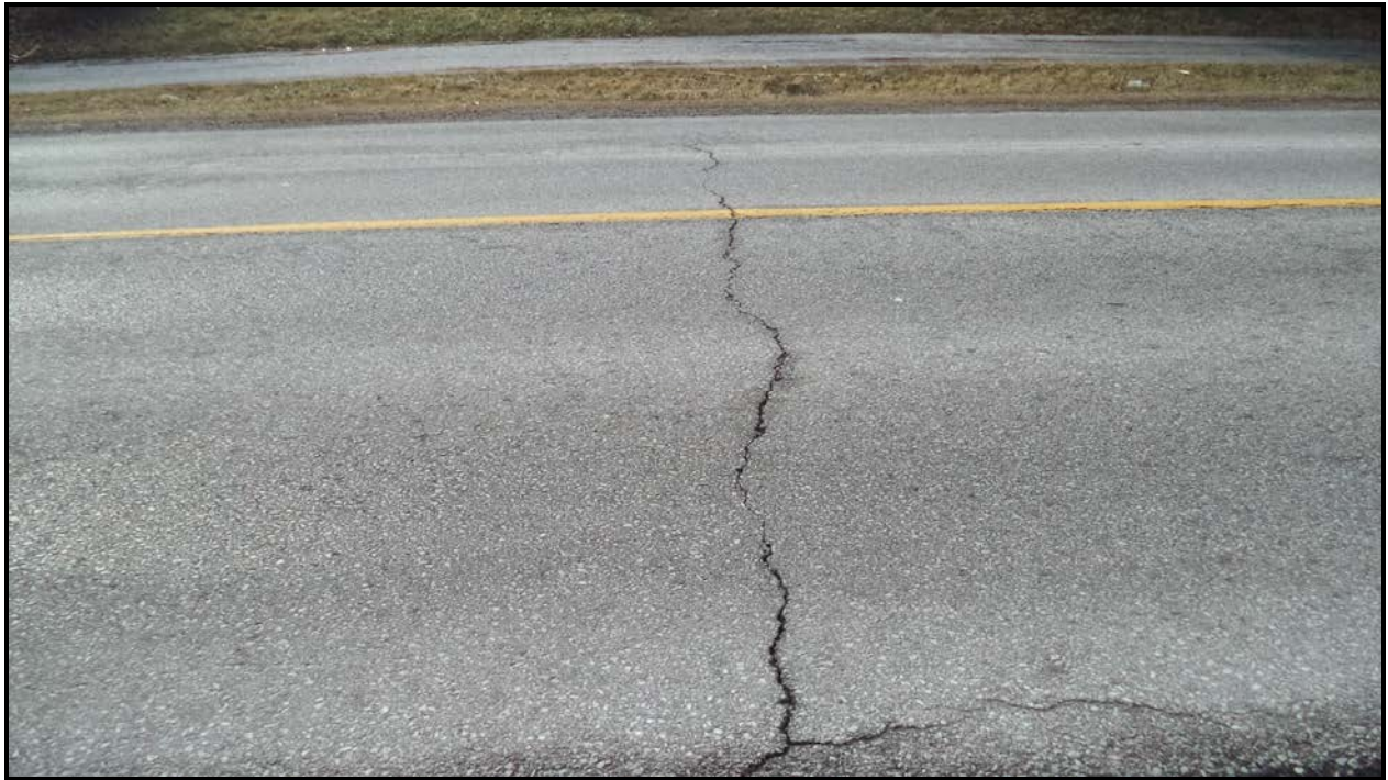
Photograph 7 – Wearing Surface at East Approach
