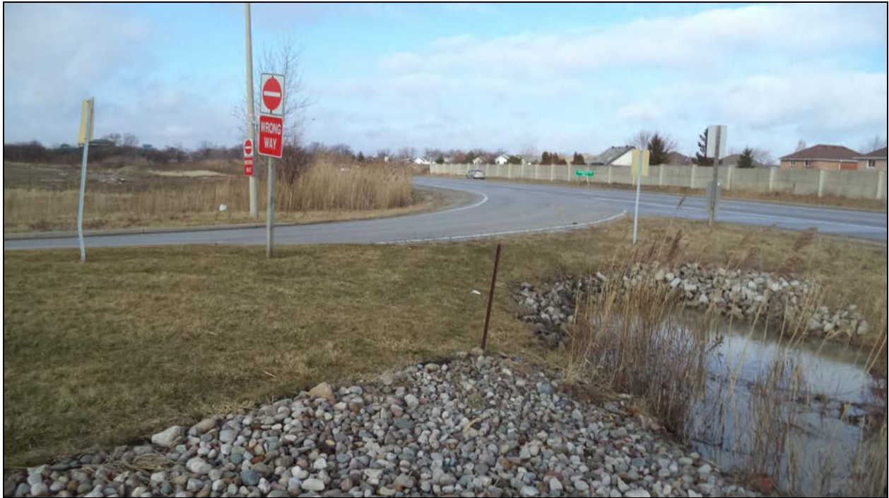
Photograph 1 – Road over Culvert (Looking West)
