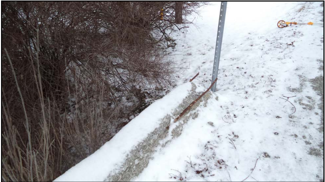
Photograph 7 – Eastern Wingwalls - North
