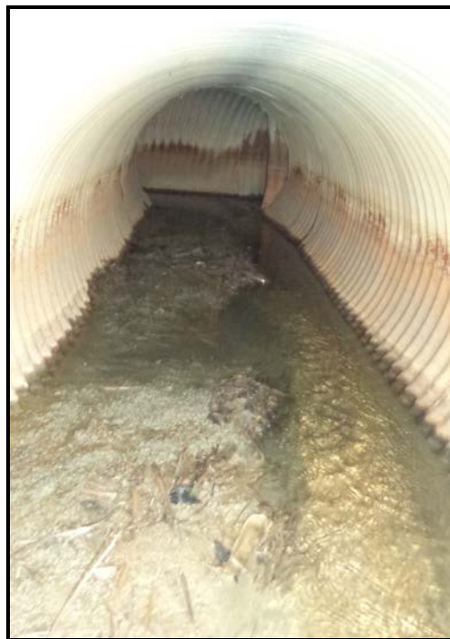
Photograph 2 – Culvert Barrel Intersection with Culvert No. 68 (Looking East)
