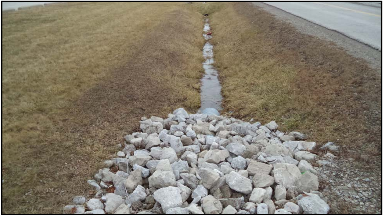
Photograph 7 – Water Stream (Tecumseh Rd East, North Side - Looking East)
