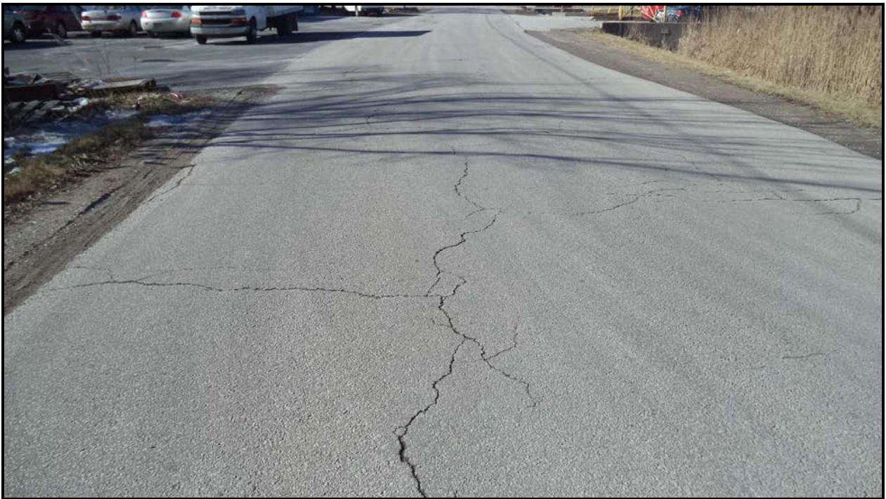
Photograph 6 – Wearing Surface over Culvert (Looking East)
