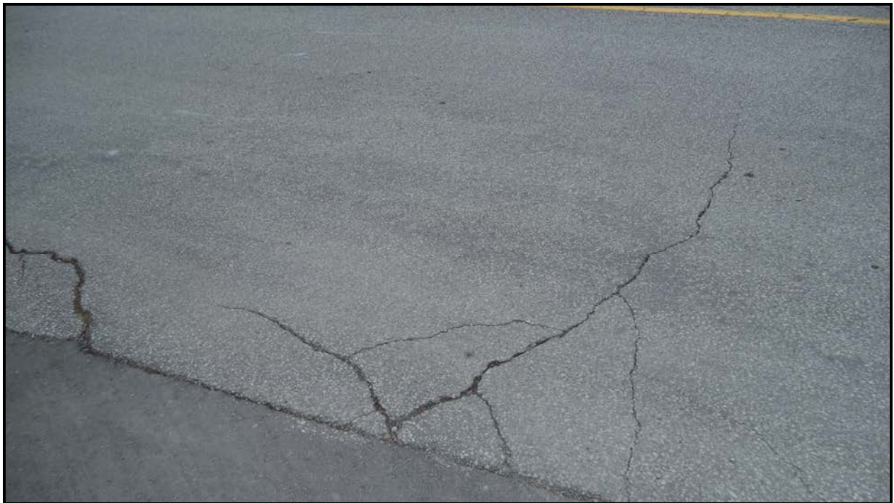
Photograph 6 – Wearing Surface over Culvert (Looking West)
