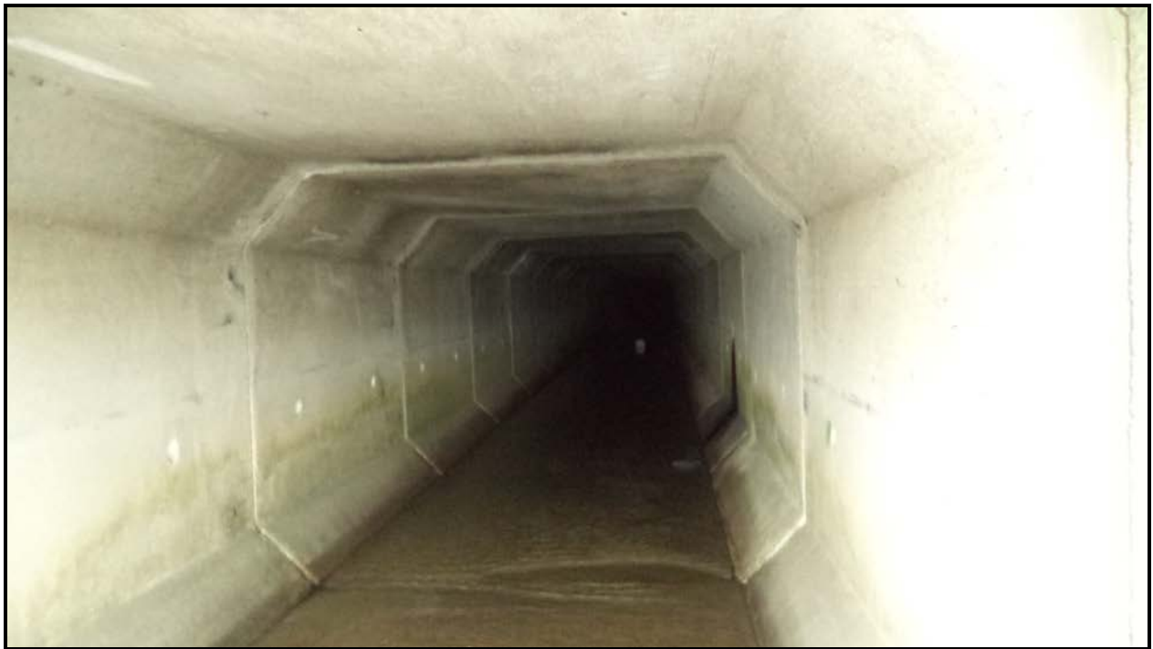
Photograph 2 – Culvert inside Box
