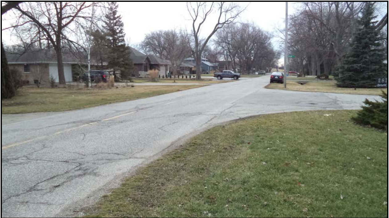
Photograph 1 – Road over Culvert (Looking South)
