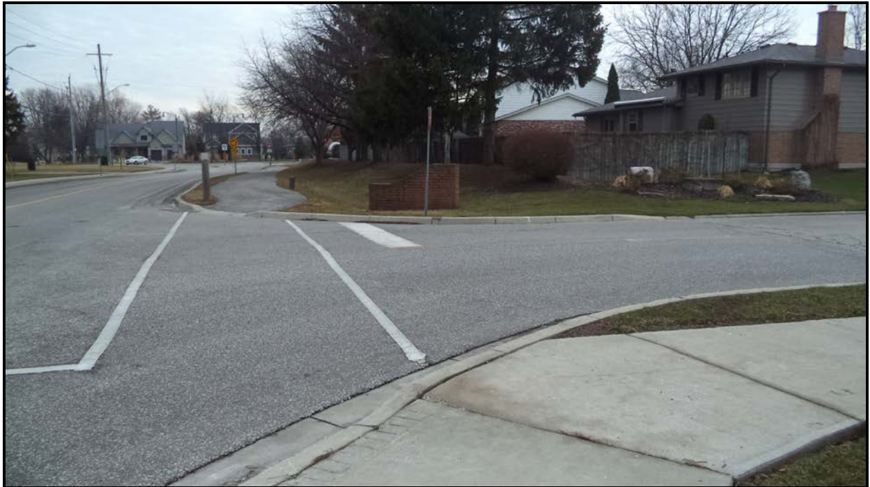
Photograph 7 – Wearing Surface over Culvert (Looking East)
