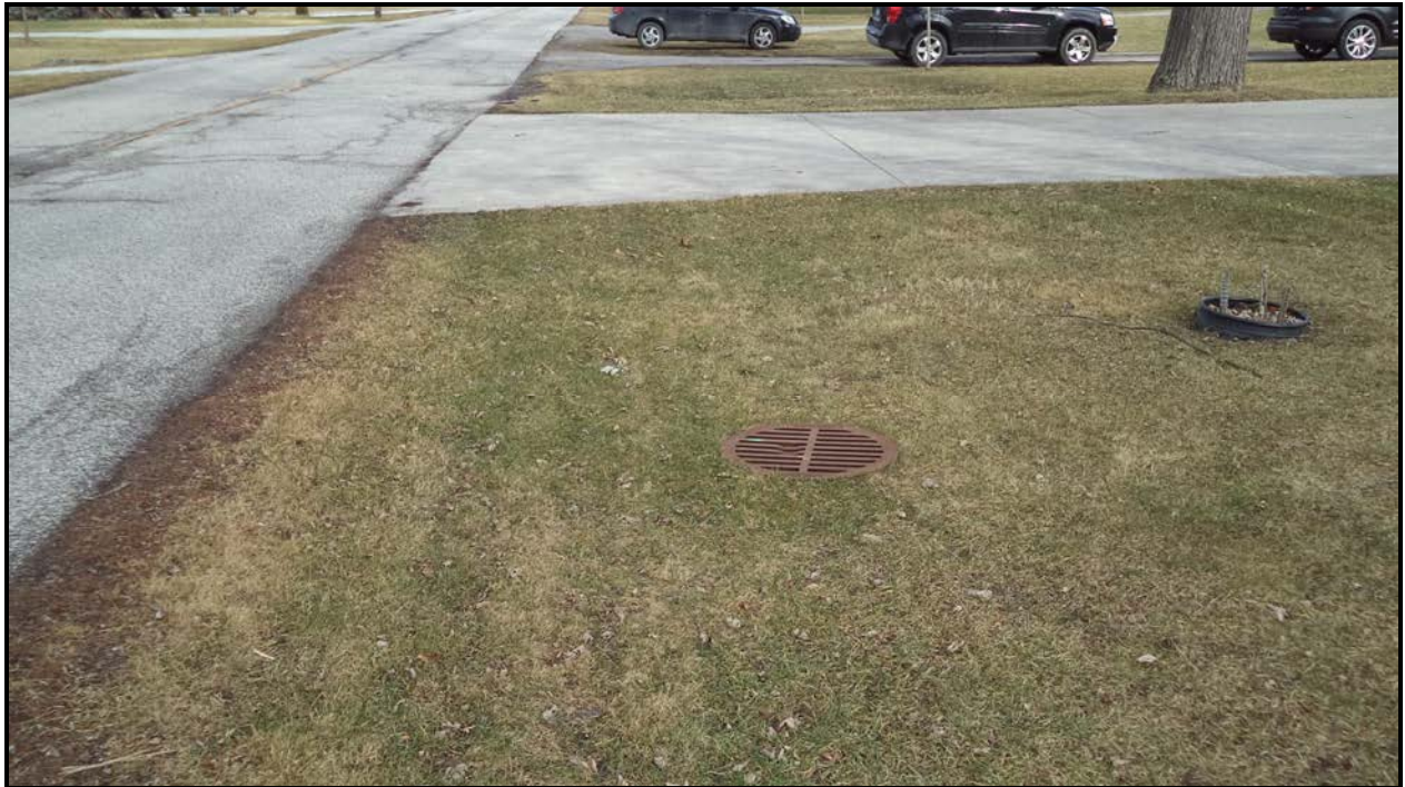
Photograph 3 – North Inlet Manhole
