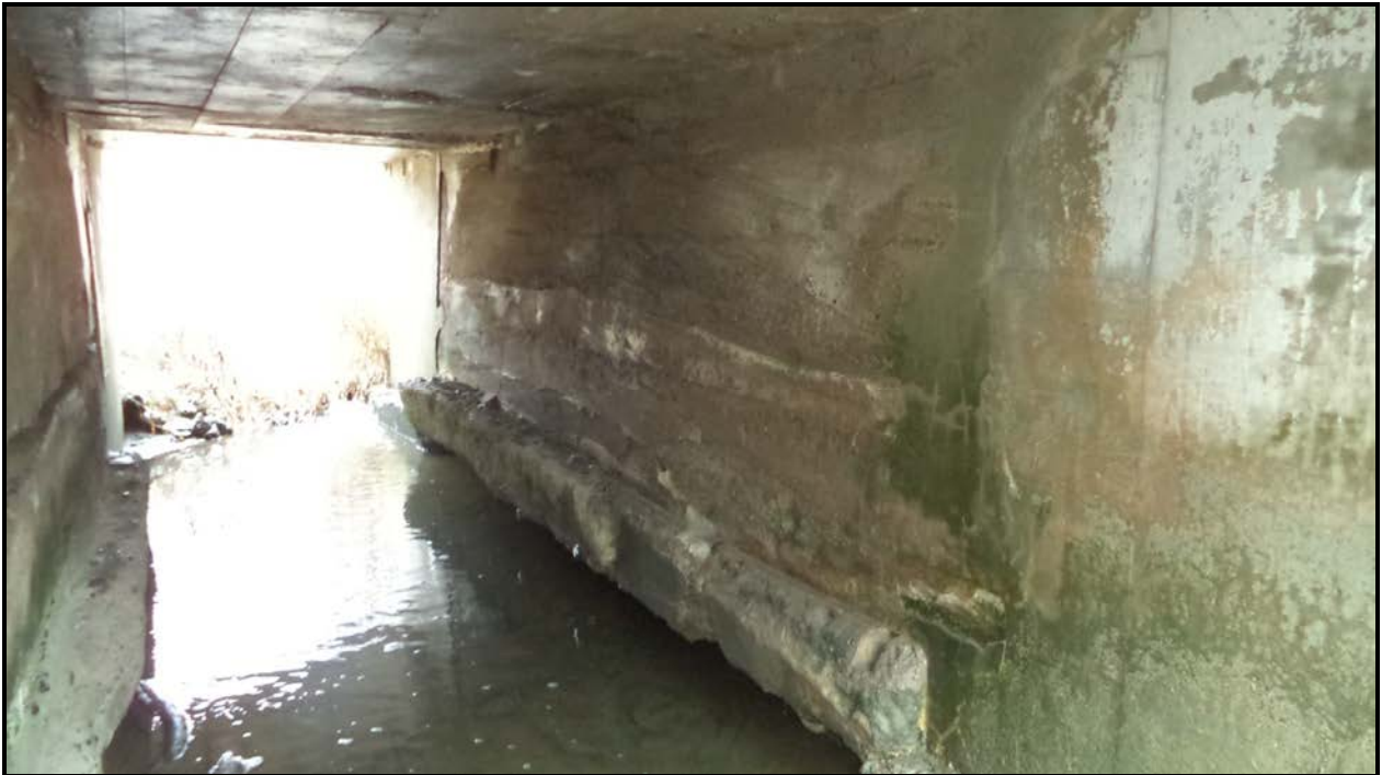
Photograph 3 – Culvert Barrel (Looking East)
