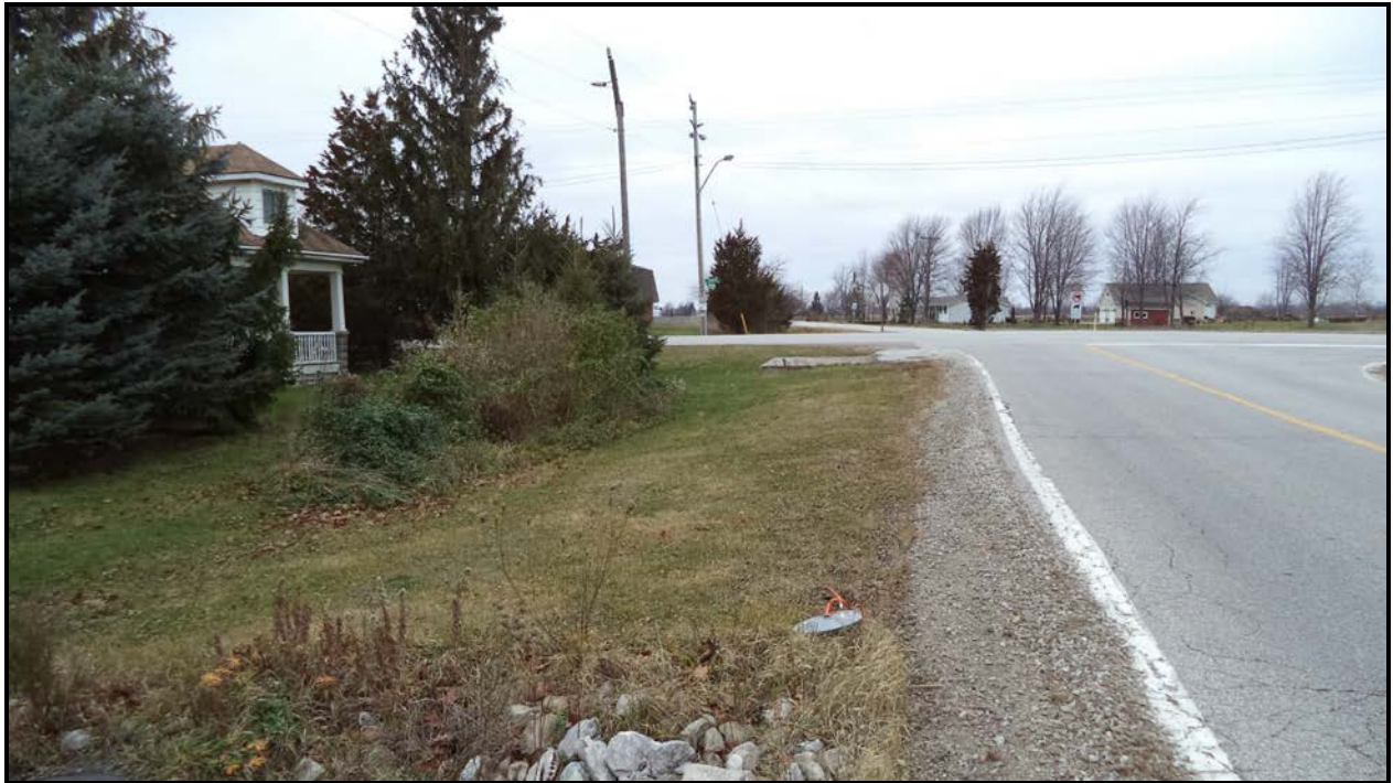
Photograph 1 – Road over Culvert (Looking West)
