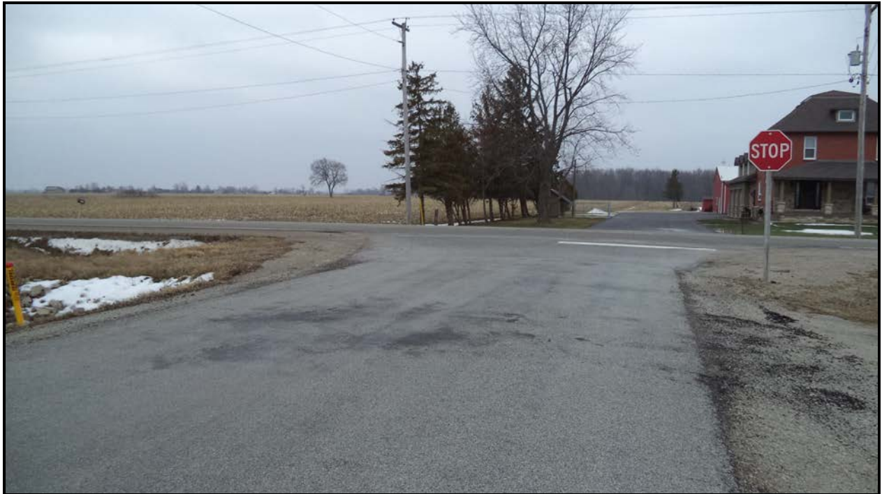
Photograph 1 – Road over Culvert (Looking South)
