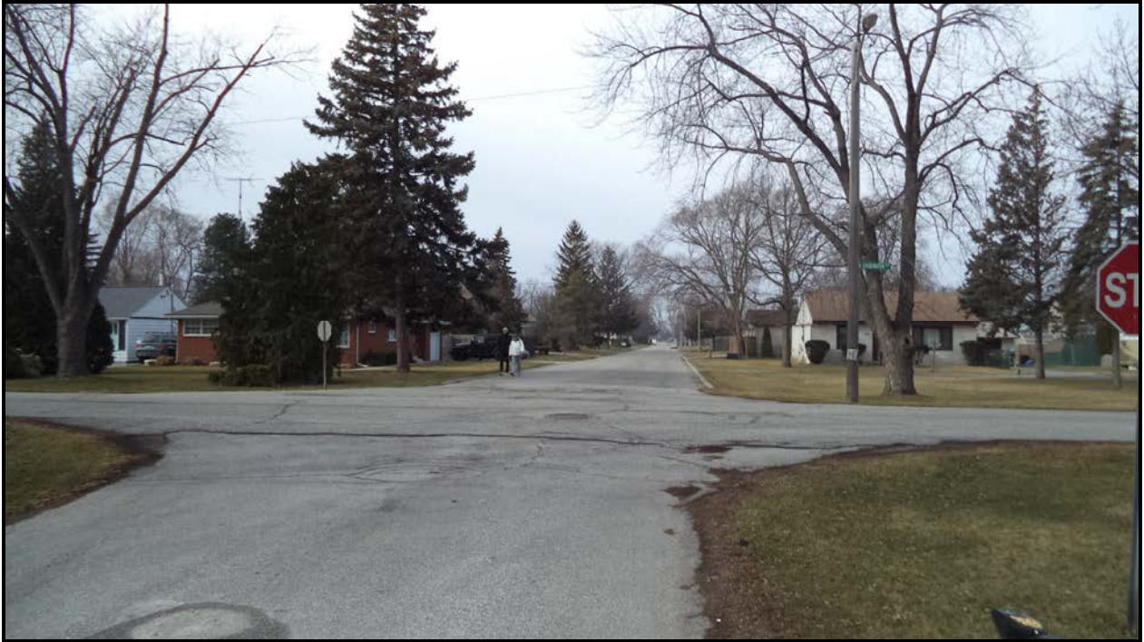
Photograph 1 – Road over Culvert (Looking West)
