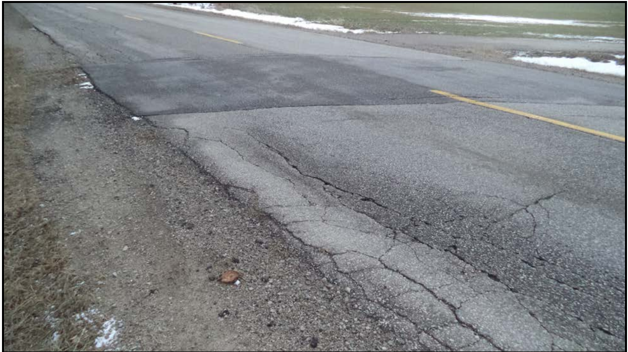
Photograph 5 – Wearing Surface over Culvert (Looking East)
