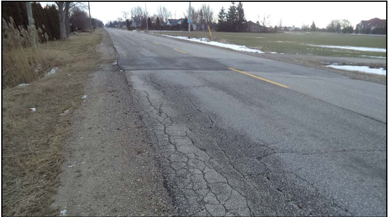
Photograph 1 – Road over Culvert (Looking South)
