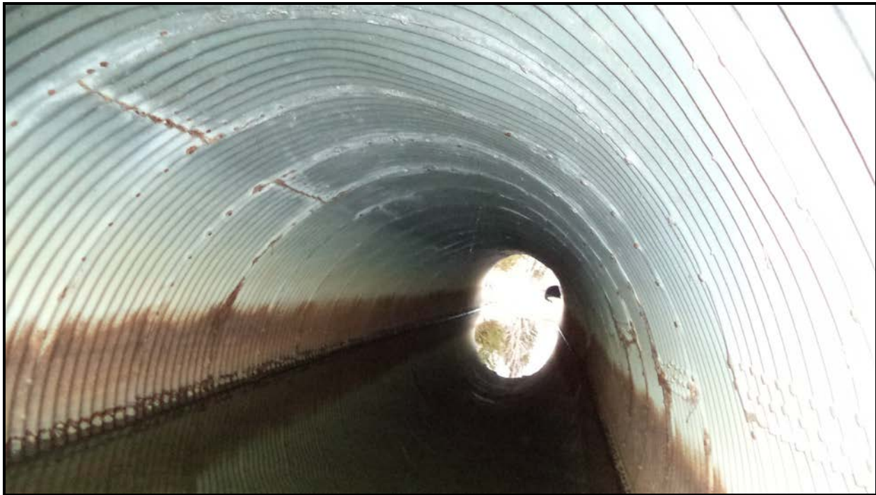
Photograph 2 – Culvert Barrel (Looking West)
