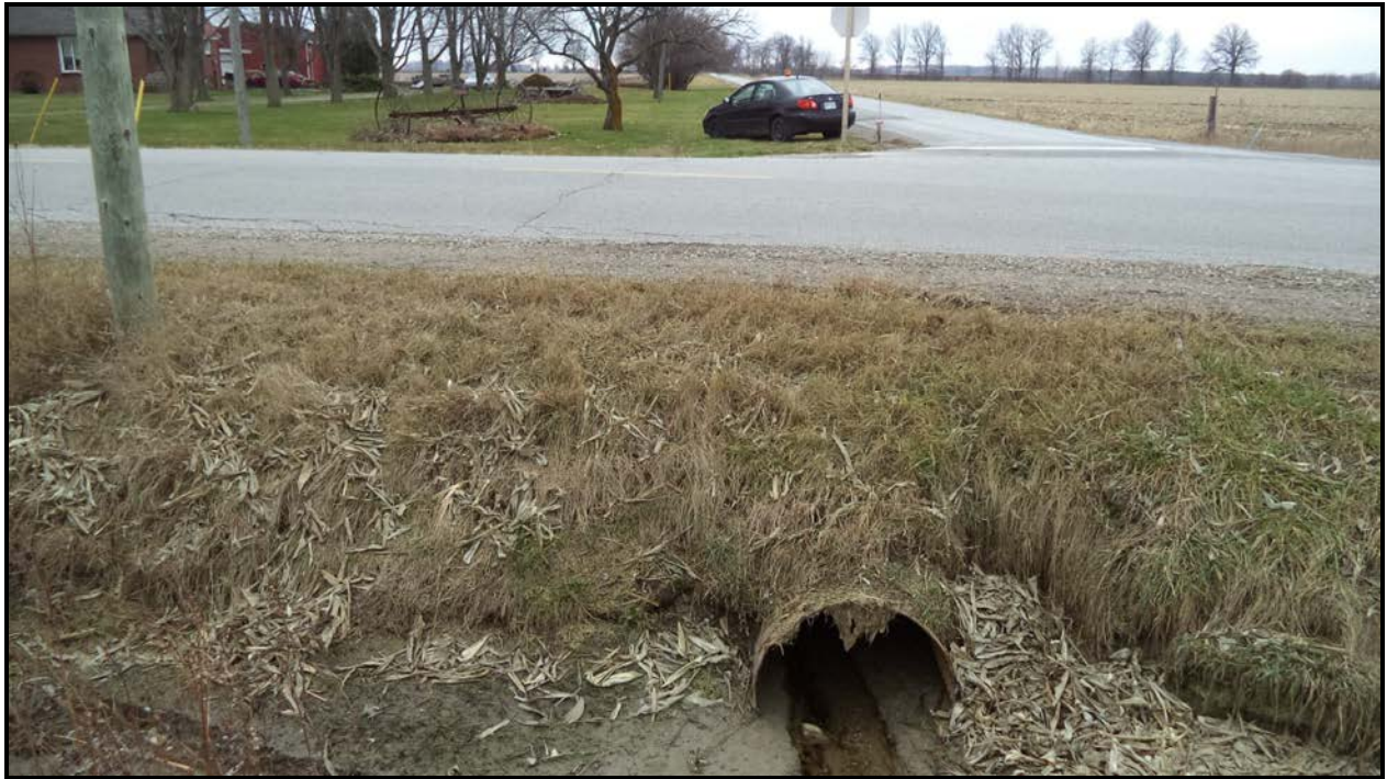
Photograph 5 – Wearing Surface over Culvert (Looking West)
