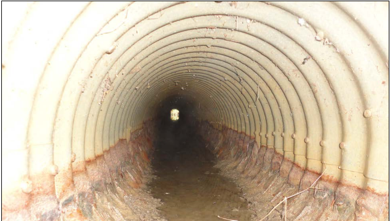
Photograph 3 – Culvert Barrel (Looking West)
