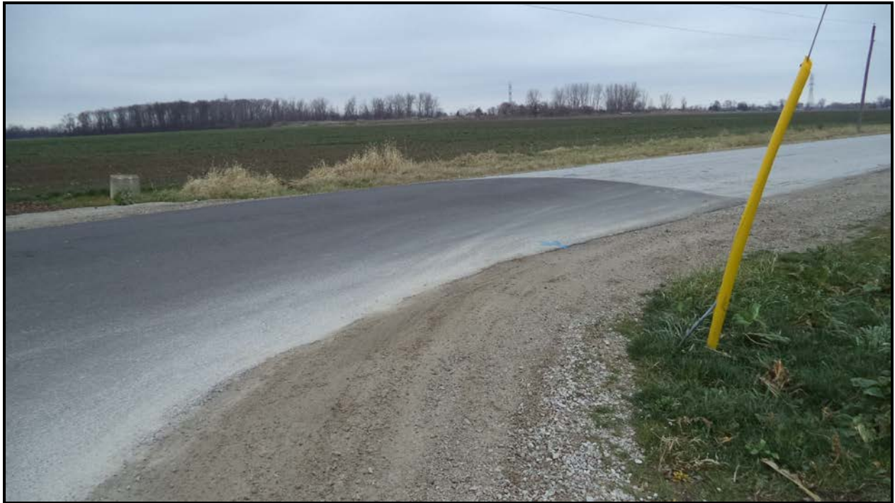
Photograph 5 – Wearing Surface at North Approach
