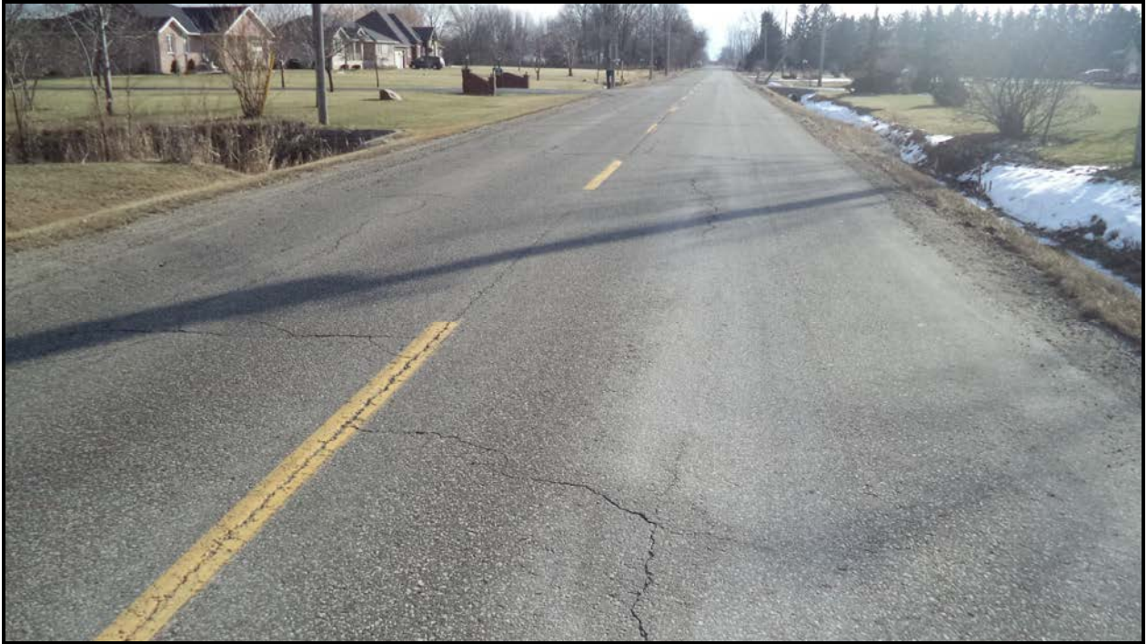
Photograph 1 – Road over Culvert (Looking South)
