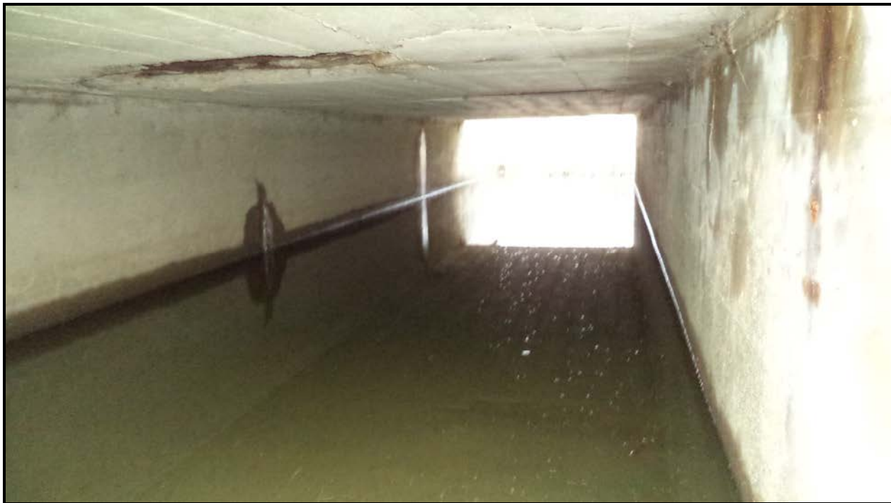
Photograph 2 – Culvert Soffit (Looking South)
