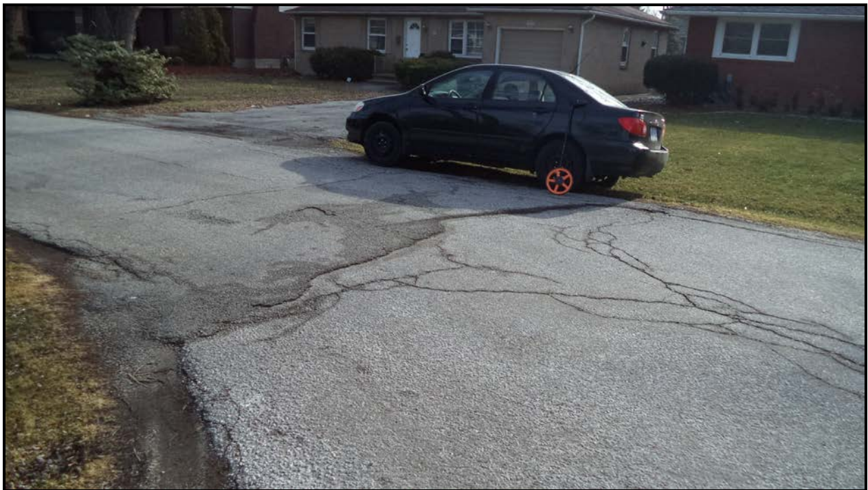
Photograph 6 – Wearing Surface at East approach
