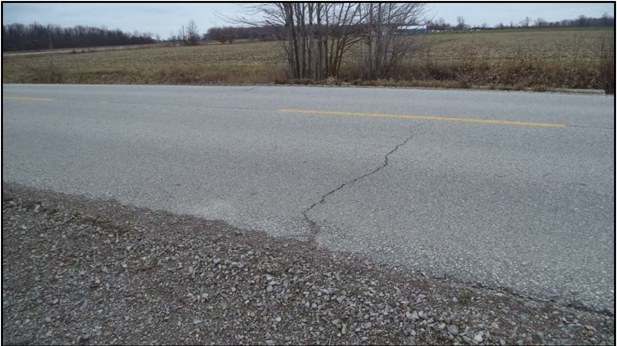
Photograph 5 – Wearing Surface over Culvert (Looking South)
