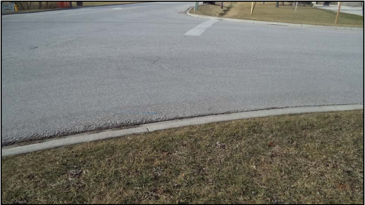
Photograph 5 – Wearing Surface over Culvert (Looking West)
