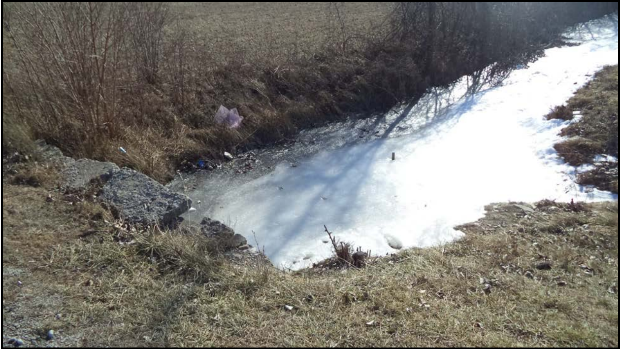
Photograph 7 – Water Stream (Moynahan Street East Side - Looking East)
