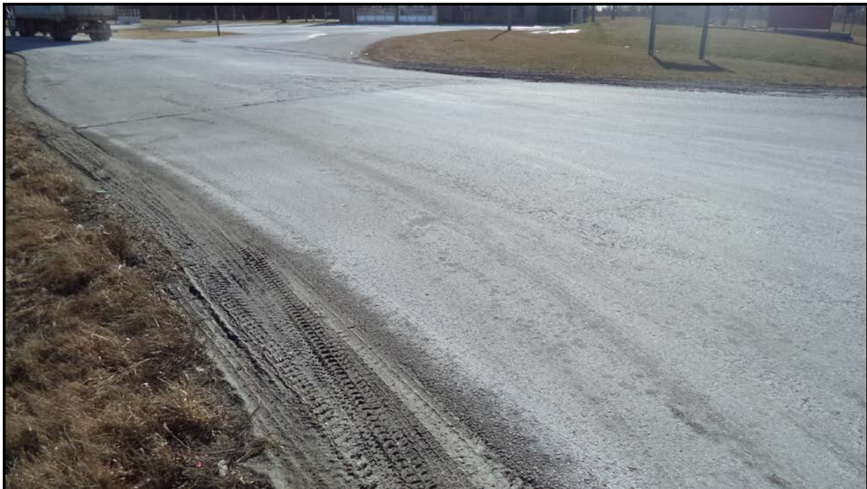
Photograph 2 – Wearing Surface at East Approach
