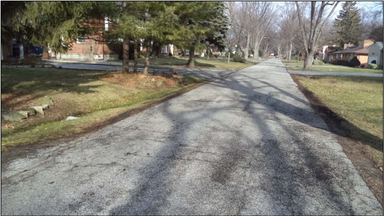
Photograph 1 – Road over Culvert (Looking North)
