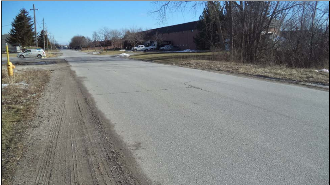
Photograph 1 – Road over Culvert (Looking North)
