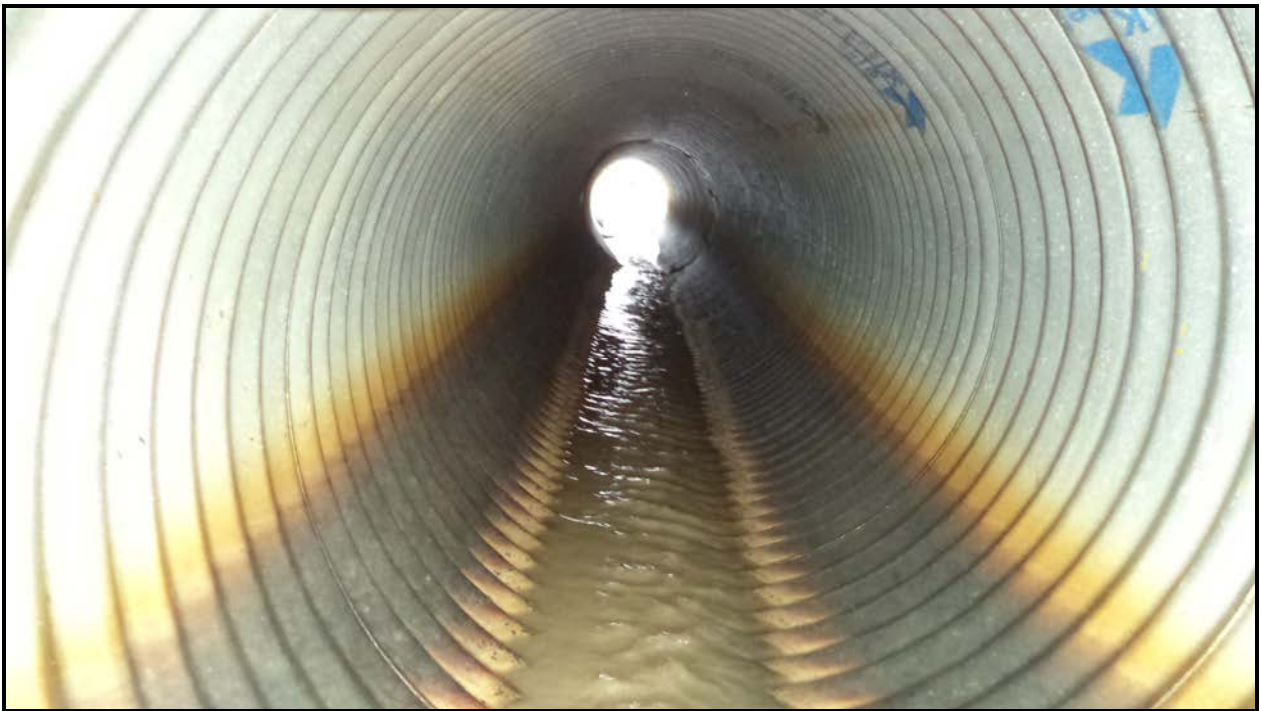
Photograph 2 – Culvert Barrel (Looking West)
