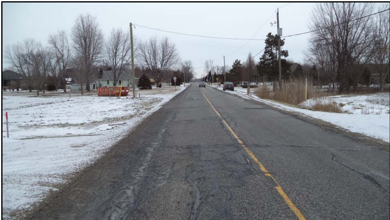
Photograph 2 – Road over Culvert (Looking North)
