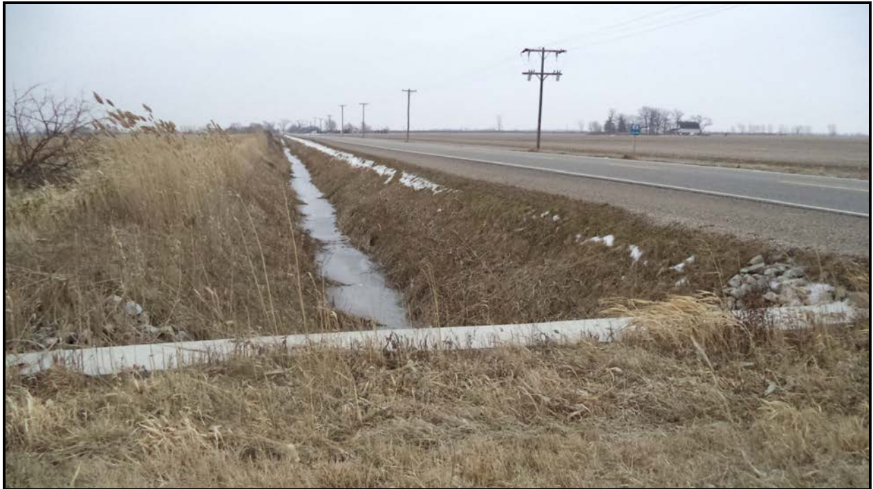
Photograph 7 – Water Stream (Malden Road West Side – Looking East)
