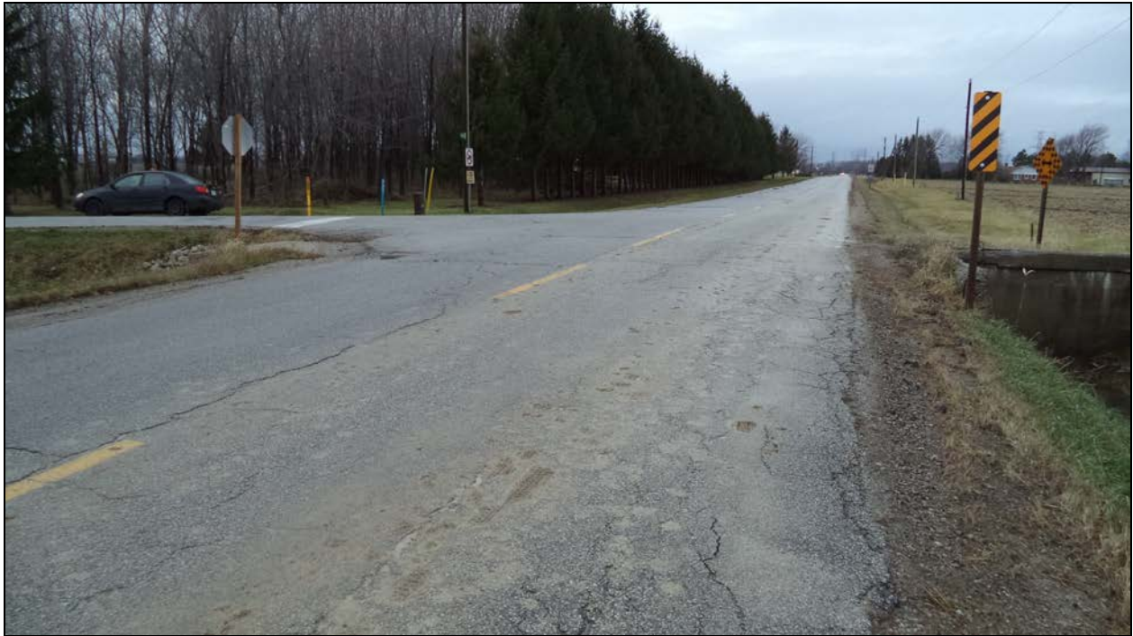
Photograph 1 – Road over Culvert (Looking West)
