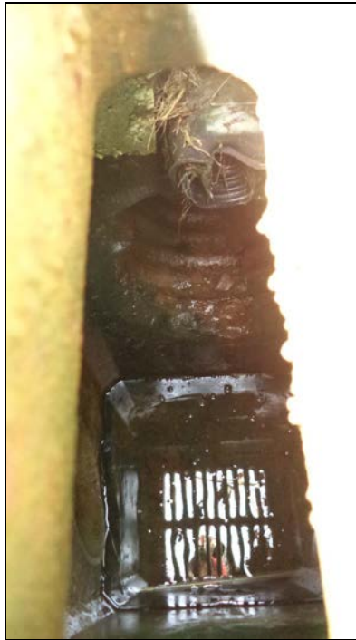
Photograph 5 – South Inlet Manhole
