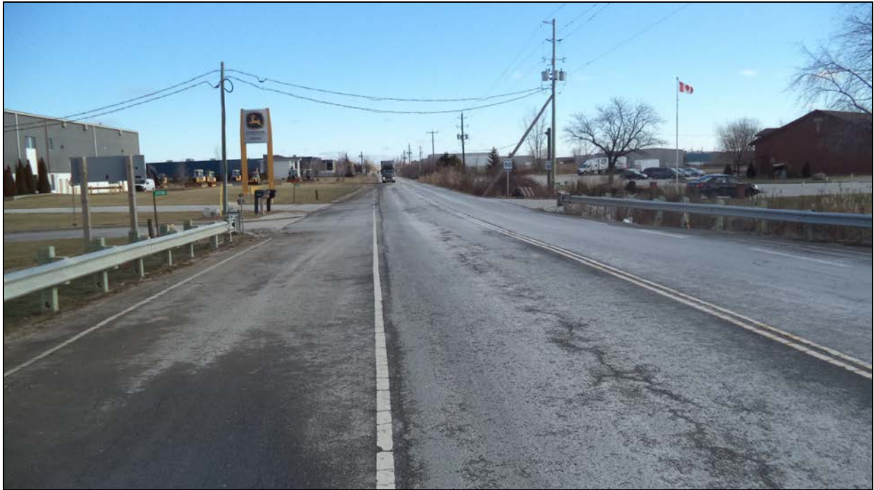
Photograph 1 – Road over Culvert (Looking North)
