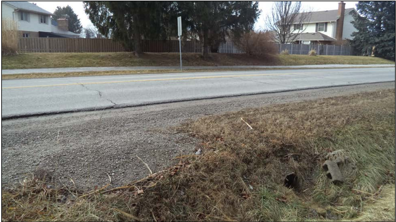
Photograph 1 – Road over Culvert (Looking South)
