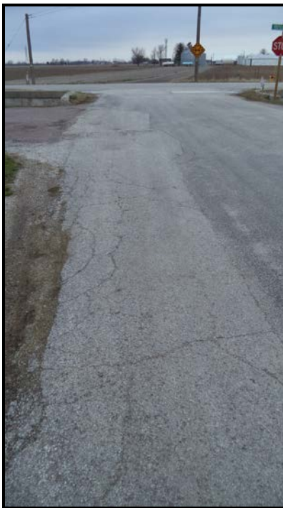
Photograph 10 – Wearing Surface at South Approach (Looking North)
