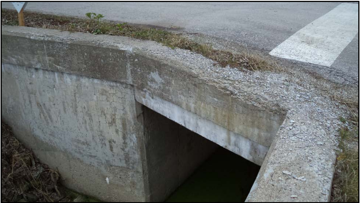
Photograph 6 – Headwall (East Elevation)
