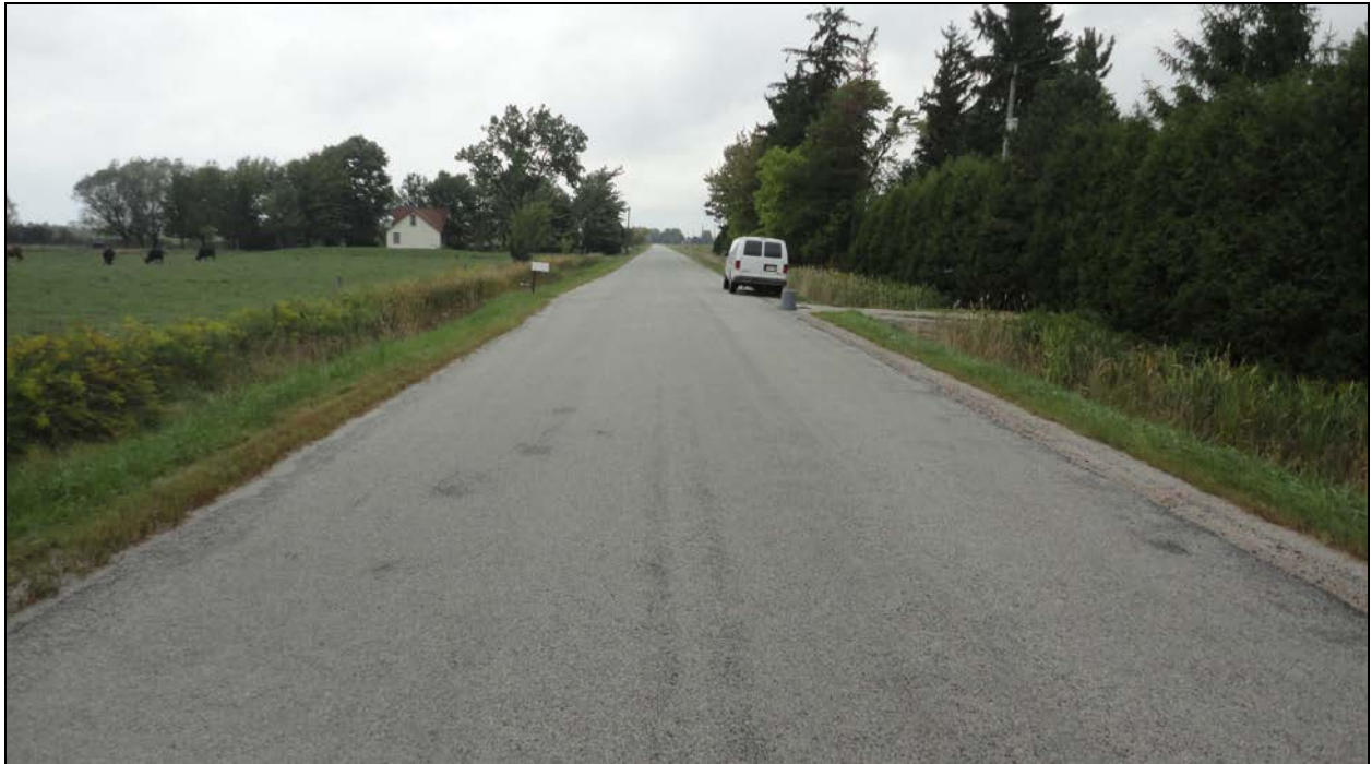
Photograph 1 – Wearing Surface over Culvert (Looking North)
