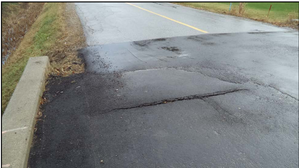
Photograph 8 – Wearing Surface at East Approach
