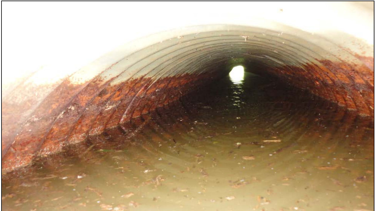
Photograph 5 – Culvert Barrel (Looking East)
