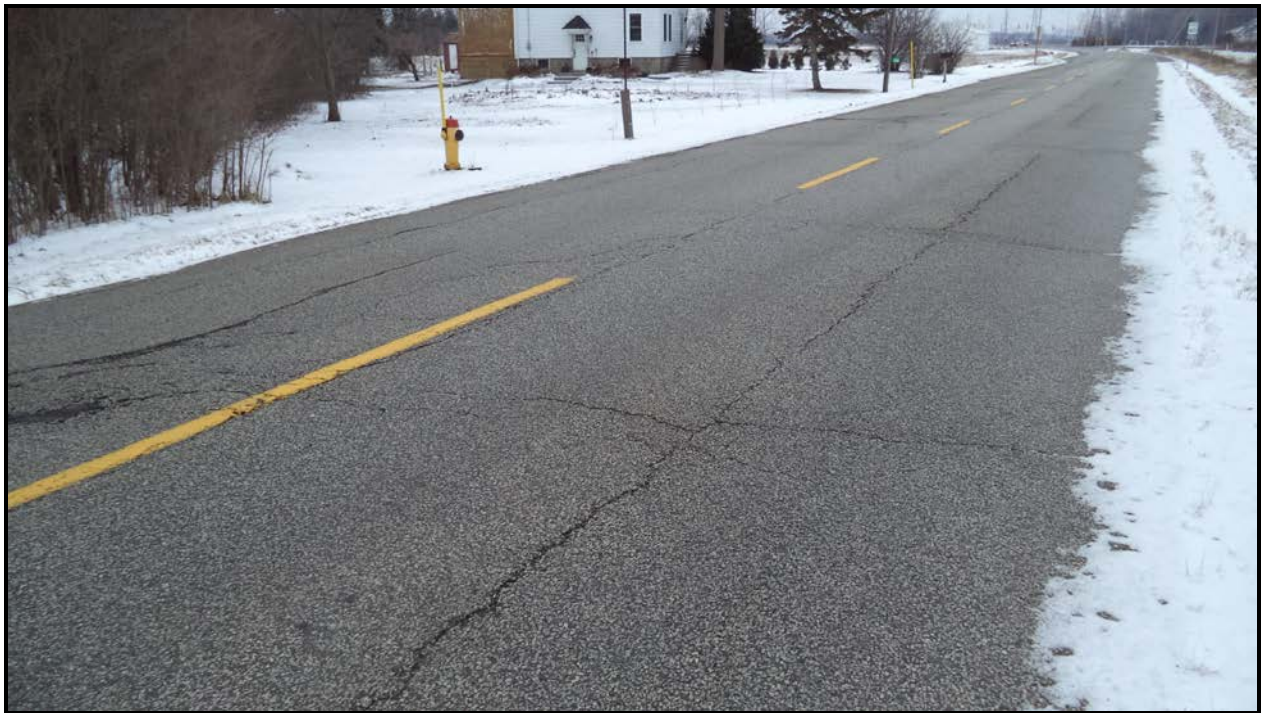
Photograph 8 – Wearing Surface at West Approach (Looking West)
