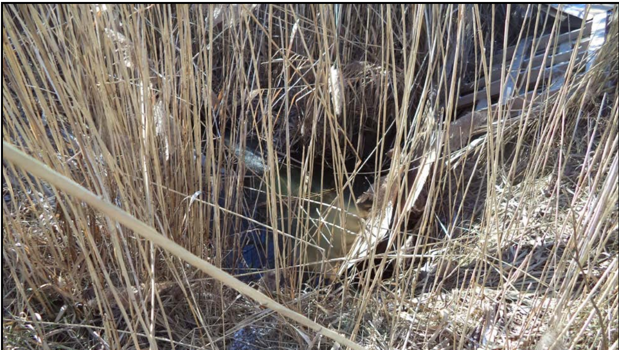
Photograph 2 – Culvert Inlet at South Elevation
