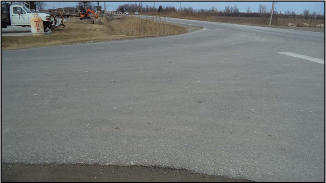
Photograph 7 – Wearing Surface over Culvert (Looking North)
