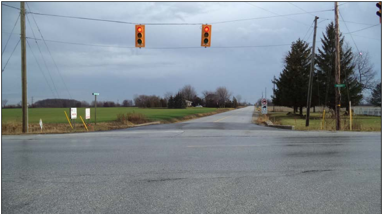
Photograph 1 – Road over Culvert (Looking East)
