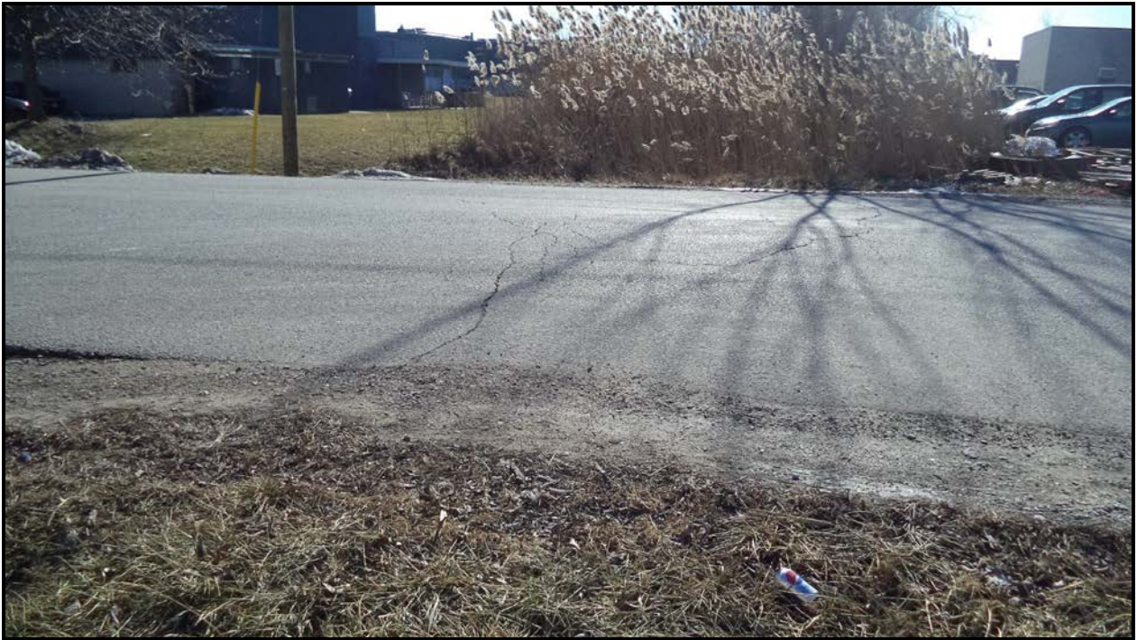
Photograph 5 – Wearing Surface over Culvert (Looking South)
