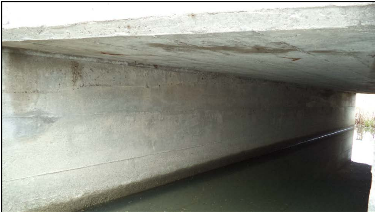
Photograph 2 – Wearing Surface over Culvert (Looking East)
