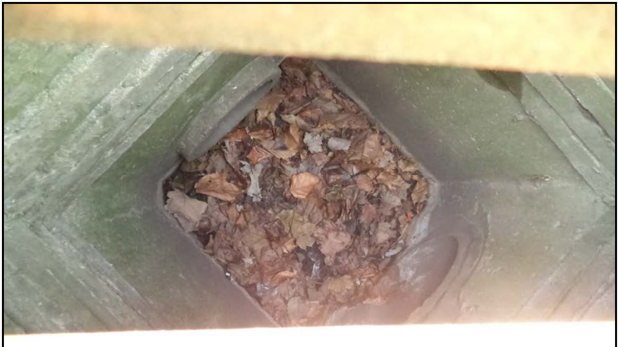
Photograph 4 – East Inlet Manhole
