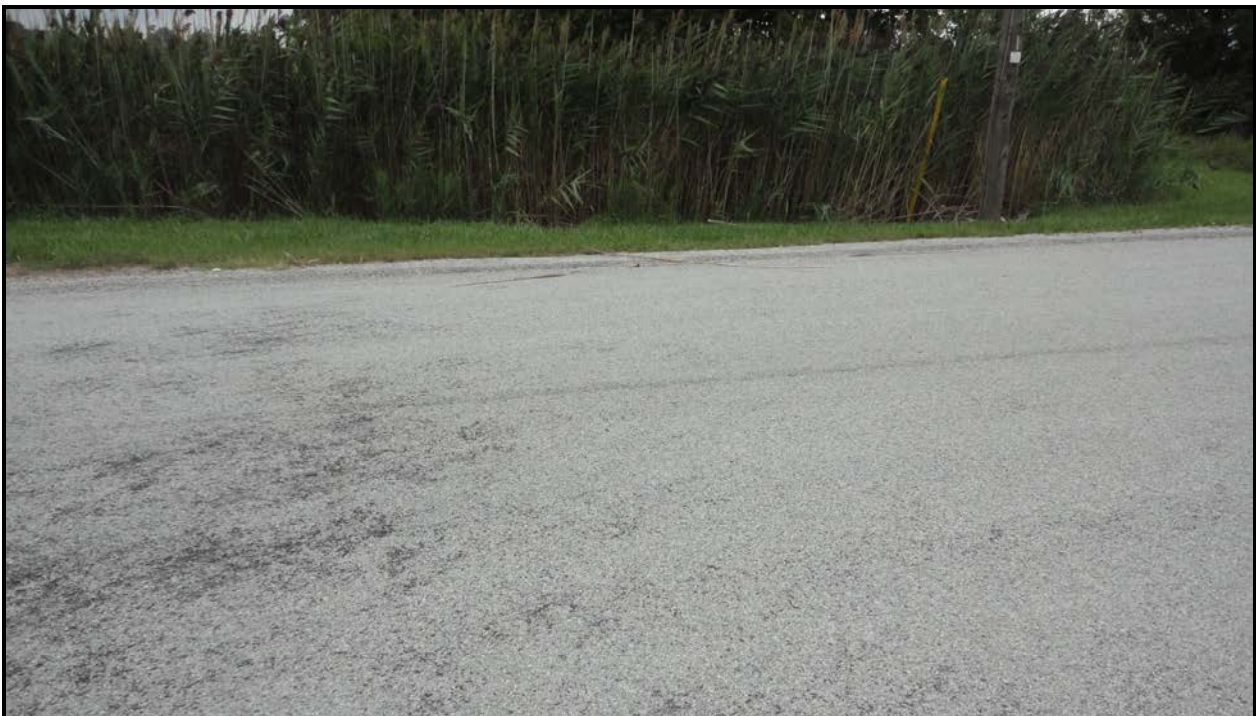
Photograph 2 – Wearing Surface over Culvert (Looking West)
