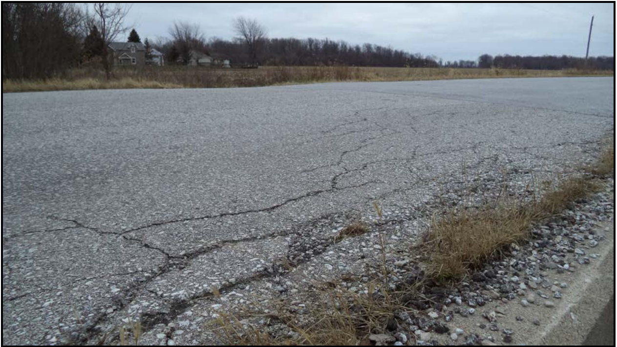
Photograph 5 – Wearing Surface over Culvert (Looking East)
