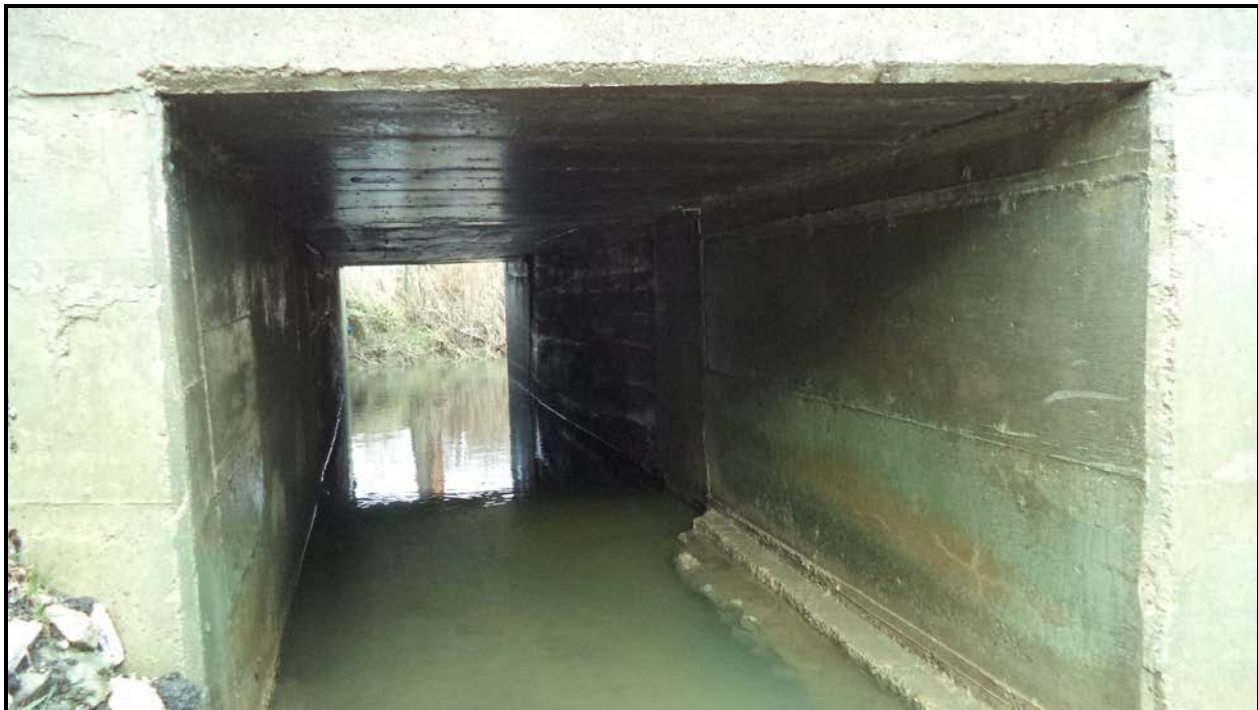
Photograph 2 – Culvert Barrel (Looking North)
