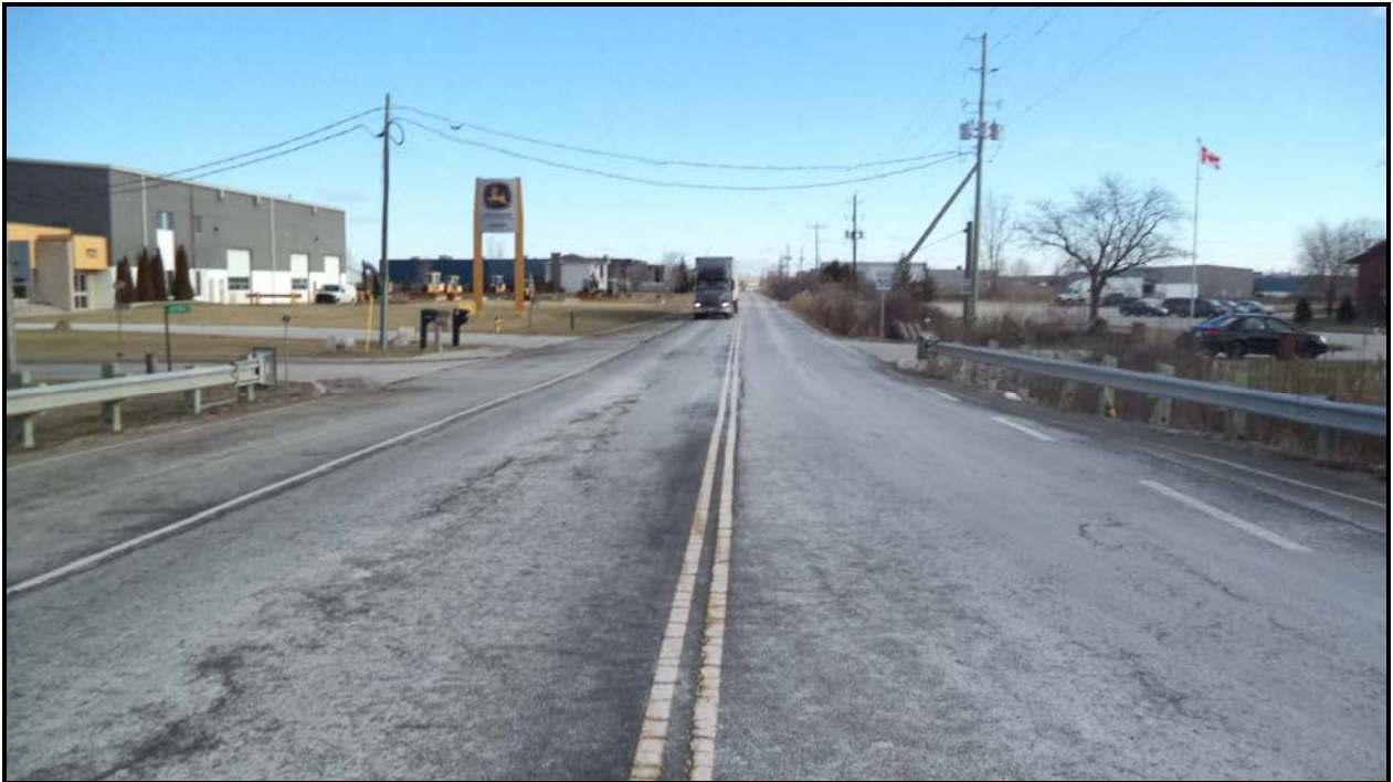
Photograph 5 – Wearing Surface over Culvert (Looking South)
