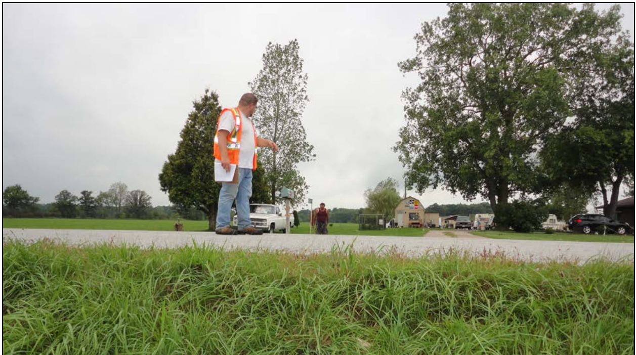
Photograph 4 – Road over Culvert (Looking West)
