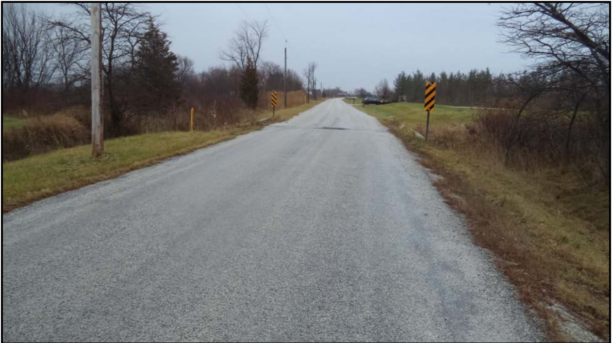
Photograph 1 – Road over Culvert (Looking South)
