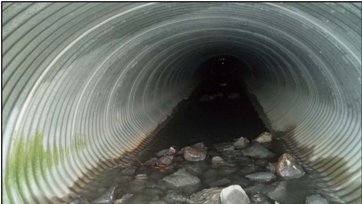
Photograph 2 – Culvert Barrel
