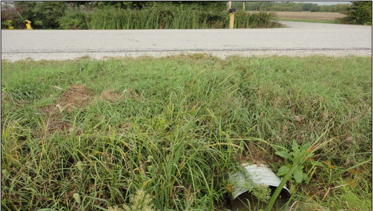
Photograph 7 – Road over Culvert & East Inlet (Looking South)
