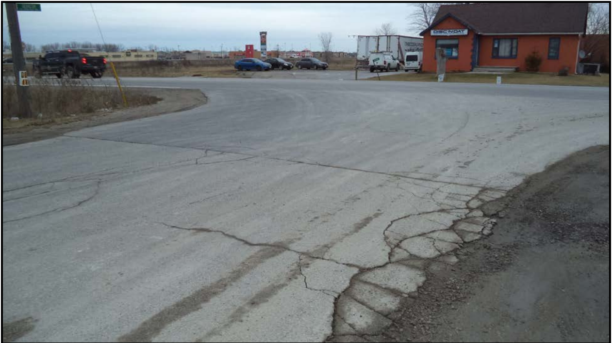
Photograph 1 – Road over Culvert (Looking East)
