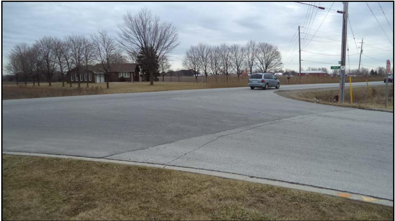
Photograph 1 – Road over Culvert (Looking South)
