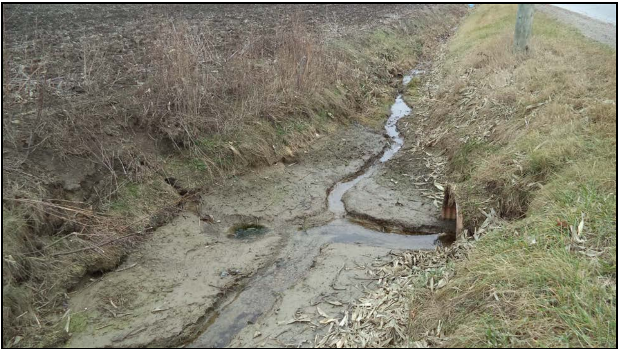
Photograph 4 – North Elevation (Looking East)
