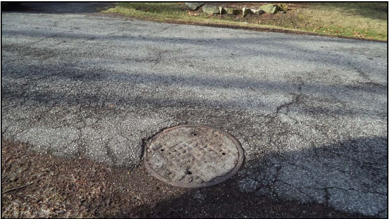
Photograph 4 – Wearing Surface over Culvert (Looking West)
