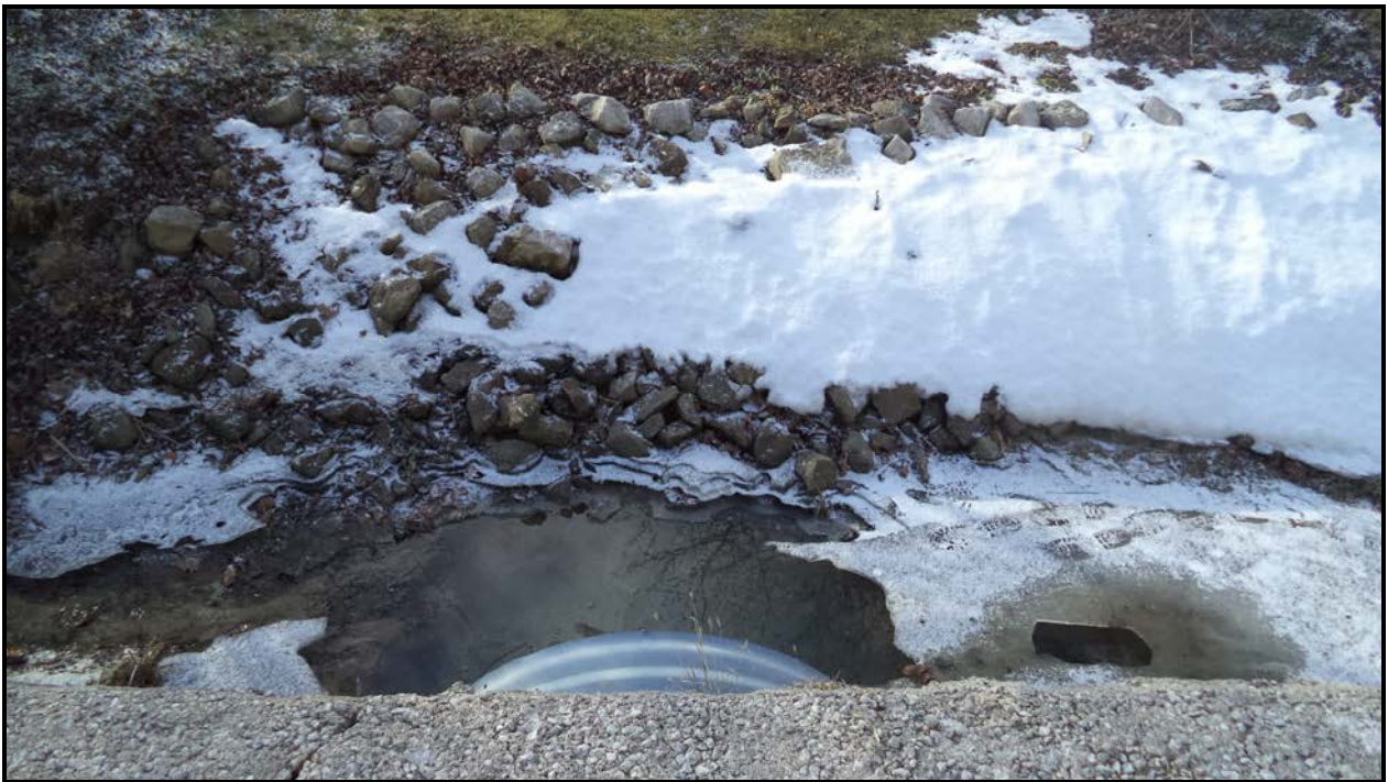
Photograph 8 – Water Stream (North Talbot Road South Side - Looking South)
