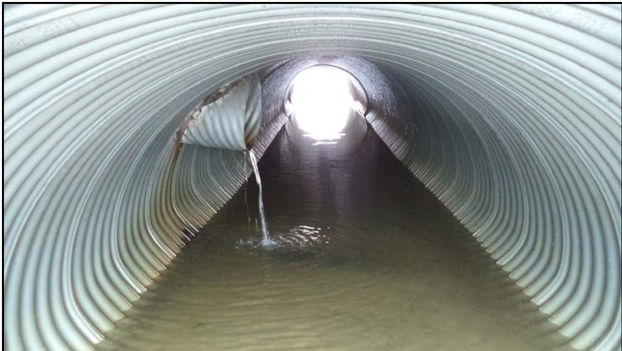
Photograph 2 – Culvert Barrel (Looking East)
