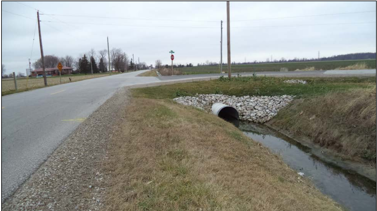
Photograph 1 – Road over Culvert (Looking West)
