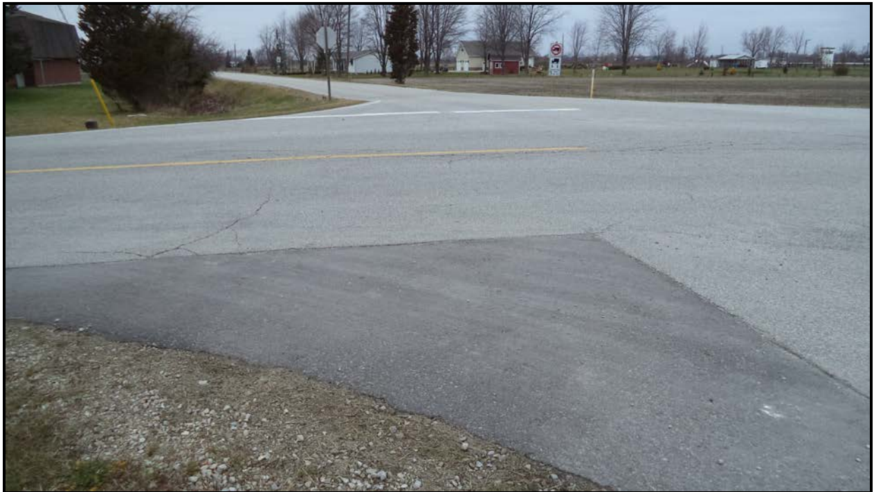
Photograph 2 – Road over Culvert (Looking West)
