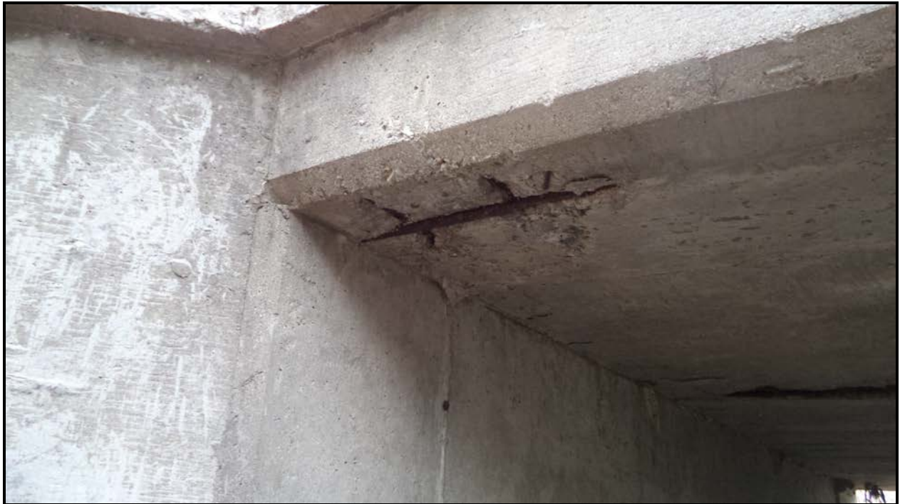
Photograph 3 – Culvert Barrel - Soffit
