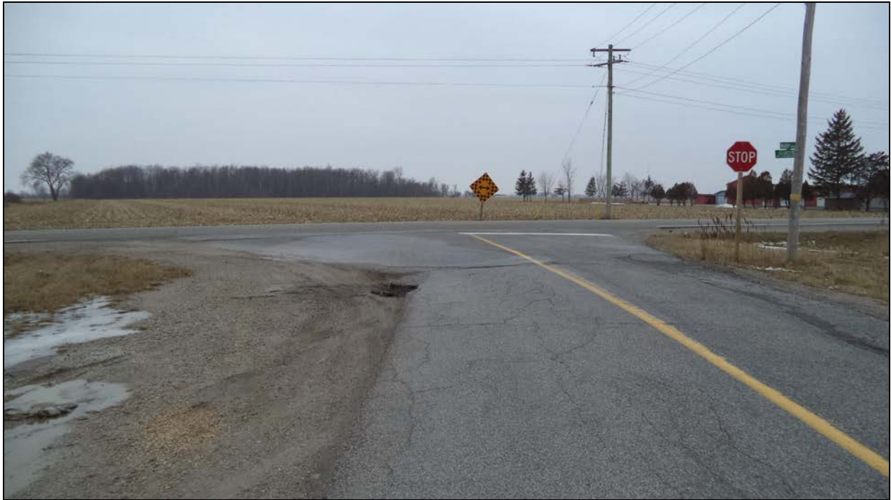
Photograph 1 – Road over Culvert (Looking South)
