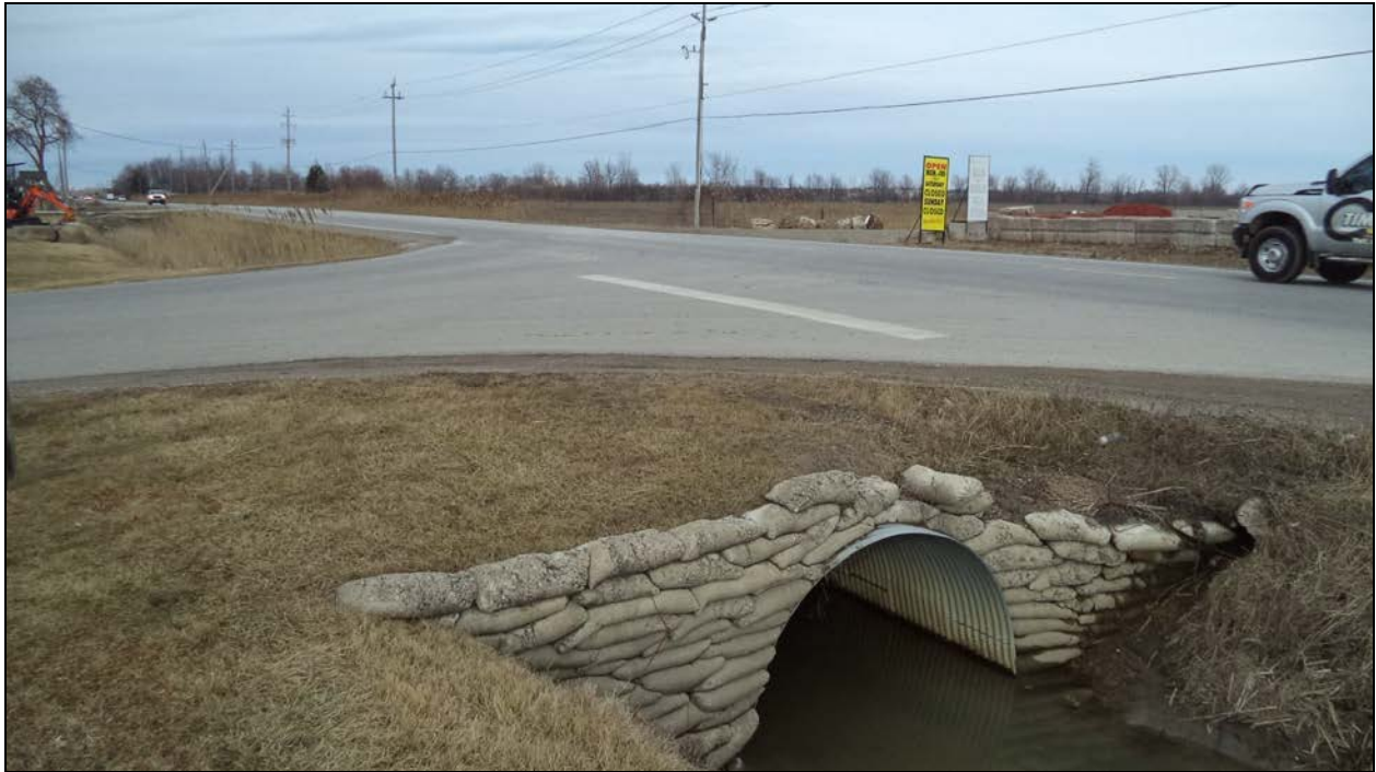
Photograph 1 – Road over Culvert (Looking North)
