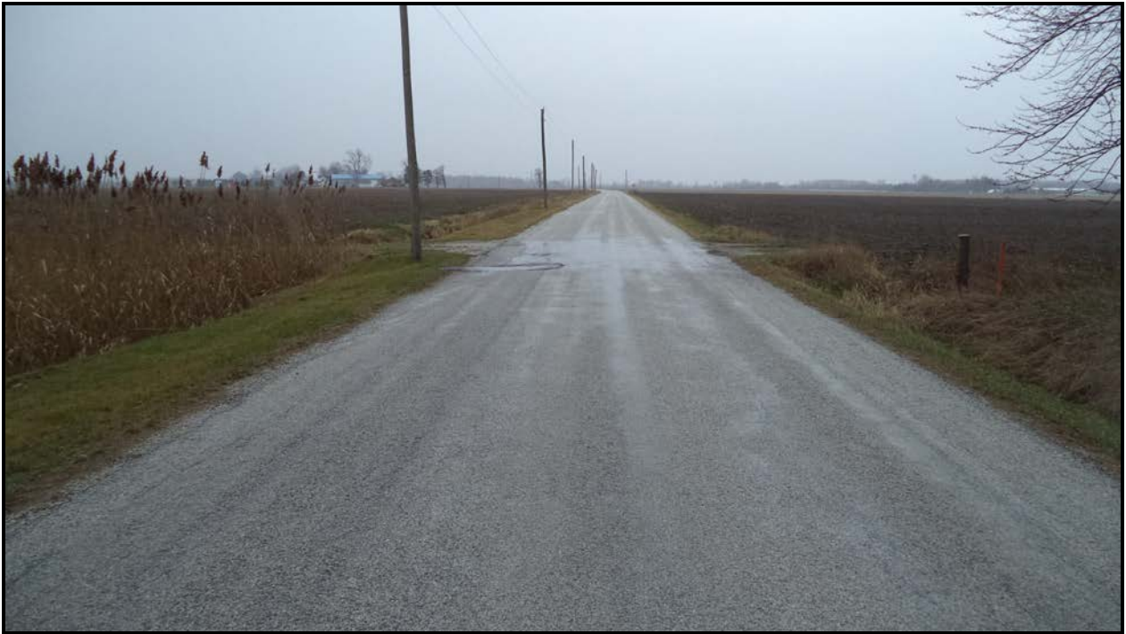
Photograph 1 – Road over Culvert (Looking South)
