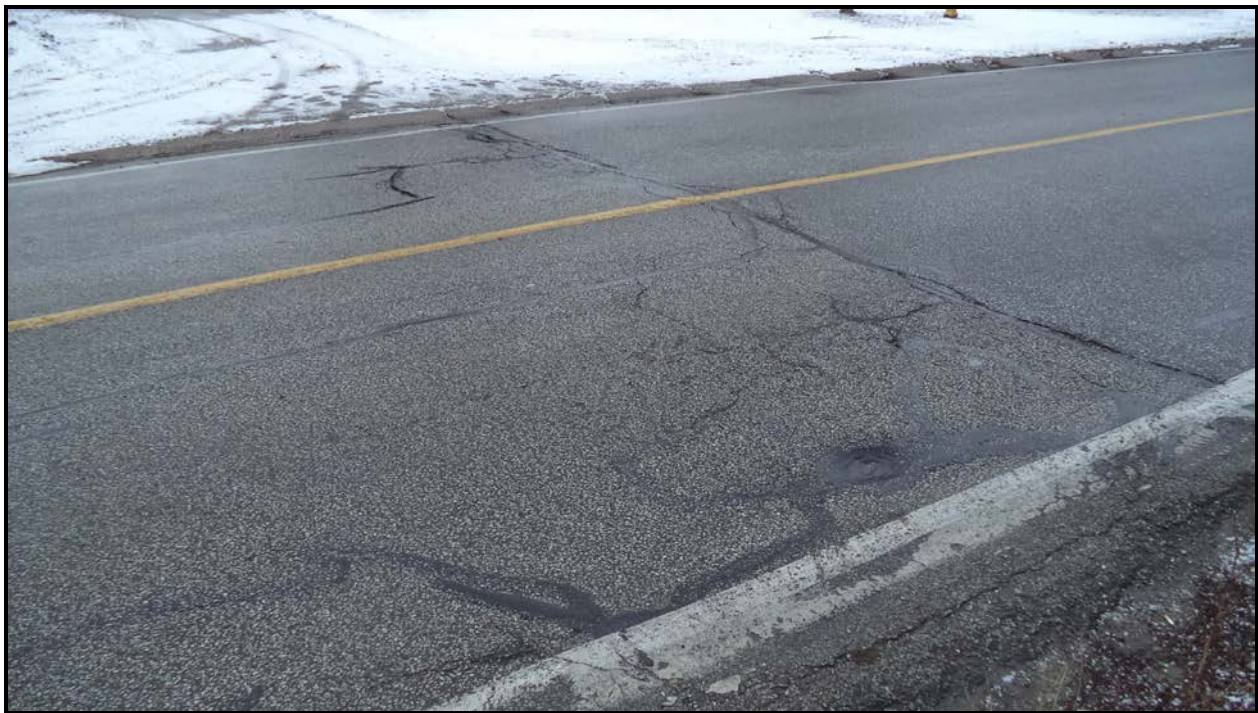
Photograph 4 – Wearing Surface over Culvert (Looking South)
