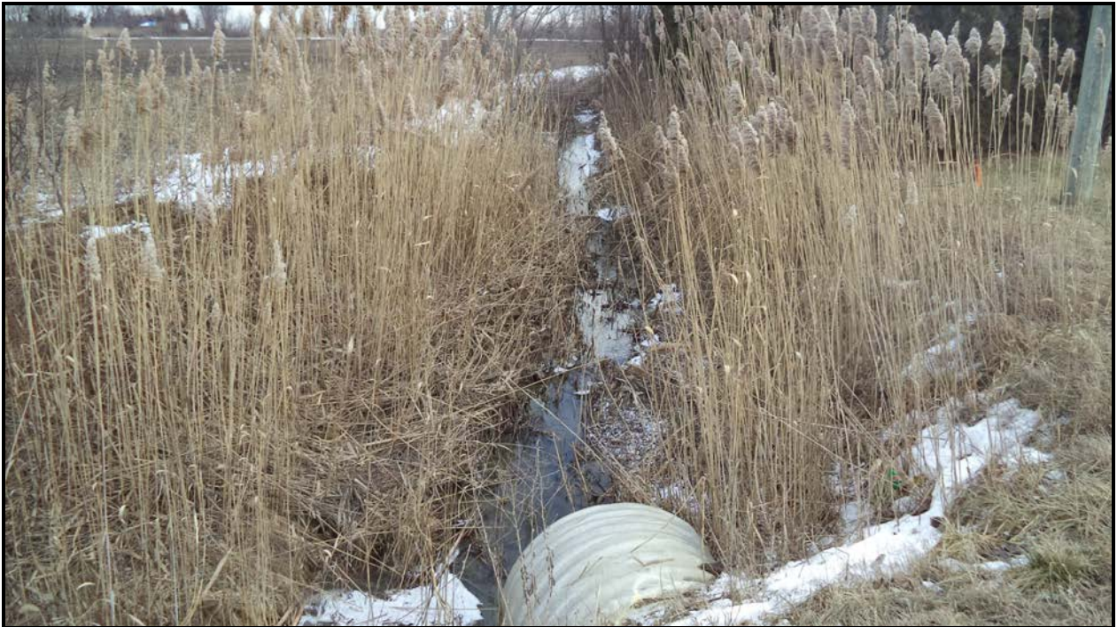
Photograph 7 – Water Stream (North Talbot Road North Side - Looking North)
