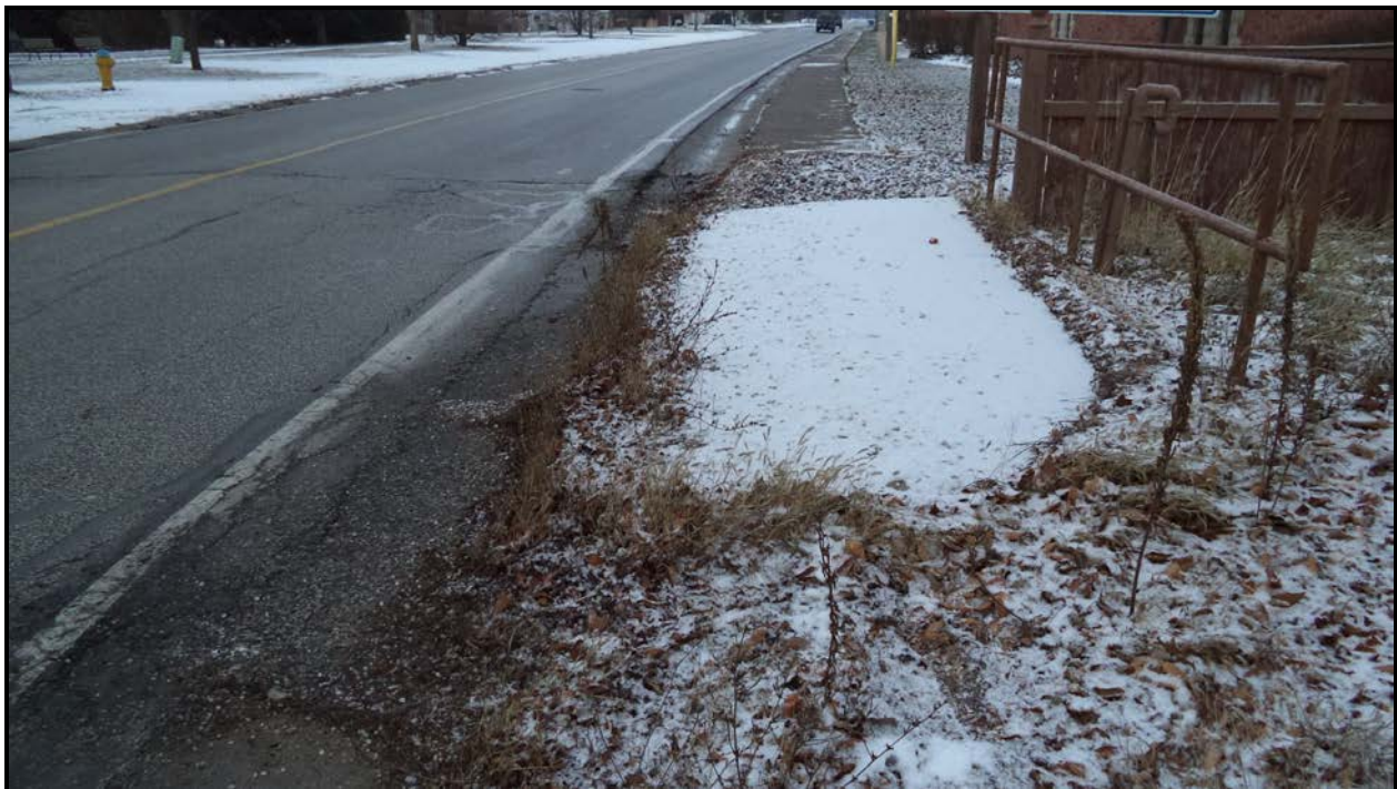
Photograph 2 – Sidewalk and Handrail over North Outlet (Looking West)
