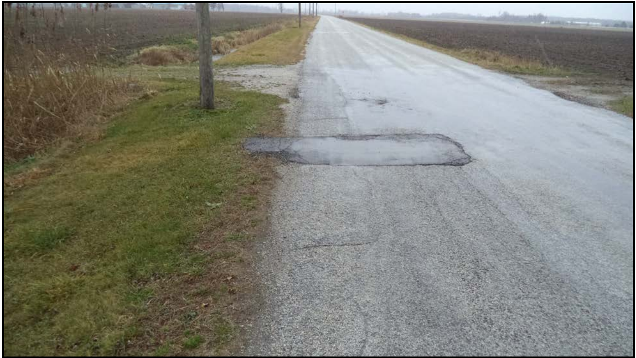
Photograph 7 – Wearing Surface over Culvert (Looking South)
