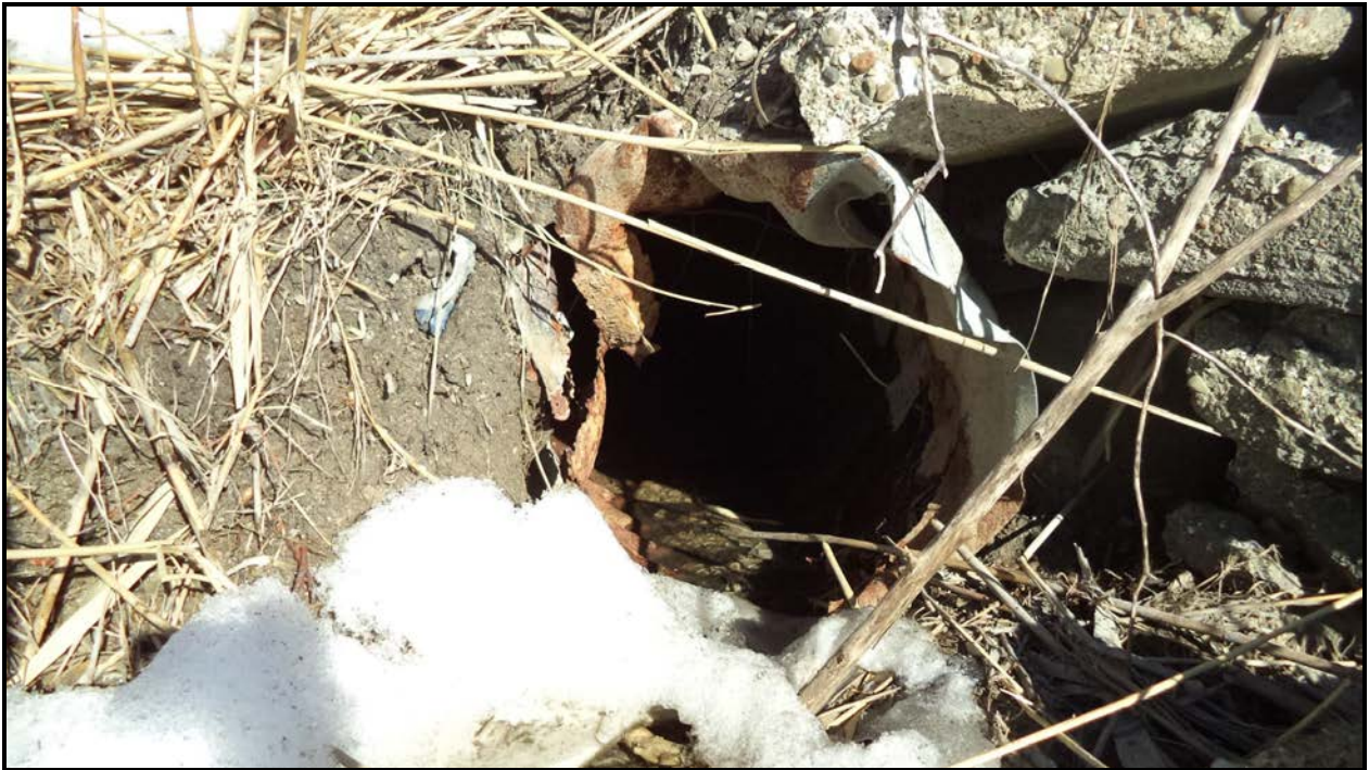
Photograph 4 – Culvert Inlet at South Elevation
