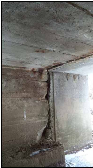
Photograph 4 – Culvert Barrel (At joint between Old/New Structure)
