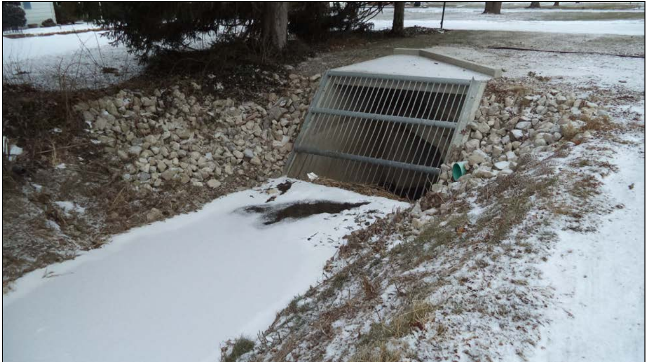
Photograph 1 – Western Culvert Inlet (Looking North)
