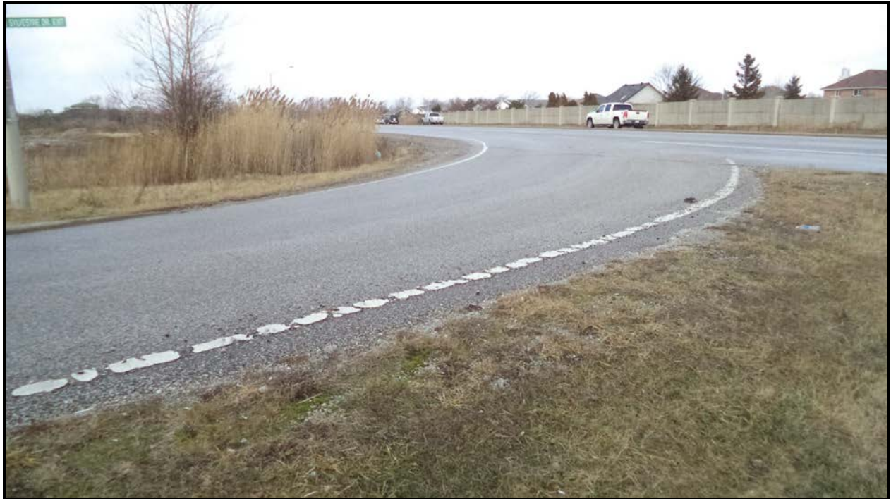
Photograph 5 – Wearing Surface over Culvert (Looking West)
