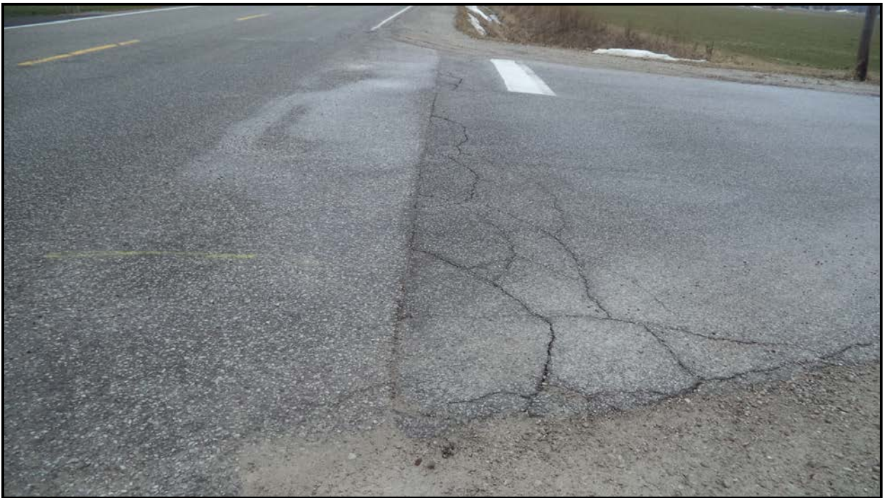
Photograph 6 – Wearing Surface at South Approach
