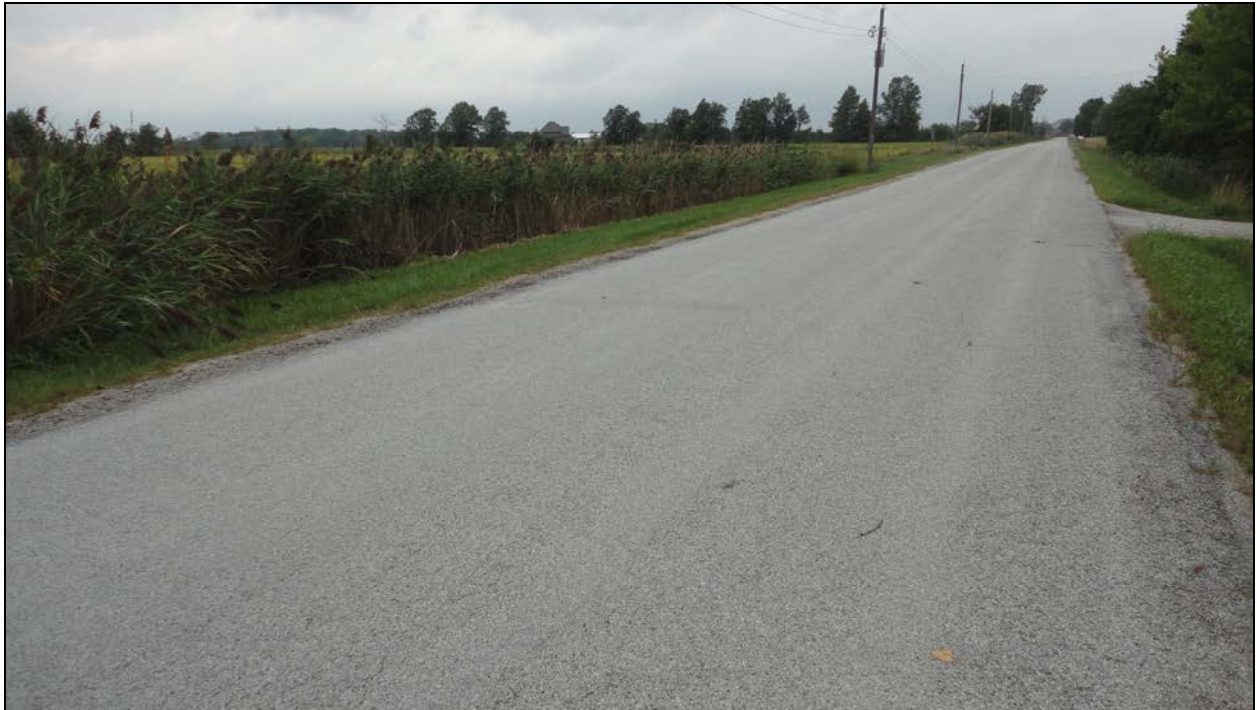
Photograph 1 – Wearing Surface over Culvert (Looking North)
