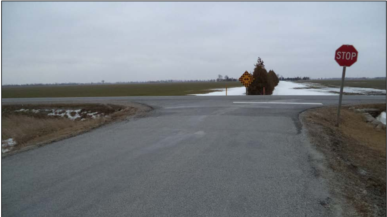
Photograph 1 – Road over Culvert (Looking South)
