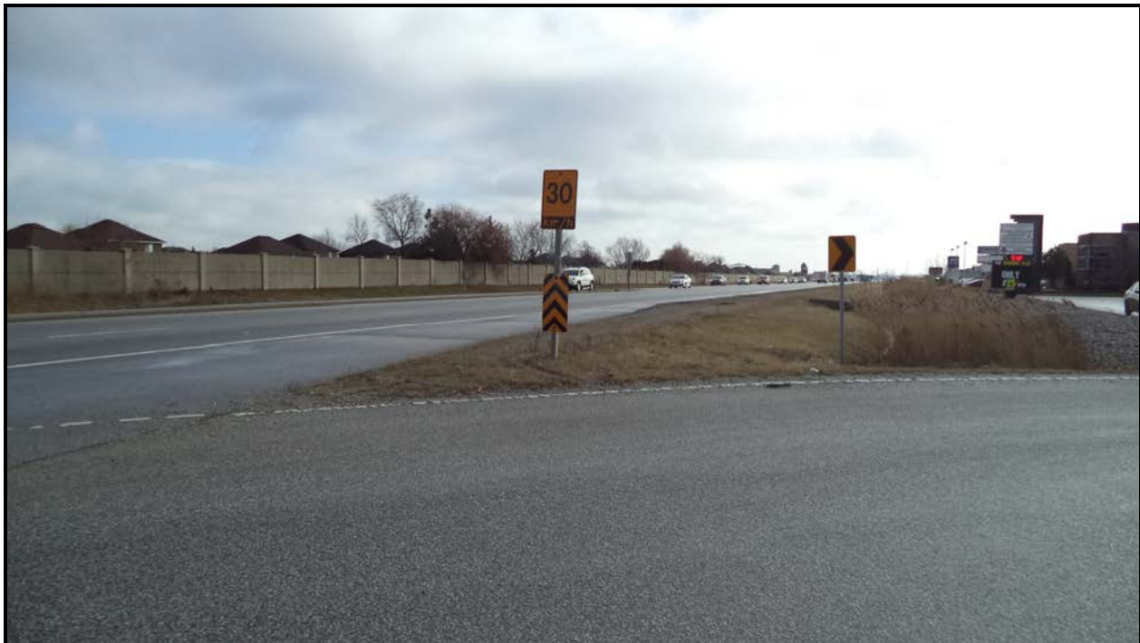
Photograph 2 – Road over Culvert (Looking East)
