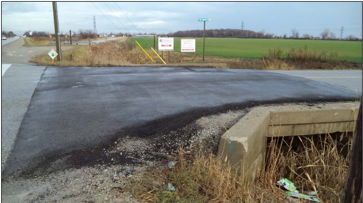
Photograph 7 – Wearing Surface over Culvert (Looking North)
