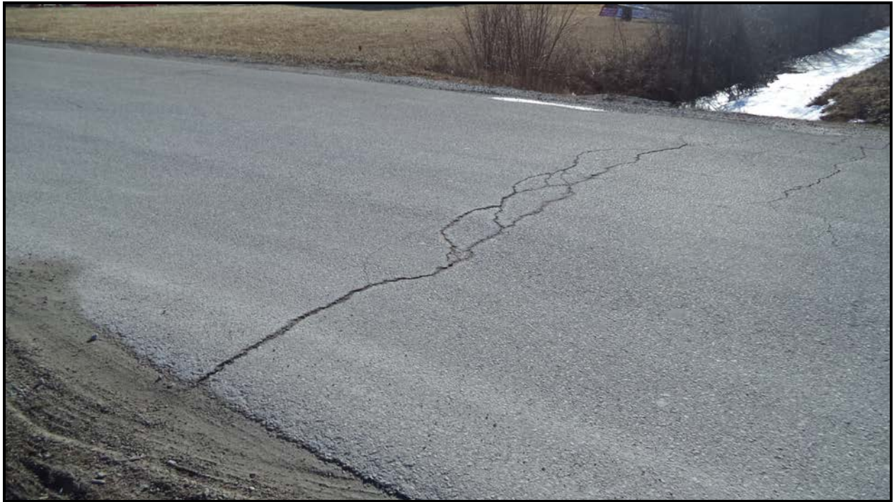
Photograph 5 – Wearing Surface over Culvert (Looking South)
