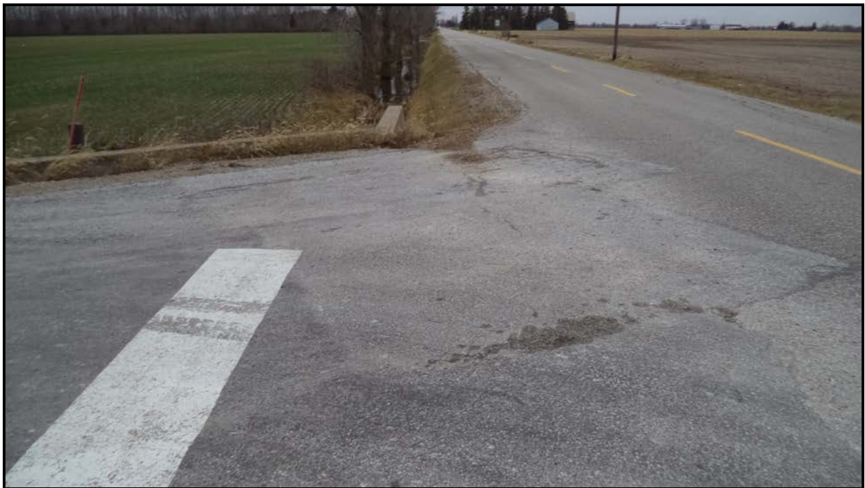
Photograph 6 – Wearing Surface over Culvert (Looking West)
