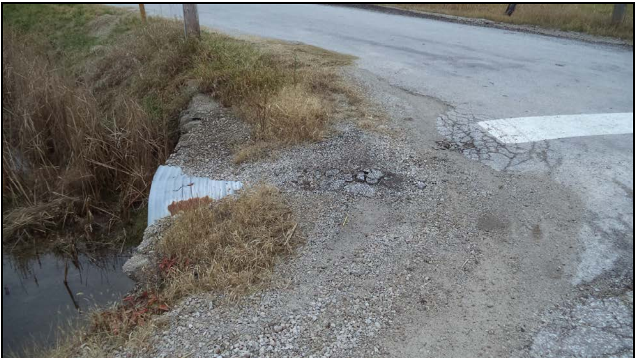
Photograph 8 – Wearing Surface over Culvert (Looking West)
