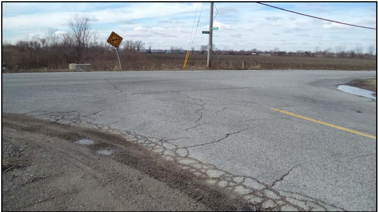
Photograph 6 – Wearing Surface at East Approach (Looking West)
