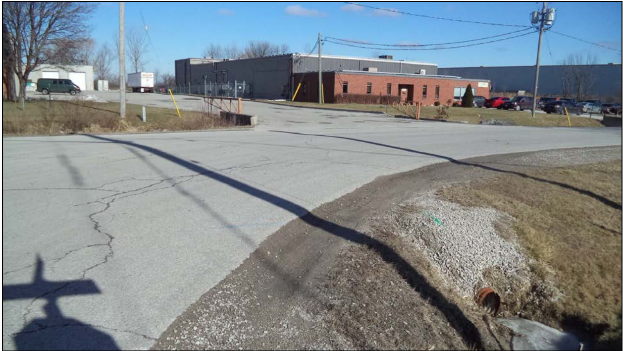
Photograph 1 – Road over Culvert (Looking South)
