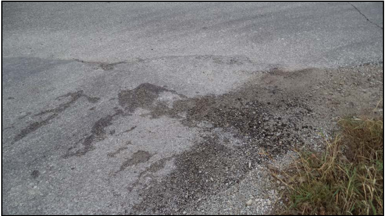
Photograph 7 – Wearing Surface over Culvert Deck
