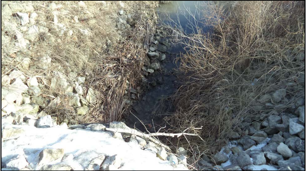
Photograph 5 – Water Stream (Blackacre Drive North Side - Looking North)
