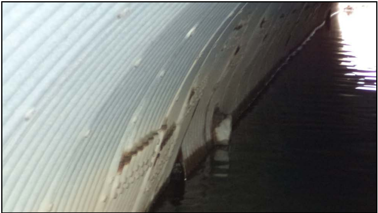
Photograph 4 – Culvert Barrel Connection
