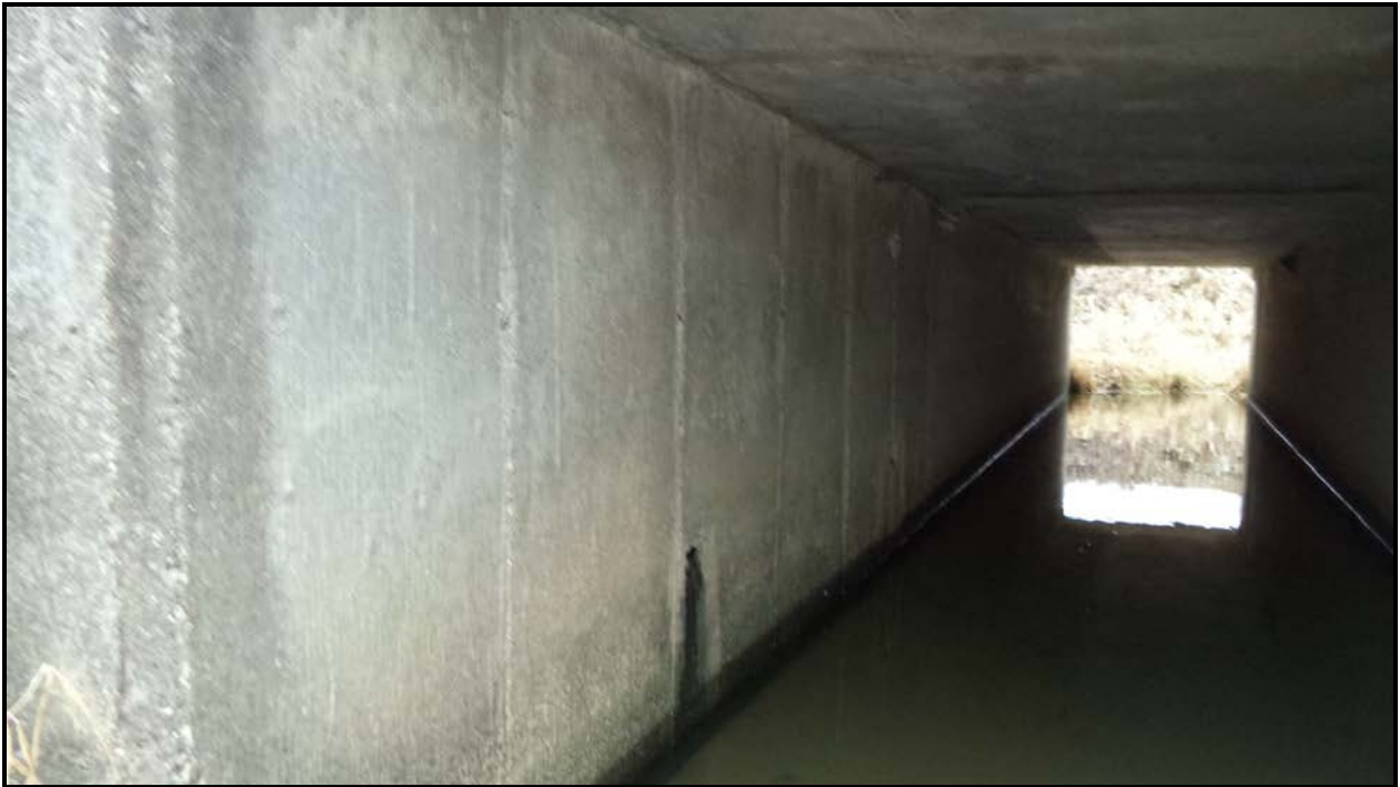
Photograph 2 – Culvert inside Box (Looking North)
