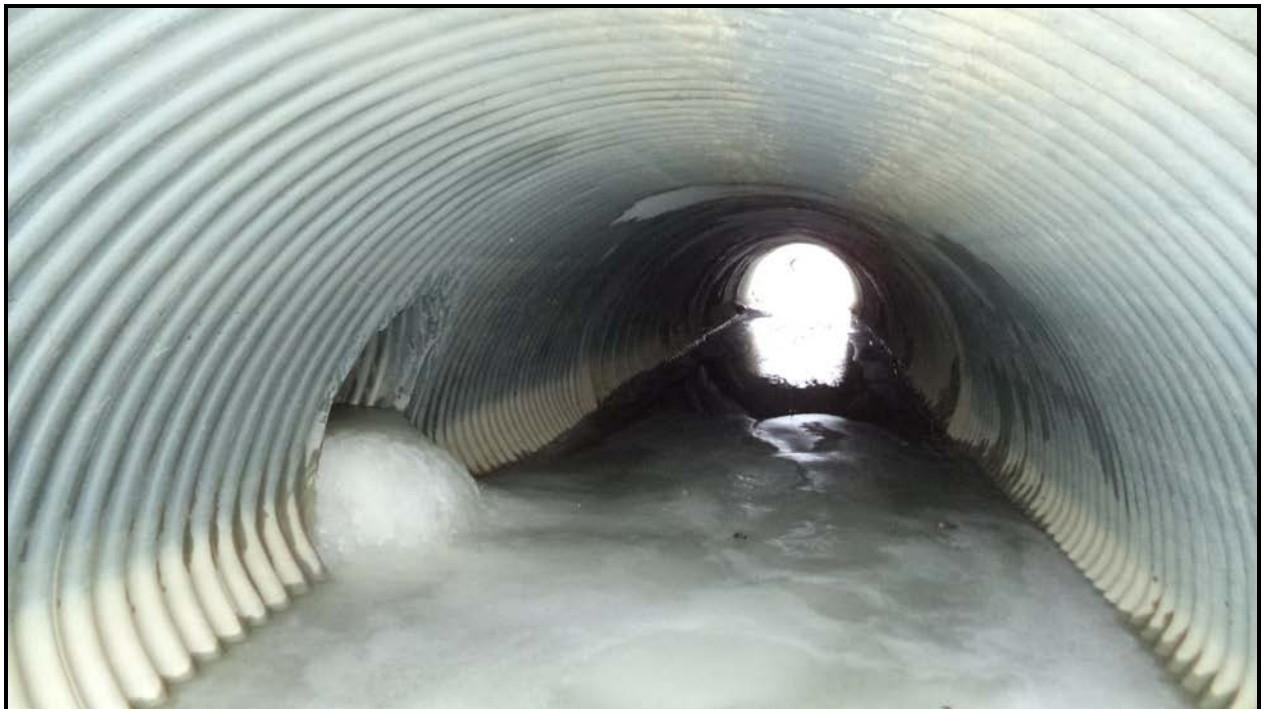
Photograph 2 – Culvert Barrel (Looking West)
