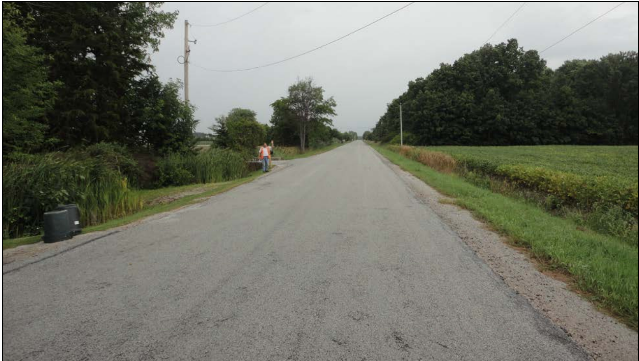
Photograph 1 – Road view over Culvert (Looking North)
