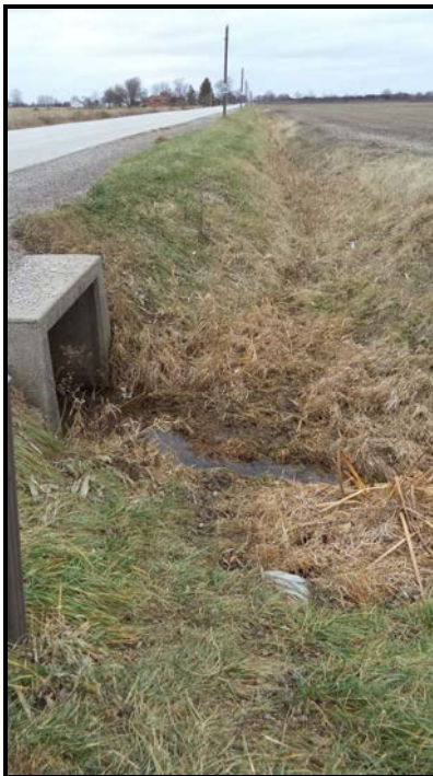
Photograph 8 – Water Stream (S. Talbot Road North Side - Looking West)
