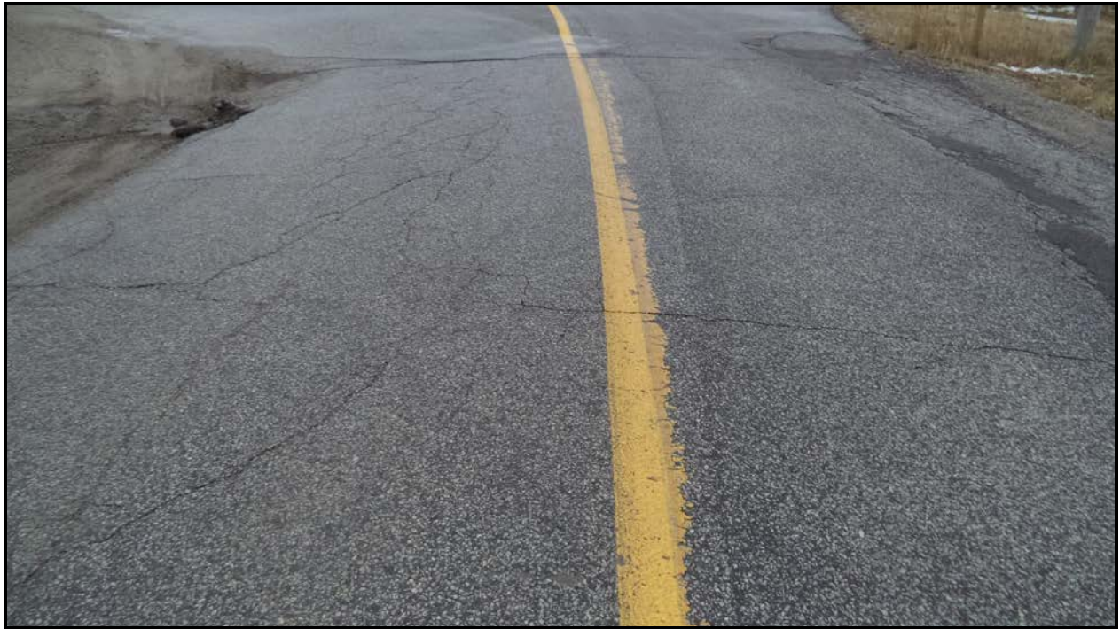
Photograph 5 – Wearing Surface over Culvert (Looking South)
