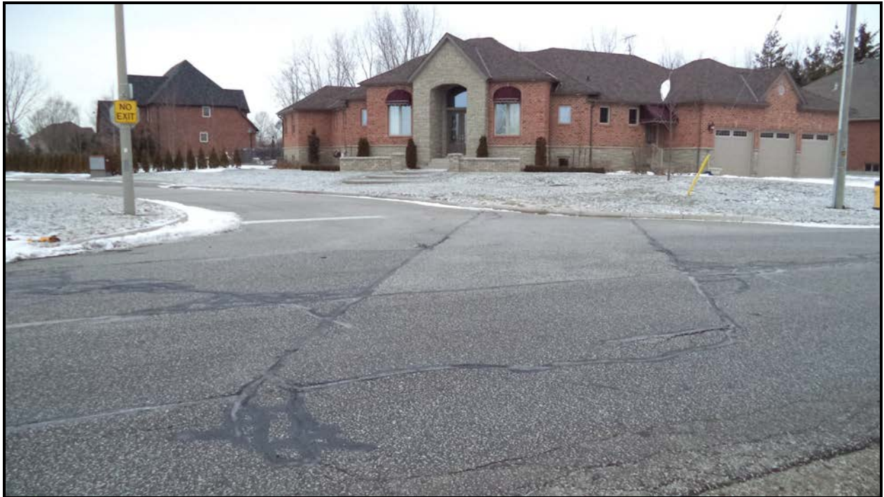
Photograph 5 – Wearing Surface over Culvert (Looking West)
