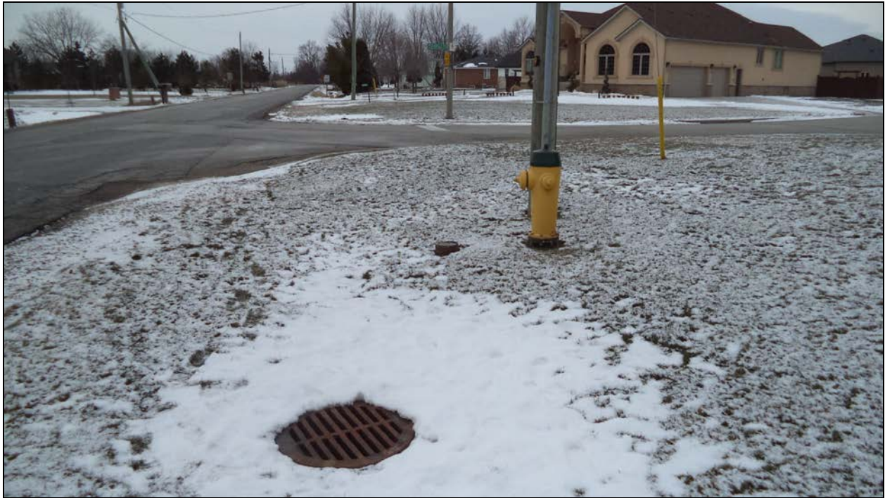
Photograph 1 – Road over Culvert (Looking South)
