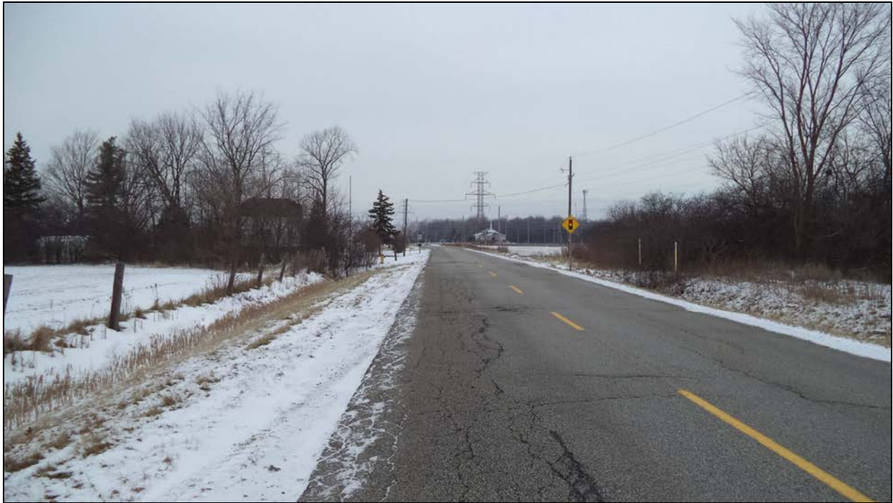
Photograph 1 – Road over Culvert (Looking West)
