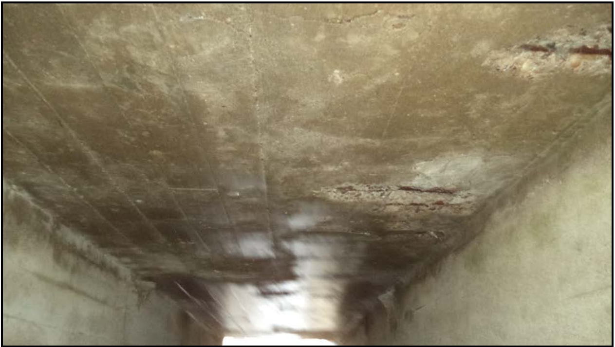
Photograph 2 – Culvert Barrel (Looking East)
