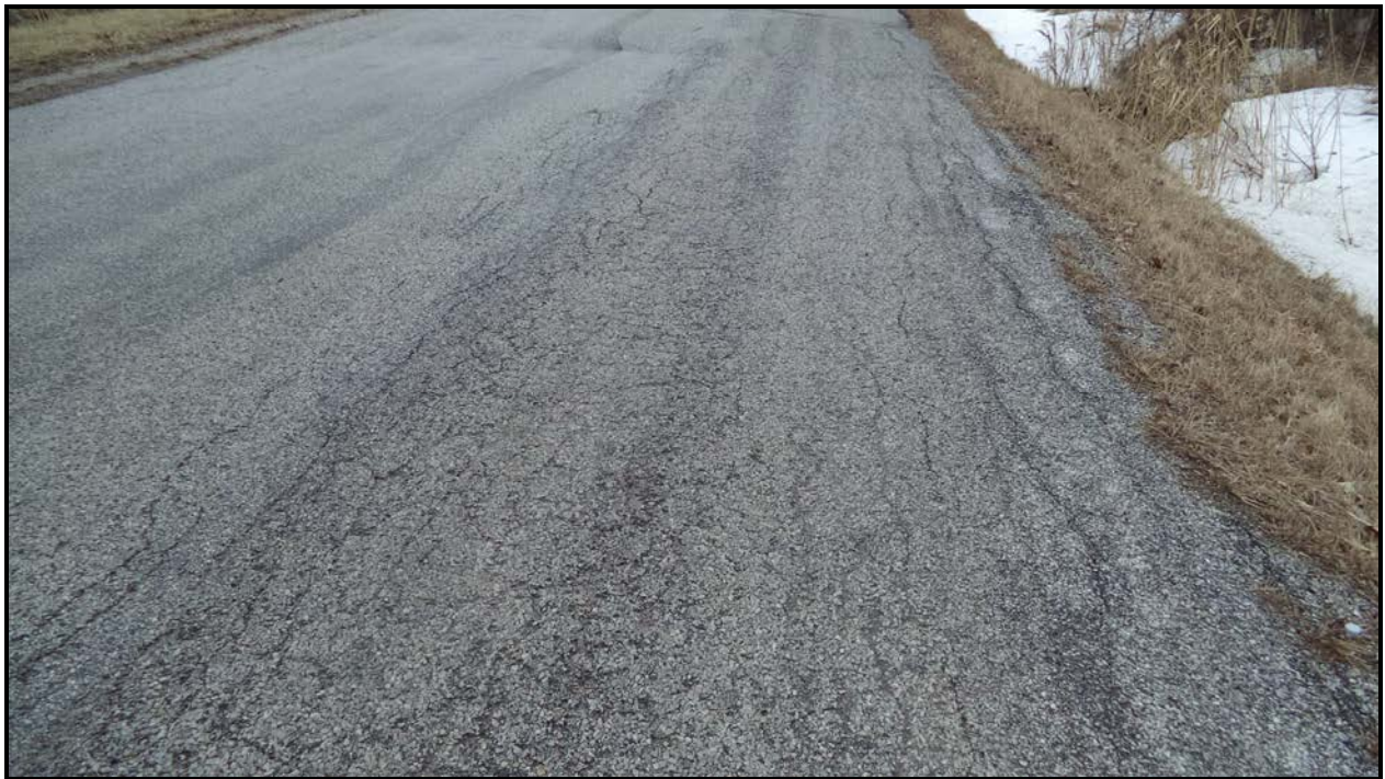
Photograph 6 – Wearing Surface at North Approach
