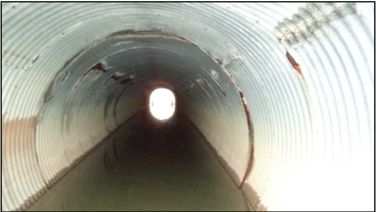
Photograph 2 – Culvert Barrel Looking North
