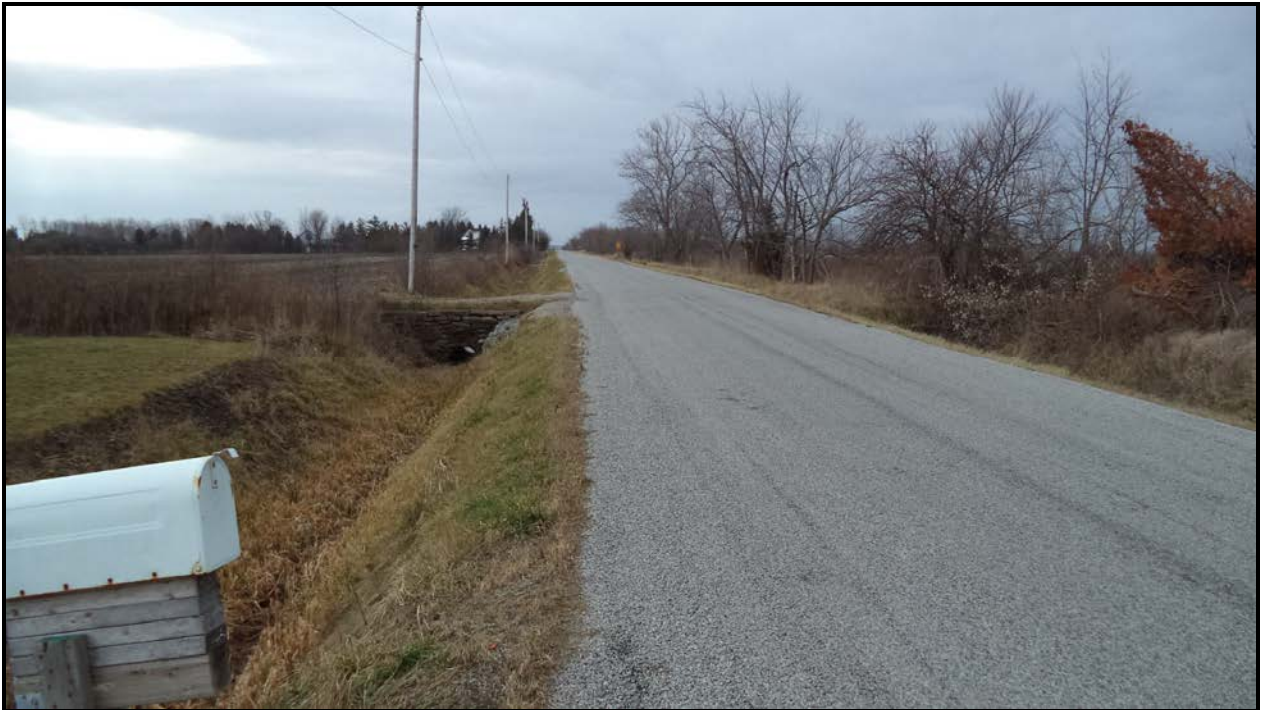
Photograph 1 – Road over Culvert (Looking South)
