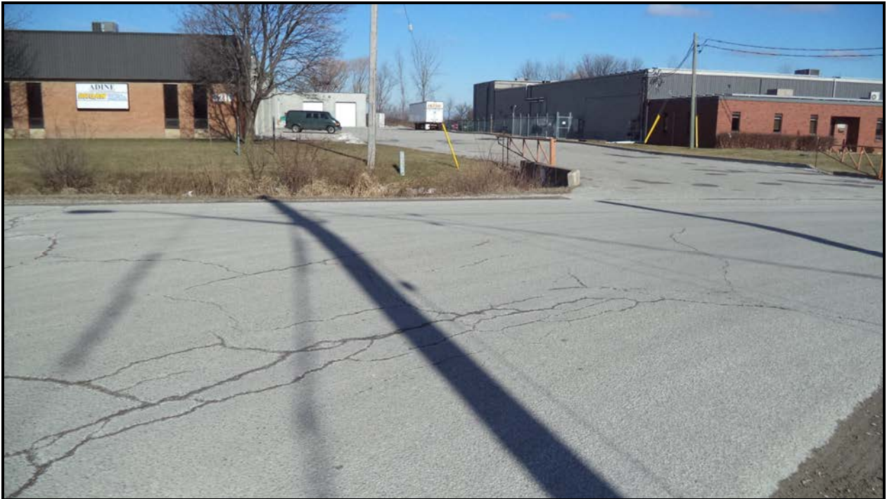
Photograph 5 – Wearing Surface over Culvert (Looking North)
