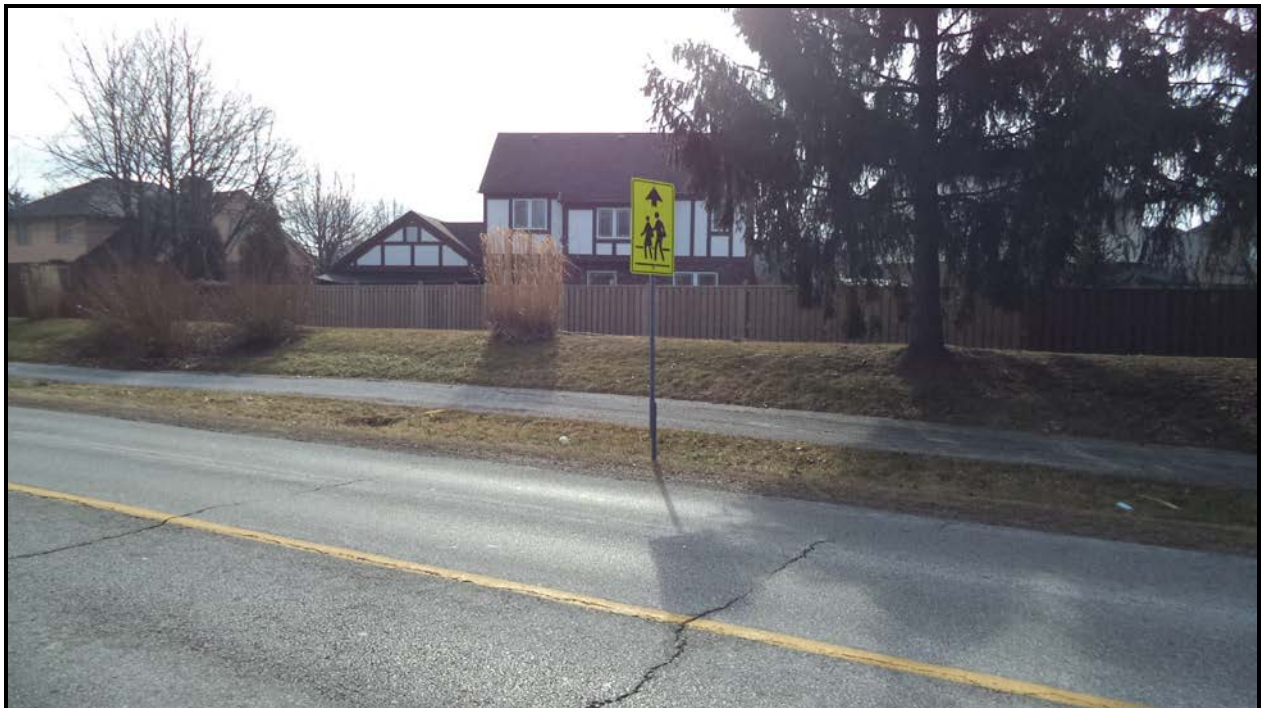
Photograph 6 – Wearing Surface over Culvert (Looking East)
