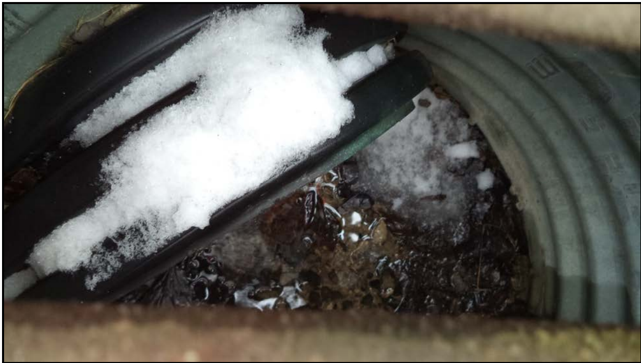
Photograph 2 – Culvert Barrel (at South Inlet)
