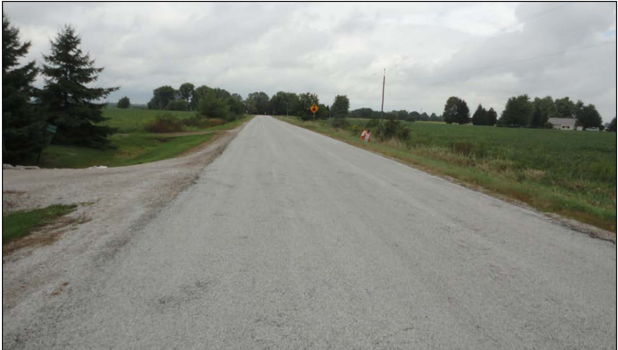
Photograph 1 – Road view over Culvert (Looking North)
