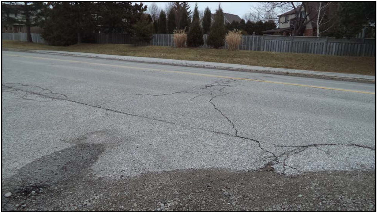
Photograph 6 – Wearing Surface at South Approach
