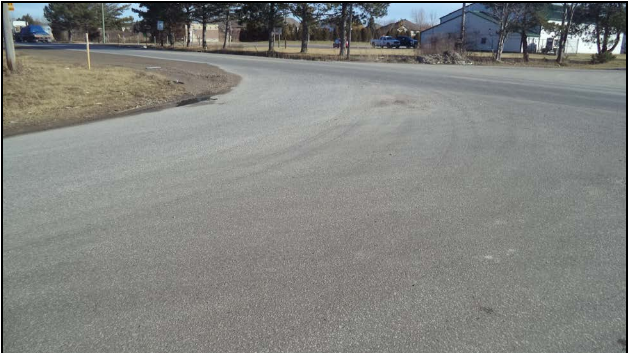
Photograph 5 – Wearing Surface over Culvert (Looking South)
