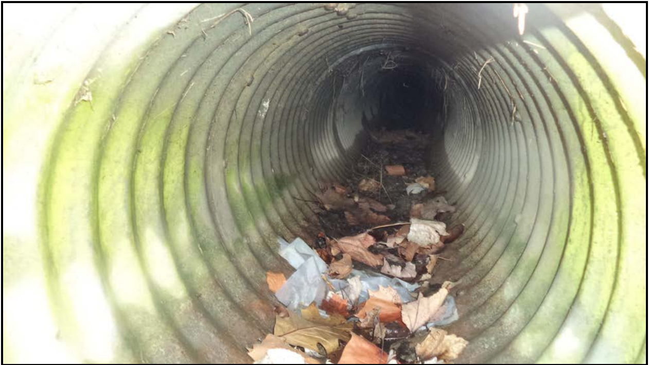
Photograph 2 – Culvert Barrel
