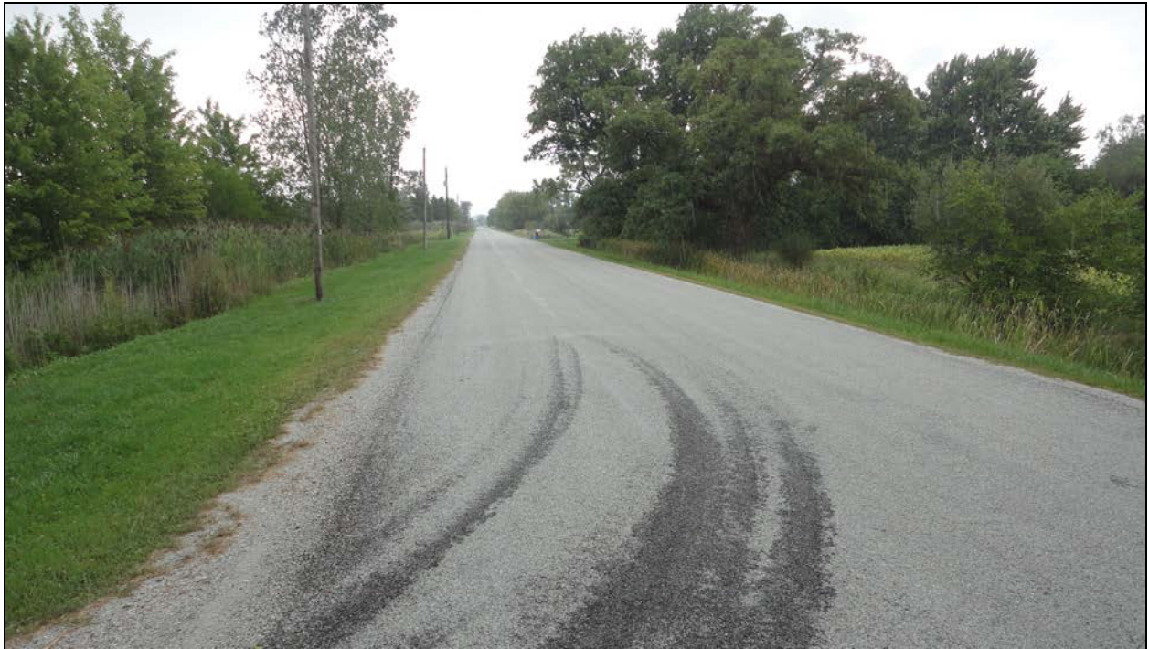
Photograph 1 – Wearing Surface over Culvert (Looking North)
