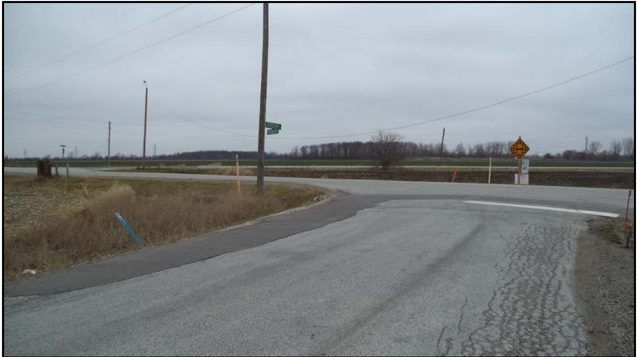
Photograph 1 – Road over Culvert (Looking North)
