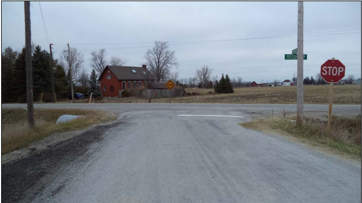
Photograph 1 – Road over Culvert (Looking North)
