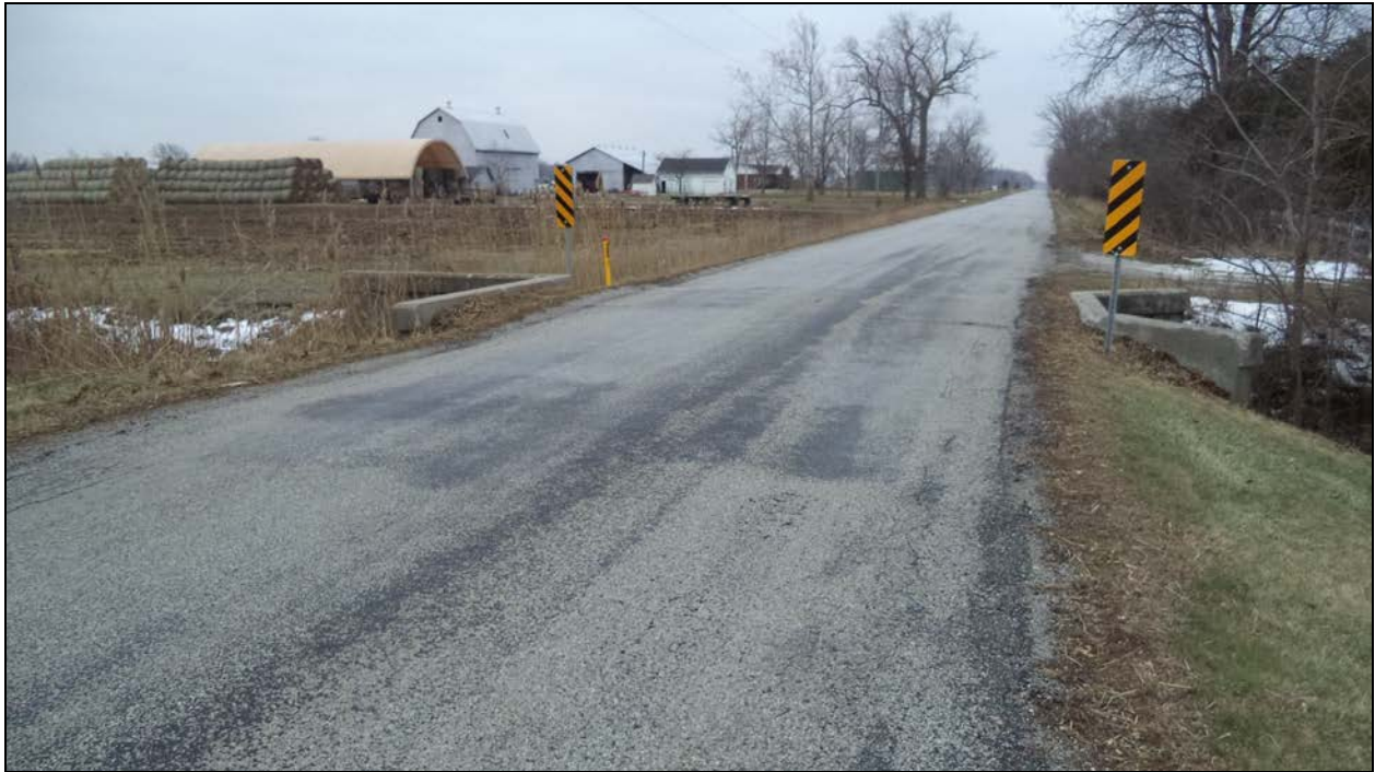
Photograph 1 – Road over Culvert (Looking South)
