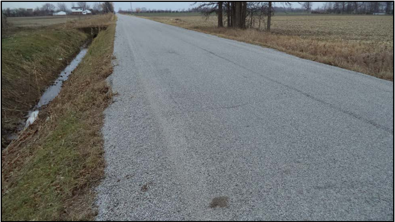
Photograph 1 – Road over Culvert (Looking South)
