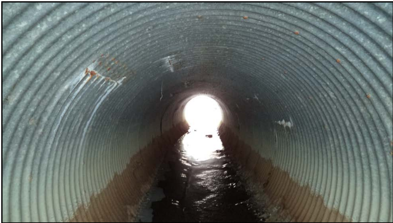
Photograph 2 – Culvert Barrel (Looking South)
