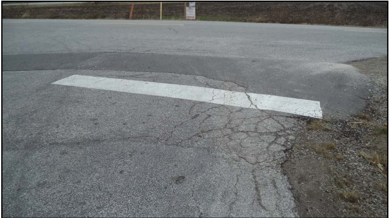
Photograph 5 – Wearing Surface over Culvert (Looking North)
