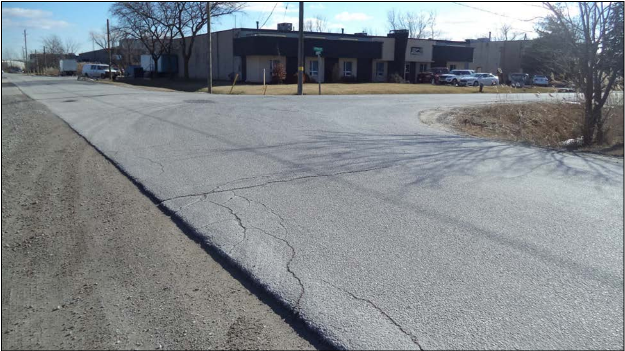
Photograph 1 – Road over Culvert (Looking East)
