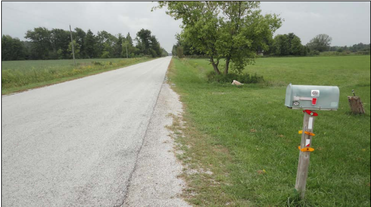
Photograph 1 – Road view over Culvert (Looking South)
