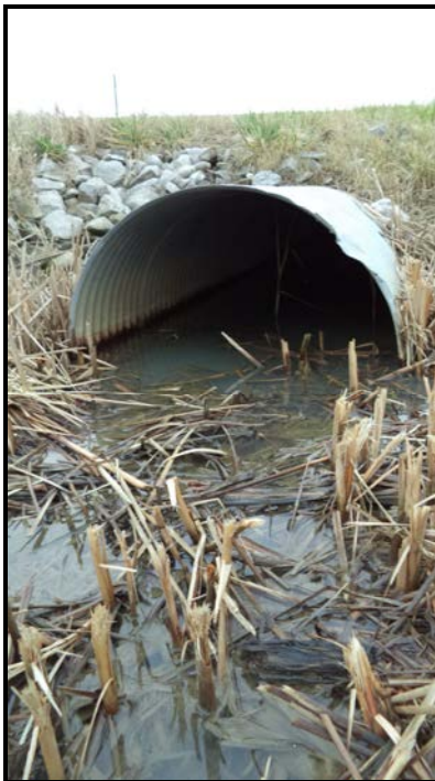
Photograph 2 – Culvert Barrel (West Elevation)
