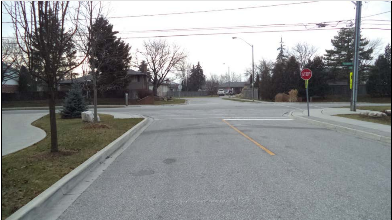
Photograph 1 – Road over Culvert (Looking North)
