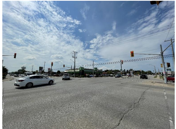
Figure 7: Intersection of Manning and Tecumseh Roads looking northwest.
