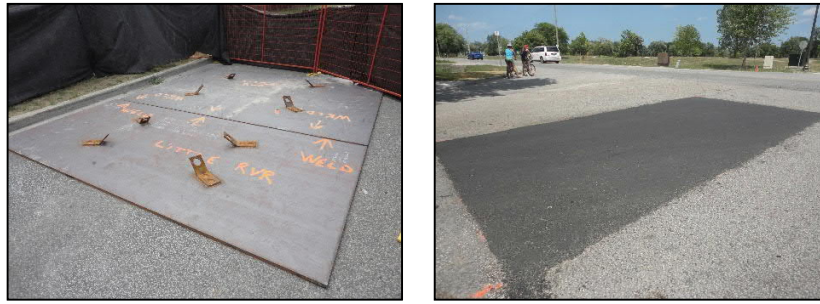
Figure 4: Temporary repair construction (2016)
