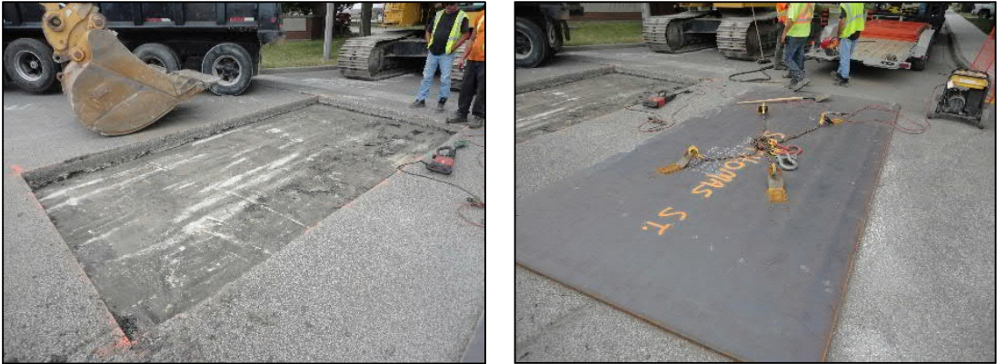
Figure 2: Photos from temporary repairs (2016) construction
