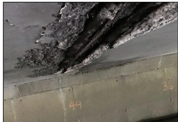
Figure 1: Asphalt over steel plate repair on deck top (left), typ. soffit deterioration (right)
