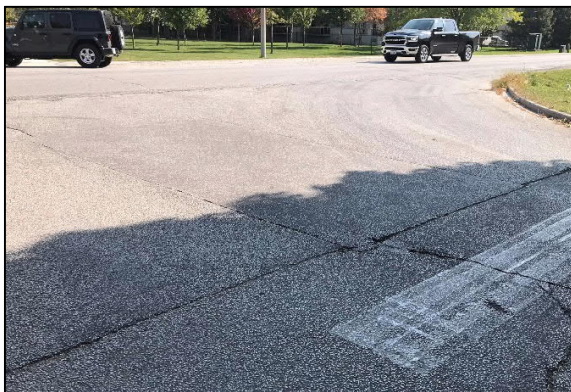
Figure 1: Asphalt over steel plate repair on deck top (left), typ. soffit deterioration (right)
