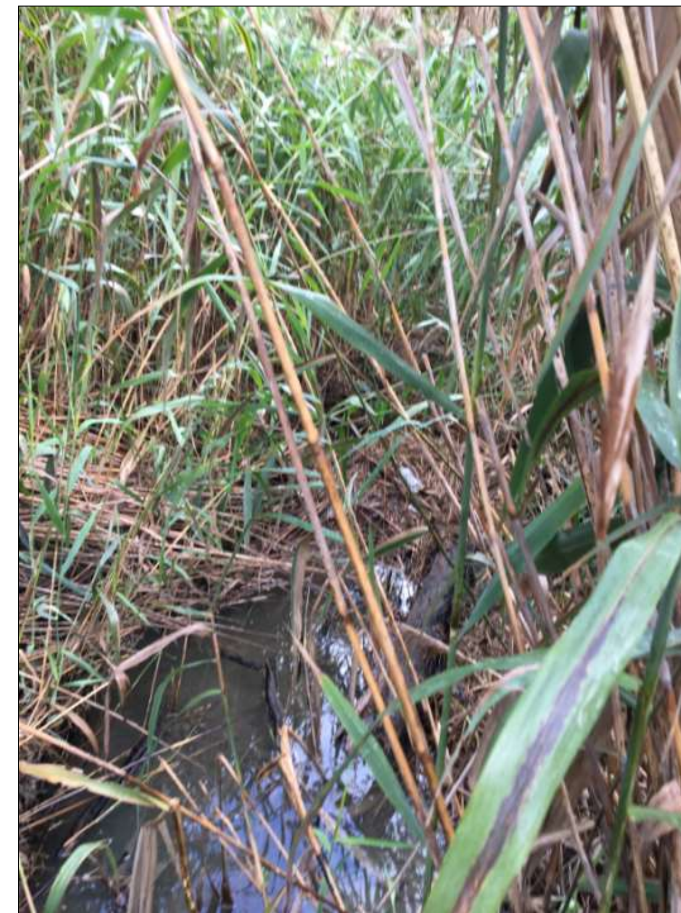
PARTIAL BLOCKAGE IN DRAIN
