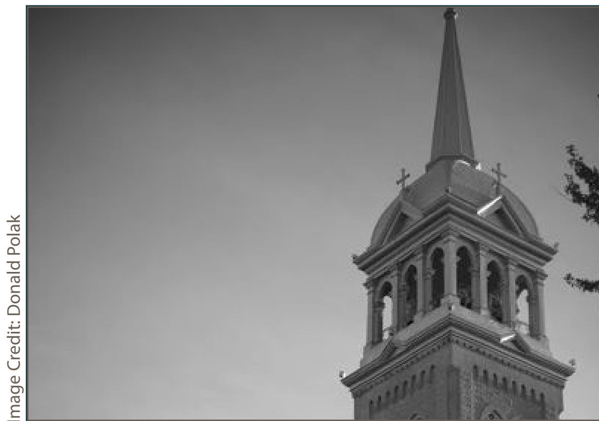
8 Building and Site Improvements - St. Anne Church Restoration
