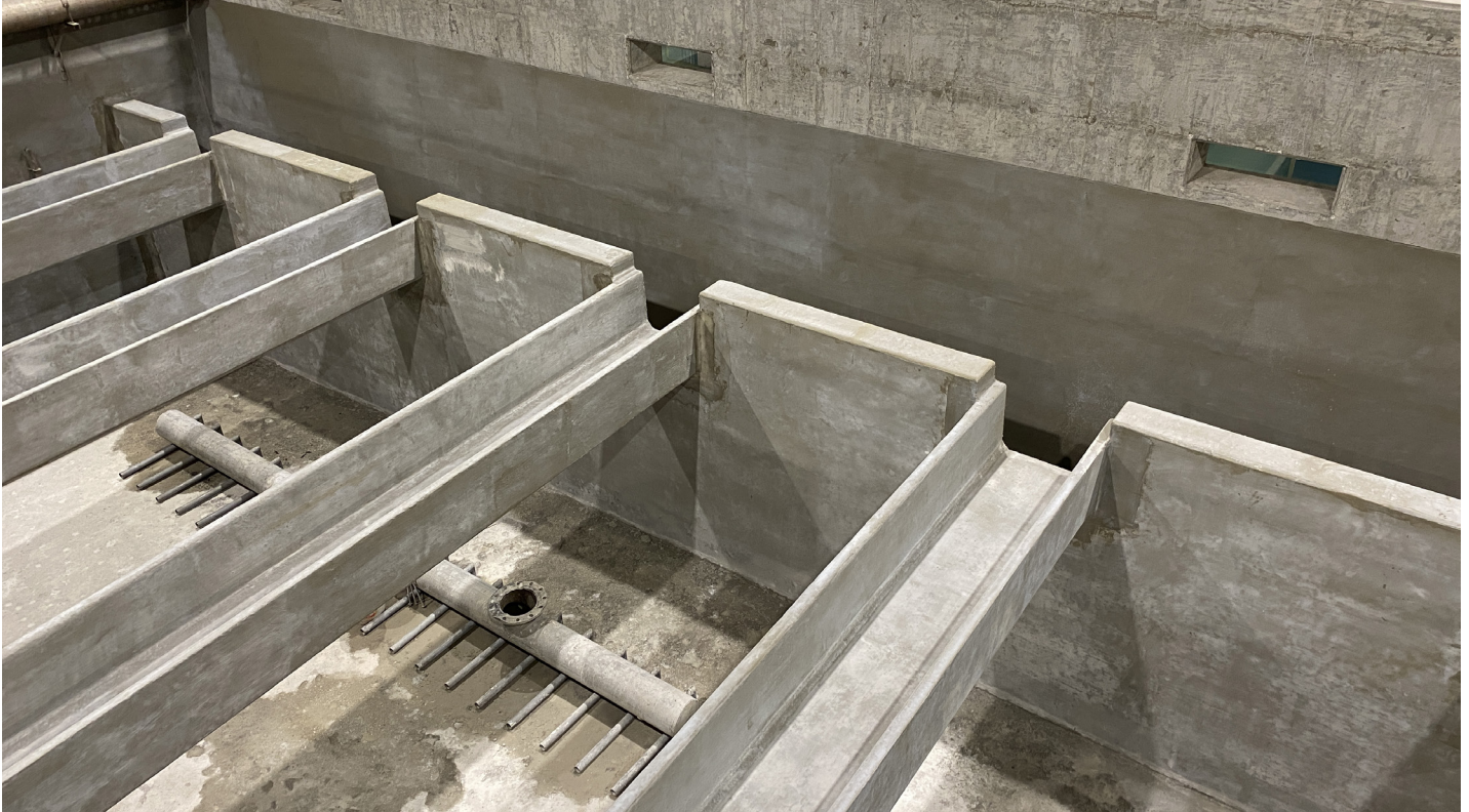
Filter Bed Rehabilitation (Phase 4): Filter #6 concrete surface waterproofing
