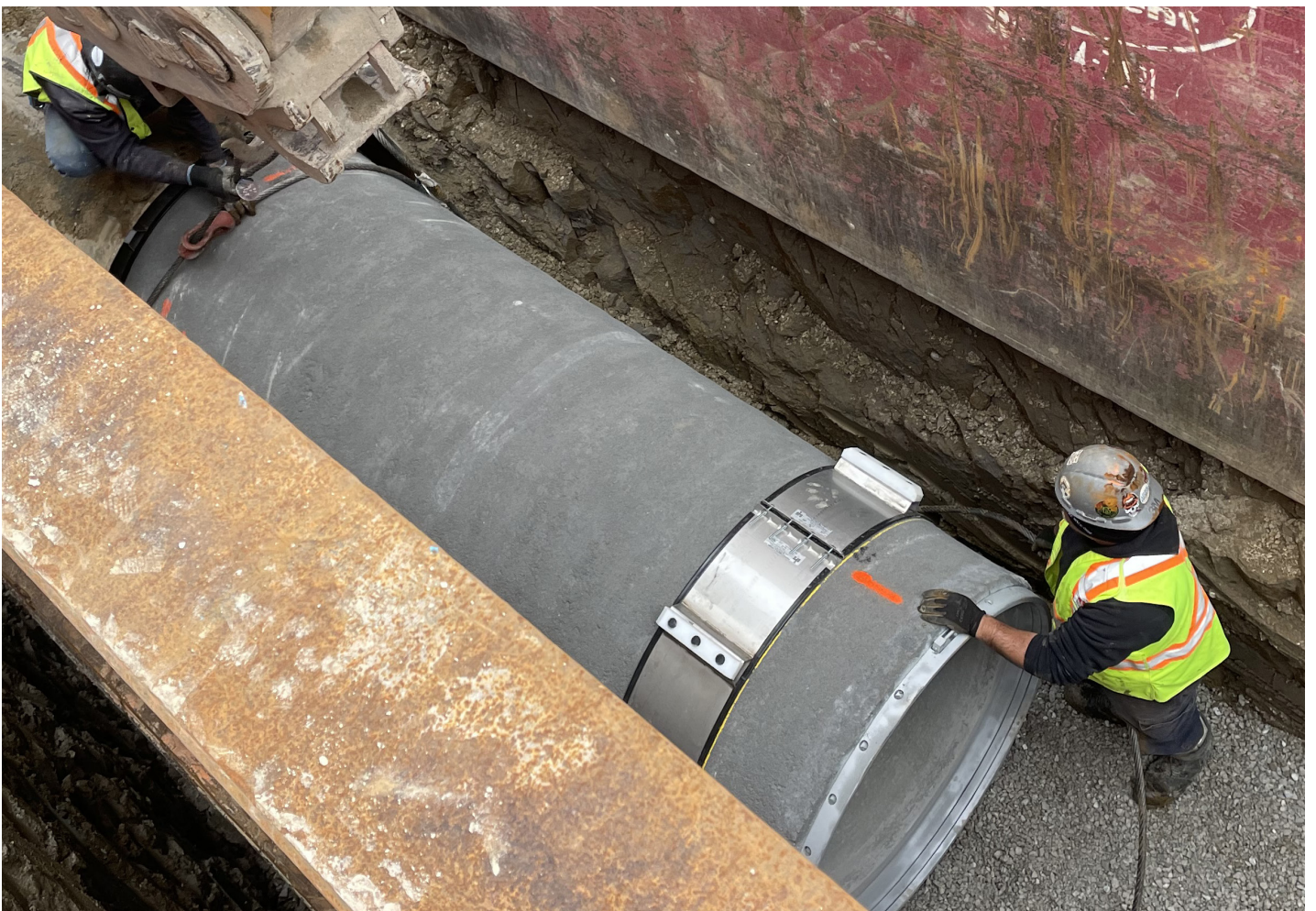
Pipe being placed in the caisson
