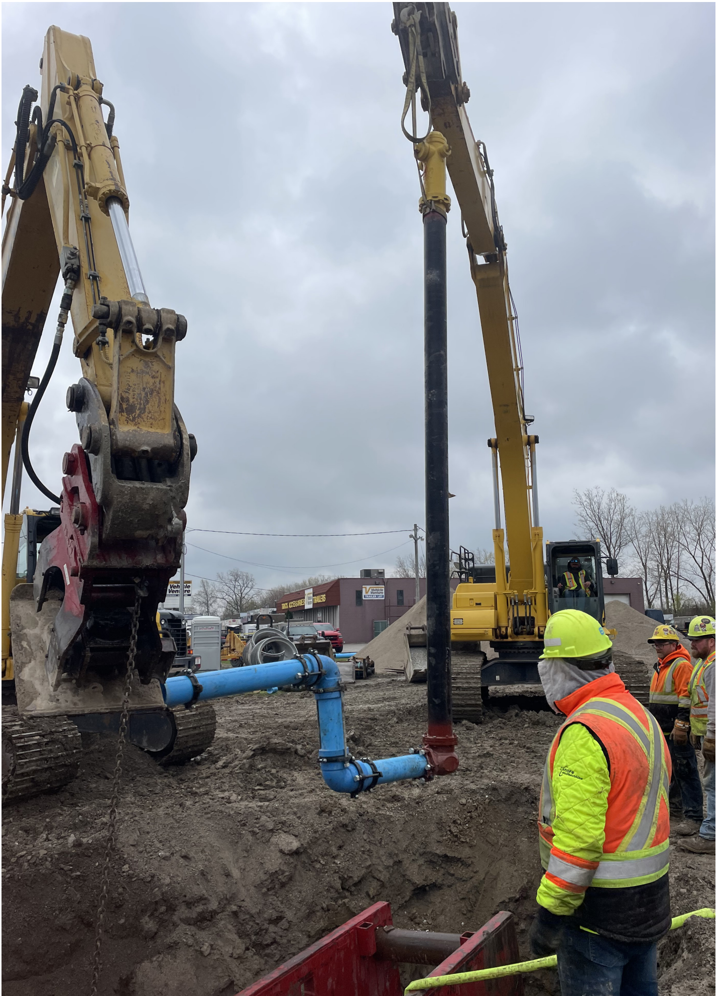
5.0 m hydrant being installed
