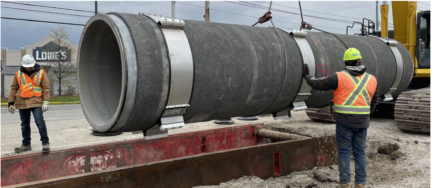
Pipe with spacers ready to be placed in the caisson
