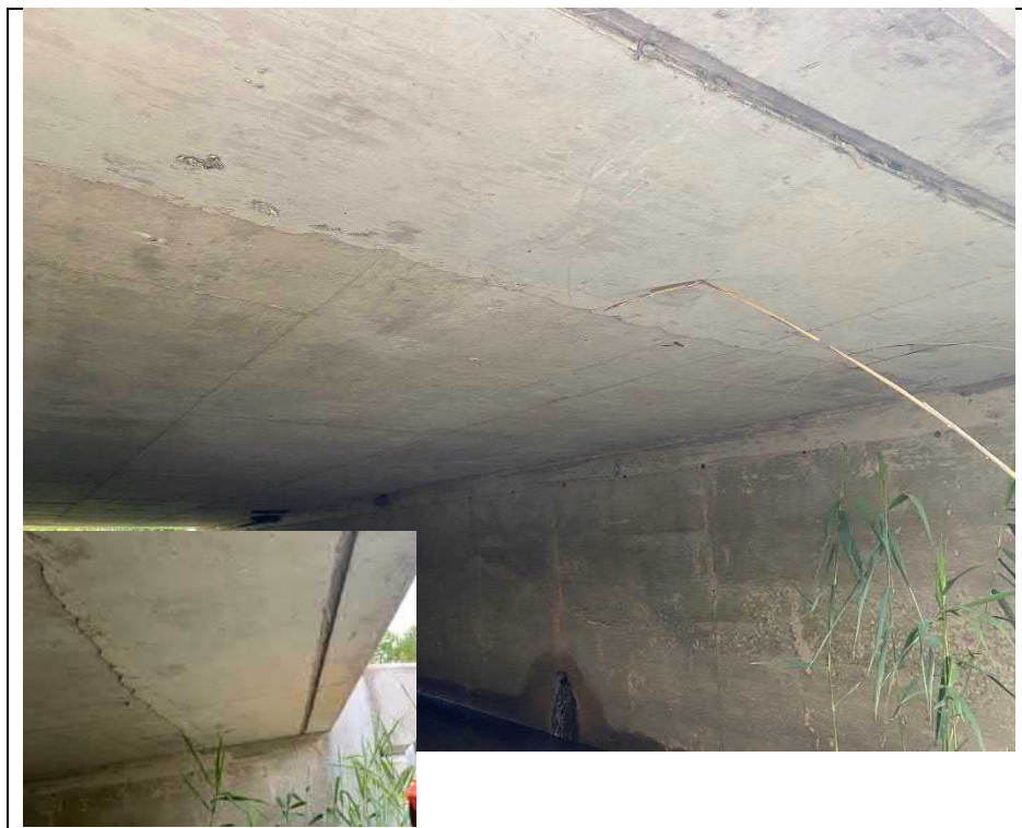
Photograph 8: Typical condition of deck soffit (East end shown)
