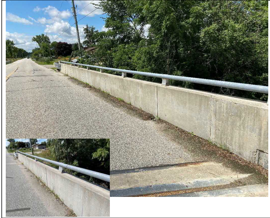
Photograph 9: Typical condition of parapet walls
