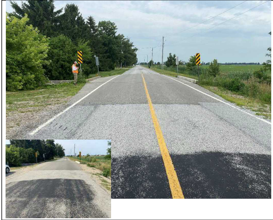
Photograph 1: South approach (Looking North)
