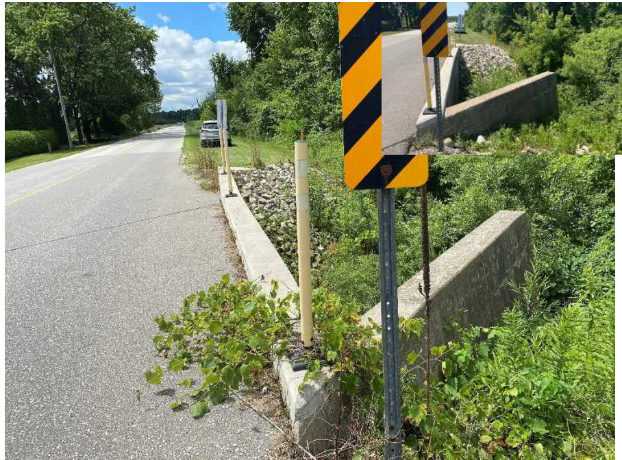
Photograph 3: Object marker and raised curbs on west side (Looking South)
