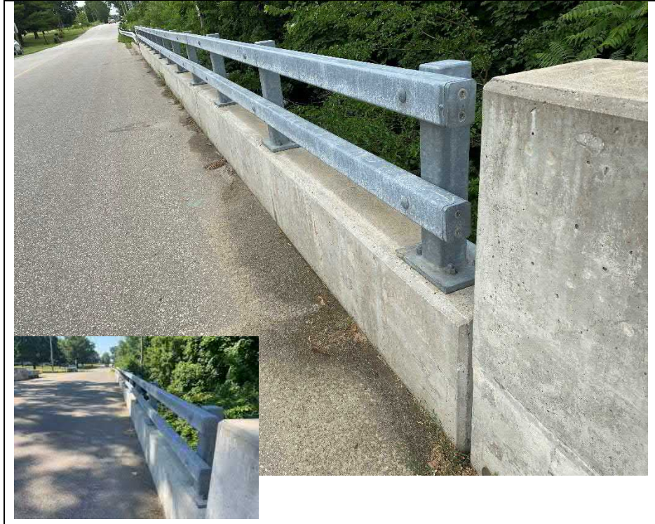
Photograph 9: Parapet wall on the west side of the structure
