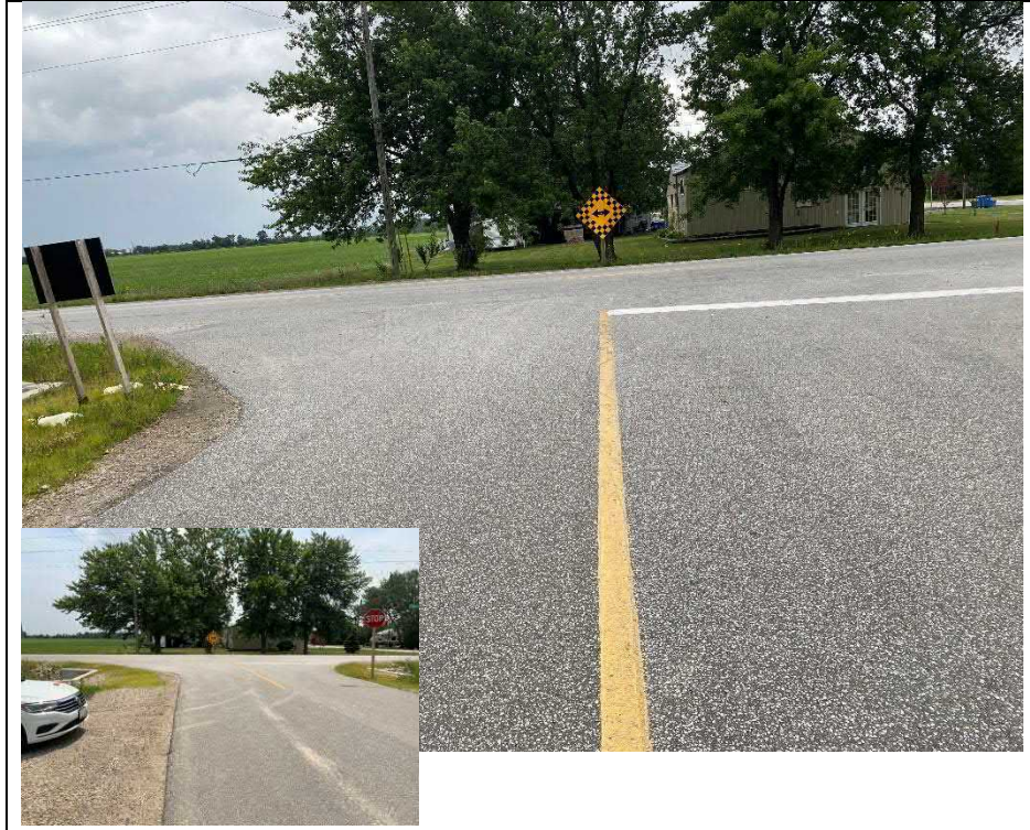
Photograph 1: North approach (Looking South)
