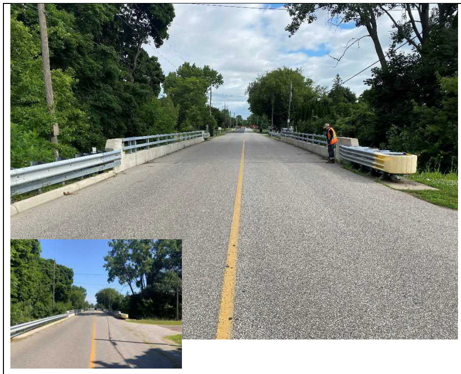
Photograph 2: South approach (Looking North)
