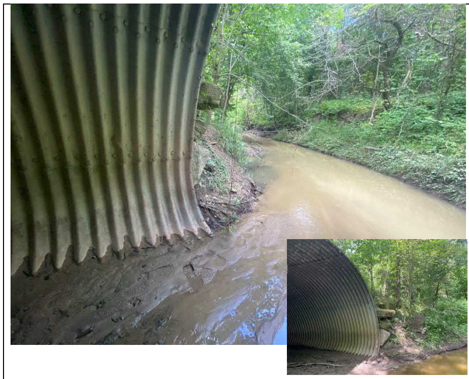
Photograph 8: North spring line (Looking West)
