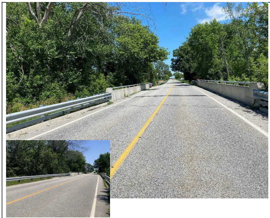
Photograph 2: Overview of structure looking west
