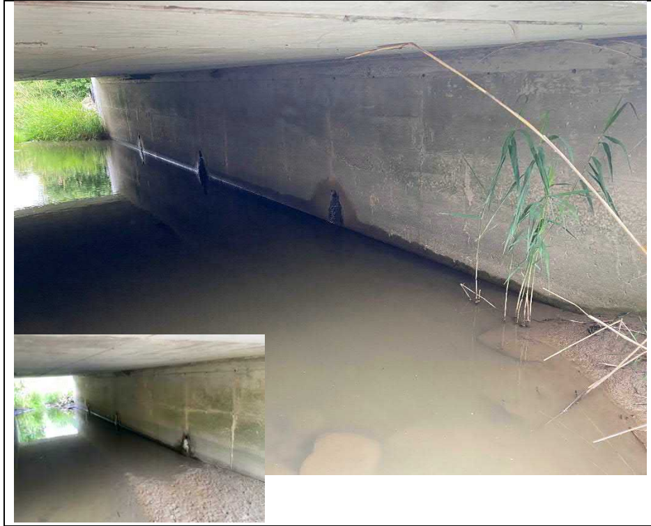
Photograph 9: Abutment wall and deck soffit inside the structure
