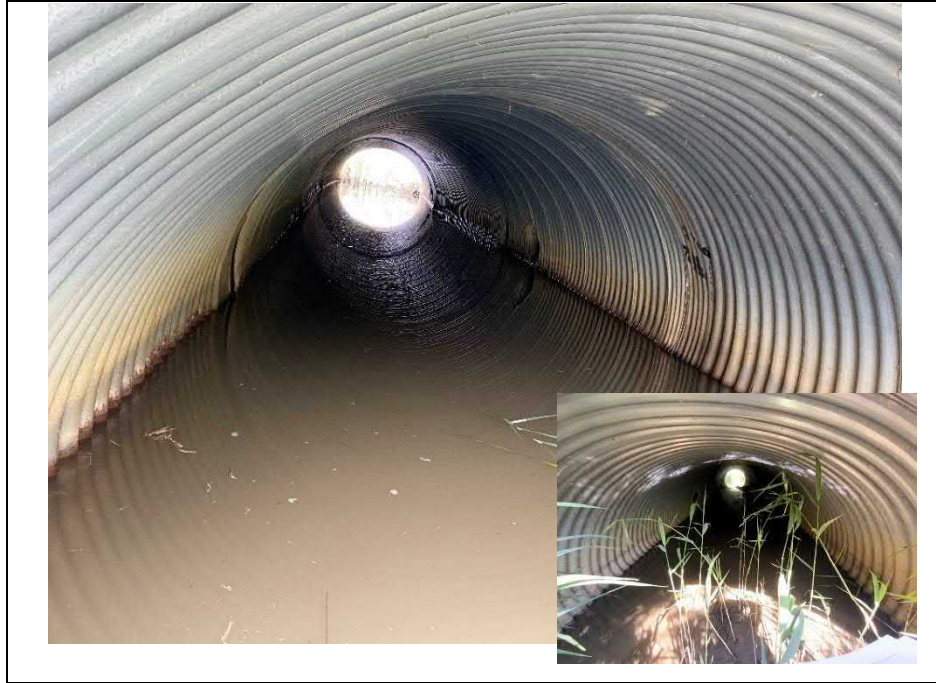
Photograph 7: Typical condition of the culvert barrel
