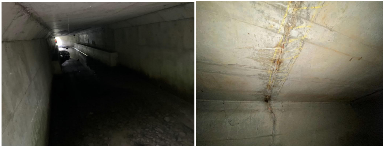
(a) Culvert barrel
