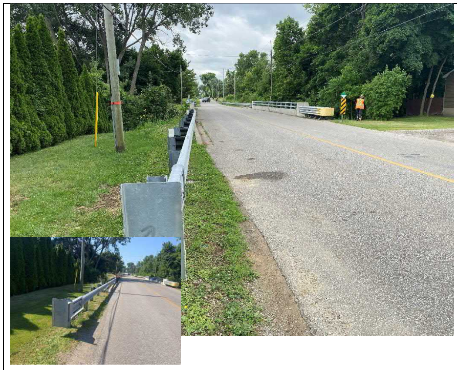
Photograph 8: Guide rail at the north approach
