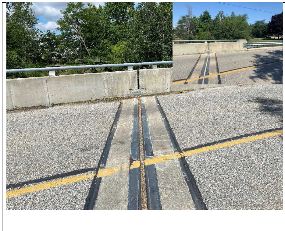
Photograph 6: Typical condition of expansion joints (South joint shown)
