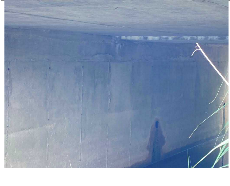
Photograph 11: Soffit patch repair completed in 2019 (Looking Southwest)
