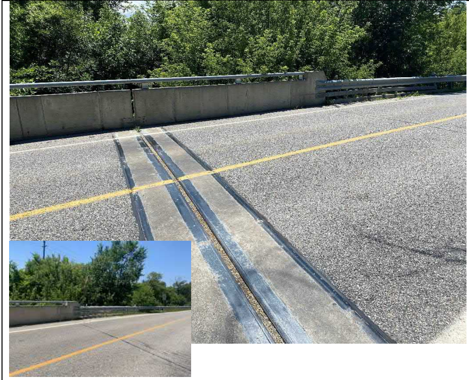
Photograph 5: Expansion joint and railing system at northeast quadrant of structure
