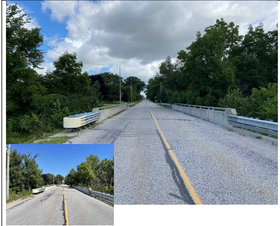
Photograph 1: Overview of structure (Looking North)
