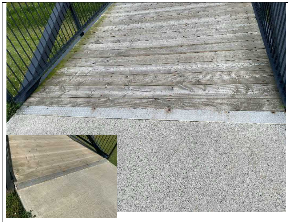
Photograph 16: Threshold plate at east approach
