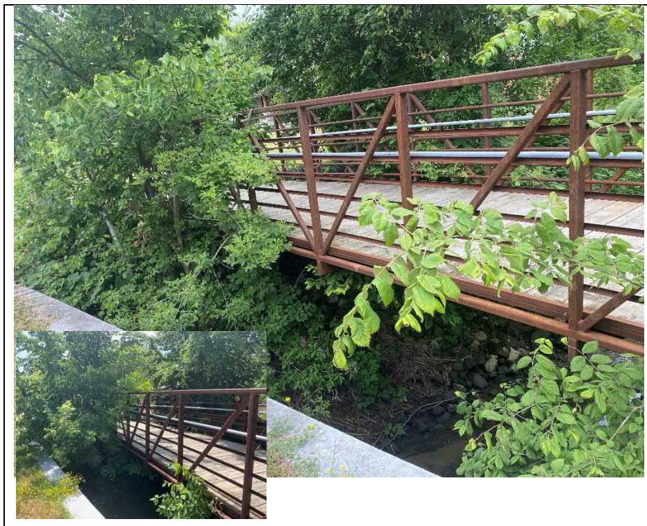
Photograph 8: Typical top chord, railing system, truss verticals and diagonals
