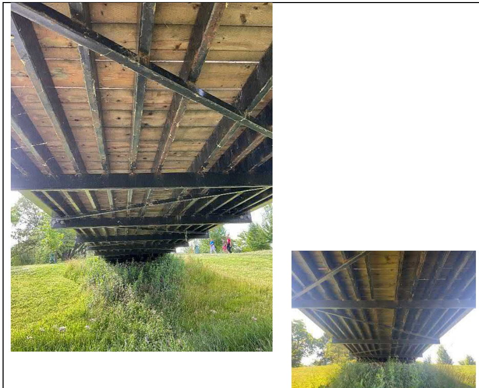
Photograph 8: Underside of deck (Looking West)
