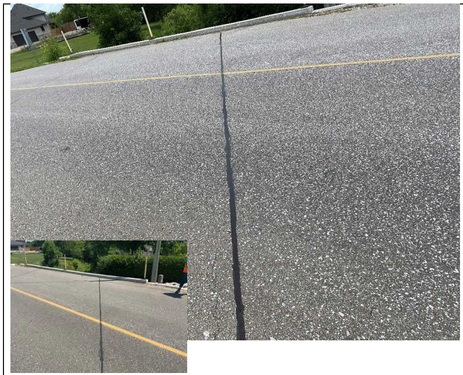
Photograph 2: Wearing surface over the structure (Looking North)
