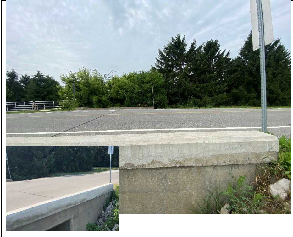
Photograph 3: Wearing surface over the structure (Looking West)
