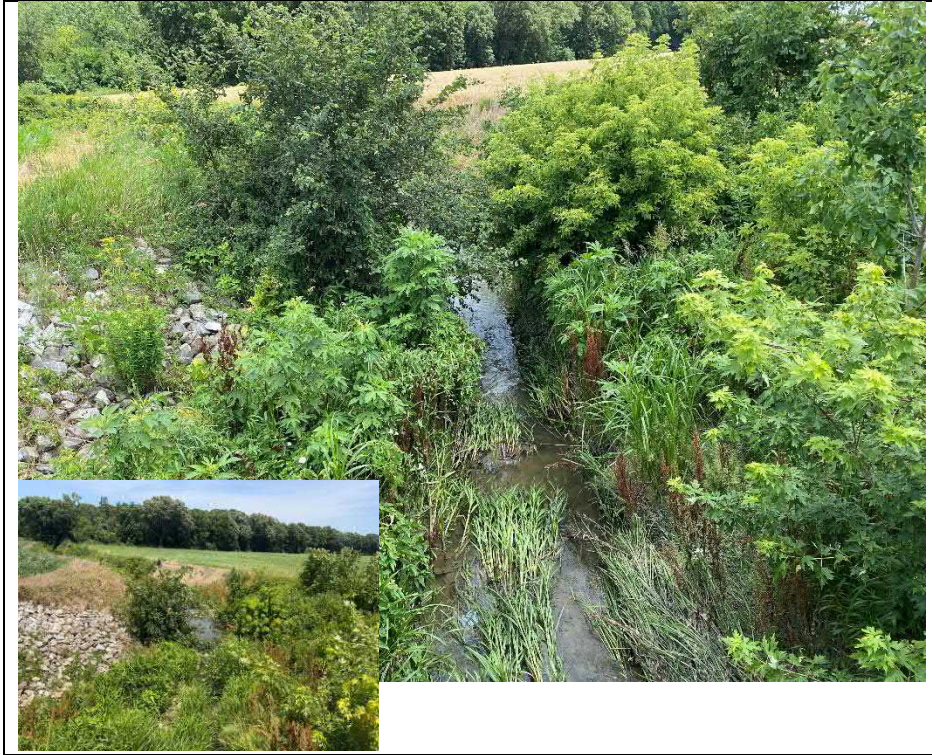
Photograph 13: North embankments and waterway (Looking North)
