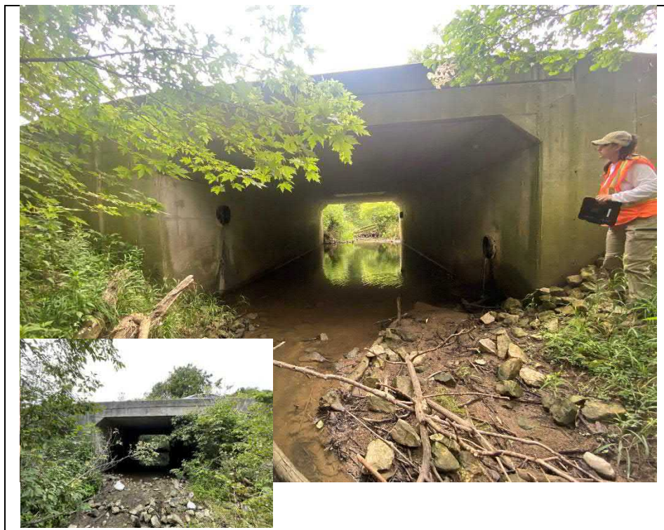
Photograph 6: East elevation (Looking South)
