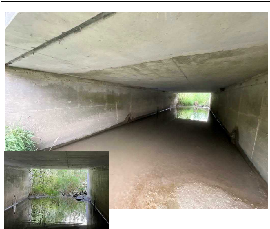
Photograph 6: Typical condition culvert barrel
