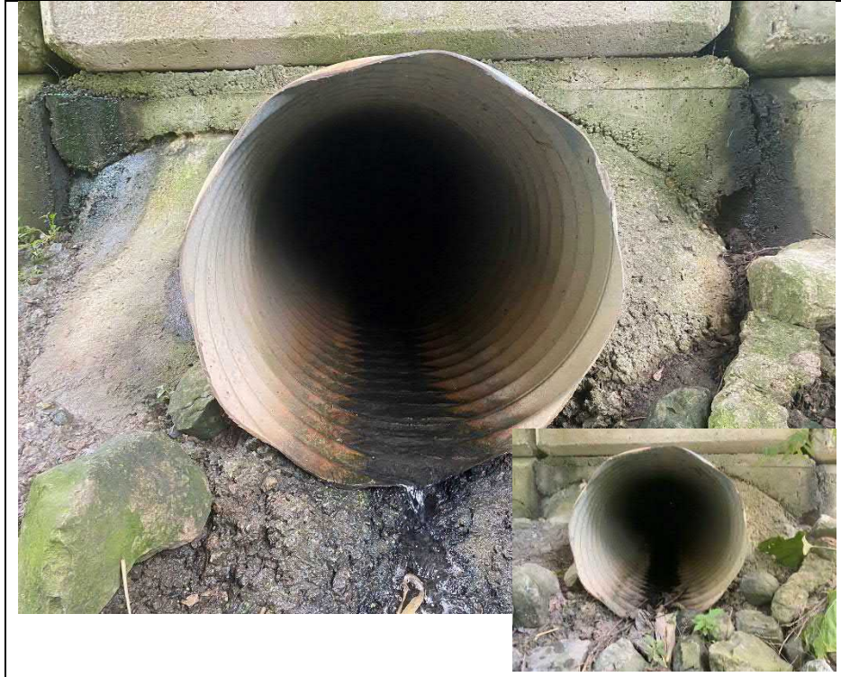
Photograph 11: CSP outlet (Looking North)
