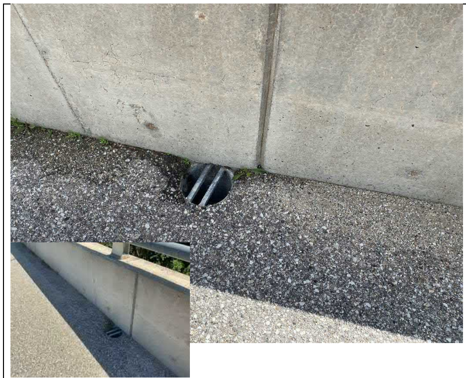
Photograph 8: Deck drainage and east parapet wall (Looking North)
