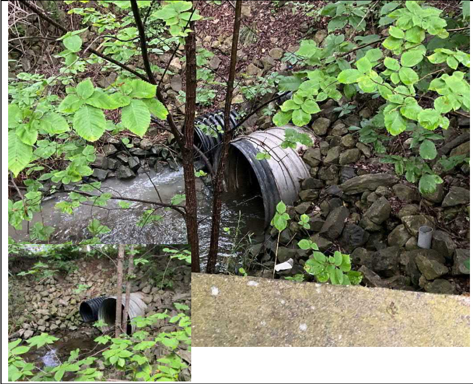
Photograph 15: Watercourse at west extent of culvert (Looking West)
