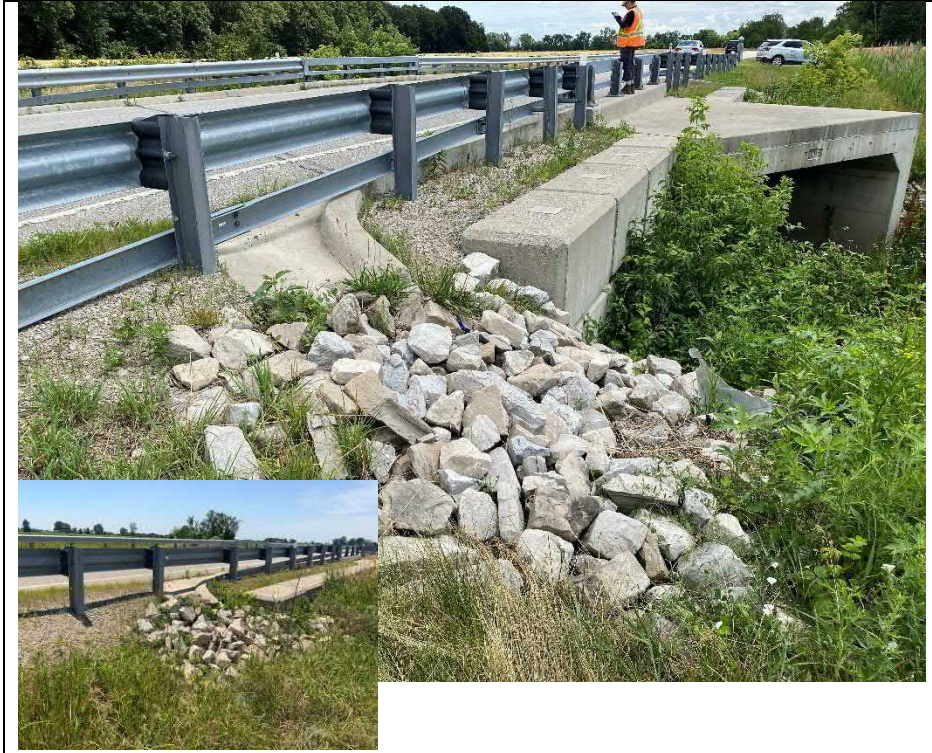
Photograph 5: Spillway at southwest quadrant of structure
