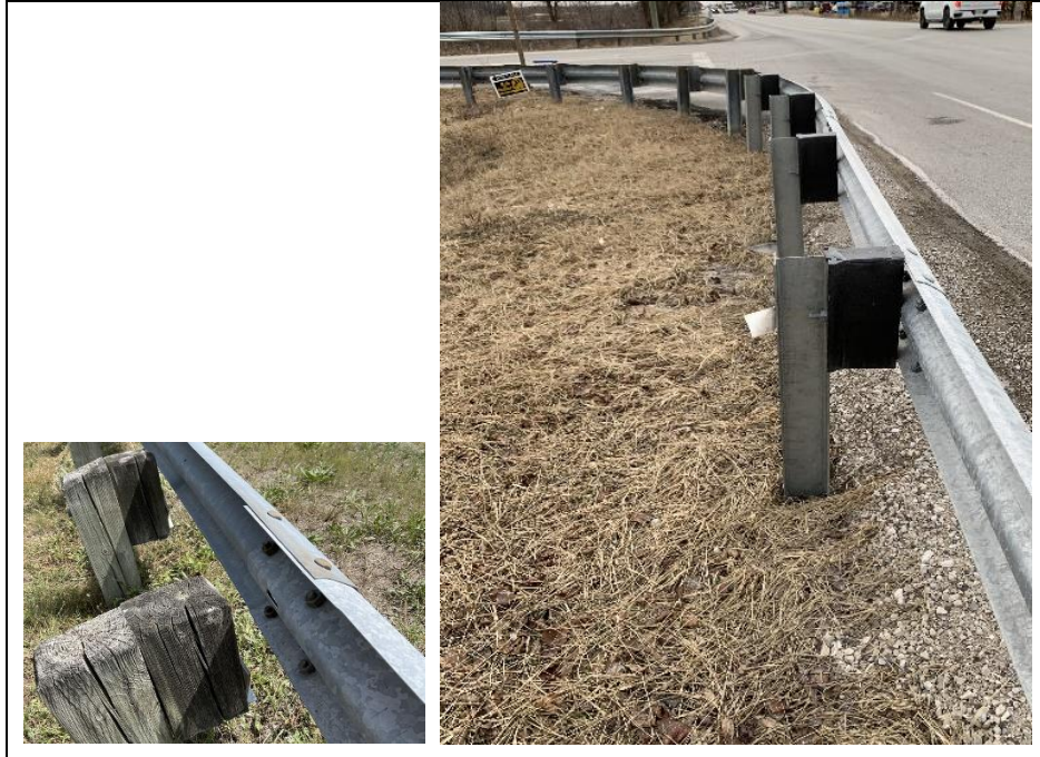
Photograph 7: New typical guiderail posts
