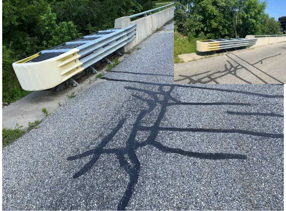
Photograph 3: Wearing surface at the south approach (Looking West)
