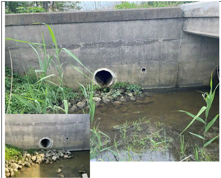
Photograph 8: Typical condition of CSP outlet through the southeast wingwall
