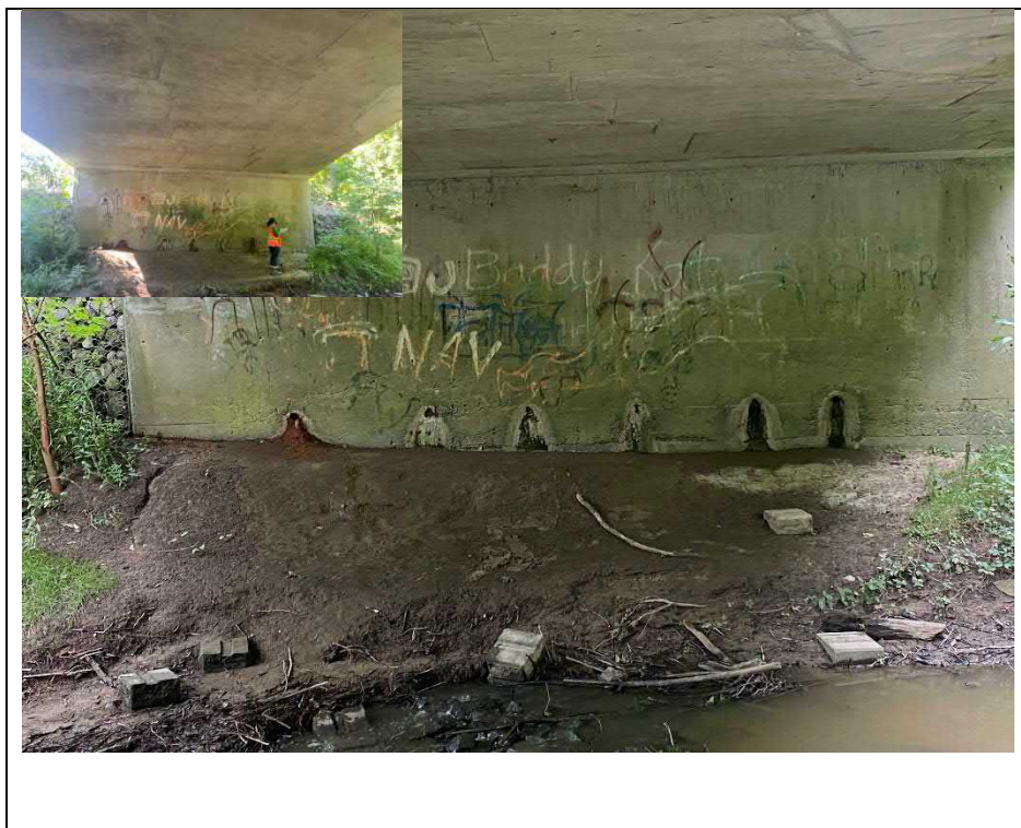
Photograph 16: South abutment wall
