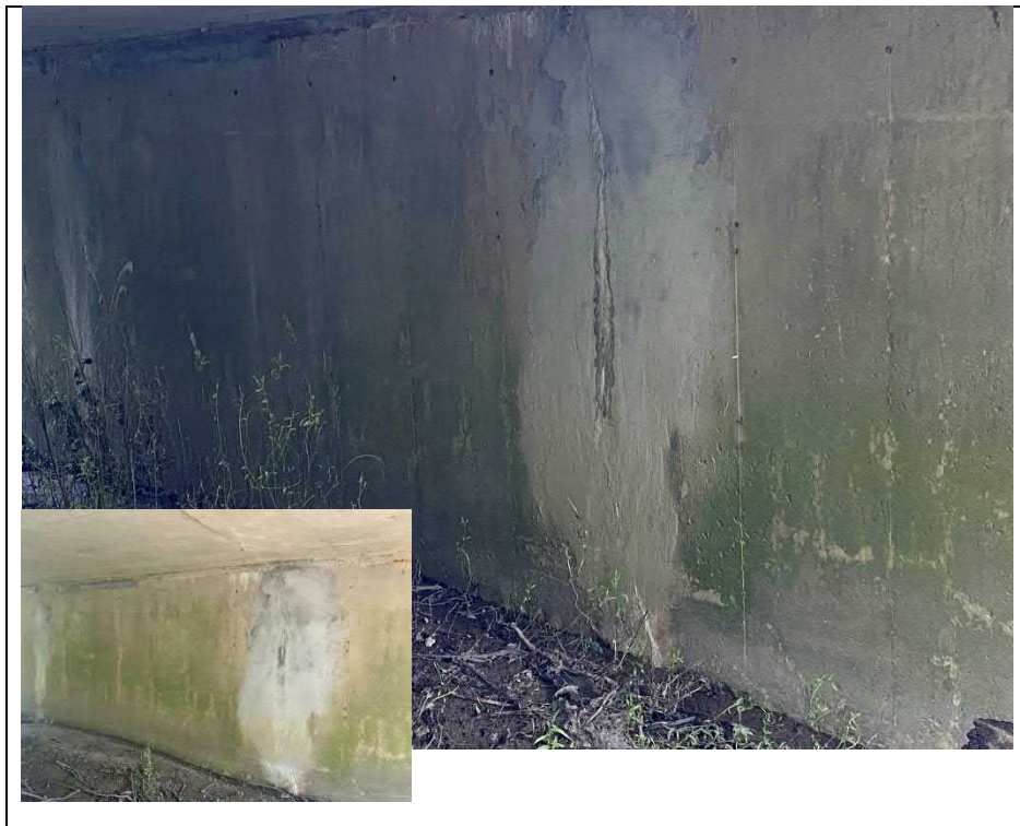
Photograph 8: Crack repairs at north abutment wall
