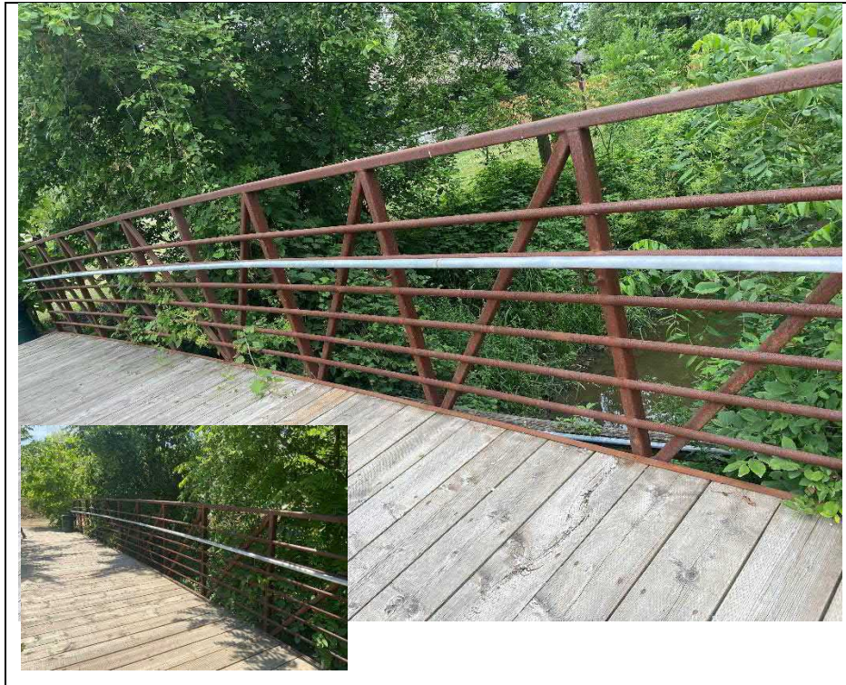
Photograph 7: Top chord, railing system, truss verticals and diagonals (Looking Southwest)
