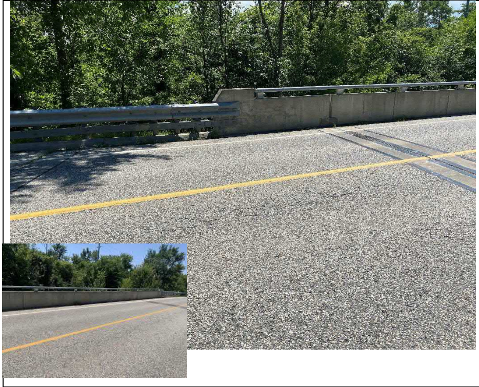
Photograph 3: Typical condition of wearing surface
