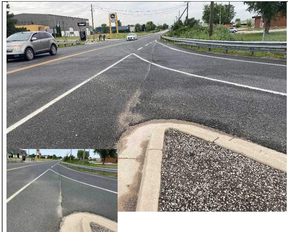
Photograph 6: Pavement joint between the deck and approach wearing surfaces (Looking Northeast)
