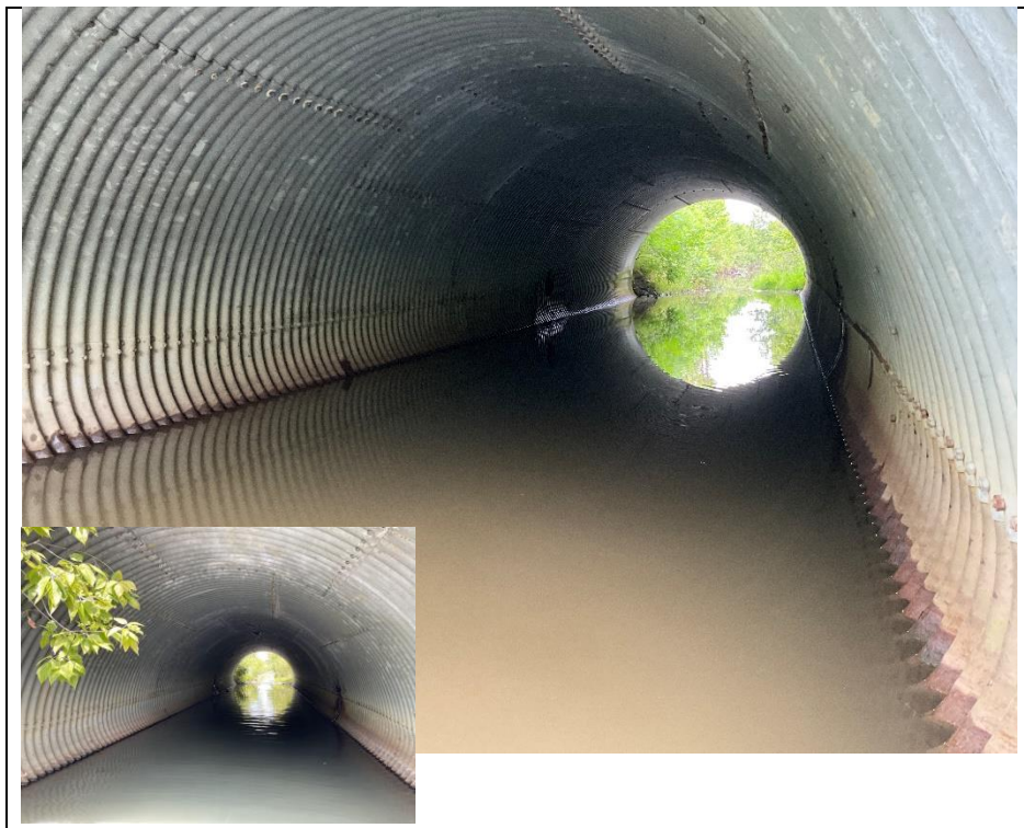
Photograph 10: Typical condition of culvert barrel
