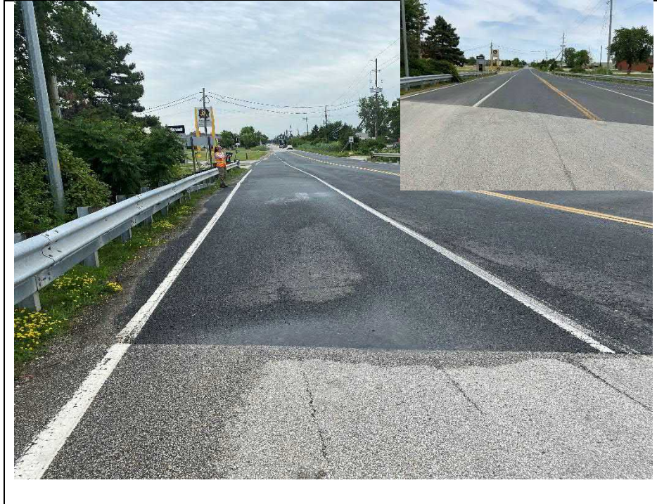
Photograph 5: E.B.L wearing surface (Looking Northeast)
