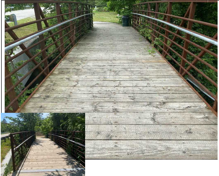
Photograph 5: Top of Deck (Looking South)
