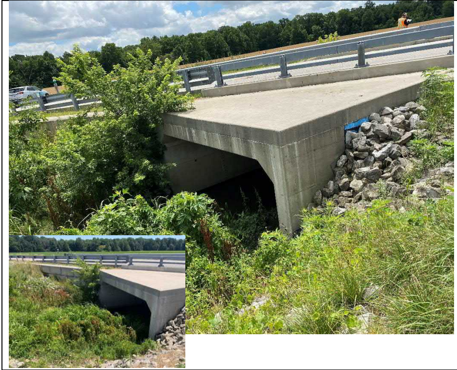
Photograph 15: Embankments and retaining walls at north side of culvert (Looking East)
