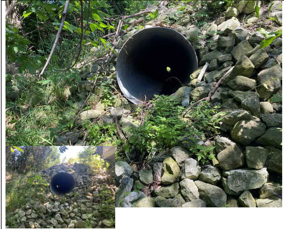
Photograph 15: Embankments at northeast quadrant of structure (Looking East)
