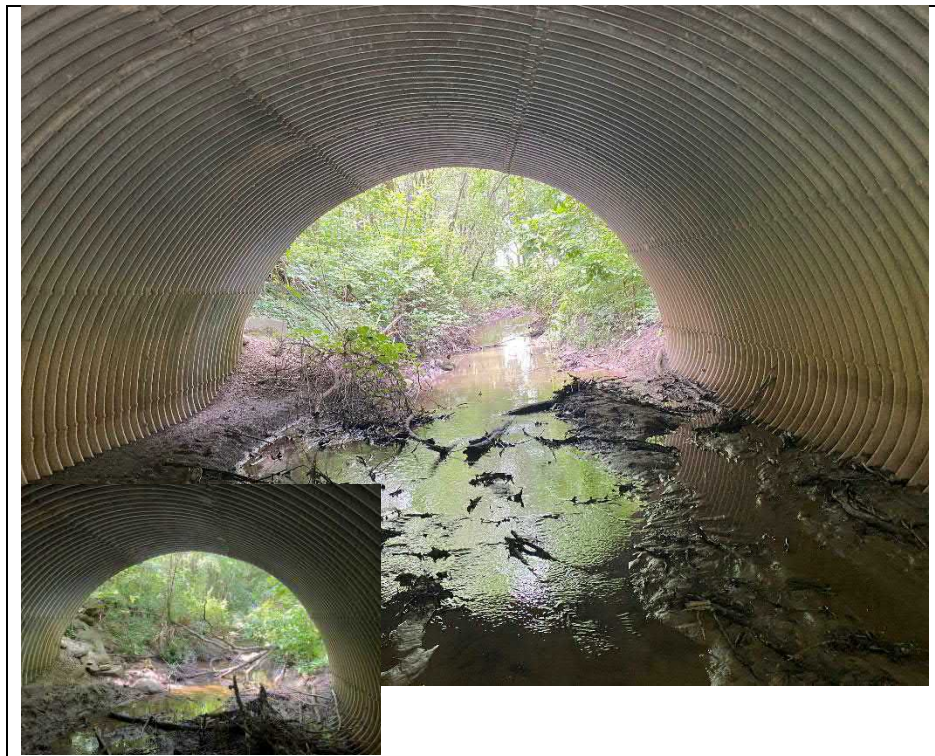
Photograph 6: Culvert barrel (Looking West)
