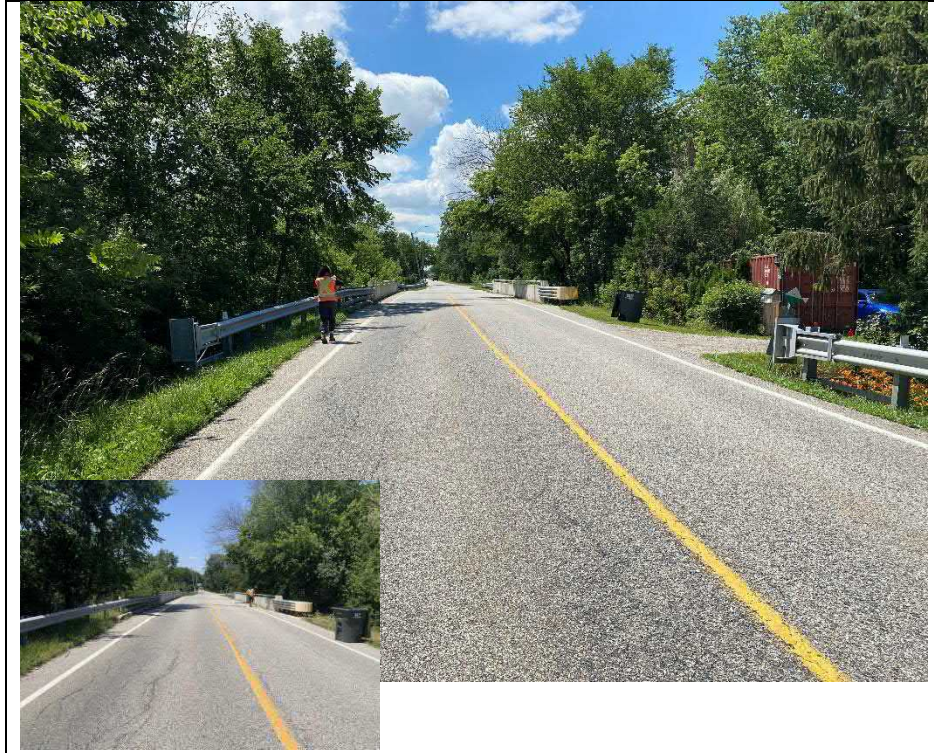
Photograph 1: Overview of structure looking east
