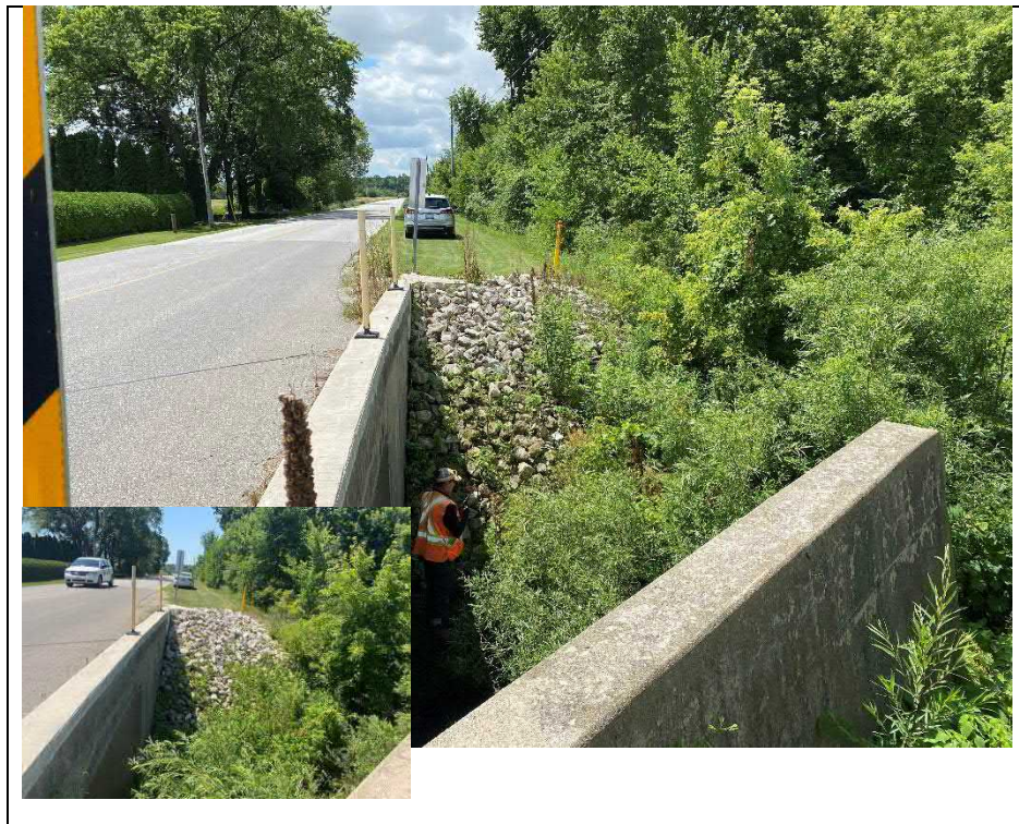
Photograph 12: New precast block retaining wall and slope protection at southwest embankment (Looking South)
