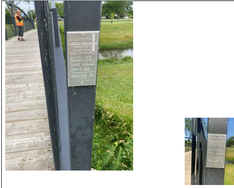
Photograph 15: Bridge ID found at northeast quadrant of structure
