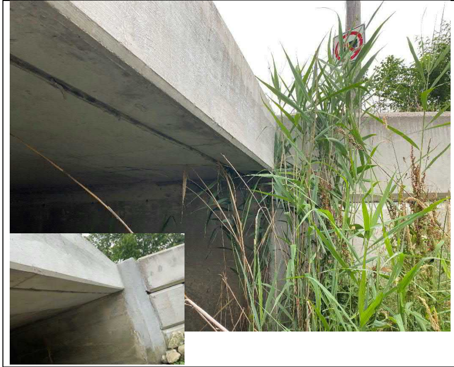
Photograph 7: Typical condition of fascia (west end shown)
