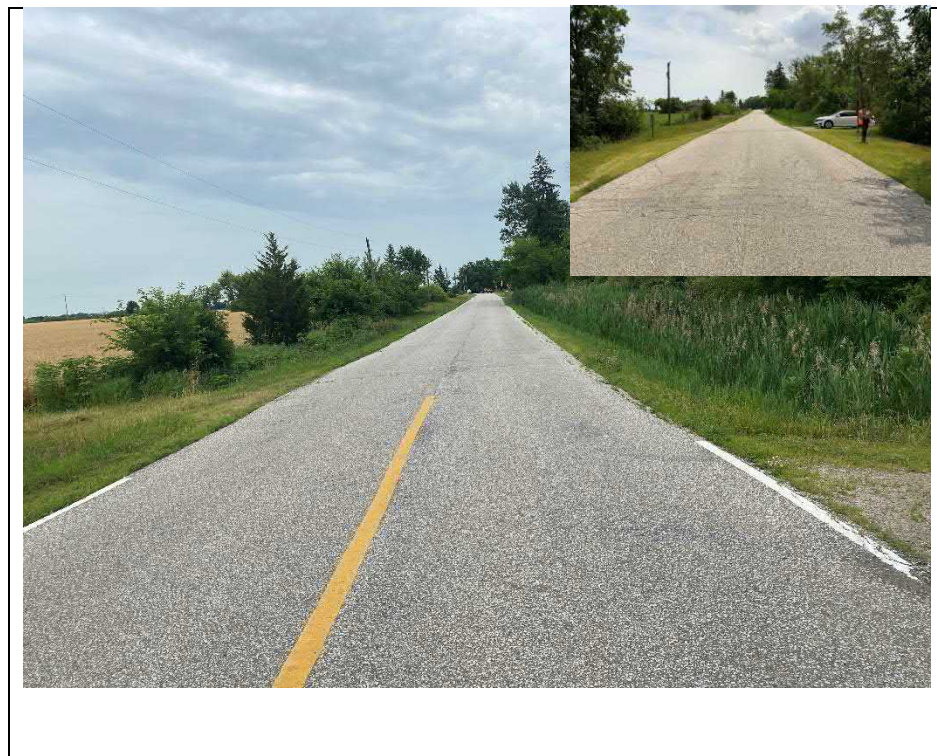
Photograph 2: North approach (Looking South)
