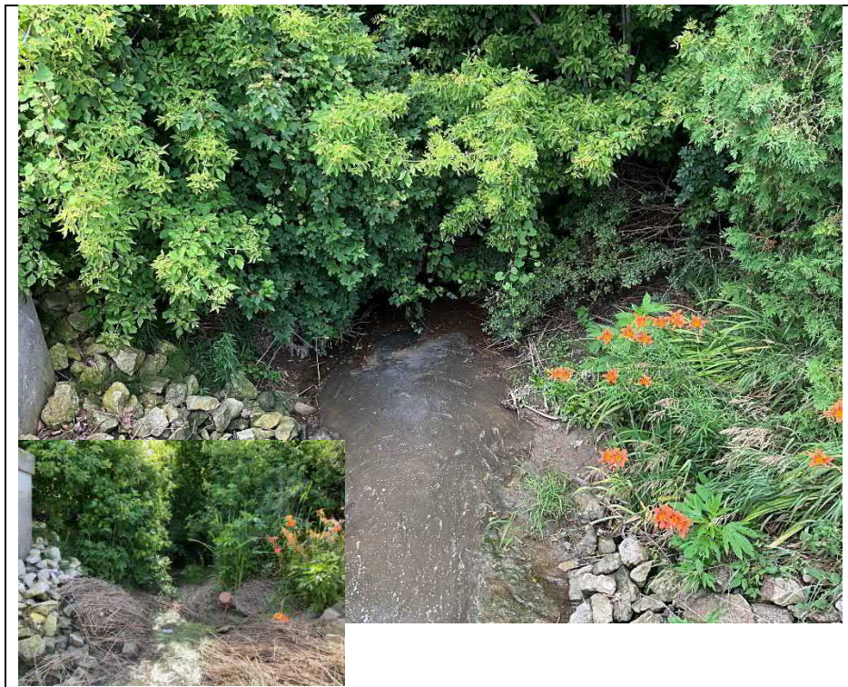
Photograph 14: Watercourse on west side of structure (Looking West)
