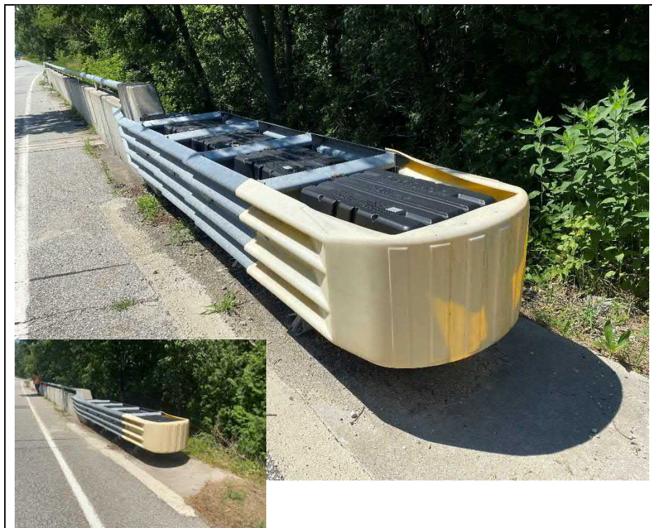
Photograph 6: SBEAT at east approach (Looking West)
