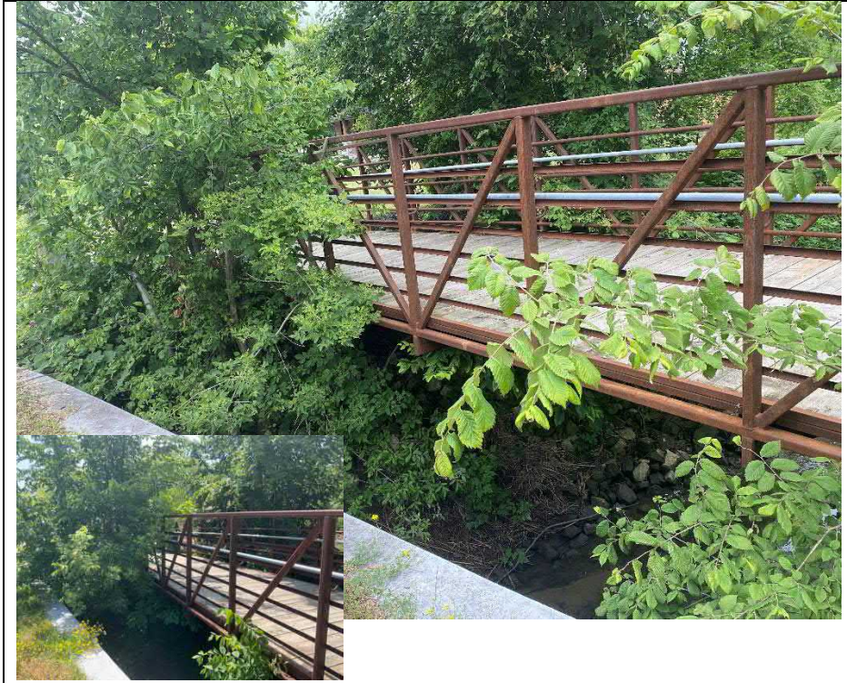
Photograph 1: East elevation of structure (Looking Southwest)
