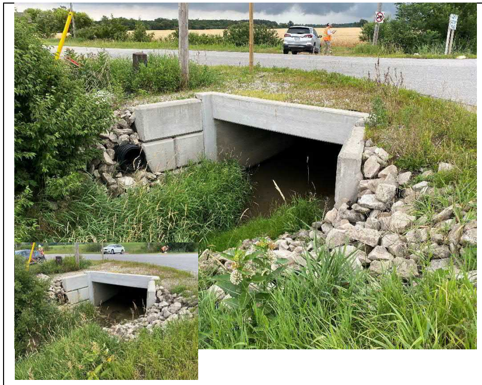
Photograph 4: West elevation (Looking Northeast)
