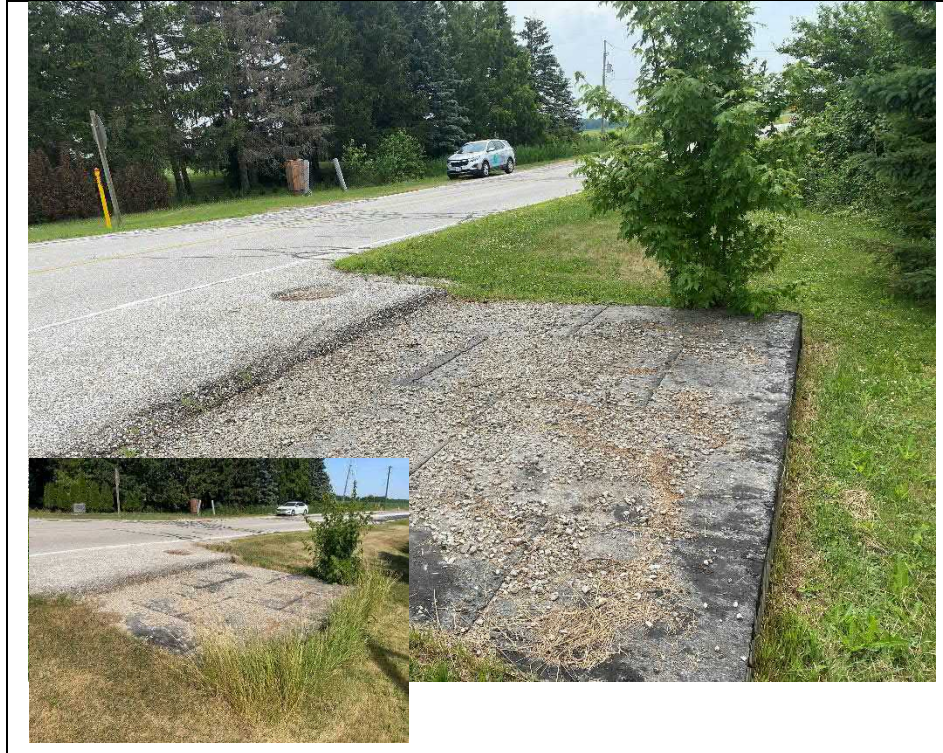
Photograph 5: Southern closed end of structure with exposed waterproofing (Looking North)
