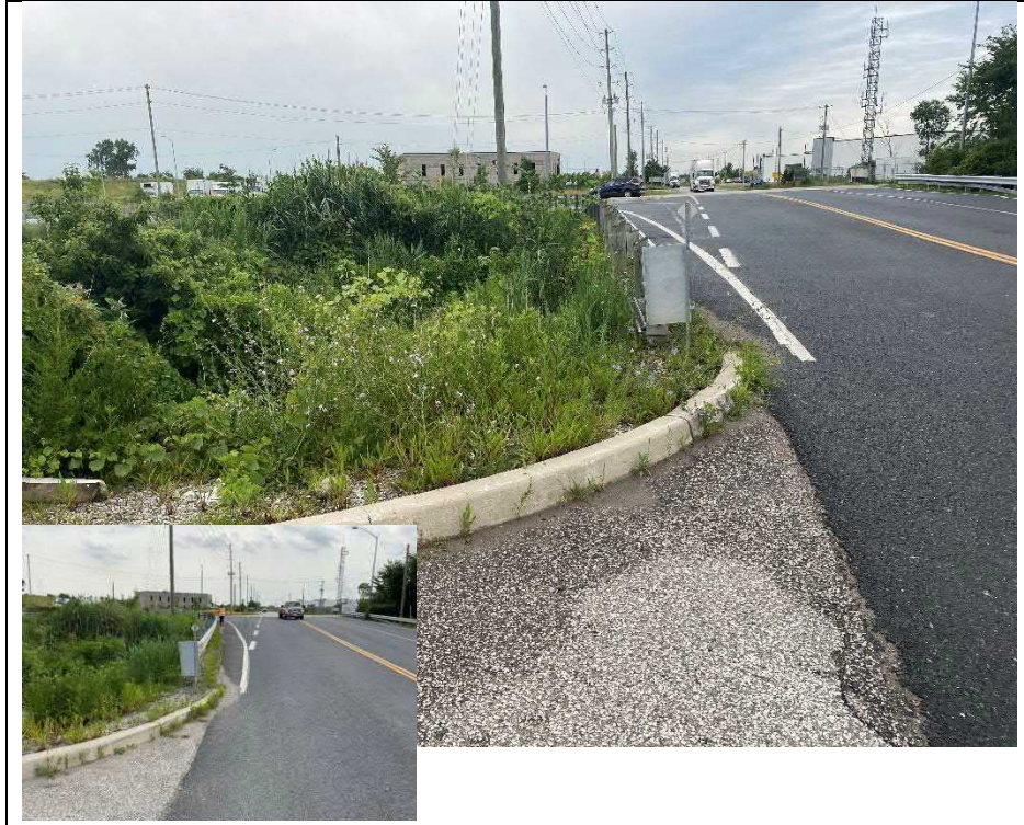
Photograph 1: South Approach (Looking Southwest)
