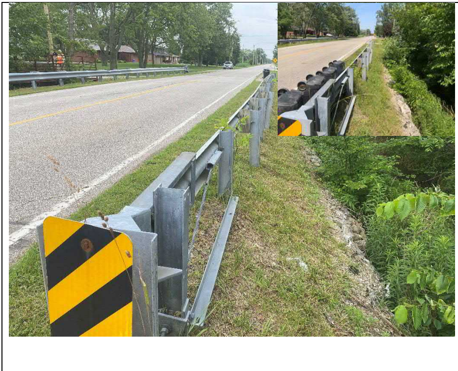
Photograph 4: Guide rail end treatment at the southeast quadrant of structure
