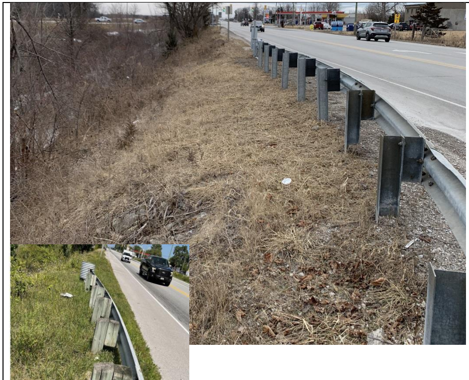
Photograph 6: New guide rail section at the northeast end
