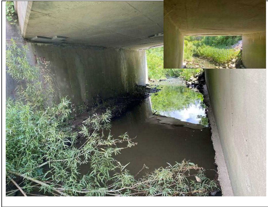
Photograph 13: Waterway, looking west from inside the structure
