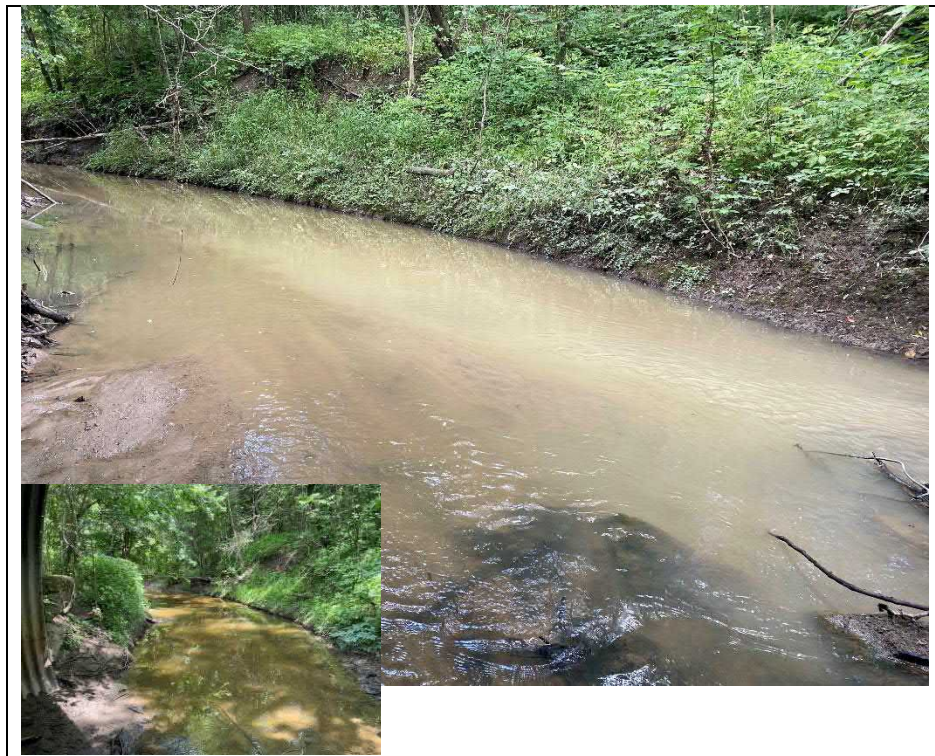
Photograph 12: Watercourse outlet at west end of structure (Looking Northwest)
