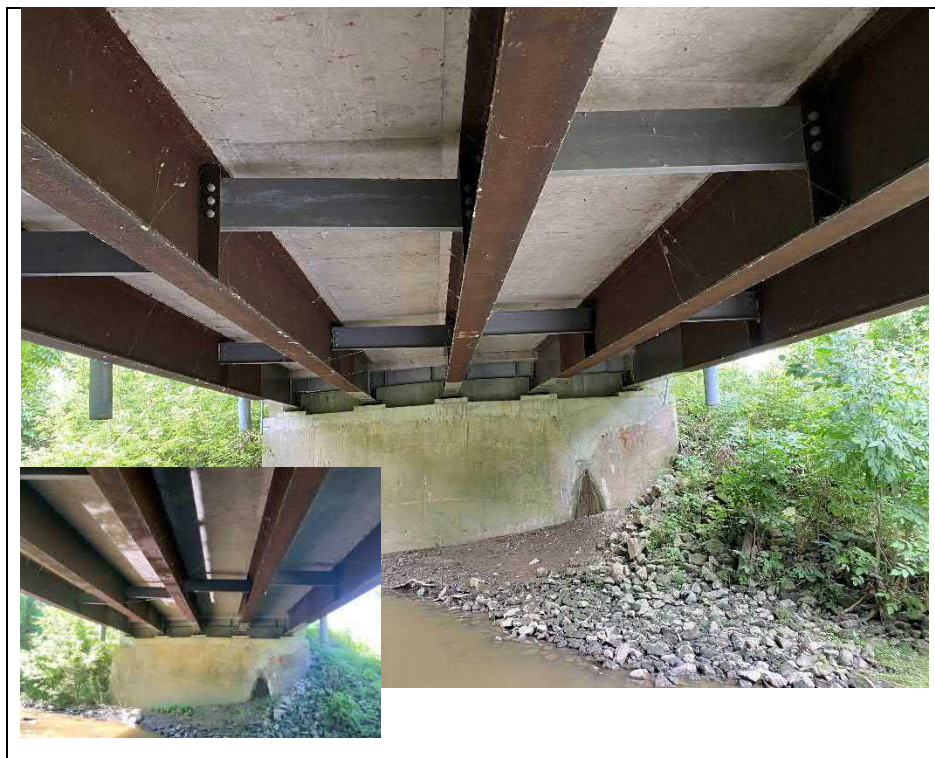
Photograph 16: Deck soffit, steel girders, and diaphragms (Looking South)
