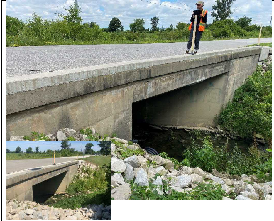
Photograph 5: East elevation of structure
