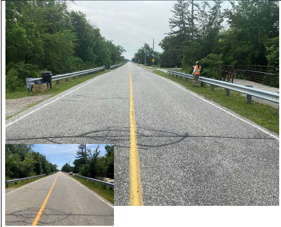
Photograph 1: North approach (Looking south)
