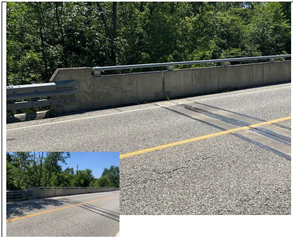
Photograph 4: Typical condition of parapet wall (Looking West)
