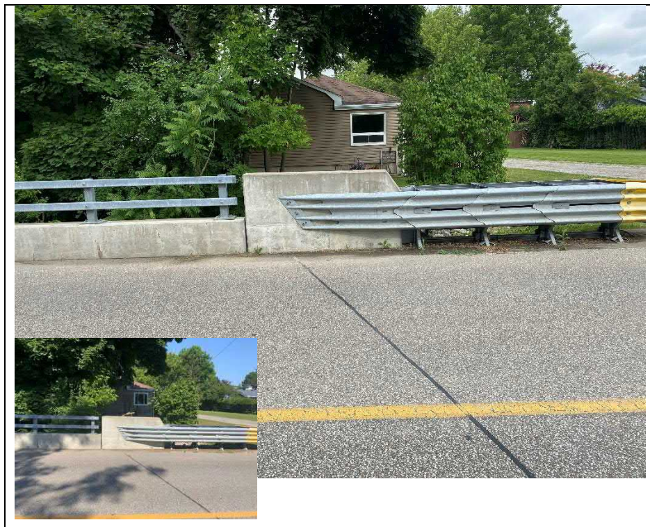
Photograph 6: Concrete barrier wall at the northwest quadrant of the structure
