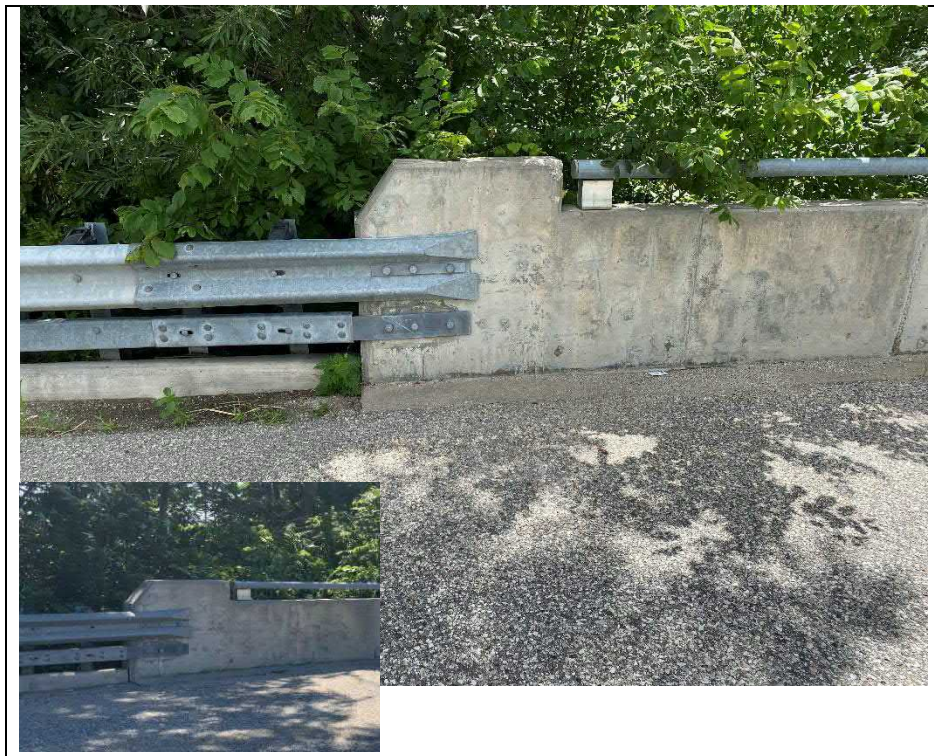
Photograph 10: Typical condition of parapet end walls
