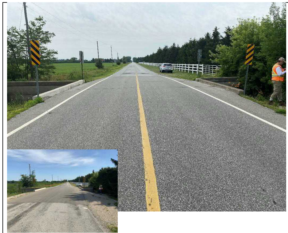
Photograph 2: North approach (Looking South)
