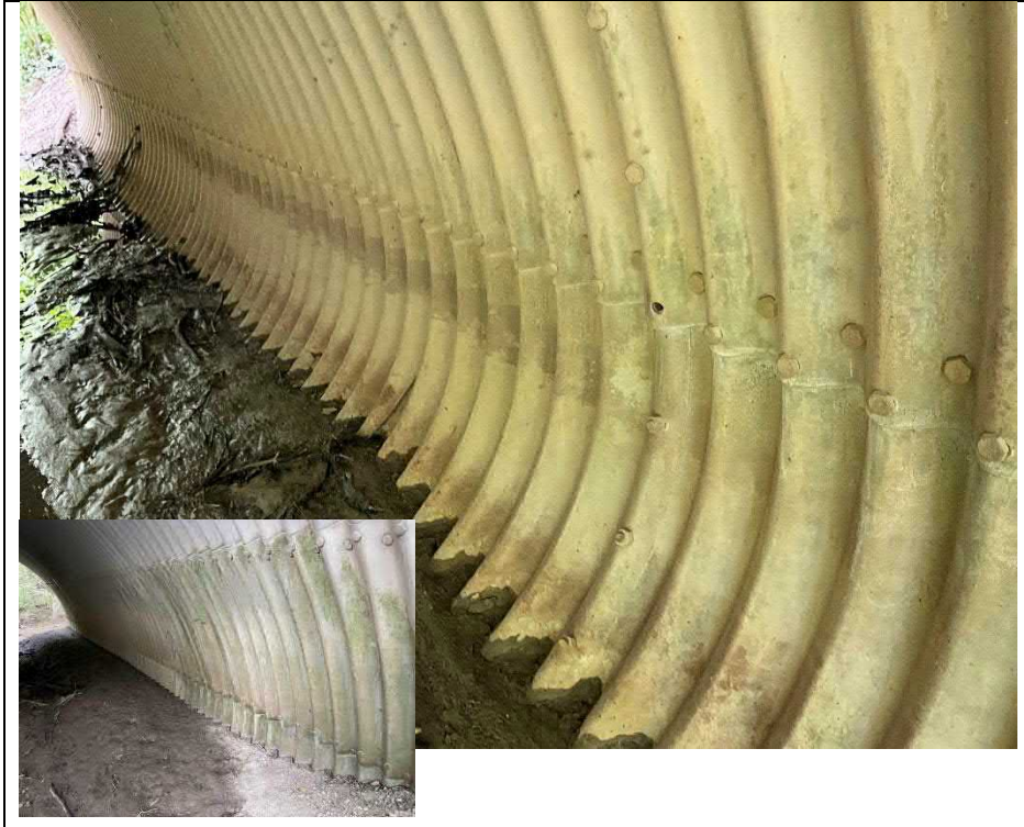
Photograph 7: Typical condition along spring line
