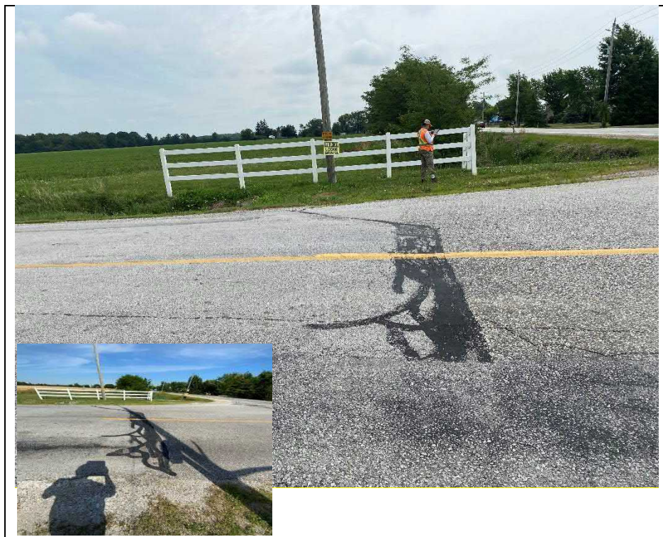
Photograph 2: Wearing surface at south approach (Looking East)
