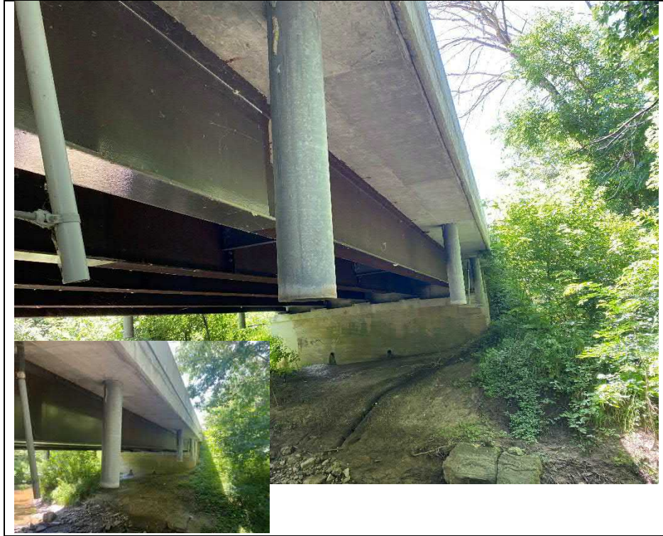
Photograph 11: Deck soffit, main girders, diaphragms, and deck drainage (Looking West)
