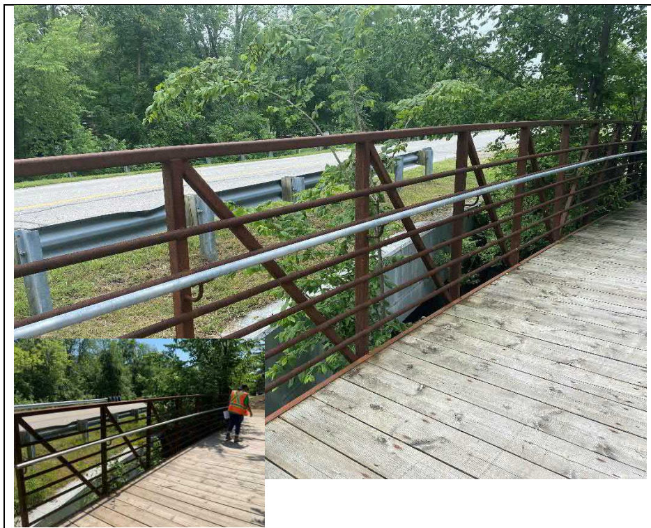
Photograph 6: Top chord, railing system, truss verticals and diagonals (Looking Southeast)
