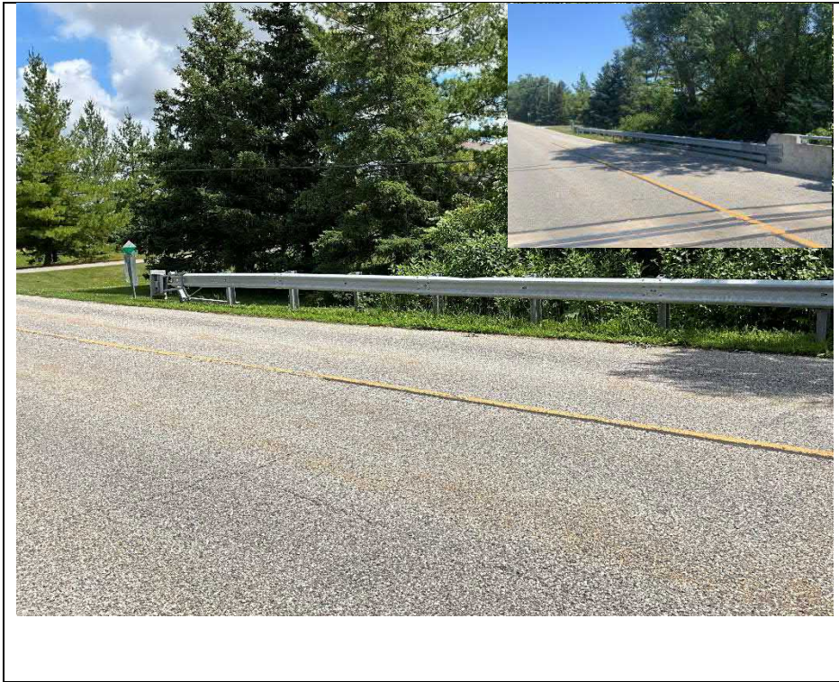
Photograph 5: Wearing surface at the north approach (Looking North)
