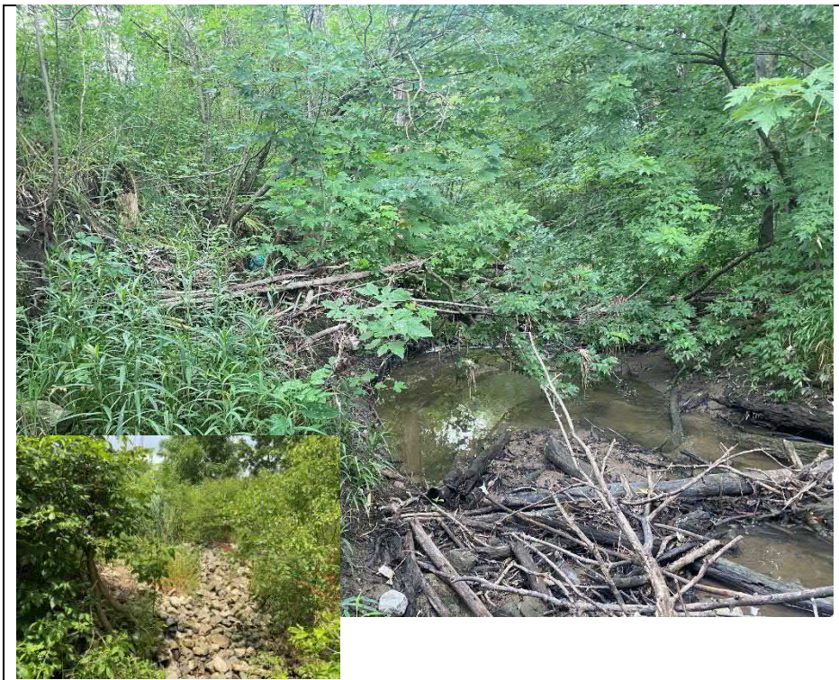
Photograph 12: Watercourse on east side of structure (Looking East)
