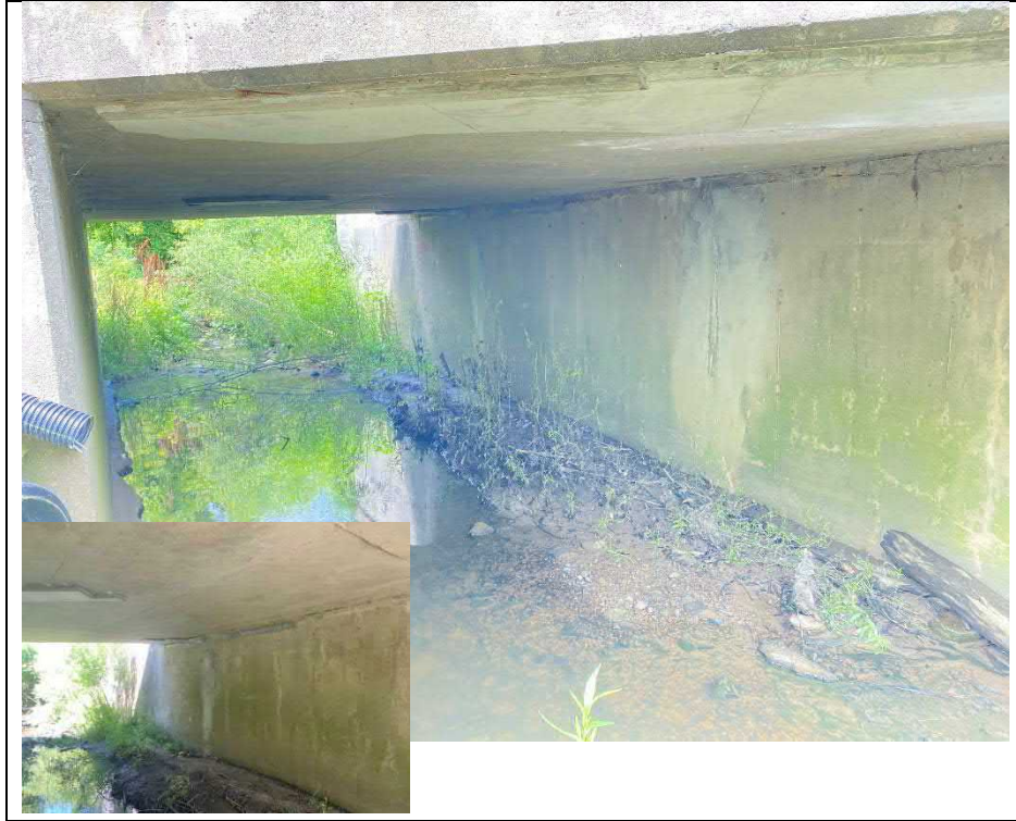
Photograph 7: Concrete soffit patch at west end of soffit
