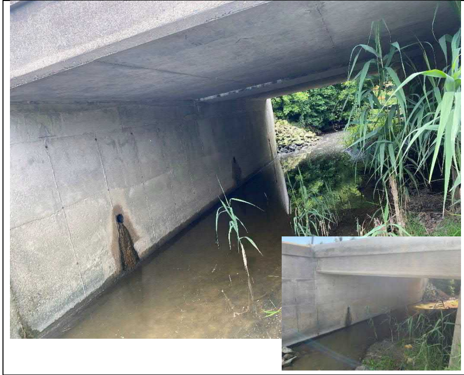
Photograph 9: South abutment wall and wall drains
