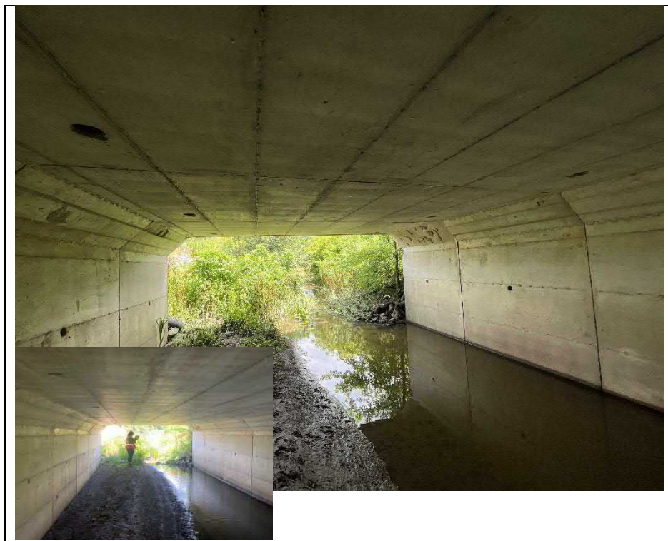
Photograph 10: Typical condition of culvert barrel (Looking North)
