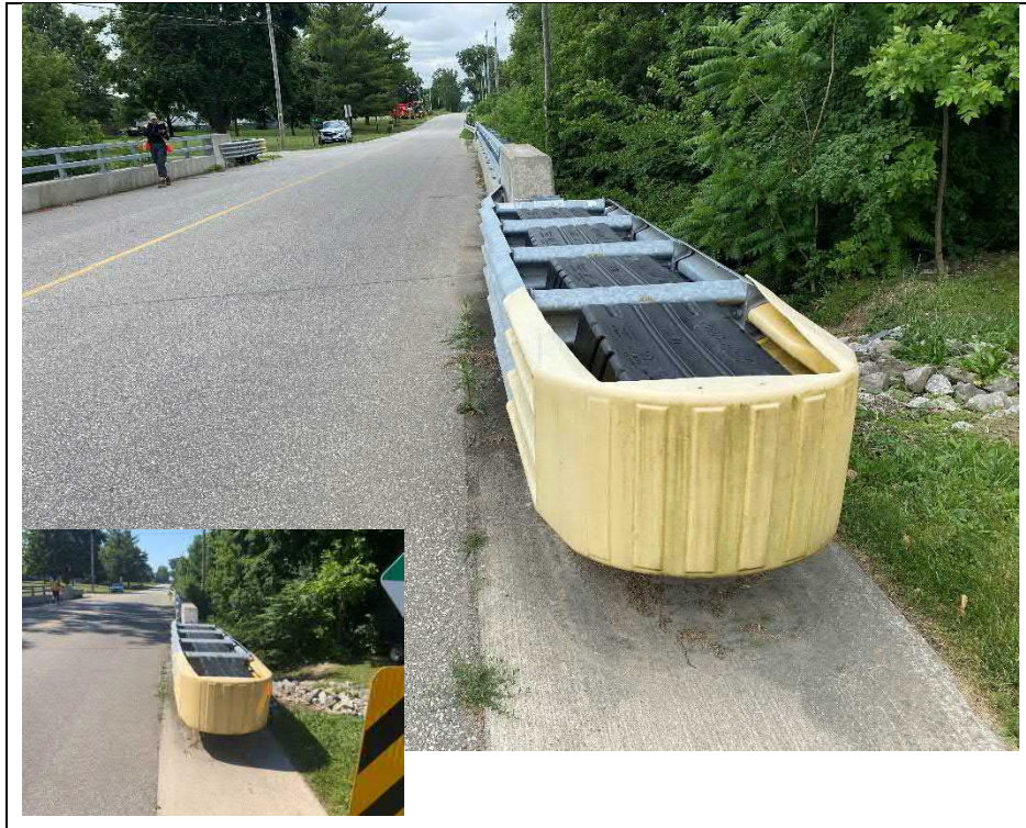
Photograph 5: End treatment at the northwest quadrant of the structure
