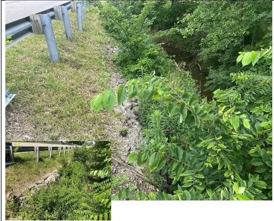
Photograph 11: Embankments, retaining elements on west side of structure (Looking North)
