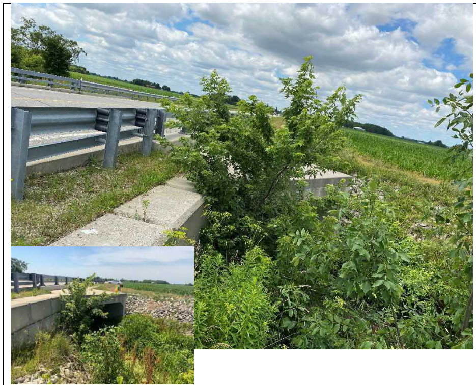
Photograph 16: Embankments and retaining walls at north side of culvert (Looking West)
