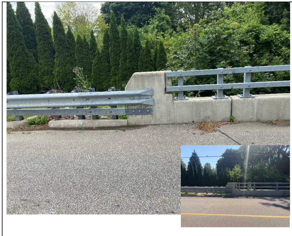
Photograph 4: Expansion joint between the deck and the north approach (Looking East)
