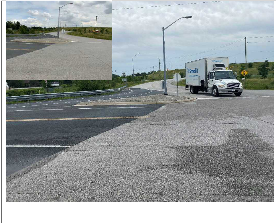
Photograph 3: South approach (Looking East)
