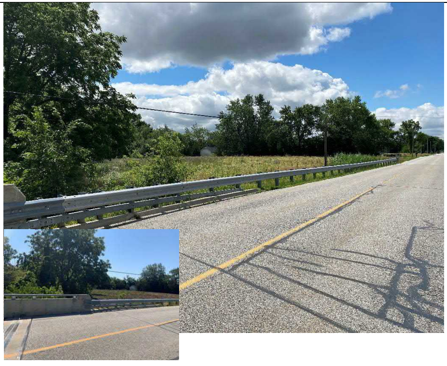
Photograph 4: Wearing surface at the south approach (Looking East)
