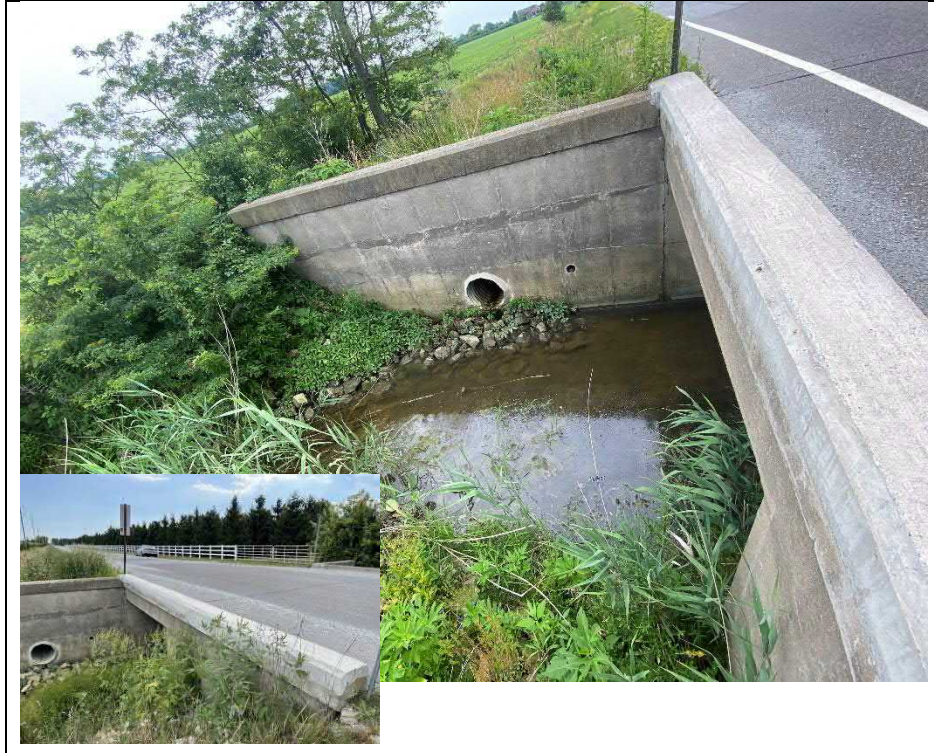
Photograph 5: Reconstructed curb on east side of structure
