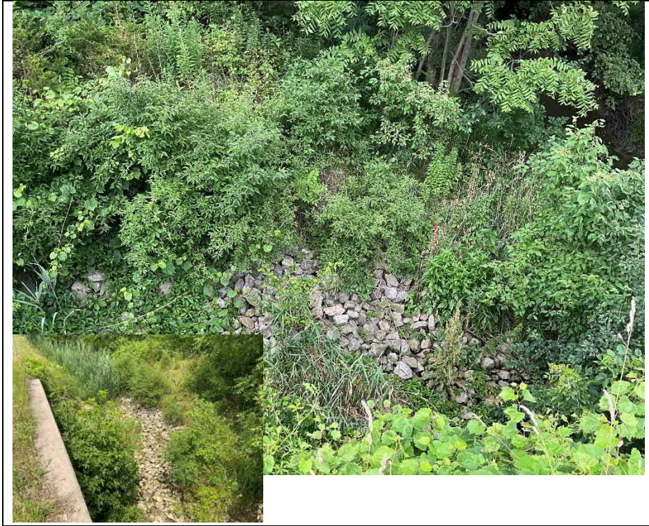
Photograph 13: North-east embankment (Looking North)
