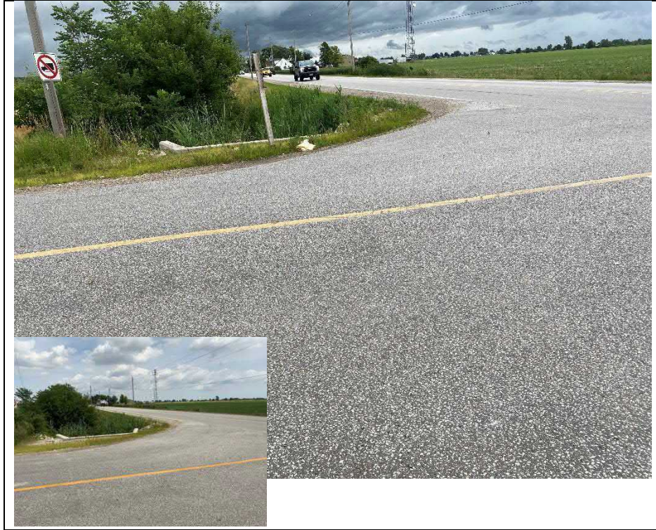
Photograph 3: Wearing surface over the structure (Looking East)
