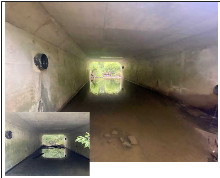
Photograph 8: Typical condition of culvert barrel
