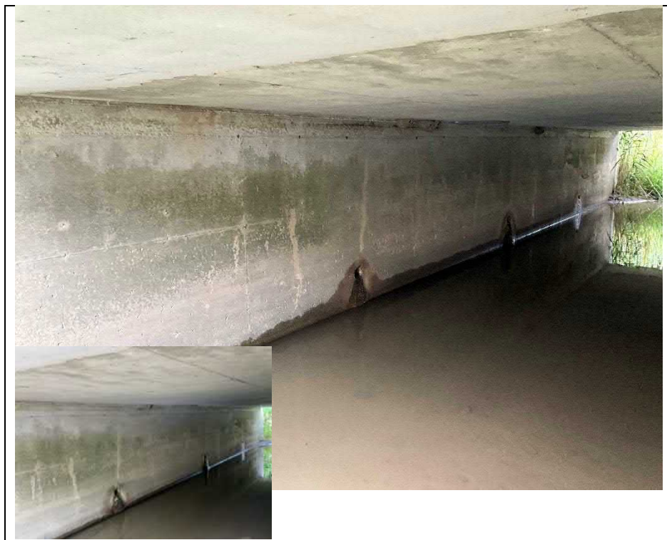
Photograph 10: Concrete patch in soffit near north abutment
