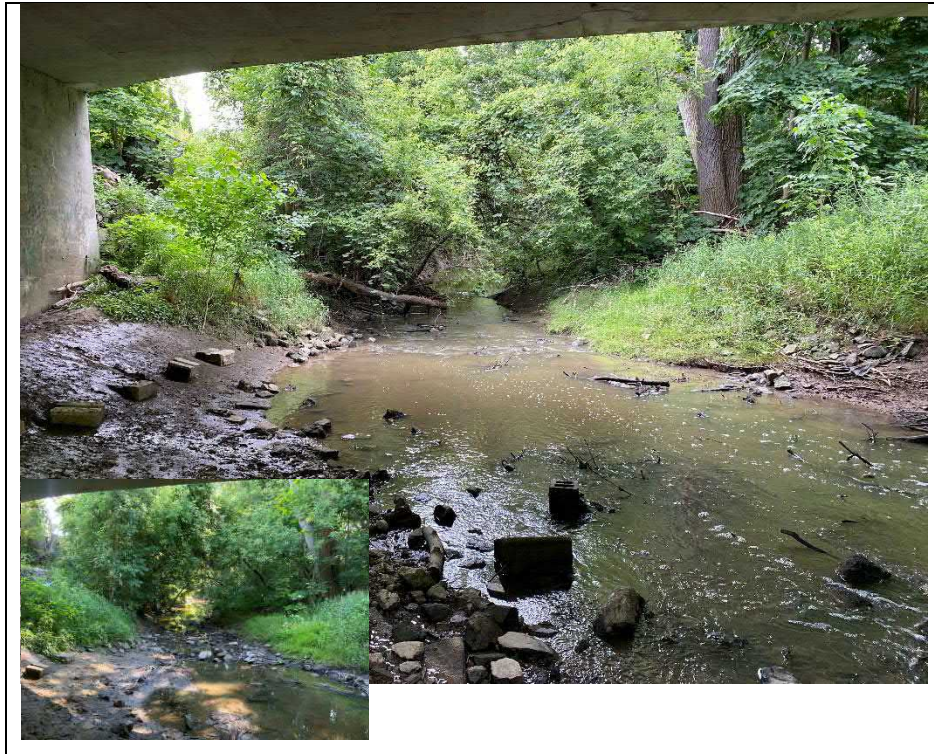
Photograph 23: Waterway, looking east from under the structure
