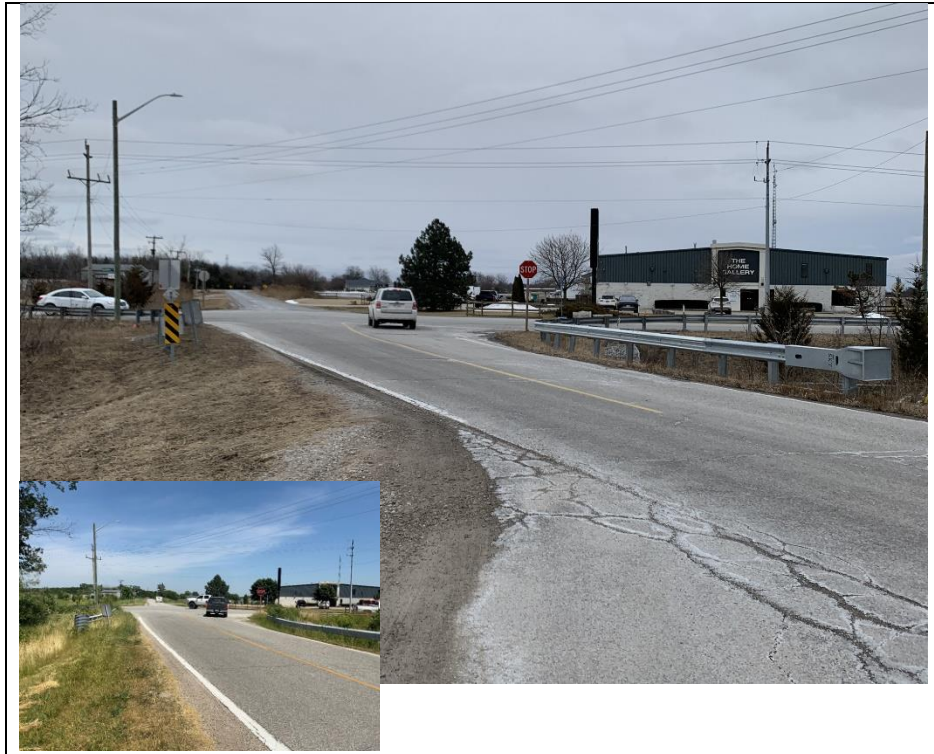
Photograph 1: West Approach (Looking East)
