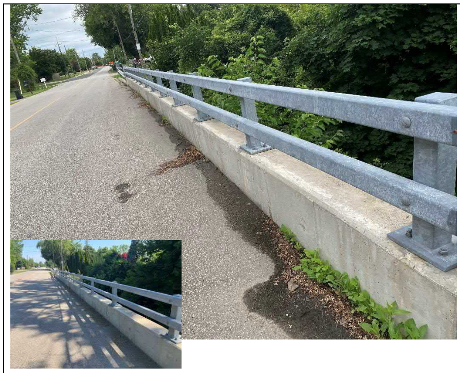
Photograph 10: Parapet wall on the east side of the structure
