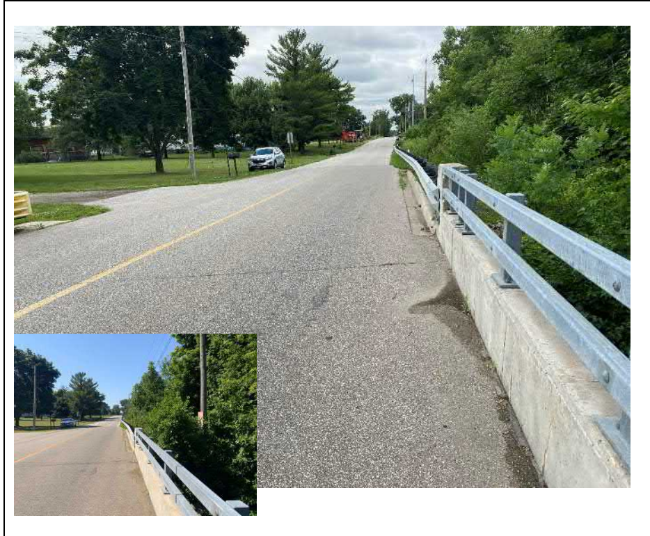
Photograph 3: North approach (Looking North)
