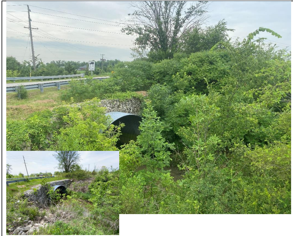
Photograph 15: North embankments with gabion basket retaining walls at north (Looking South)
