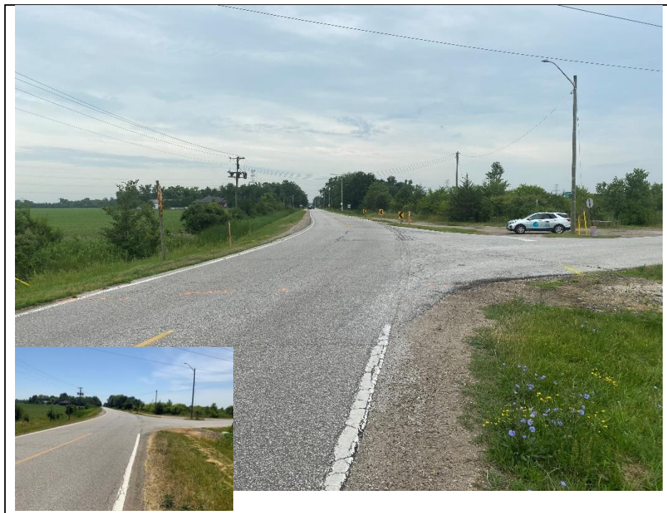
Photograph 4: Wearing surface at west approach
