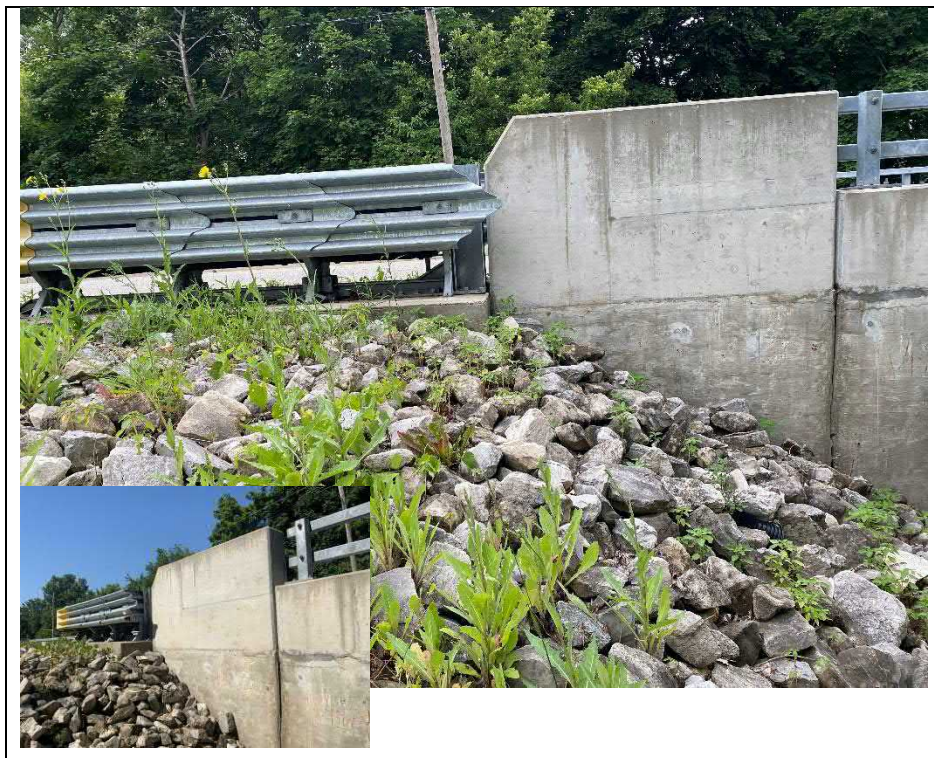
Photograph 20: Typical condition of wingwalls (Southeast quadrant shown)
