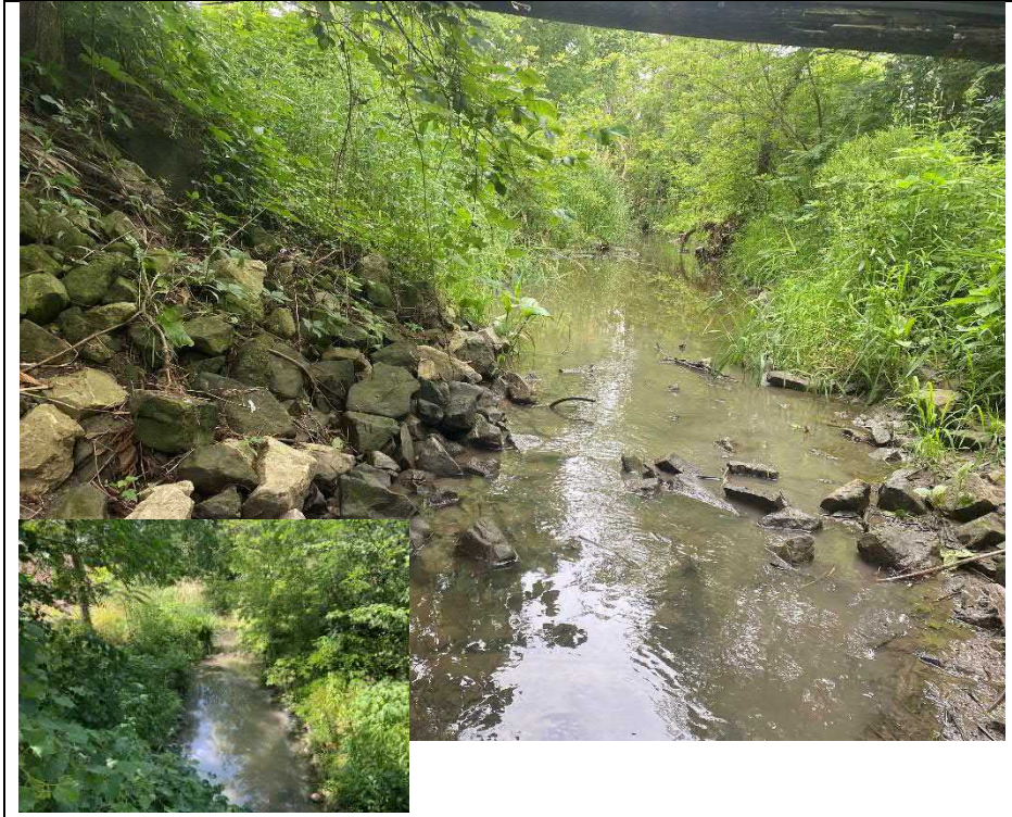
Photograph 15: Waterway at the west outlet (Looking West)
