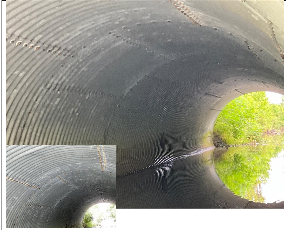
Photograph 11: Typical condition of culvert barrel soffit
