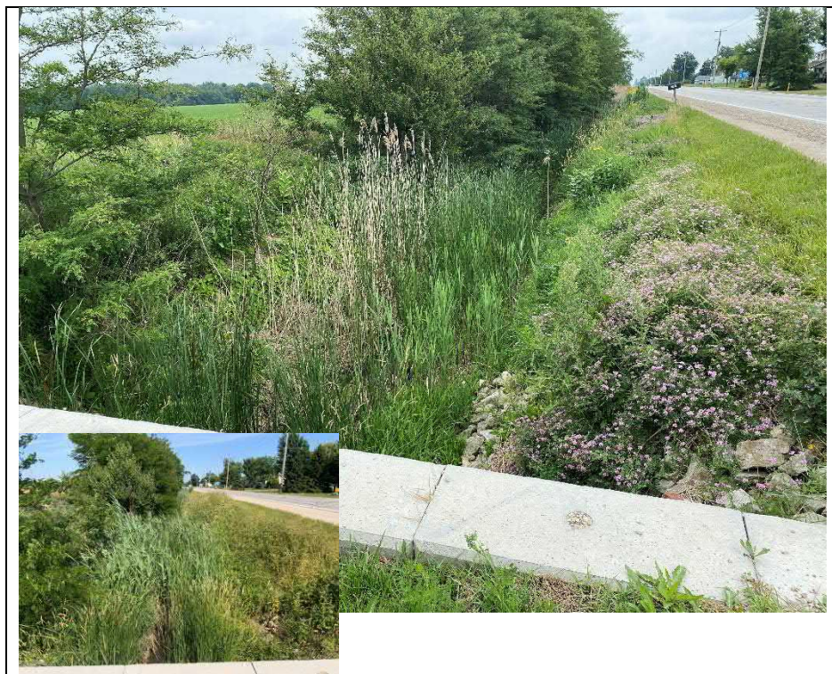
Photograph 10: Waterway, embankments and vegetation (Looking East)
