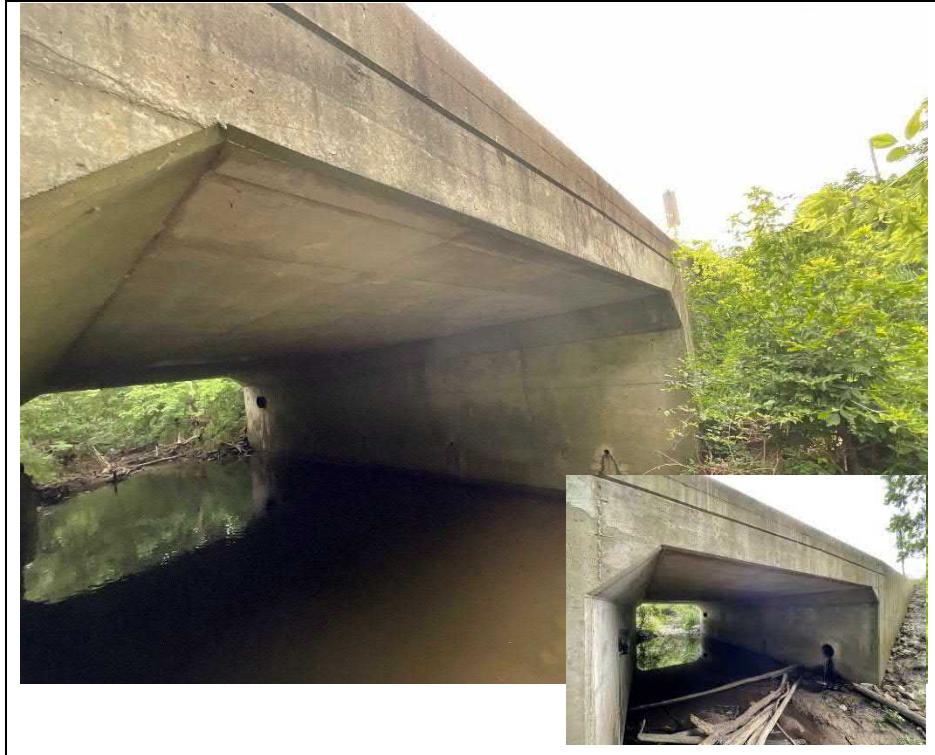
Photograph 7: West elevation (Looking East)
