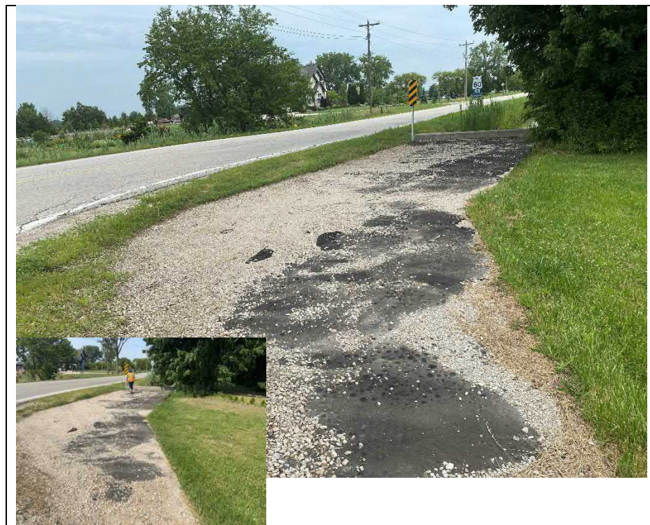
Photograph 6: Exposed waterproofing on the top of deck showing signs of bubbling and deterioration in areas not covered by granular material (Looking North)
