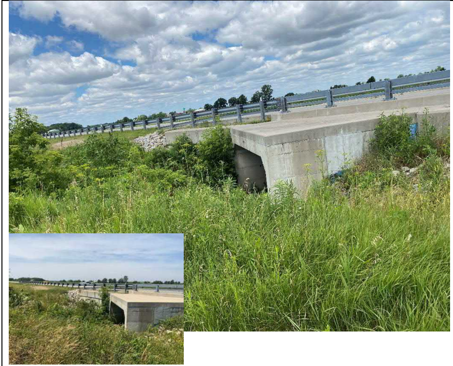
Photograph 17: Embankments and retaining walls at south side of culvert (Looking West)
