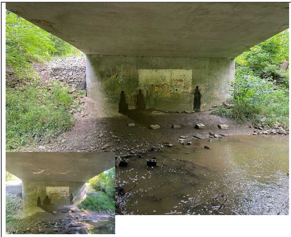
Photograph 14: North abutment wall
