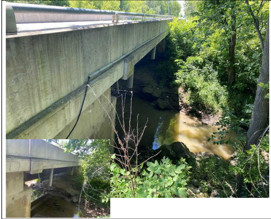
Photograph 9: North elevation of structure
