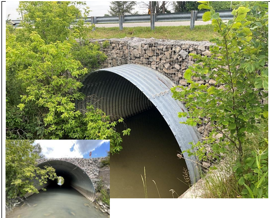
Photograph 8: North elevation and gabion headwalls
