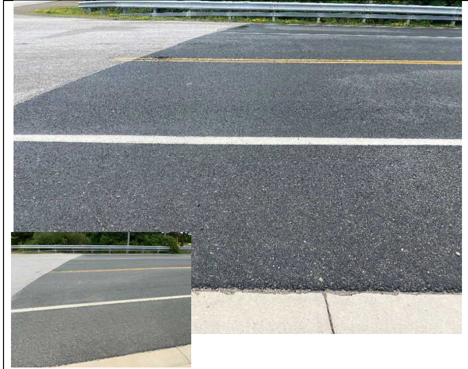
Photograph 7: Wearing surface over the structure (Looking Northwest)
