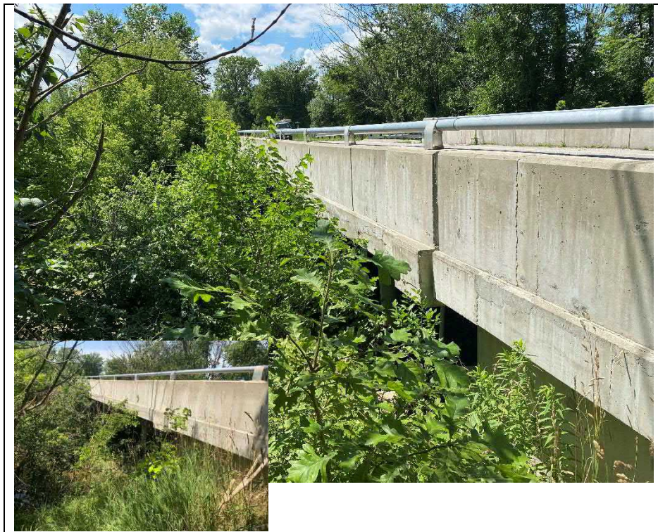
Photograph 10: South elevation of structure
