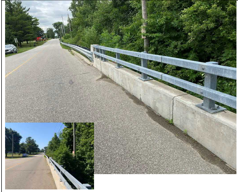
Photograph 7: Guide rail at the south approach
