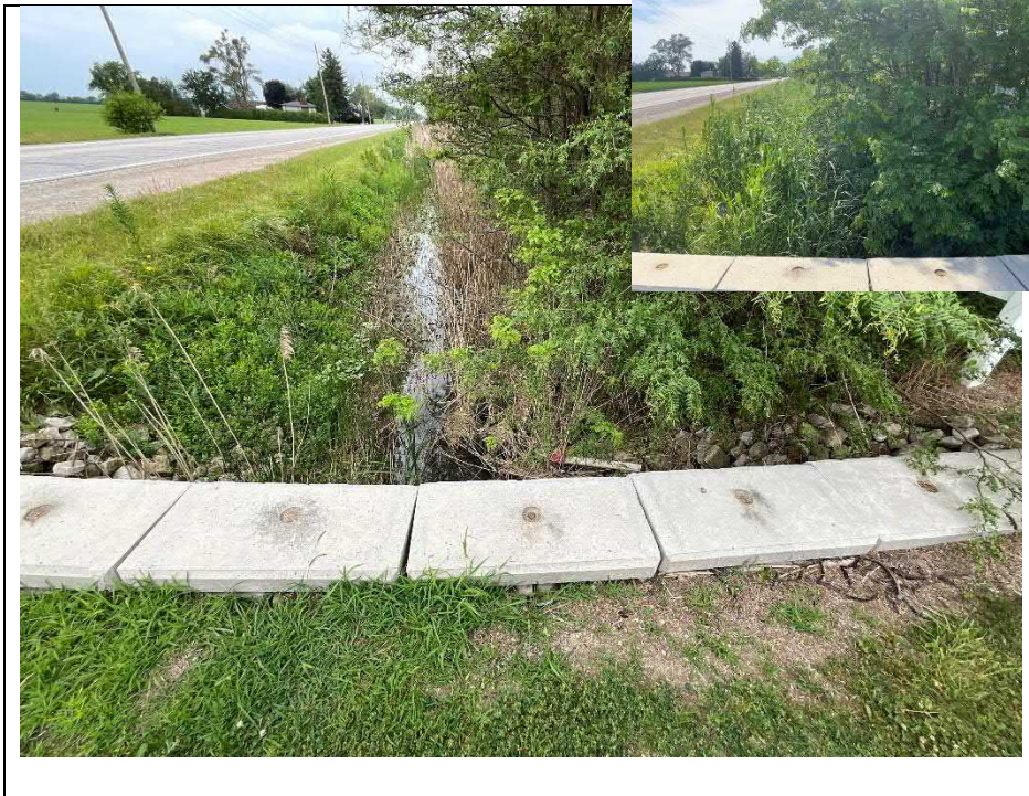
Photograph 11: Waterway, embankments and vegetation (Looking West)
