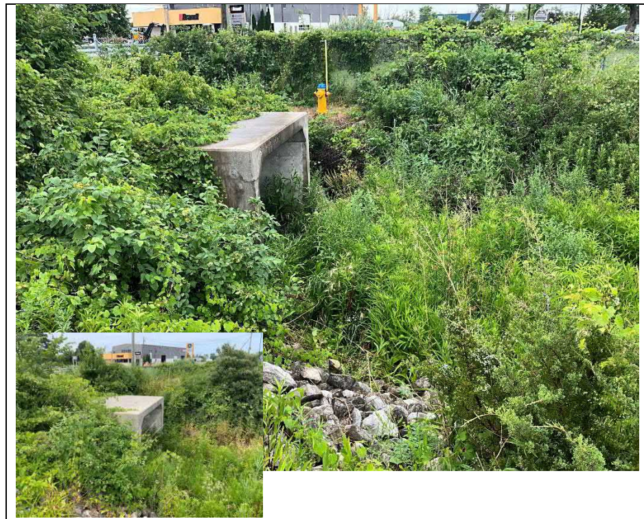
Photograph 10: East elevation (Looking North)
