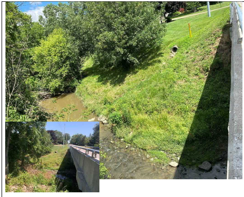
Photograph 22: Embankments and waterway at northwest quadrant of structure
