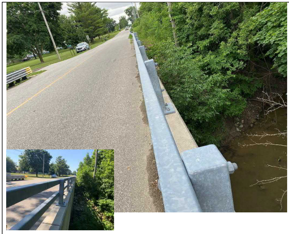
Photograph 22: Embankment at southwest quadrant of the structure
