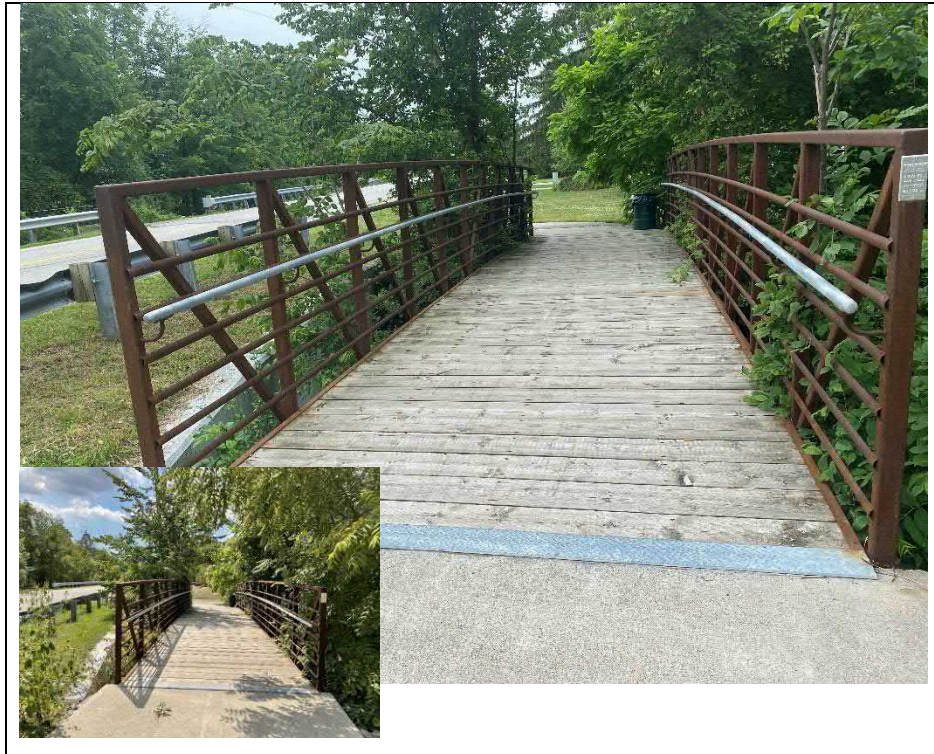
Photograph 3: North approach (Looking South)
