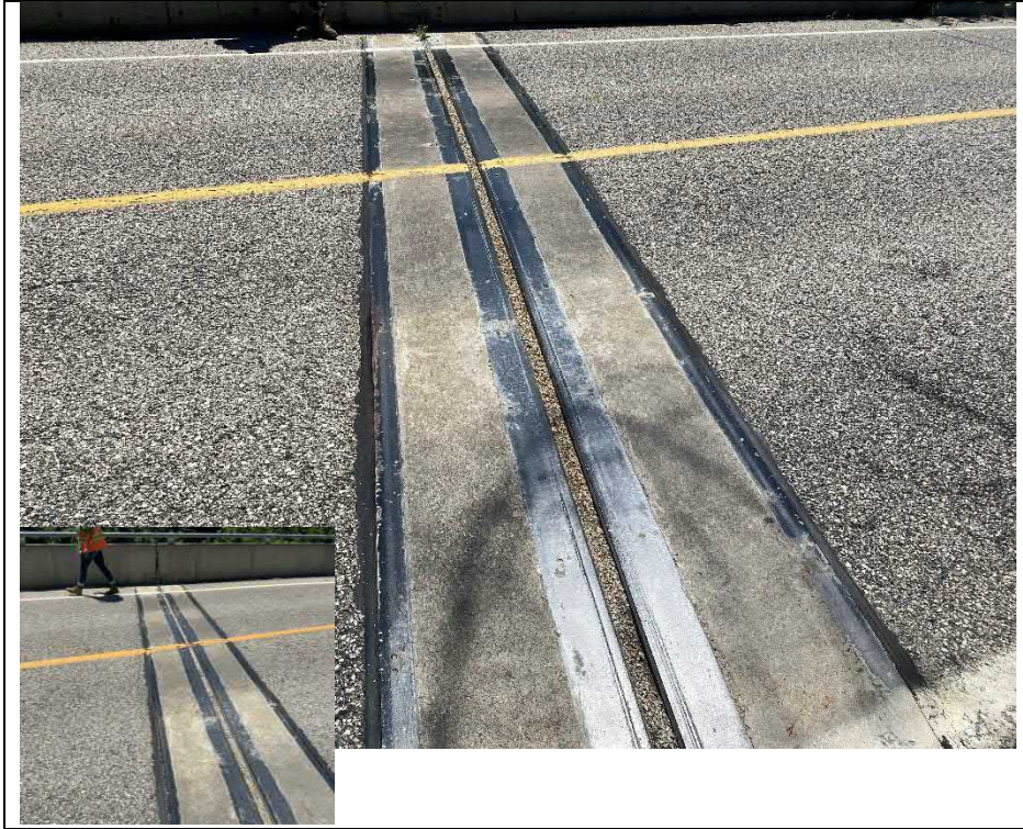
Photograph 7: Expansion joint at east side of the structure (Looking South)
