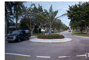
Traffic circle Horizontal deflection; Raised islands placed in the middle of intersections to force traffic to travel around
