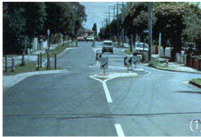
Chicane Horizontal deflection; A series of curb extensions alternating between sides of the street to create S-shaped curves
