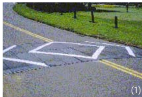
Speed hump Vertical deflection; Rounded raised areas of pavement, often placed in a series several metres apart
