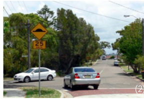
Speed table Vertical deflection; Speed humps with a flat section in the middle and ramps on either side
