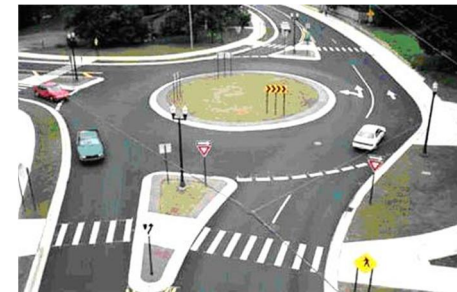
Figure E9: Roundabout with Pedestrian Crossing
