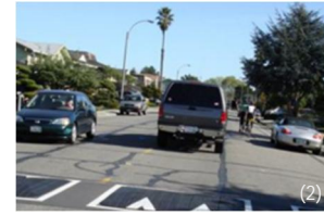
Speed cushion Vertical deflection; Speed humps with wheel cutouts to allow emergency and transit vehicles to travel over them unaffected
