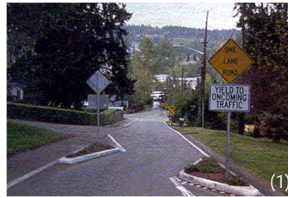
Mid-block narrowings Horizontal deflection; Curb extensions at mid-block locations
