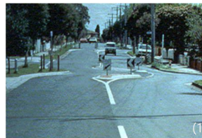
Chicane Horizontal deflection; A series of curb extensions alternating between sides of the street to create S-shaped curves
