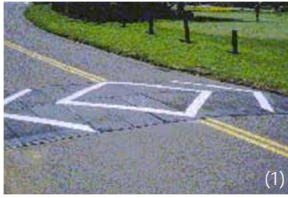
Speed hump Vertical deflection; Rounded raised areas of pavement, often placed in a series several metres apart
