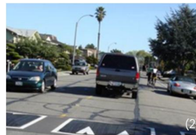
Speed cushion Vertical deflection; Speed humps with wheel cutouts to allow emergency and transit vehicles to travel over them unaffected
