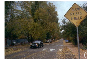
Raised pedestrian crosswalk Vertical deflection; Speed humps with a flat section in the middle, designated as a pedestrian crosswalk
