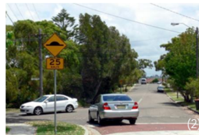
Speed table Vertical deflection; Speed humps with a flat section in the middle and ramps on either side
