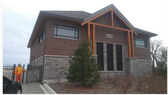
New or improved pump stations
