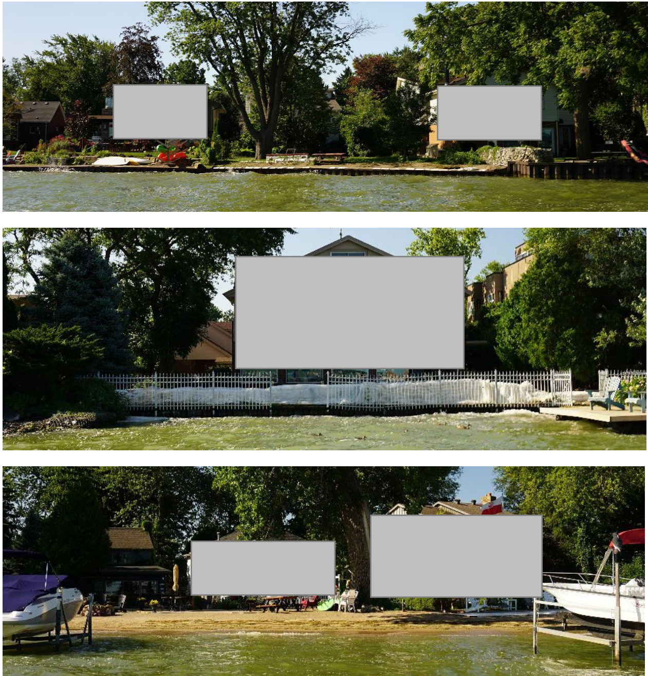
Figure 2.20 Low-crested Steel Sheet Pile Wall (top), Sandbags on Low-crested Wall (middle), and Low-crested Beach Shoreline (bottom)
