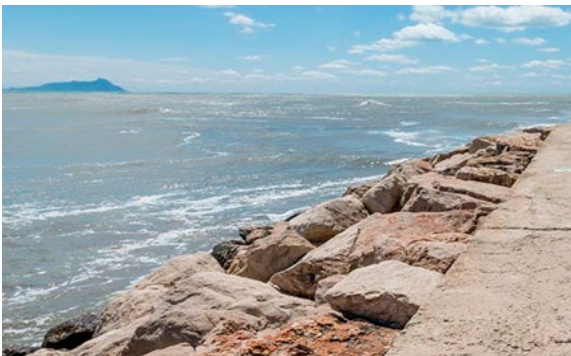
Rock toe protection for existing seawall.
