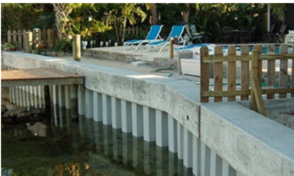
Concrete cap on steel sheet pile wall.
