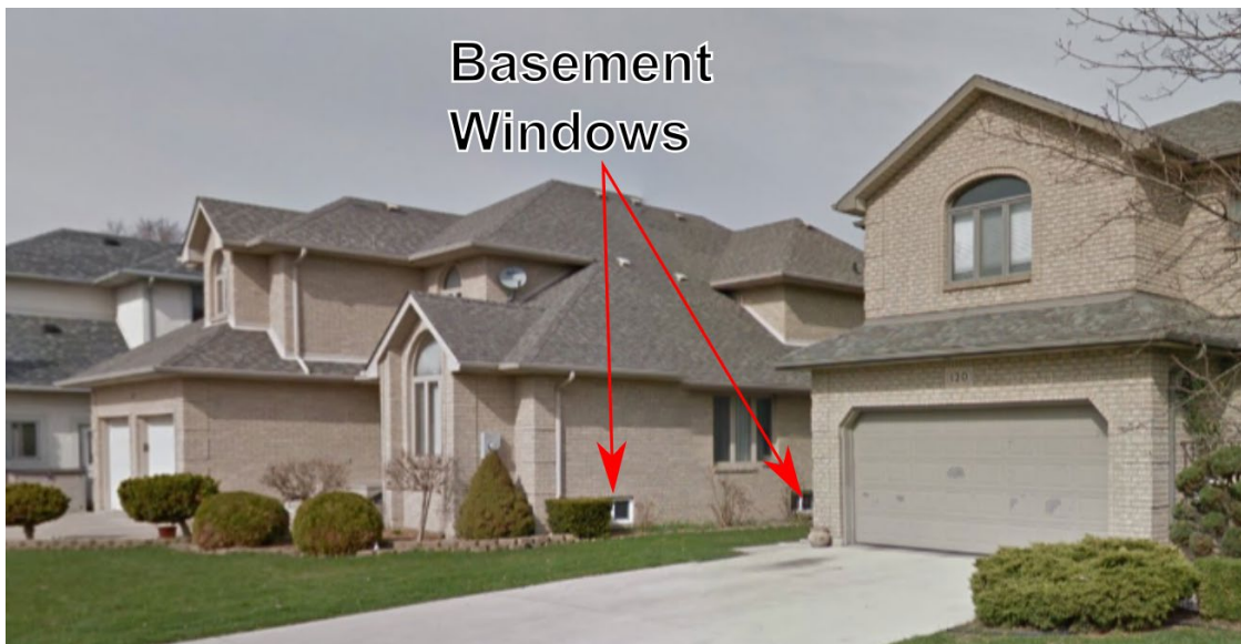
Figure 2.7 Basement Windows below the First Floor
