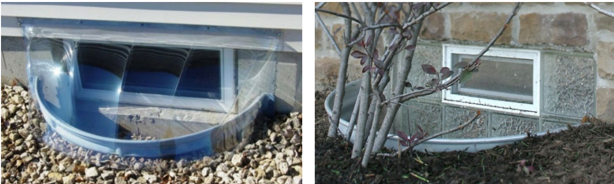
Figure 5.8 Water Shield and Solid Block Basement Window
