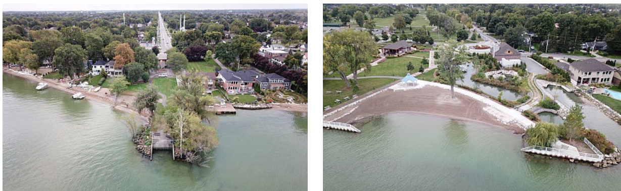
Figure 2.5 Oblique Photos at the foot of Lesperance Road and Manning Road
