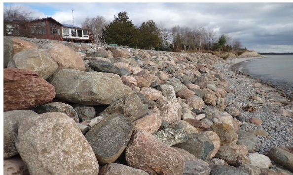
Crest elevation increased for an existing sloping rock structure.
