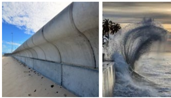
Recurved parapet wall added to seawall.
