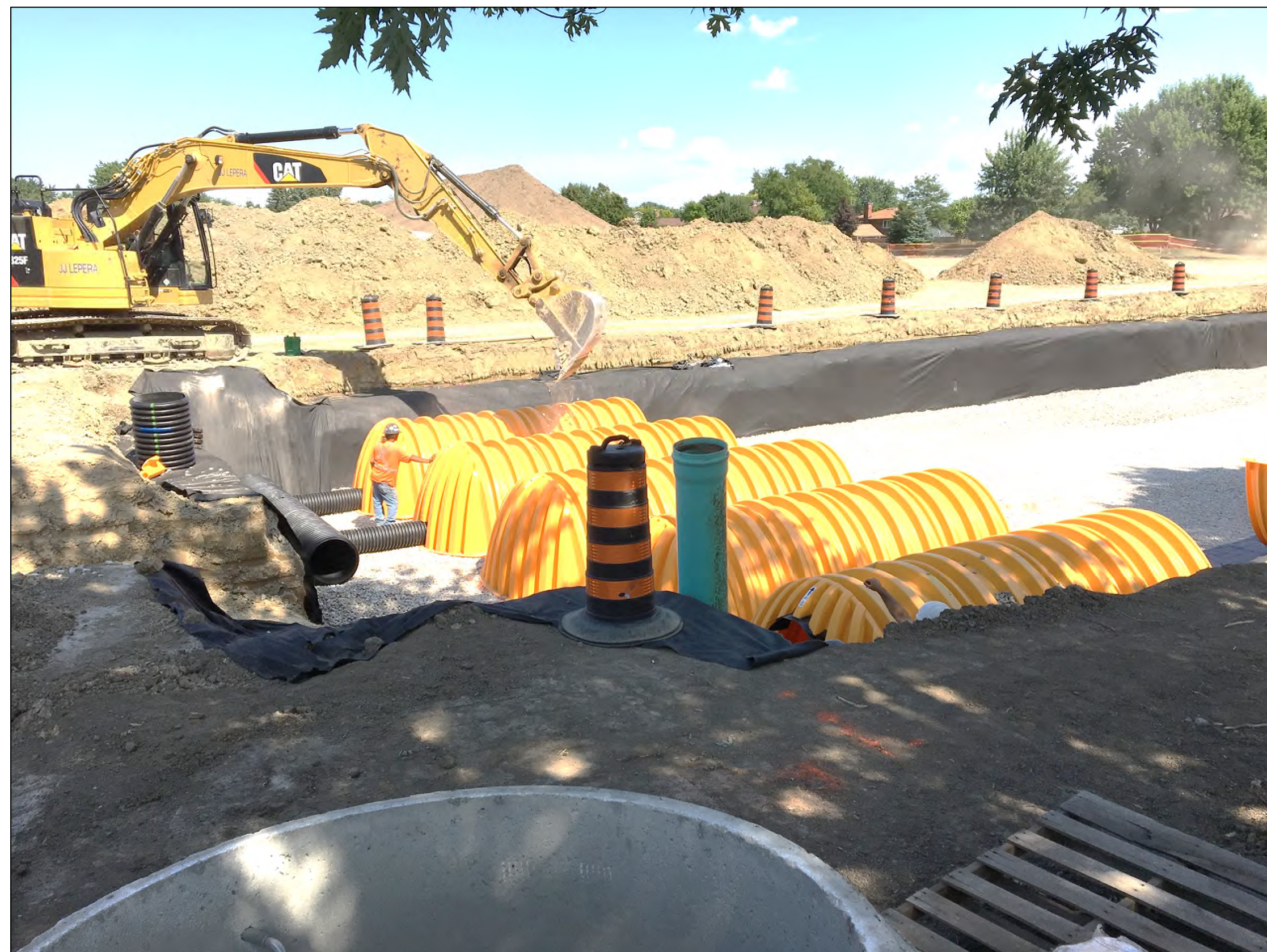
UNDERGROUND STORAGE CHAMBERS HIGH COST STORAGE ALTERNATIVE
