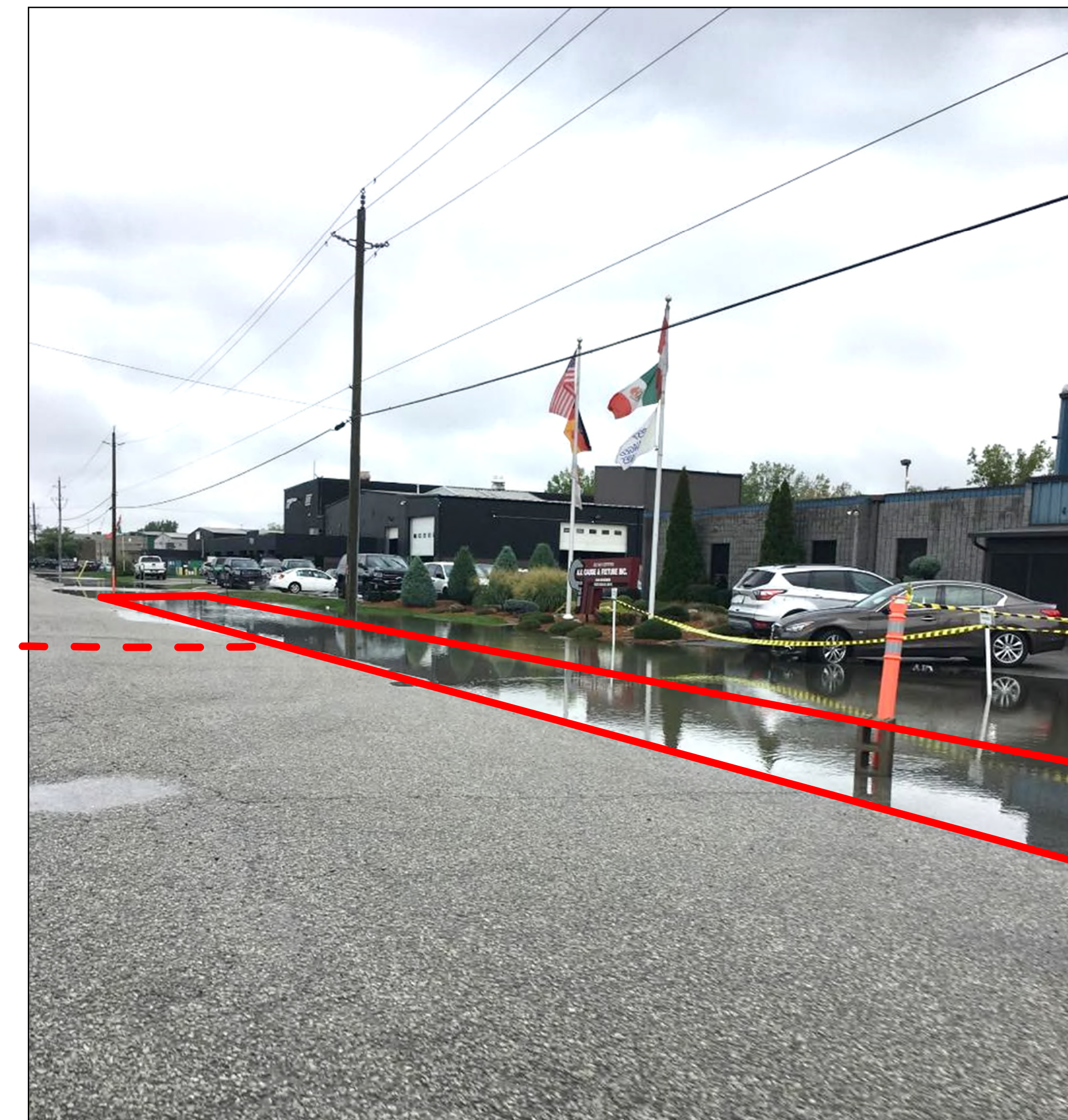
OBSERVED PONDING ON NORTH SIDE OF DELDUCA DRIVE
