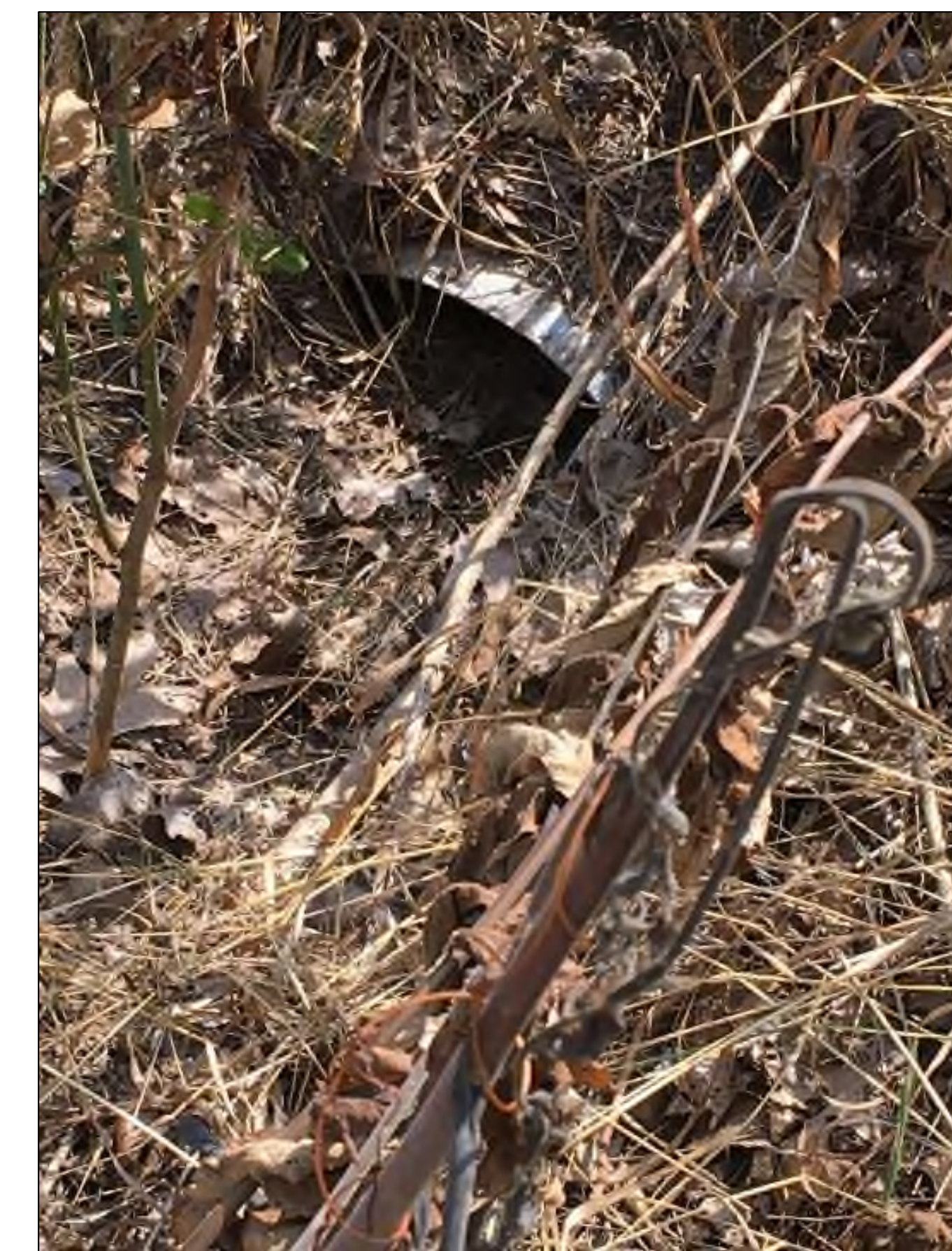
PLUGGED CULVERT
