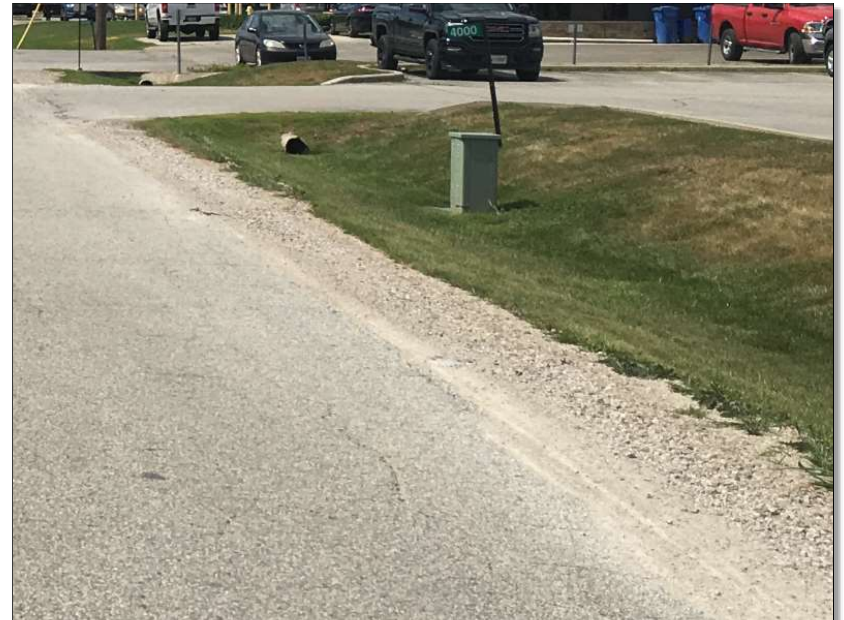
SWALE WITH DRIVEWAY CULVERT (TYPICAL)
