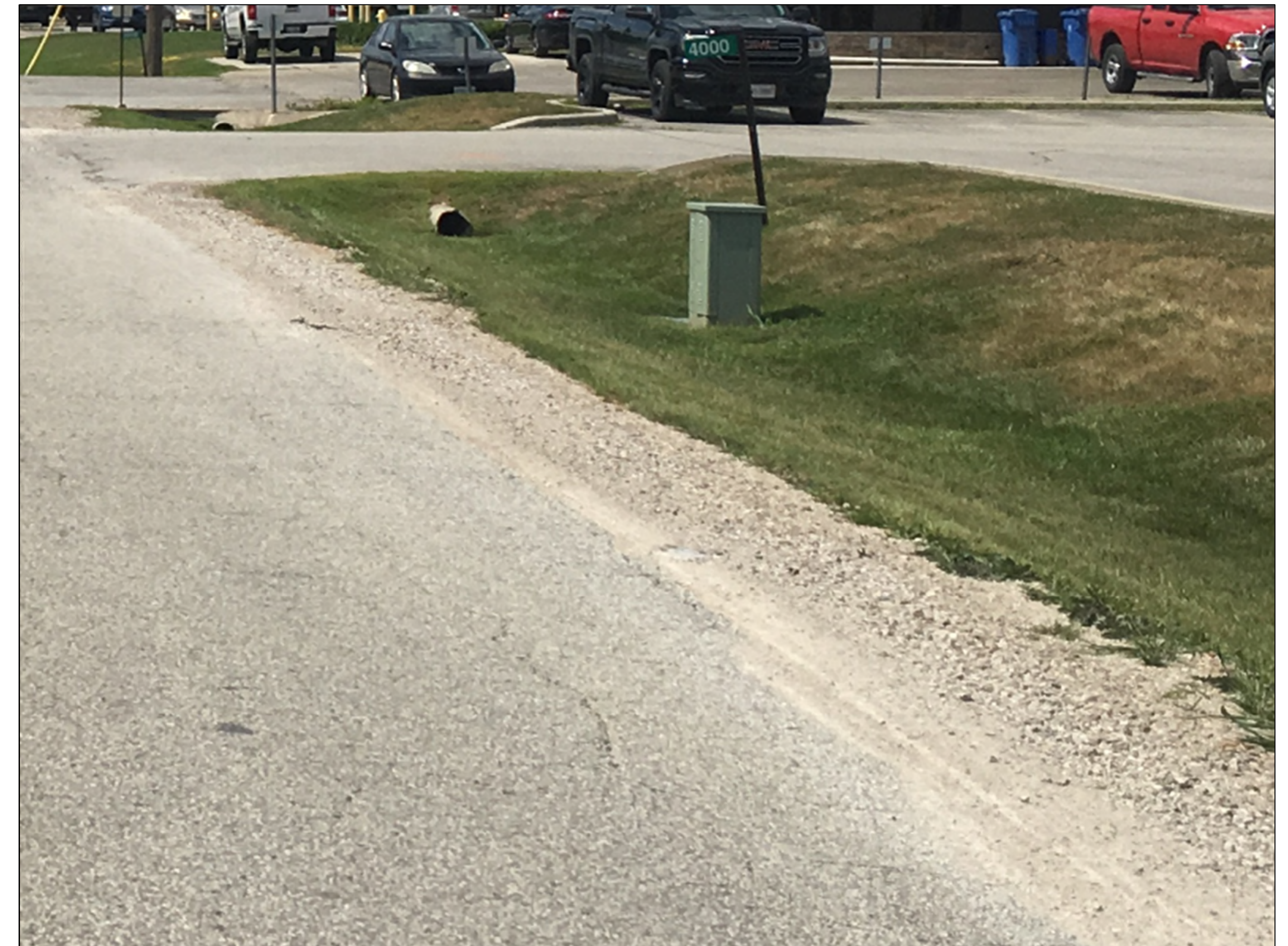
SWALE WITH DRIVEWAY CULVERT (TYPICAL)
