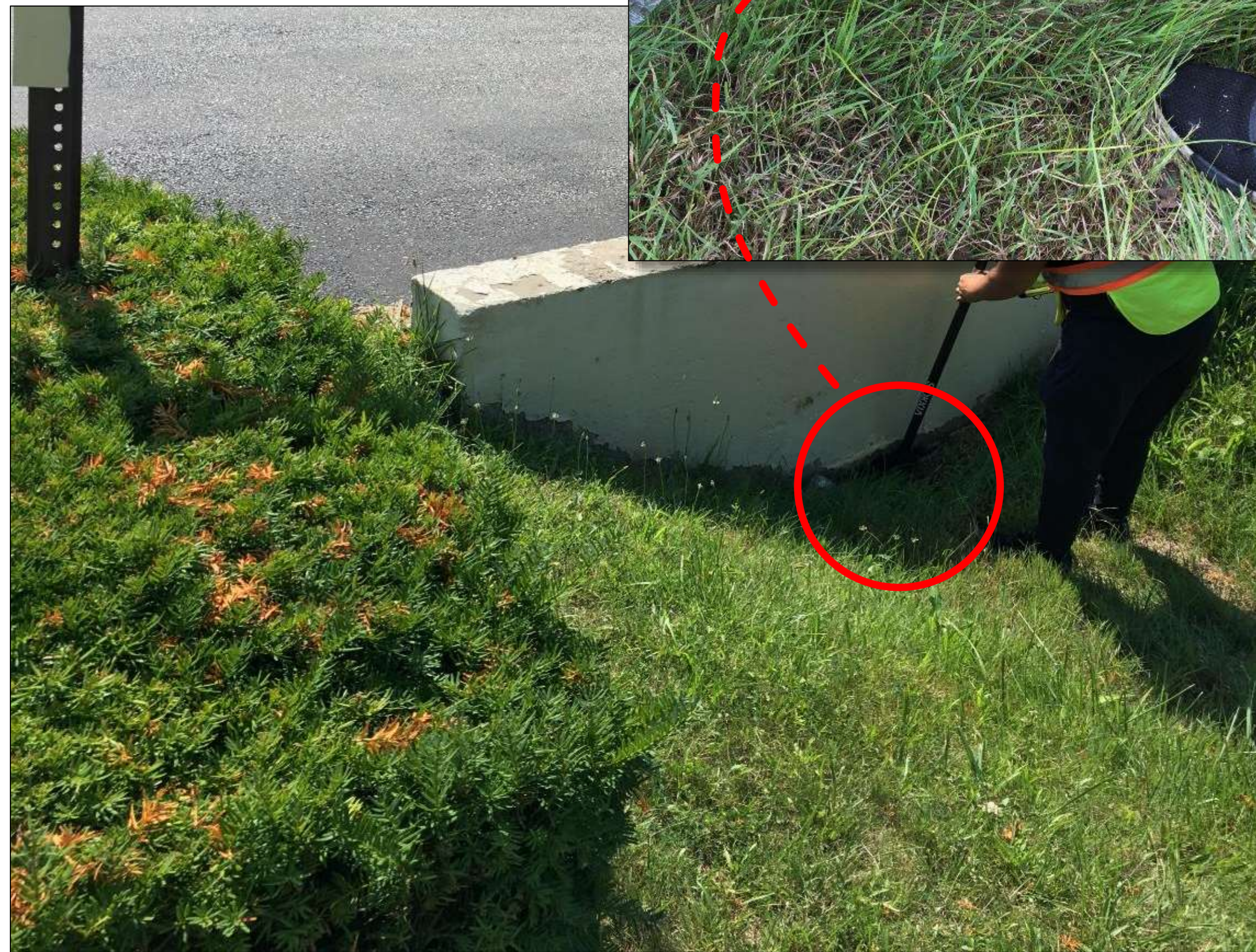
PLUGGED CULVERT
