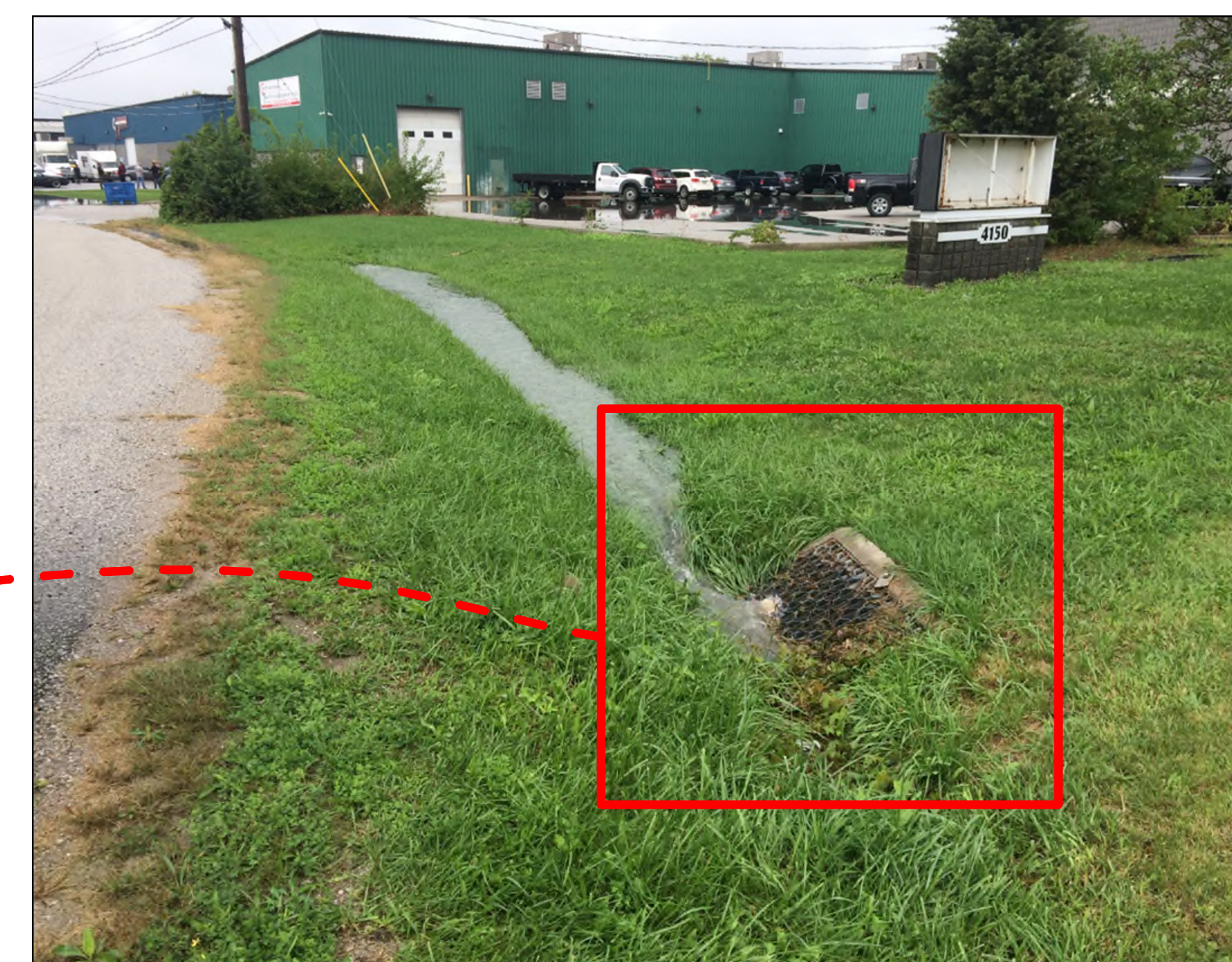
CATCH BASIN SOUTH EAST OF 4150 DELDUCA DRIVE
