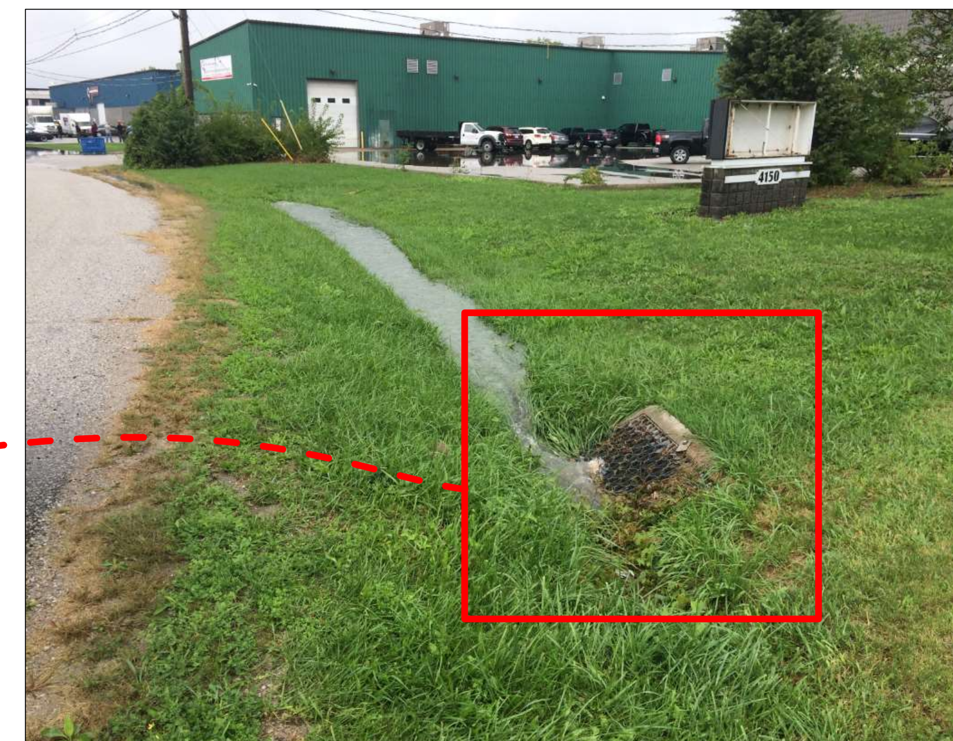
CATCH BASIN SOUTH EAST OF 4150 DELDUCA DRIVE
