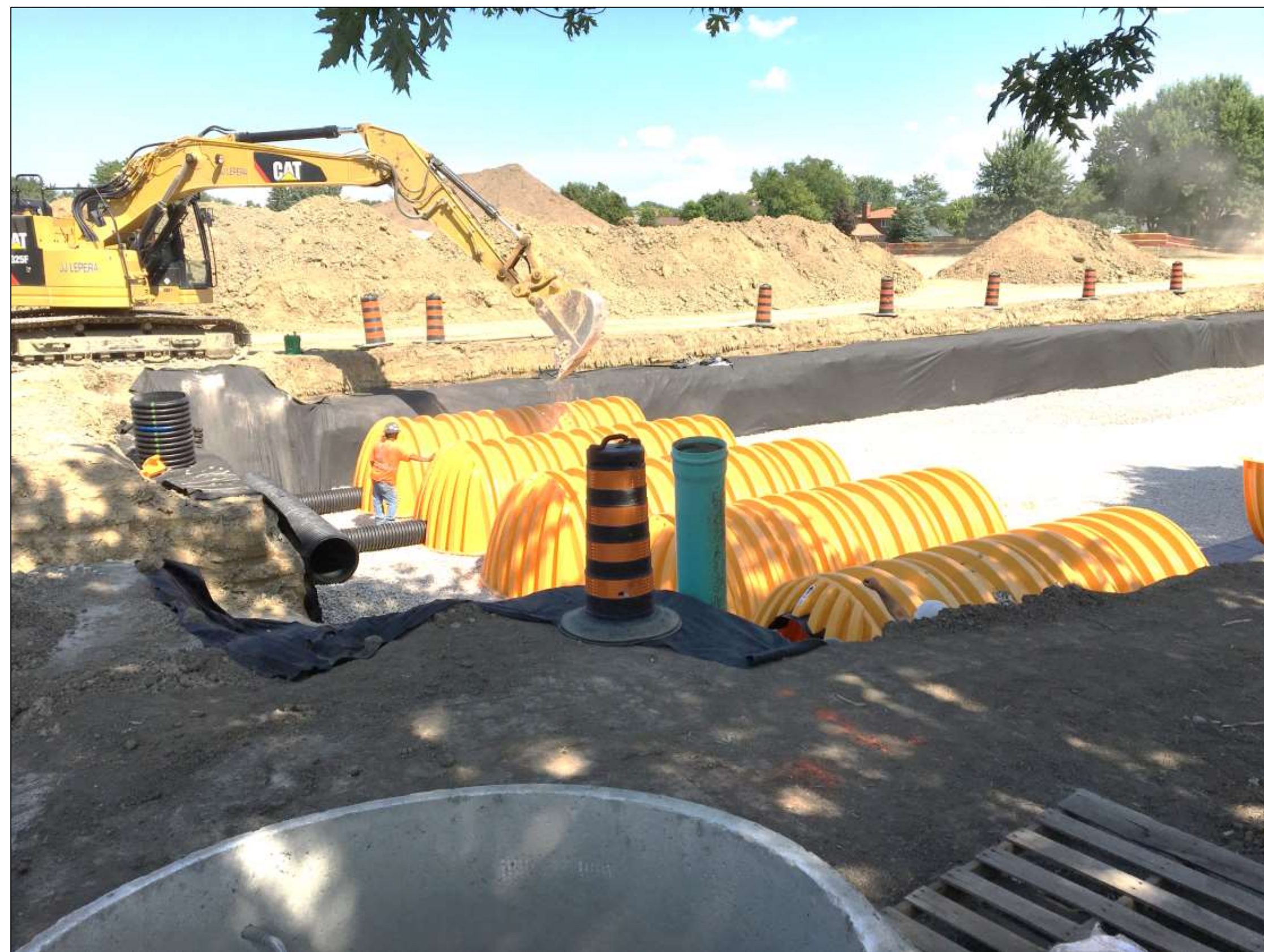
UNDERGROUND STORAGE CHAMBERS HIGH COST STORAGE ALTERNATIVE
