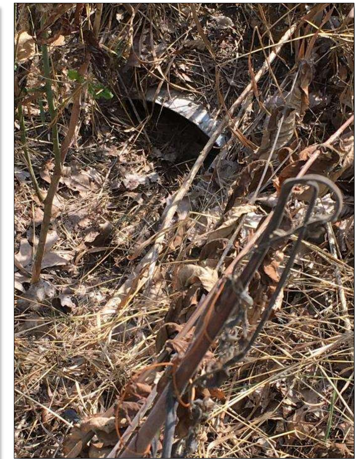
PLUGGED CULVERT
