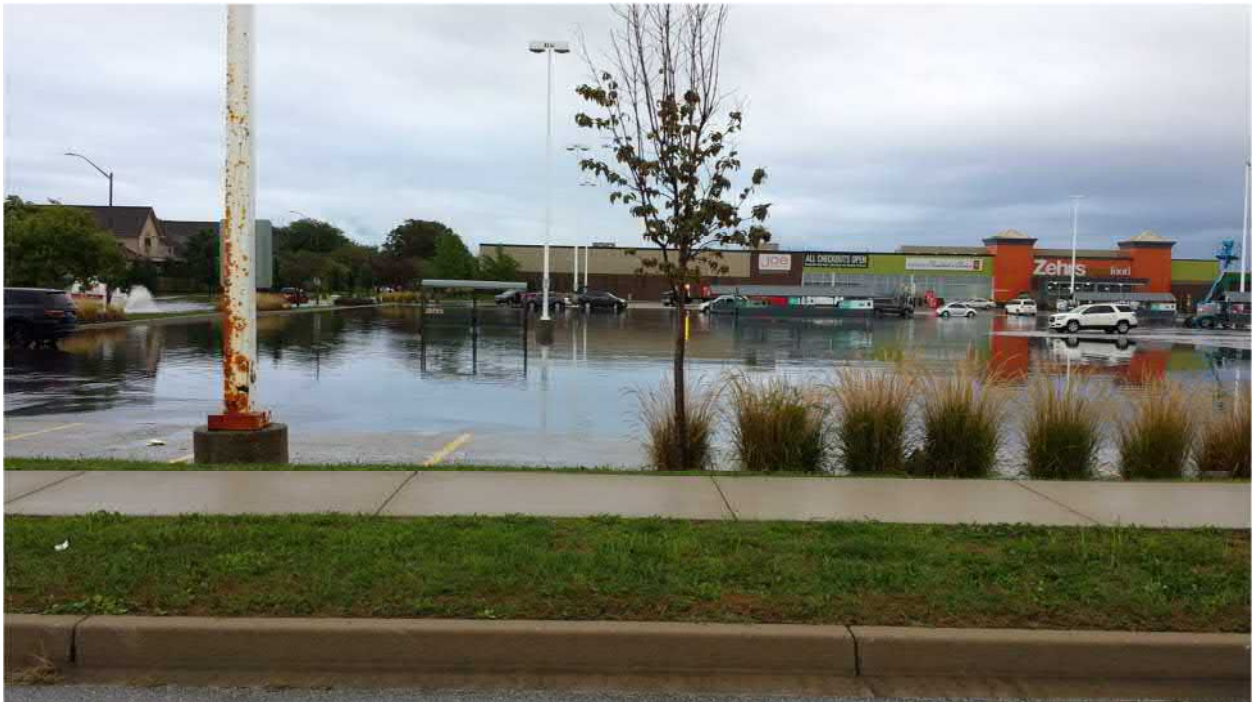
Surface flooding within Zehrs Grocery parking lot on Manning Rd. in Tecumseh, Ontario
