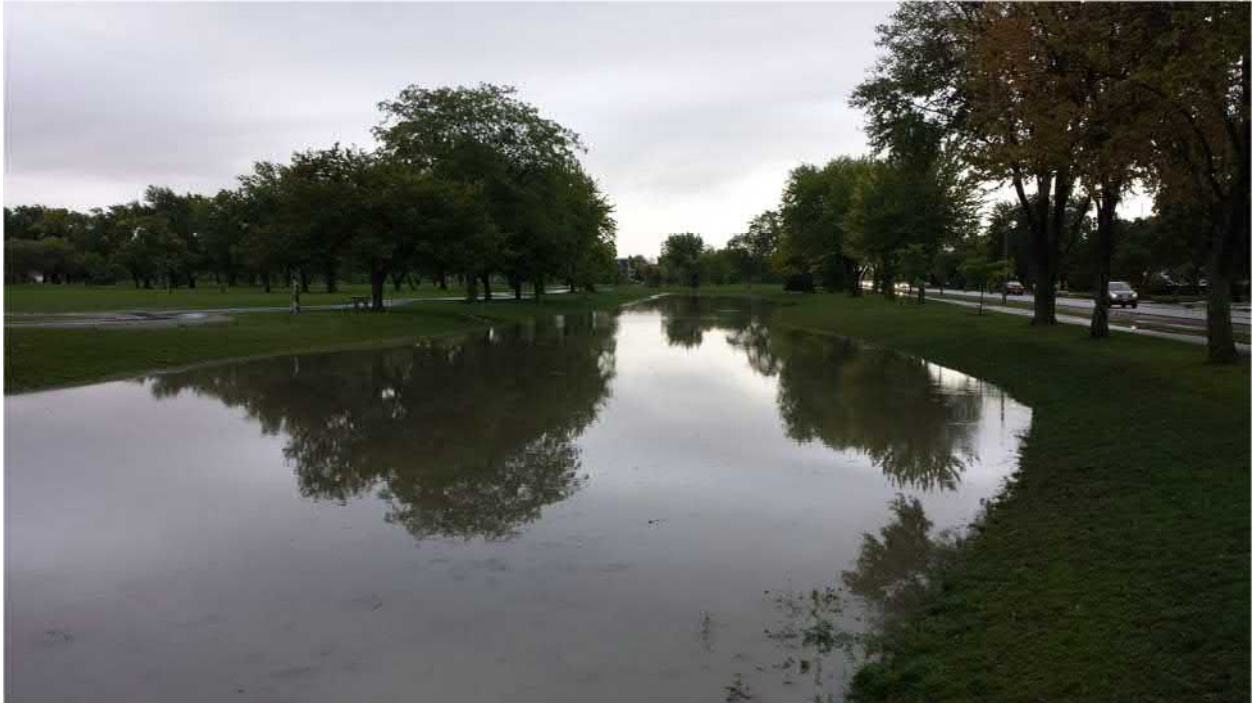
Lakewood Park Drainage Channel at bankfull East of Manning Rd. in Tecumseh, Ontario
