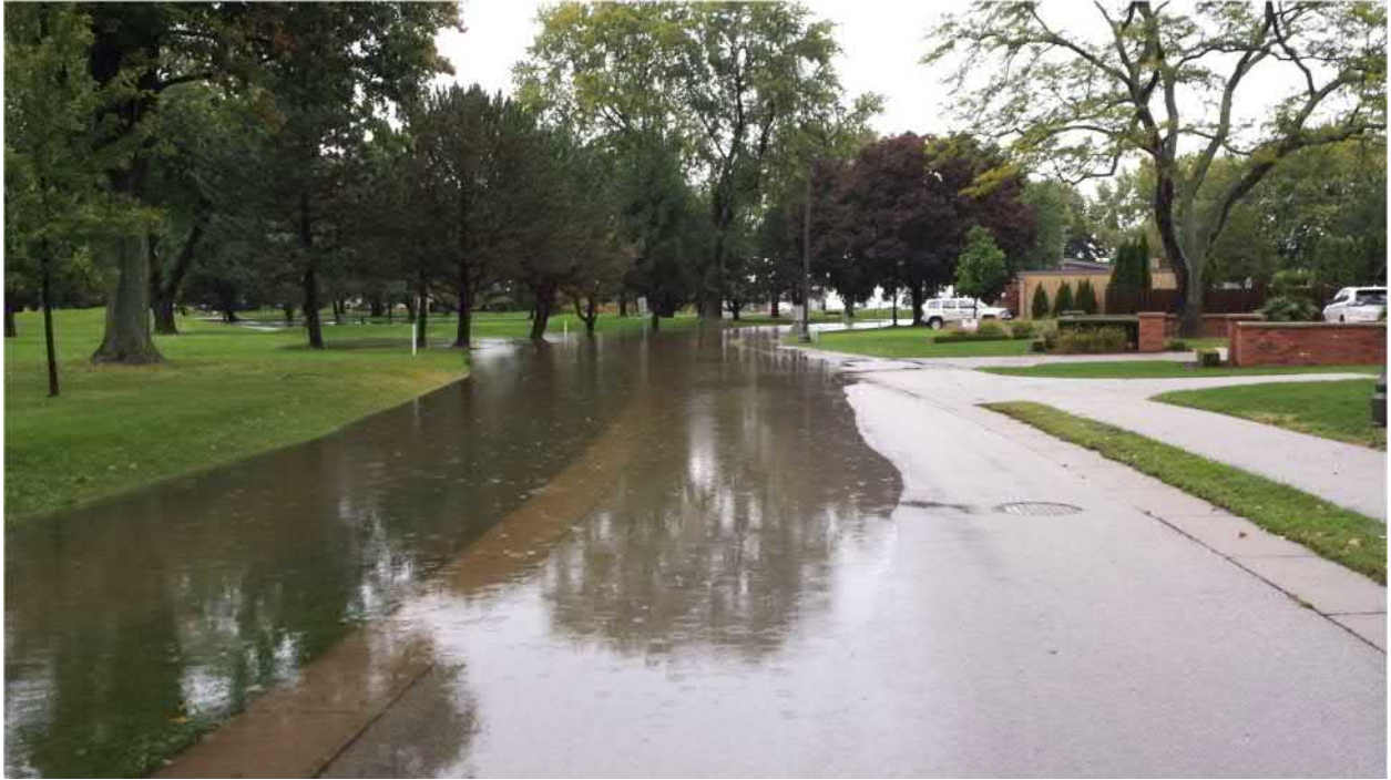
Surface flooding along Pentilly Rd. Facing North to Riverside Dr. in Tecumseh, Ontario
