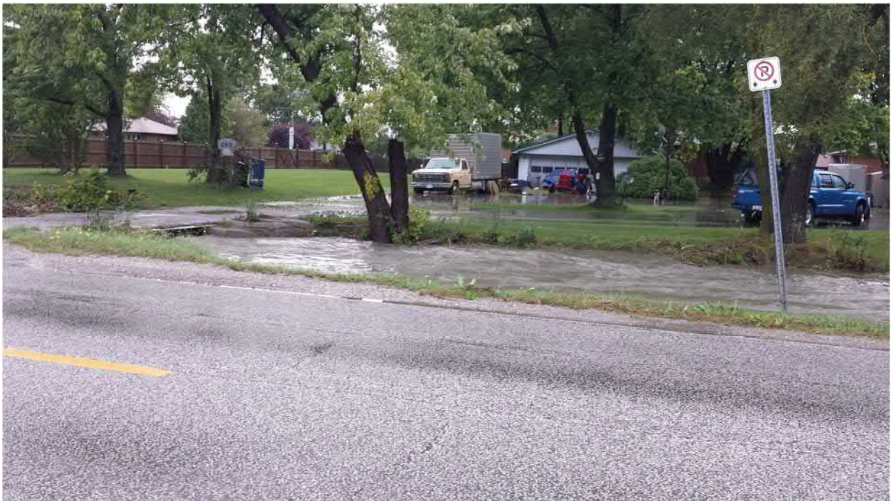
East Townline Municipal Drain at bankfull along Manning Rd. in Tecumseh, Ontario
