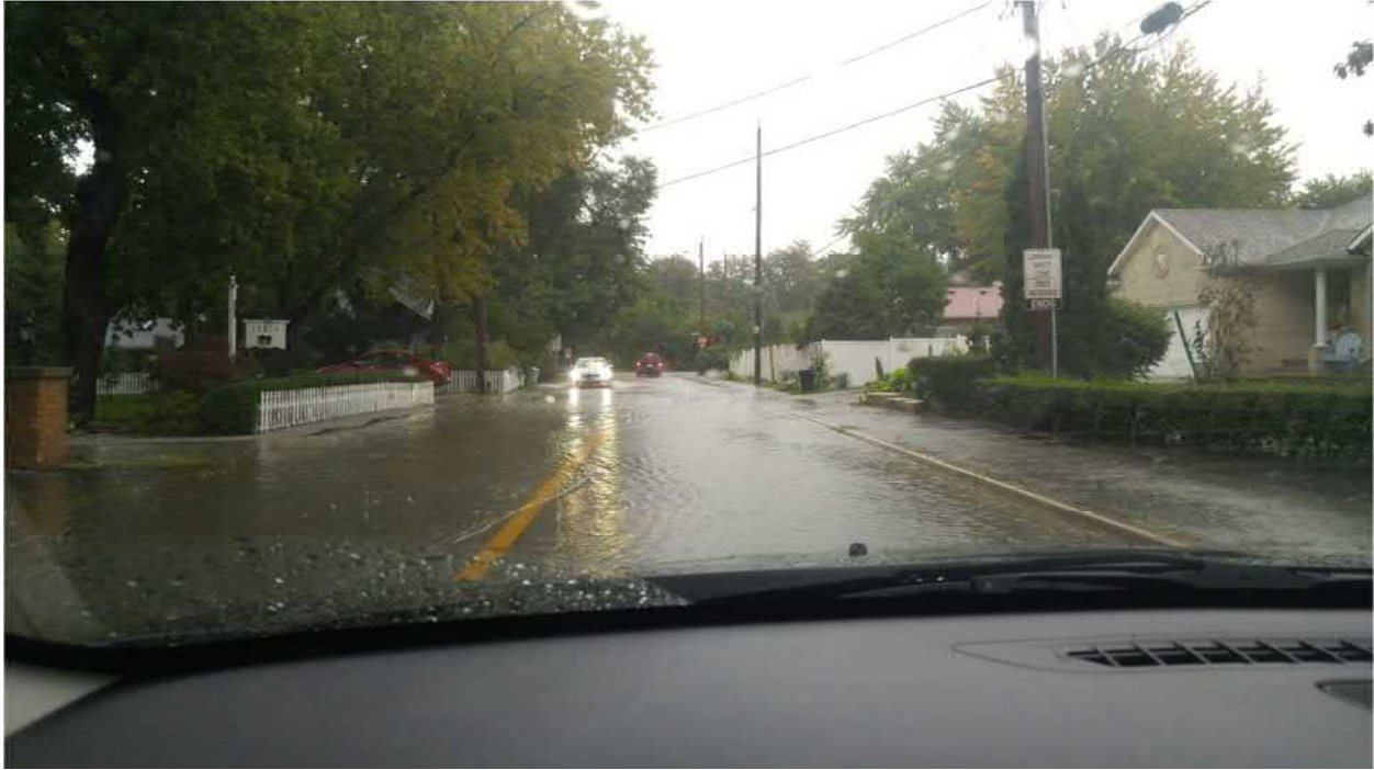
Surface flooding along St. Gregory's Rd. East of St. Marks Rd. in Tecumseh, Ontario
