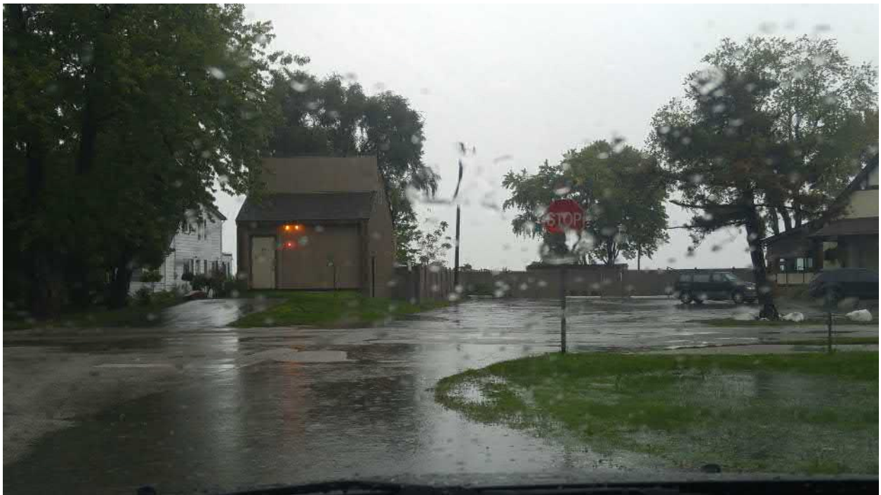
Surface flooding at the intersection of Kensington Blvd. and Riverside Dr. facing North at the Peter Cecile Storm Pump Station in Tecumseh, Ontario
